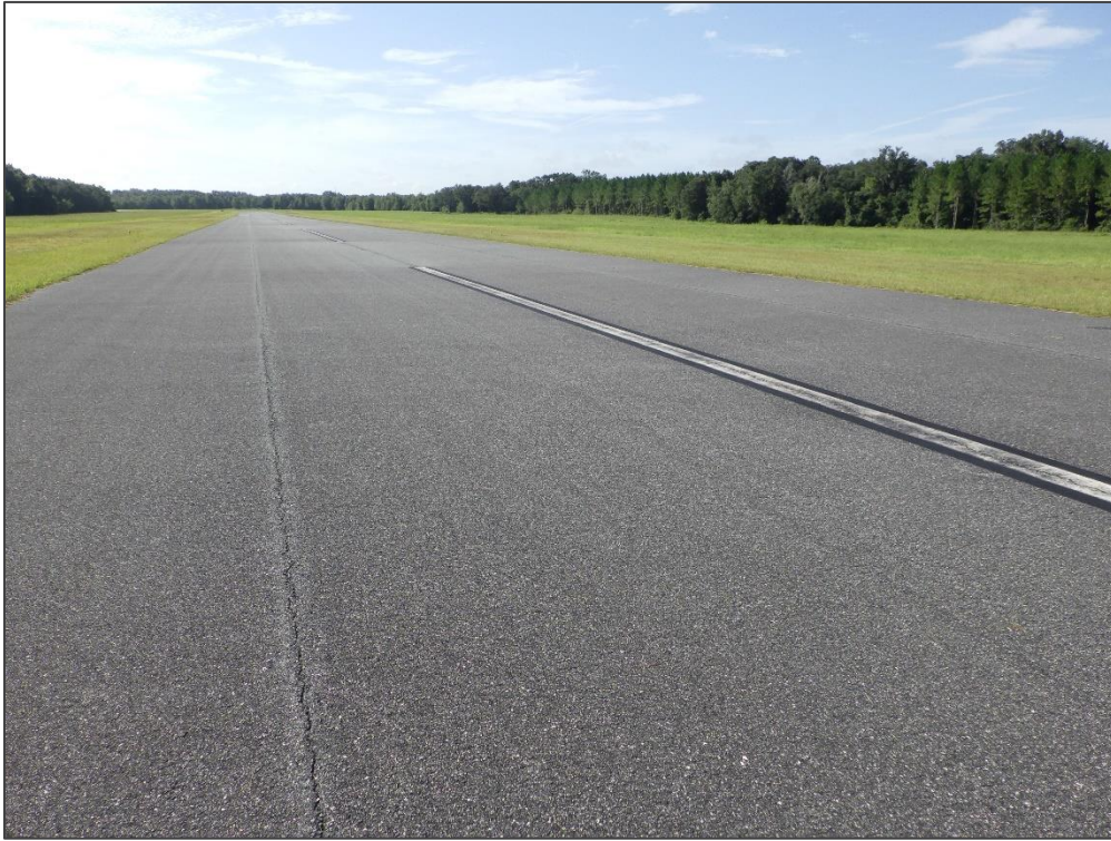
RW 14-32, Section 6215, Sample Unit 322 – Longitudinal & Transverse Cracking
