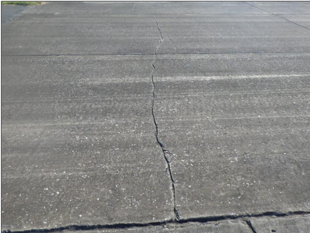
RW 14-32, Section 6205, Sample Unit 303 – Linear Cracking
