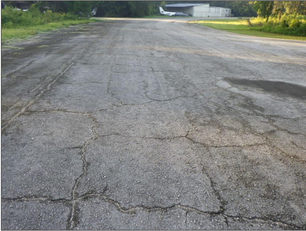
TW G, Section 450, Sample Unit 113 – Block Cracking
