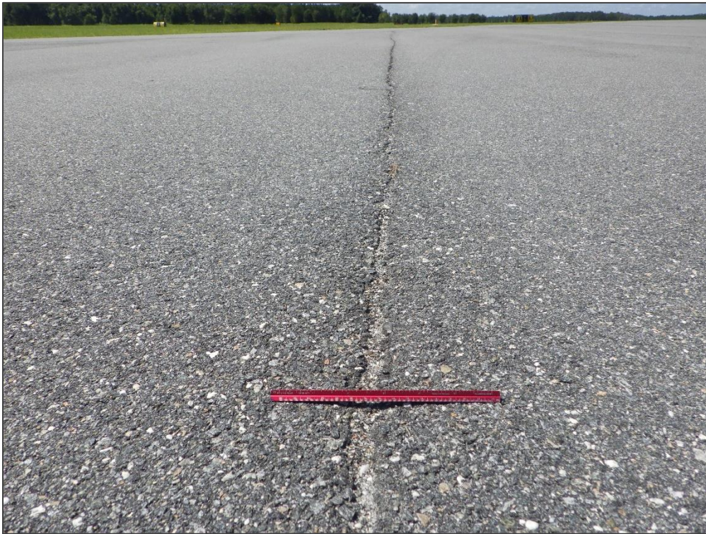
AP, Section 4110, Sample Unit 601 – Longitudinal & Transverse Cracking
