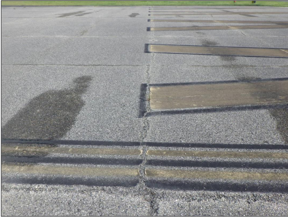
RW 5-23, Section 6112, Sample Unit 304 – Joint Reflection Cracking
