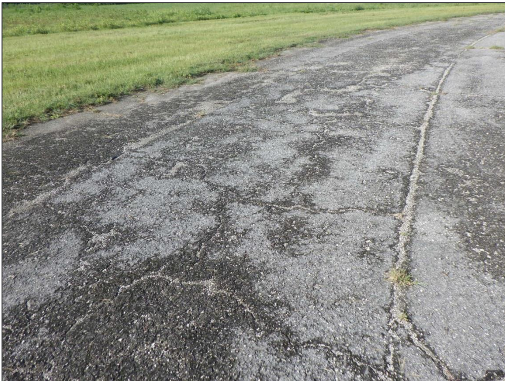
TW F, Section 550, Sample Unit 145 – Block Cracking and Raveling
