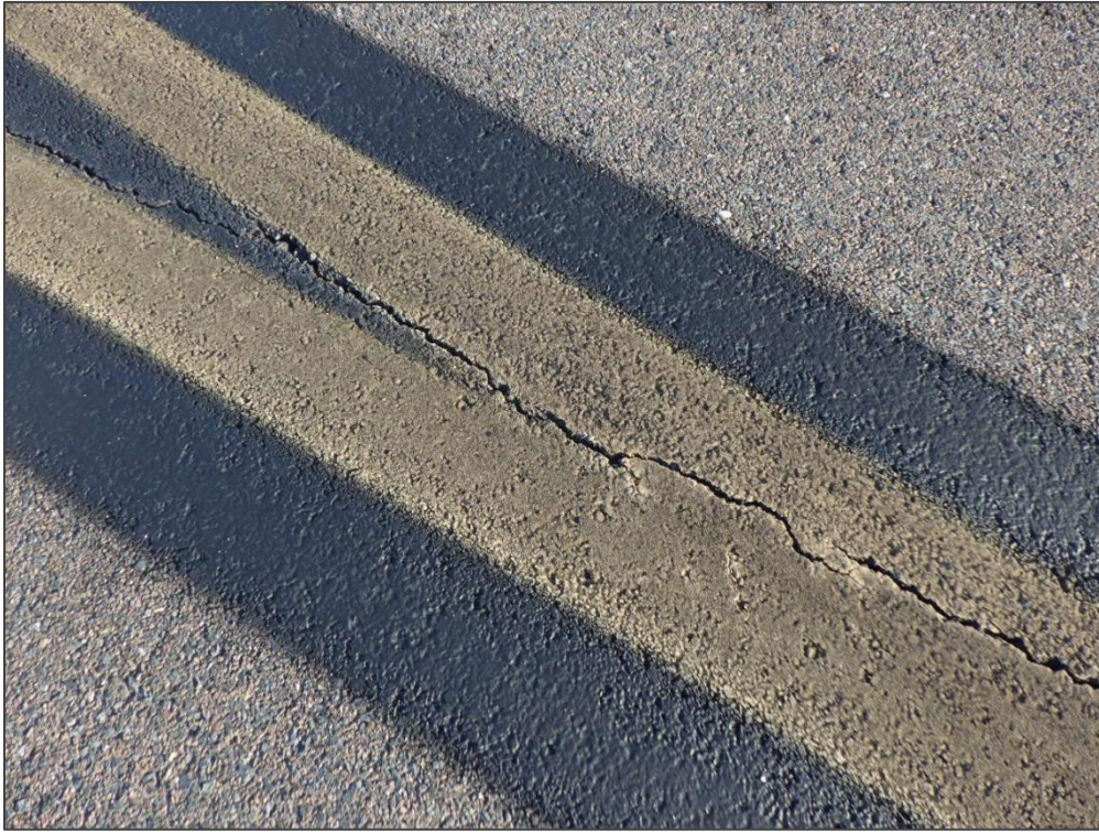
TW D, Section 505, Sample Unit 103 – Longitudinal & Transverse Cracking
