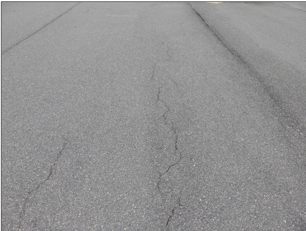
AP, Section 4110, Sample Unit 554 – Longitudinal & Transverse Cracking
