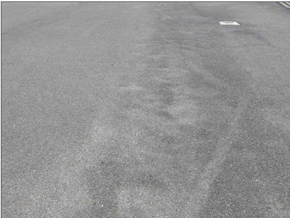
AP HANG, Section 4205, Sample Unit 100 – Swelling
