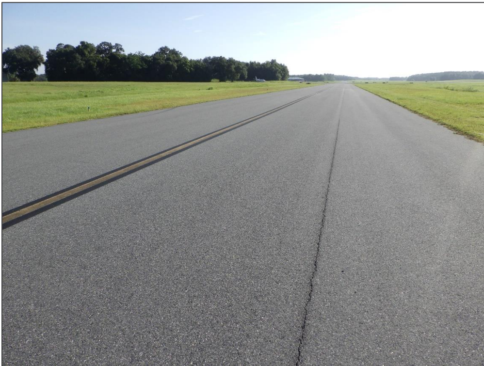
TW A, Section 205, Sample Unit 164 – Longitudinal & Transverse Cracking
