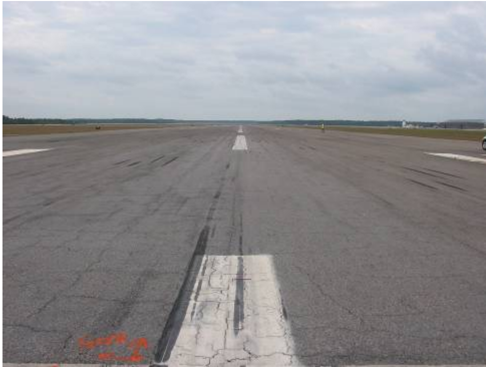
RW 18R-36L Section 6115 SU 205: Low Severity Block Cracking (May 2, 2007)
