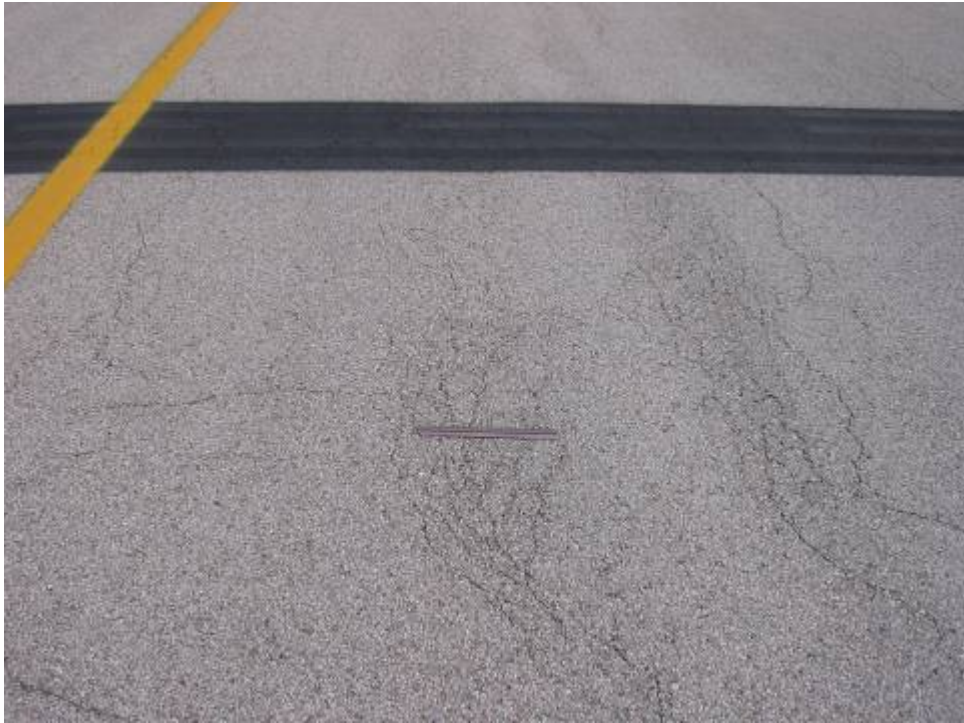
TW A Section 120 SU 305: Low Severity Alligator Cracking (May 2, 2007)
