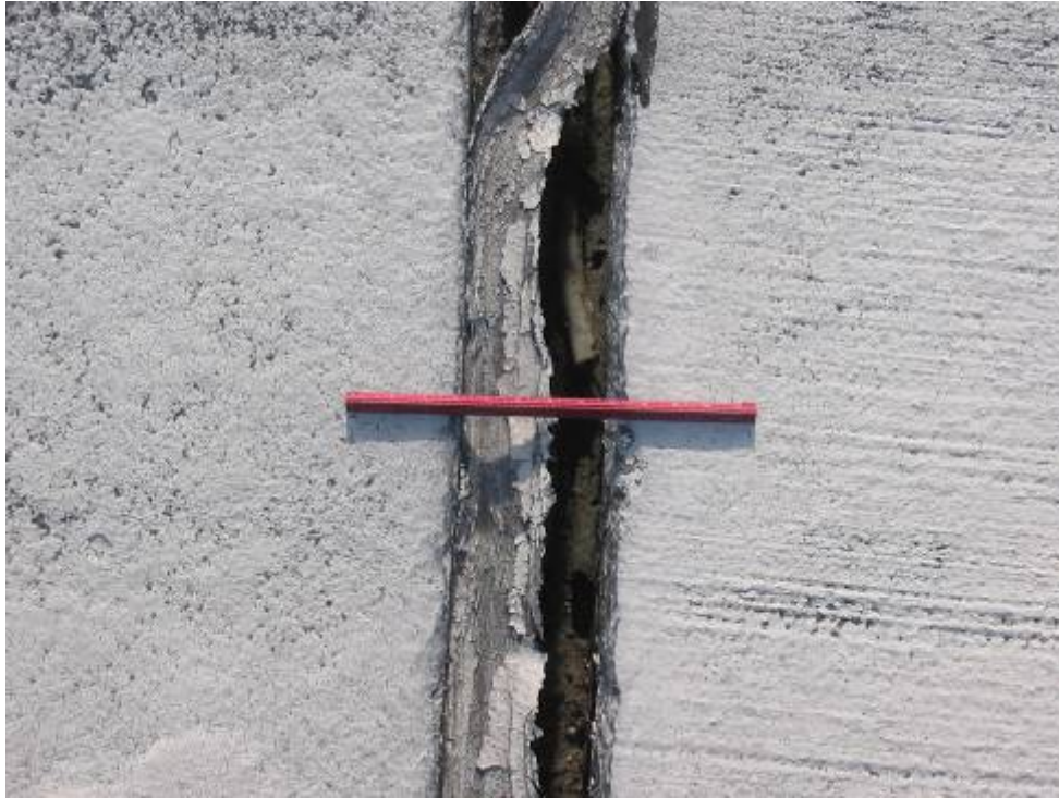
RW 18R-36L Section 6105 SU 200: High Severity JT Seal Damage (May 2, 2007)
