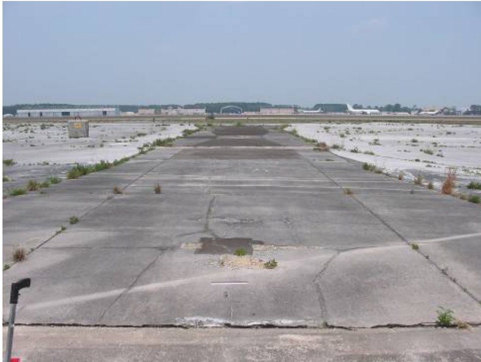
AP ENG TST Section 5210 SU 200: Medium Severity Shattered Slabs (May 2, 2007)
