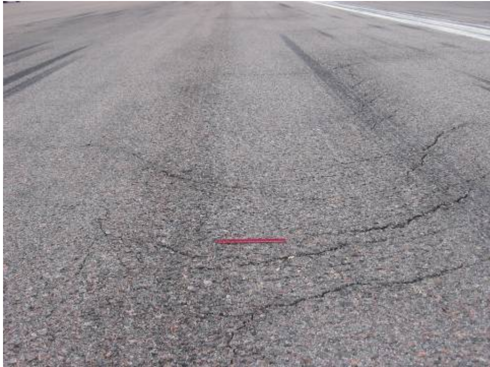
RW 18R-36L Section 6115 SU 311: Low Severity Slippage Cracking (May 2, 2007)
