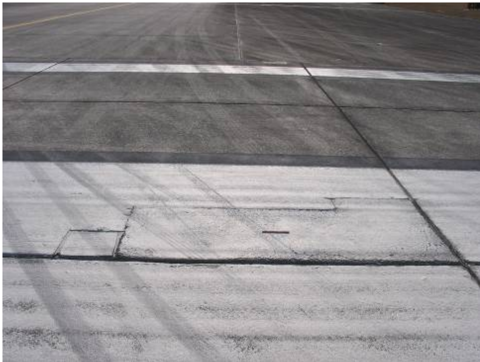
RW 18R-36L Section 6110 SU 401: Low Severity Small and Large Patch (May 2, 2007)
