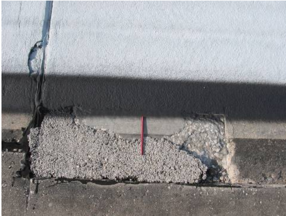
RW 18R-36L Section 6105 SU 200: Medium Severity Small Patch (May 2, 2007)
