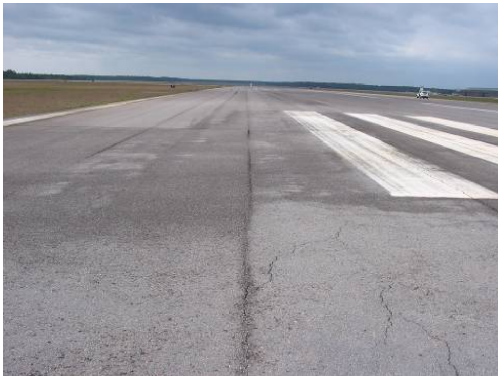
RW 18R-36L Section 6120 SU 408: Medium Severity L/T Cracking (May 2, 2007)
