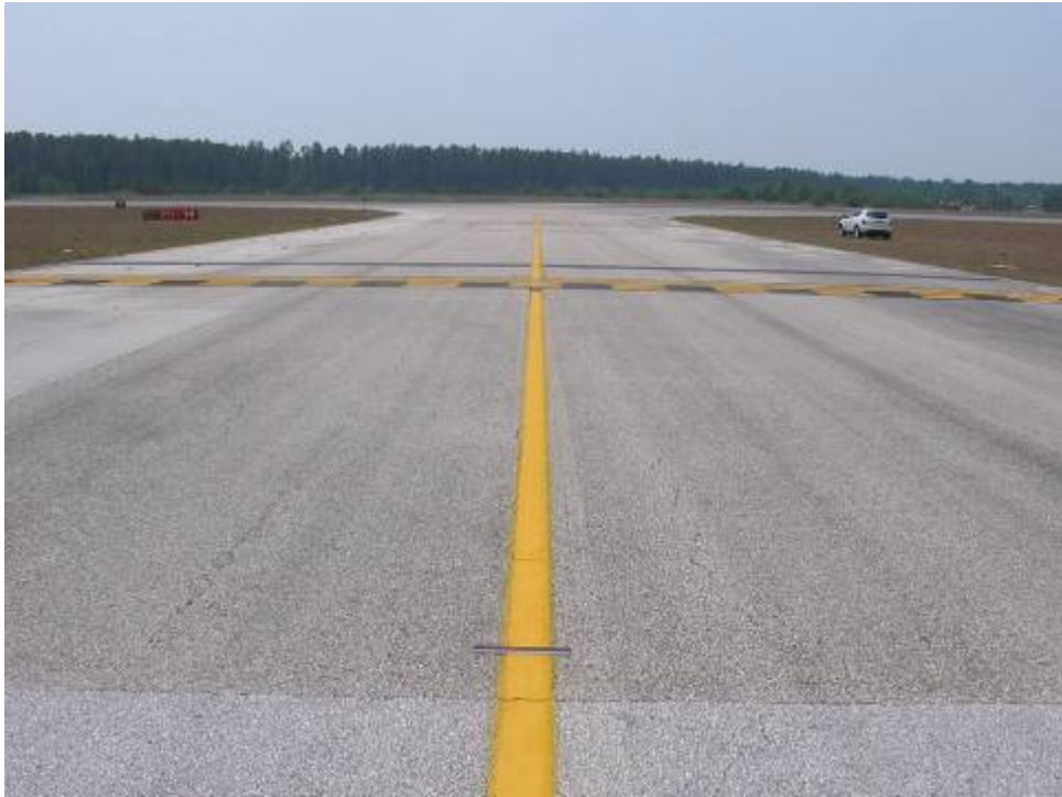
TW B2 Section 1205 SU 200: Low Severity L/T Cracking (May 2, 2007)
