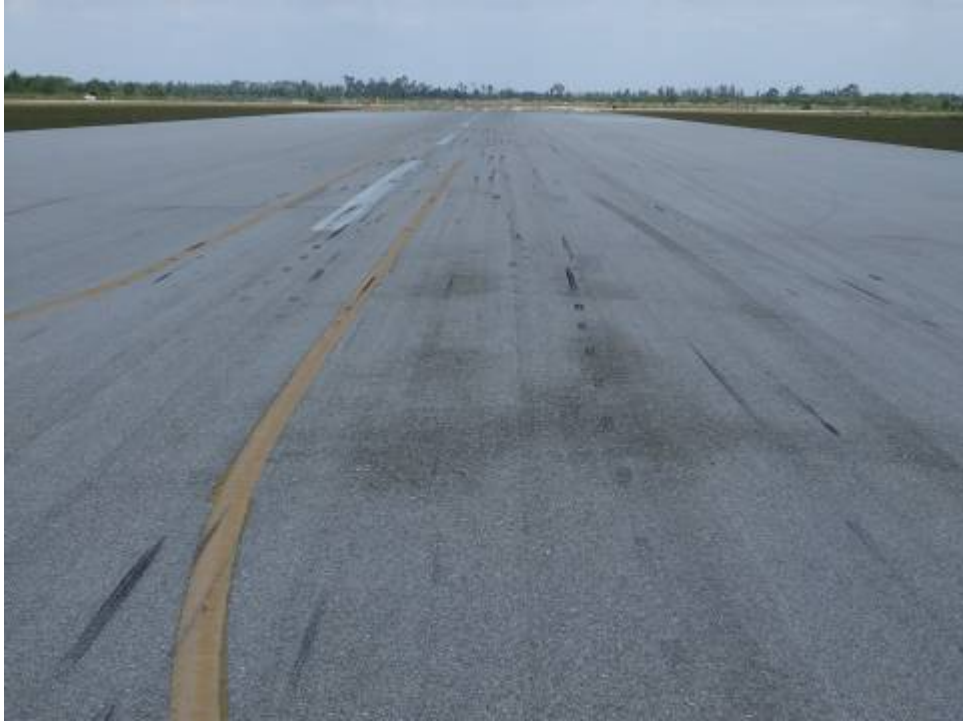
RW 15-33 Section 6210 SU 348: Low Severity L/T Cracking (December 11, 2006)
