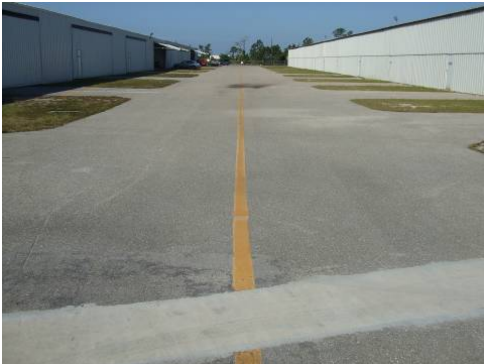
TW 4 N T-HANG Section 505 SU 300: Overview, Low Severity Patching (December 11, 2006)
