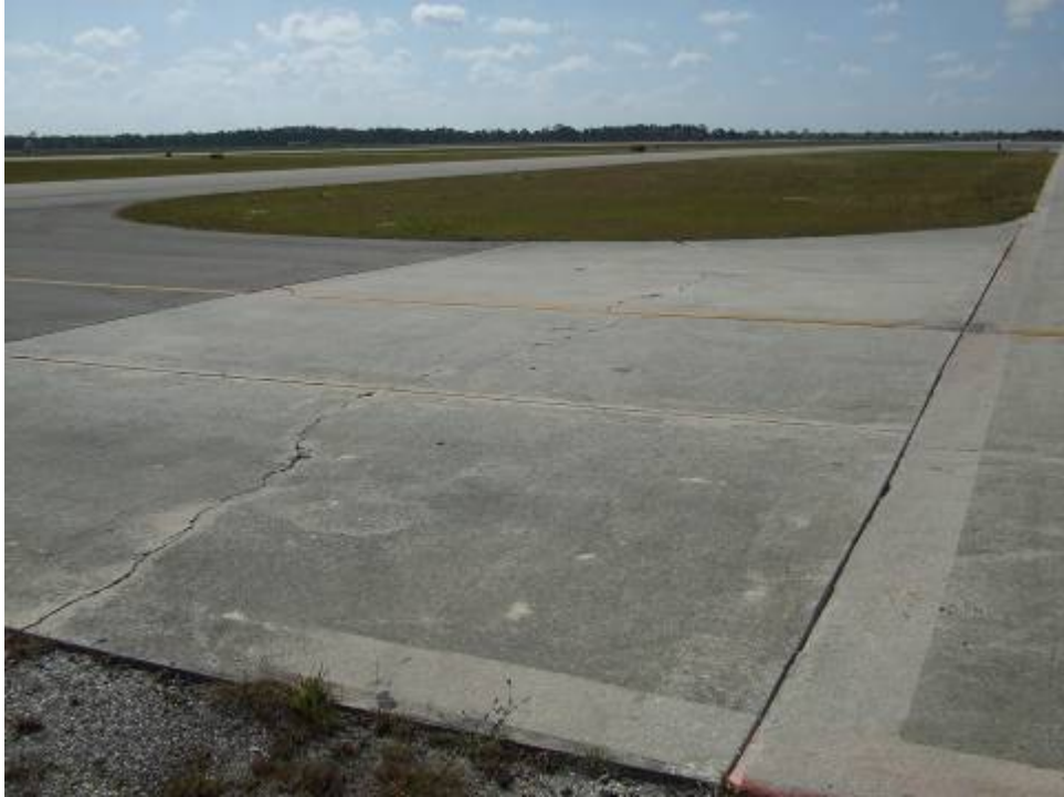
TW D Section 198 SU 102: Medium Severity Linear Cracking (December 11, 2006)
