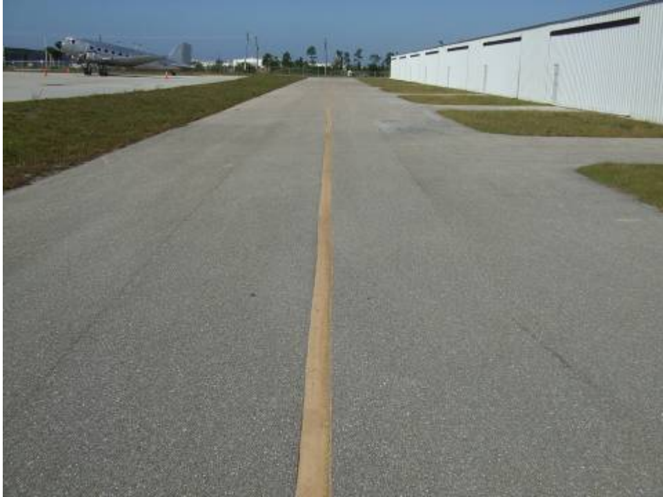
TW 5 N T-HANG Section 405 SU 200: Low Severity L/T Cracking (December 11, 2006)
