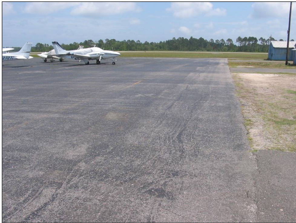
AP S Section 4110: Medium Severity Weathering (May 10, 2007)
