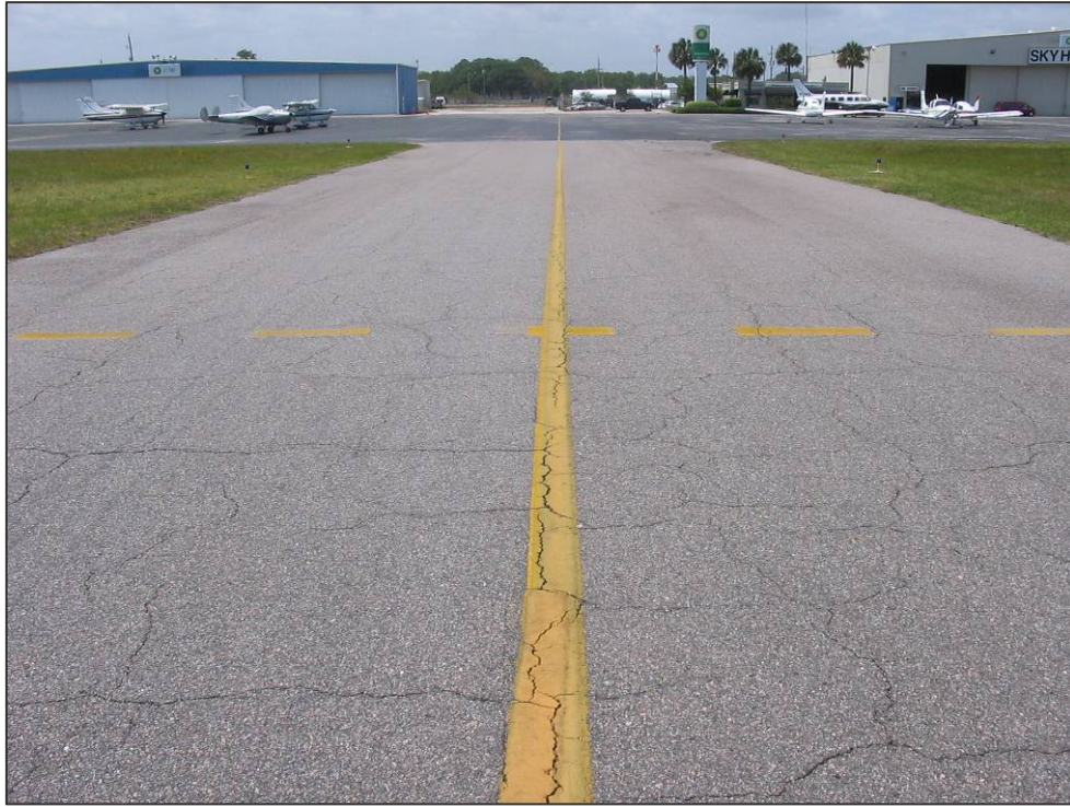
TW D& K Section 405: Low Severity Block Cracking (May 10, 2007)
