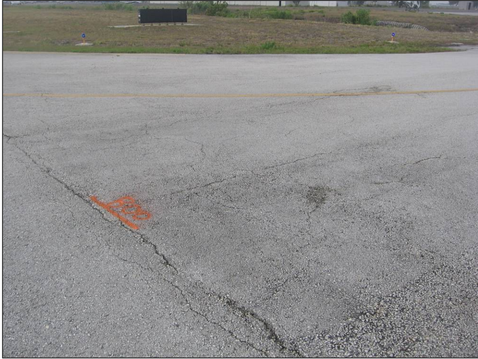
TW H Section 805 SU 800: Low Severity Block Cracking (May 10, 2007)
