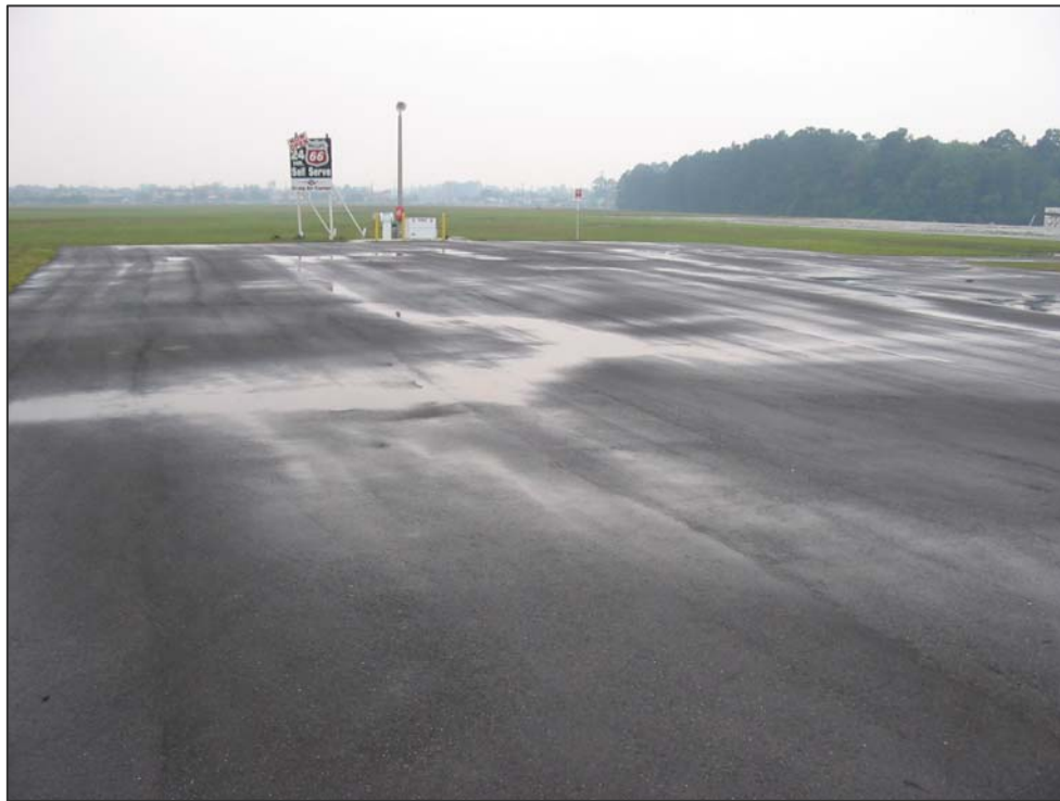
AP SW Section 4420: Low Severity Linear/Transverse Cracking (May 9, 2007)
