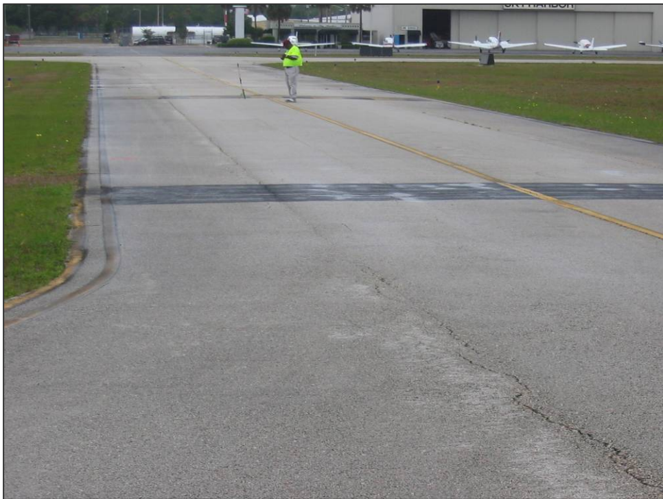
TW D& K Section 420: Medium Severity Linear/Transverse Cracking (May 9, 2007)
