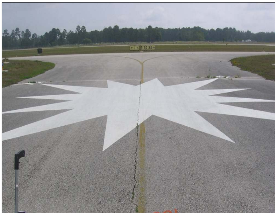
TW J Section 1010: Medium Severity Linear/Transverse Cracking (May 10, 2007)
