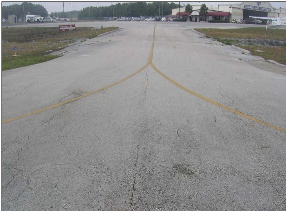
TW H Section 805: Low Severity Block Cracking (May 10, 2007)
