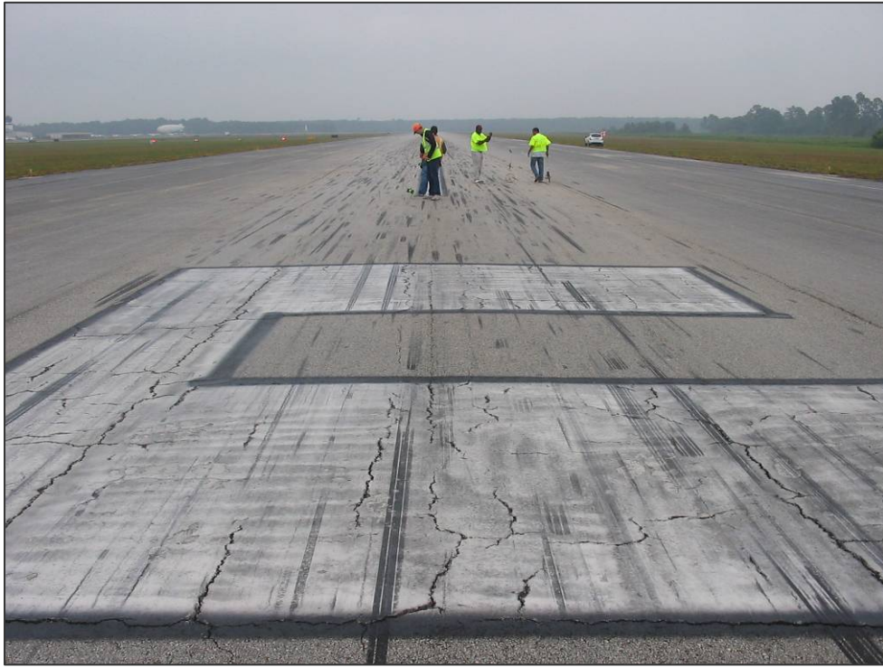
RW 5-23 Section 6105: Medium Severity L/T Cracking (May 9, 2007)
