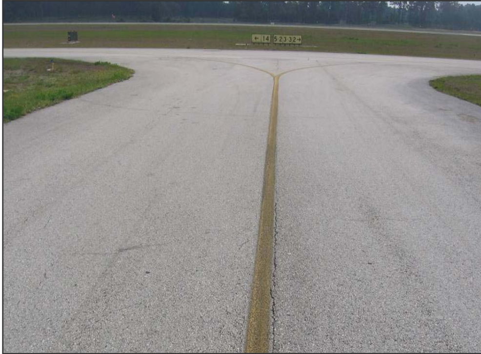
TW G Section 705: Low Severity Linear/Transverse Cracking (May 10, 2007)
