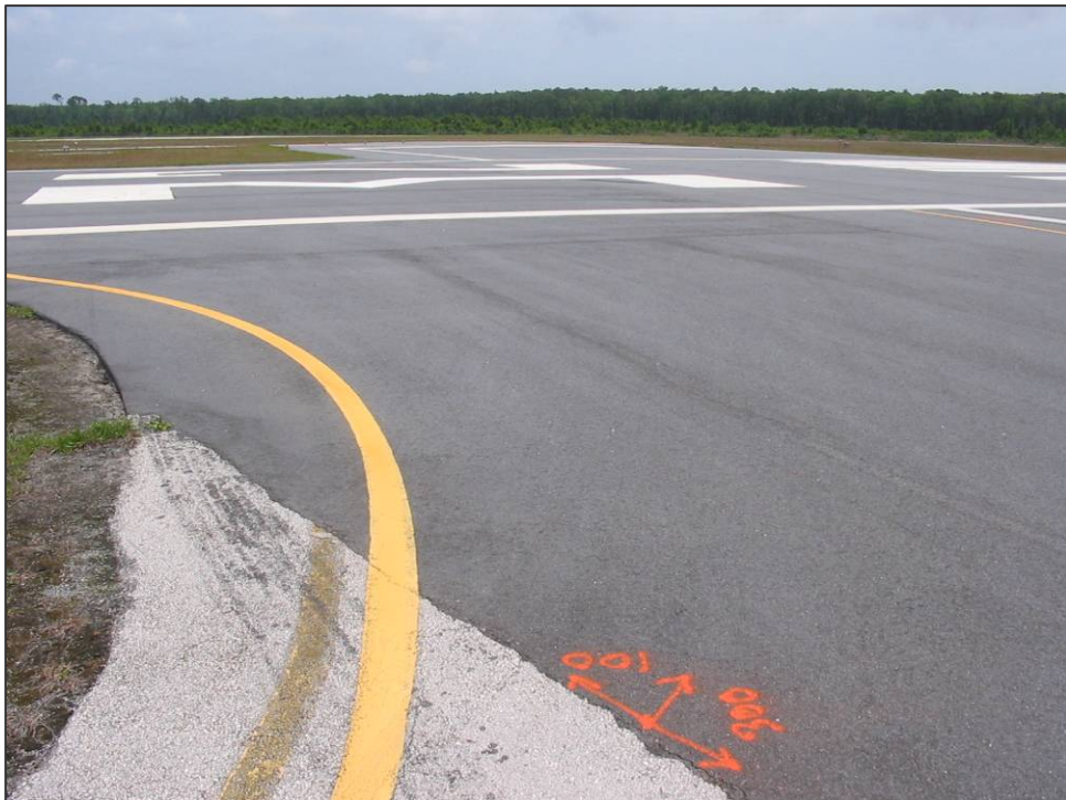
TW C Section 315: Low Severity Linear/Transverse Cracking (May 10, 2007)
