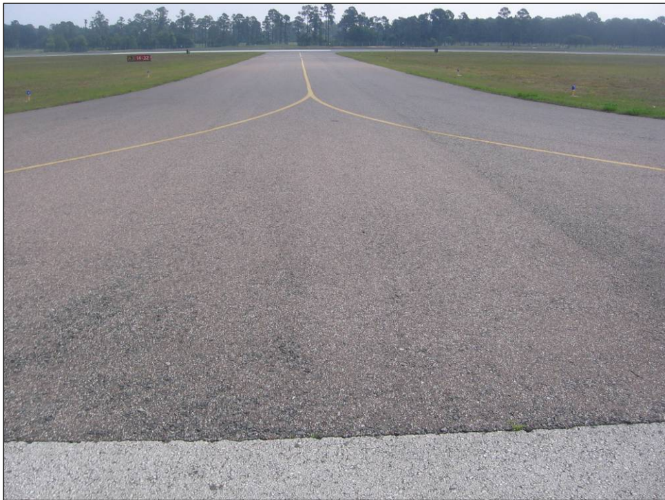
TW H Section 810: Low Severity Weathering (May 10, 2007)
