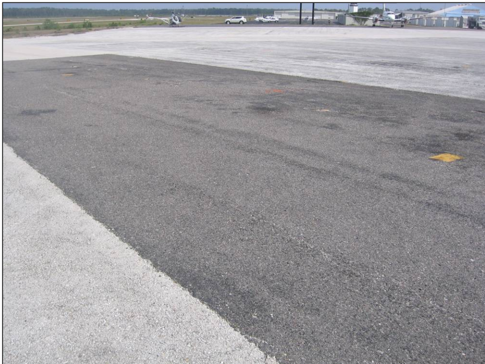
AP NW Section 4310: Low Severity Weathering (May 10, 2007)
