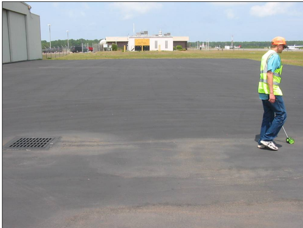
AP S Section 4115: Low Severity Linear/Transverse Cracking (May 10, 2007)
