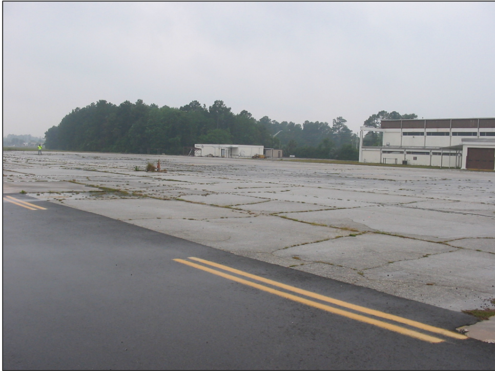
AP SW Section 4425: Medium Severity Block Cracking (May 9, 2007)
