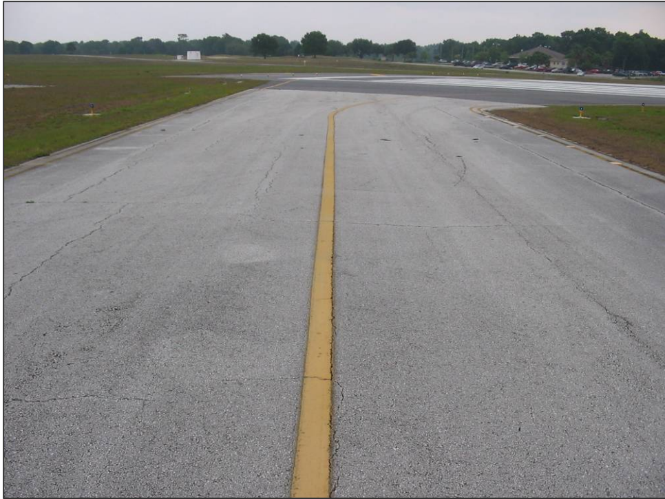
TW A Section 110: Low Severity Linear/Transverse Cracking (May 10, 2007)
