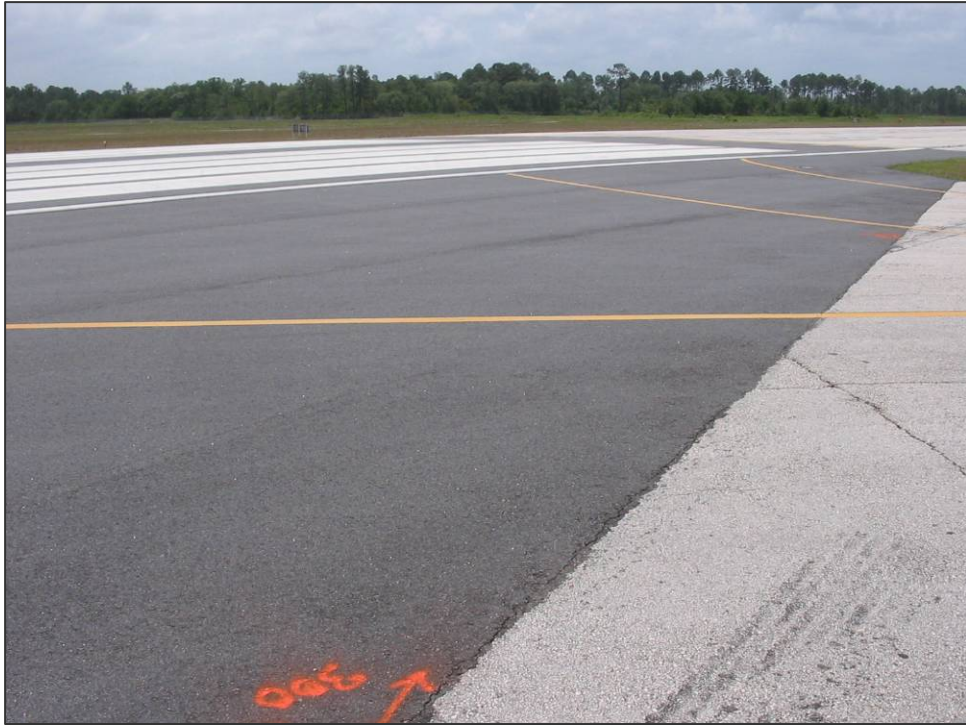
TW C Section 310: Low Severity Linear/Transverse Cracking (May 10, 2007)
