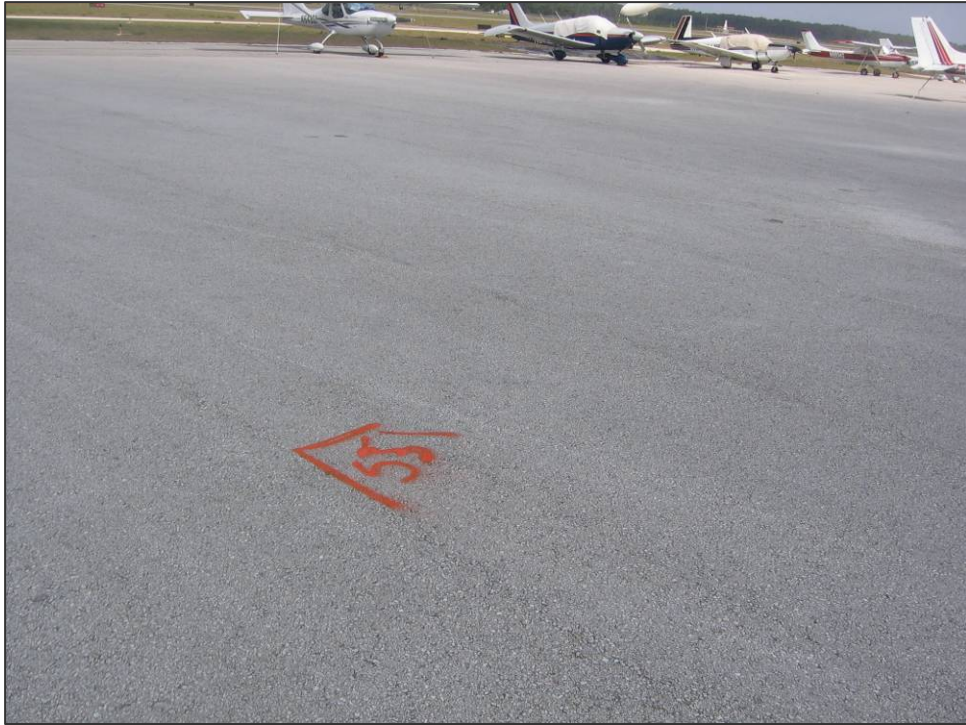
AP NW Section 4305: Low Severity Weathering (May 10, 2007)
