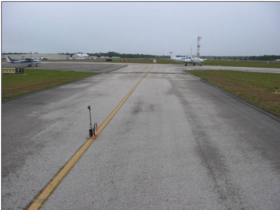
TW F Section 605: Low Severity Linear/Transverse Cracking (May 9, 2007)
