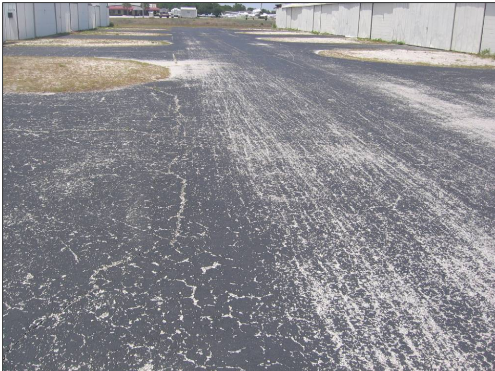
AP N Section 4215 SU 102: Medium Severity Weathering (May 10, 2007)
