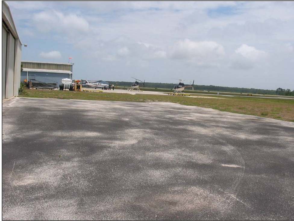
AP SW Section 4410: Low Severity Weathering (May 10, 2007)
