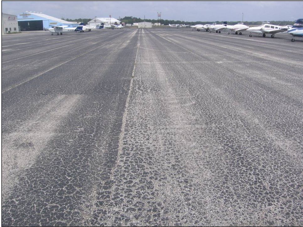
AP N Section 4210: Medium Severity Weathering (May 10, 2007)
