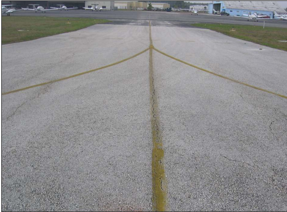
TW B Section 210: Low Severity Linear/Transverse Cracking (May 10, 2007)
