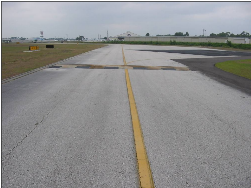
TW A Section 105: Low Severity Linear/Transverse Cracking (May 10, 2007)
