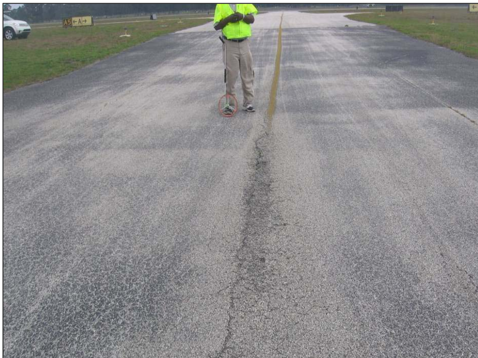
TW B Section 205 SU 201: Medium Severity Linear/Transverse Cracking (May 10, 2007)
