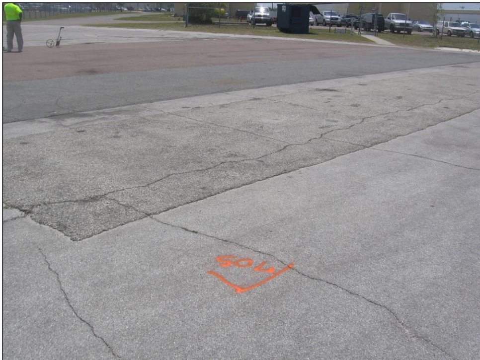
AP N Section 4205 SU 705: Medium Severity Block Cracking (May 10, 2007)
