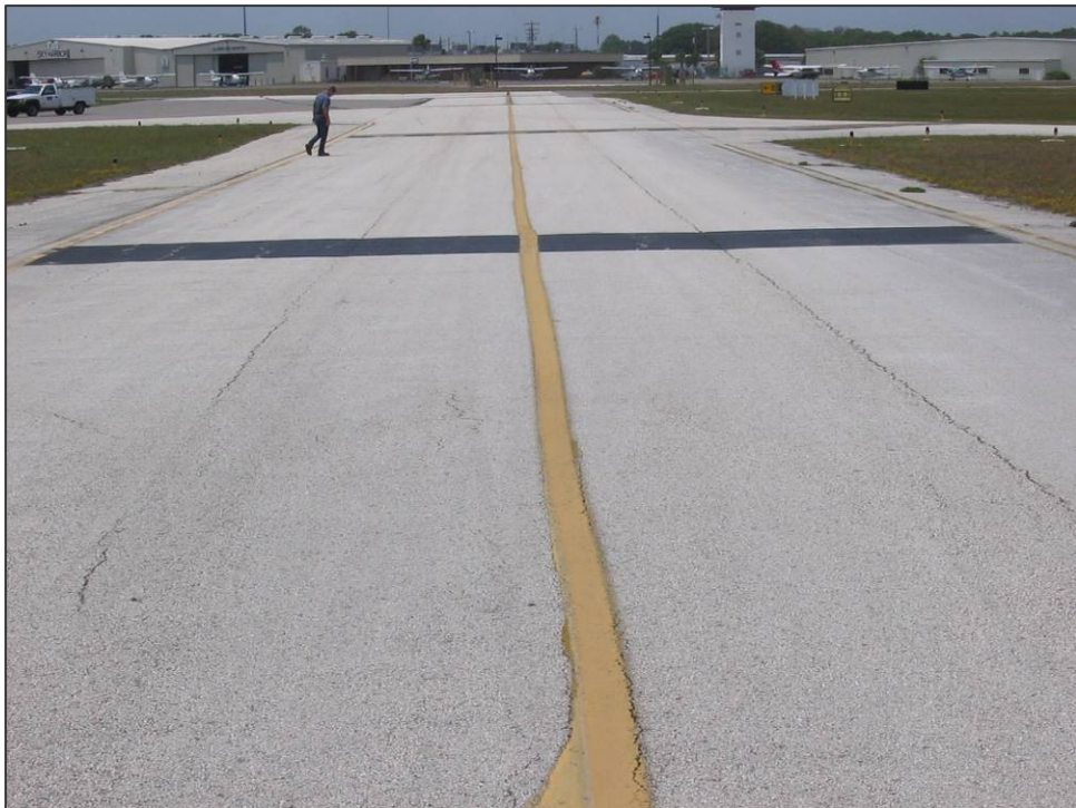
TW C Section 305: Low Severity Linear/Transverse Cracking (May 10, 2007)
