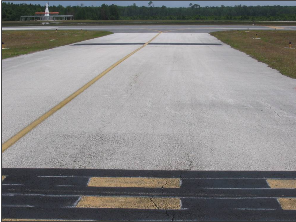
TW E Section 505: Low Severity Linear/Transverse Cracking (May 10, 2007)
