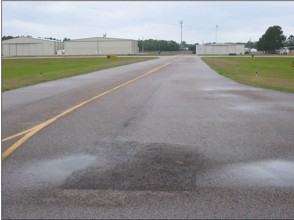
TW SW Section 1305: Low Severity Weathering (May 9, 2007)
