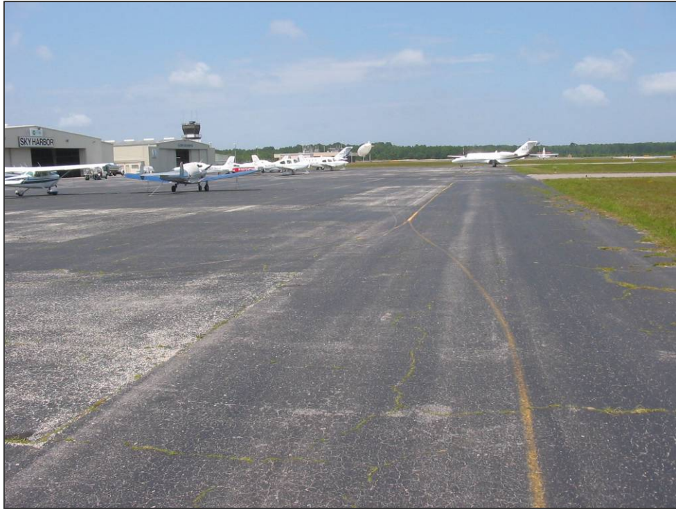
AP S Section 4105: Medium Severity Weathering (May 10, 2007)
