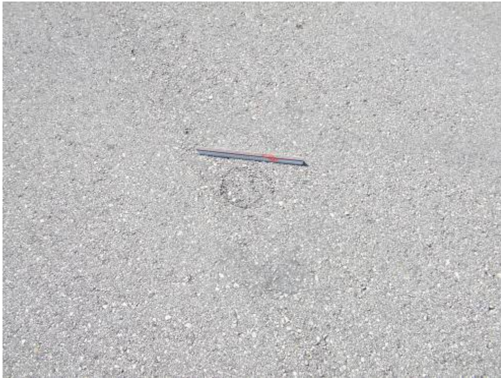
TW B Section 205 SU 300: Low Severity Patch (December 30, 2007)
