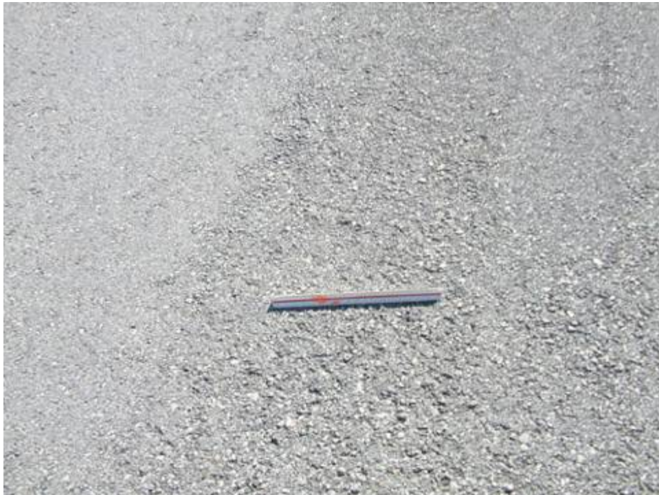
Taxiway E Section 605 SU 100: Low/Medium Severity Weathering (December 30, 2007)
