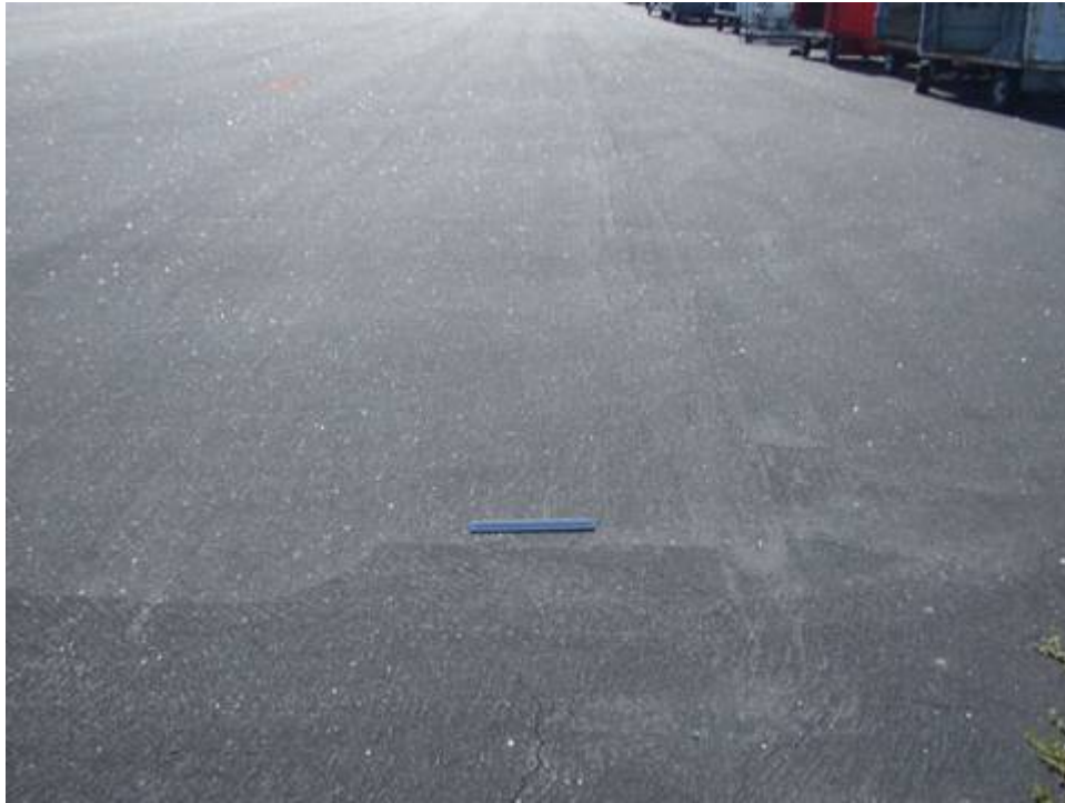
Apron E Section 520 SU 300: Low Severity L/T Cracking (December 30, 2007)
