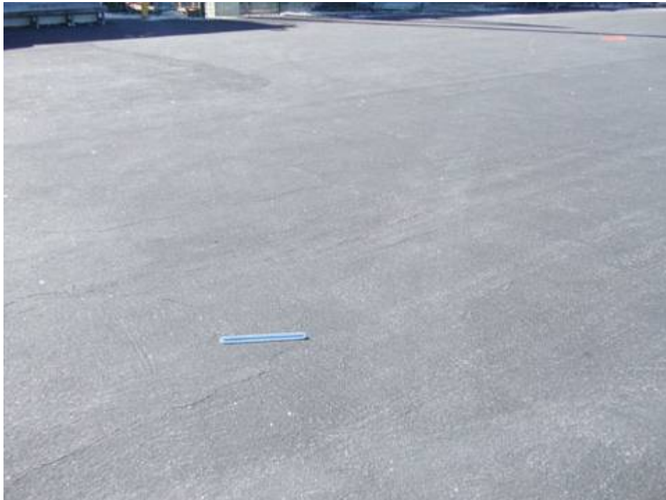
Apron E Section 4110 SU 203: Low Severity L/T Cracking (December 30, 2007)
