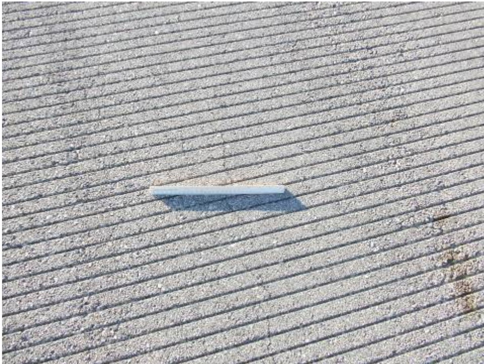
Runway 9-27 Section 6105 SU 108: Low Severity L/T Cracking (December 30, 2007)
