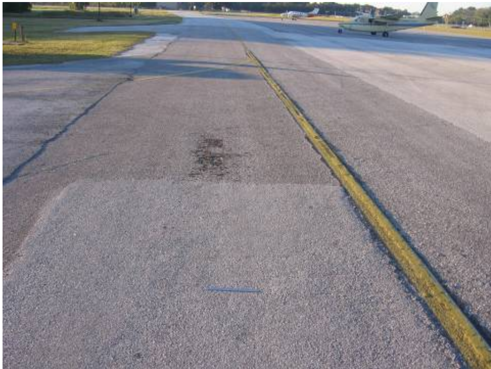
TW CONN Section 205 SU 103: Low Severity Patching and Medium Severity Weathering (October 24, 2006)
