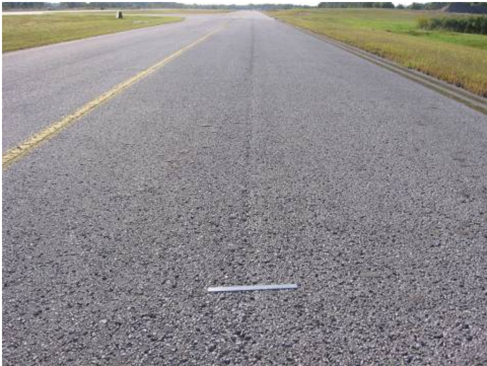
TW PARALL Section 107 SU 115: Low Severity Weathering (October 24, 2006)
