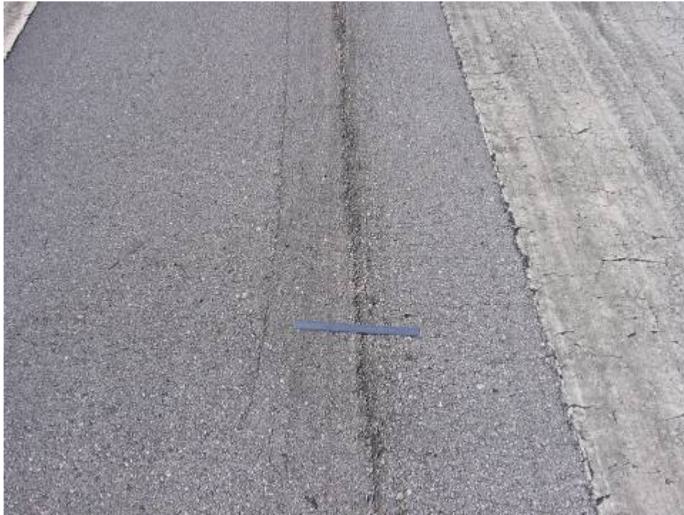
RW 9-27 Section 6115 SU 98: Low Severity L/T Cracking (October 24, 2006)
