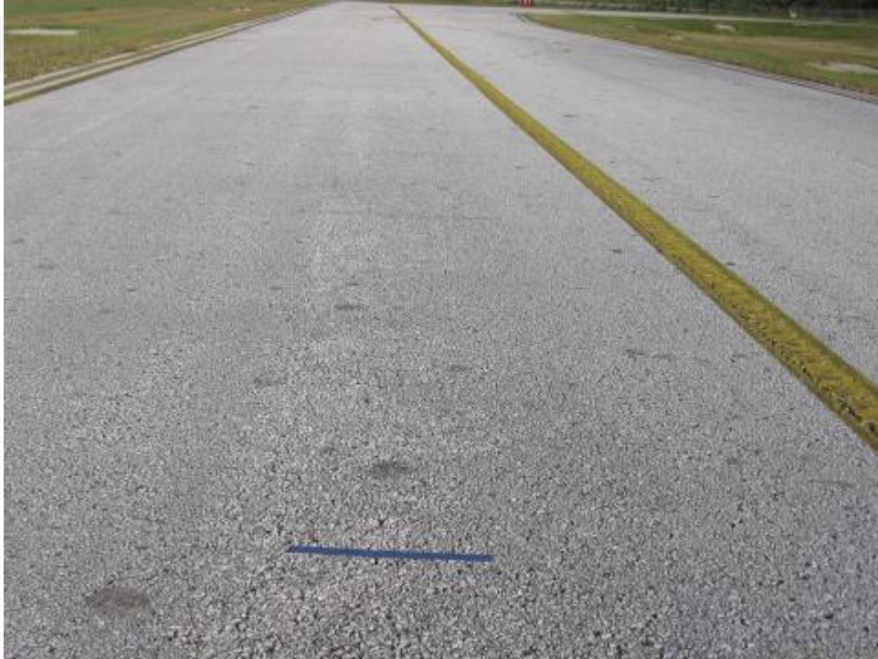
TW PARALL Section 107 SU 120: Low Severity Weathering (October 24, 2006)
