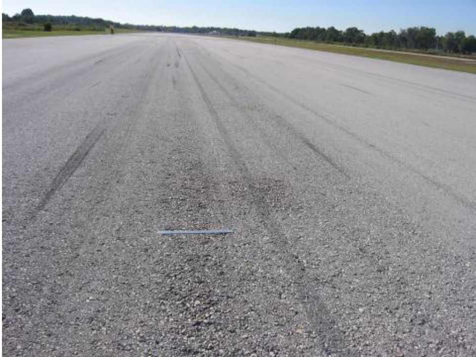
RW 9-27 Section 6110 SU 171: Low Severity Weathering (October 24, 2006)
