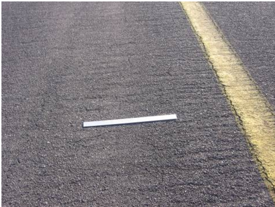
AP T-HANG Section 4205 SU 301: Low Severity Weathering (October 24, 2006)
