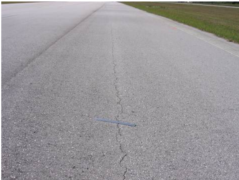
RW 9-27 Section 6105 SU 126: Low Severity L/T Cracking (October 24, 2006)
