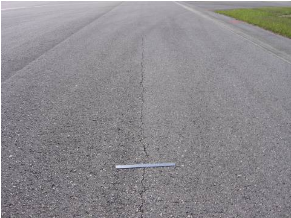
RW 9-27 Section 6105 SU 131: Low Severity L/T Cracking (October 24, 2006)
