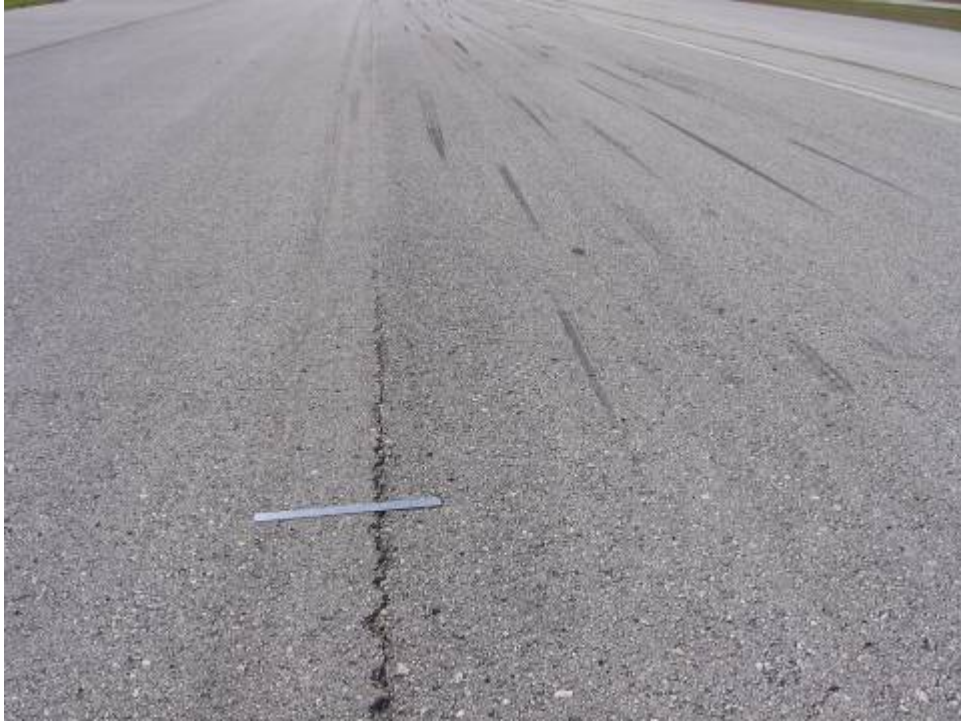
RW 9-27 Section 6110 SU 161: Low to Medium Severity L/T Cracking (October 24, 2006)
