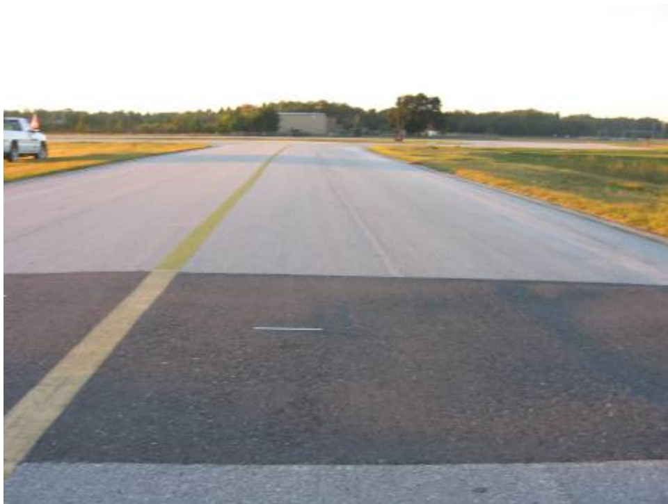
TW CONN Section 205 SU 101: Low Severity Patching (October 24, 2006)
