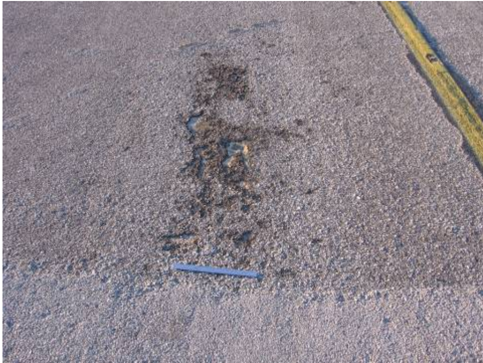
TW CONN Section 205 SU 103: Medium Severity Weathering (October 24, 2006)
