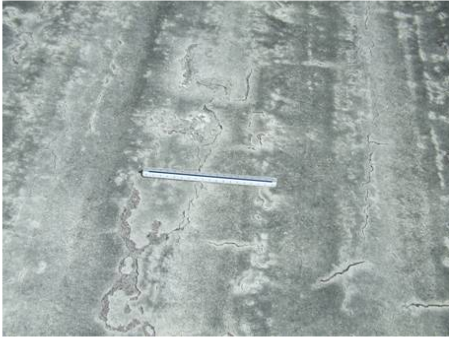
RW 13-31 Section 6205 SU 102: Low Severity Weathering (September 17, 2007)
