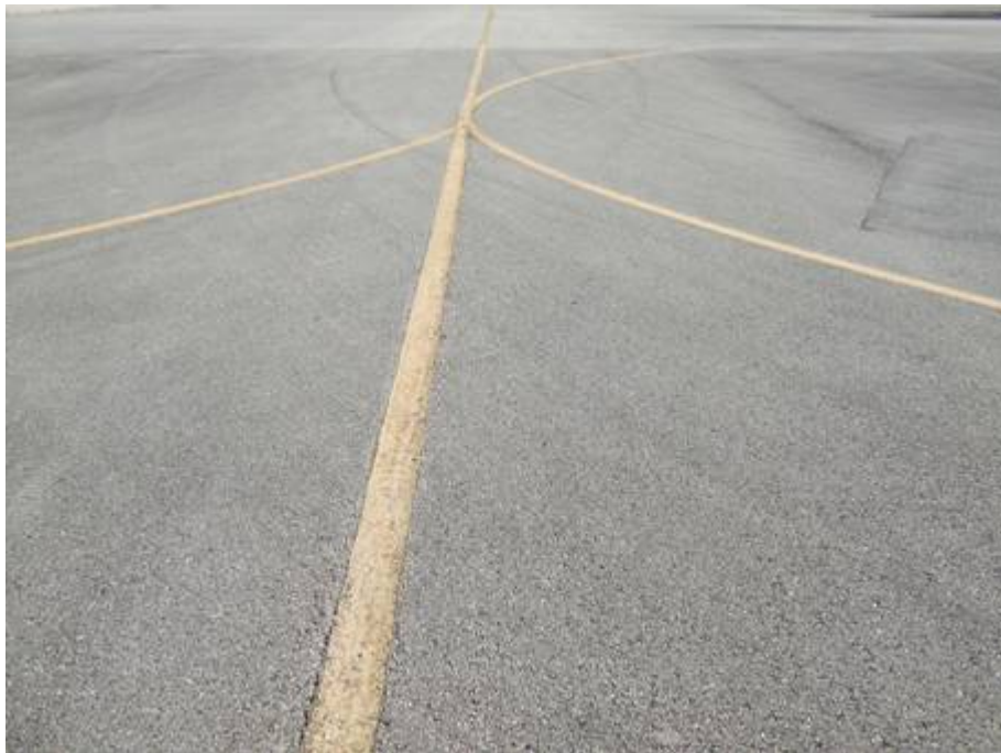
TW J Section 1010 SU 100: Low Severity L/T Cracking (September 17, 2007)
