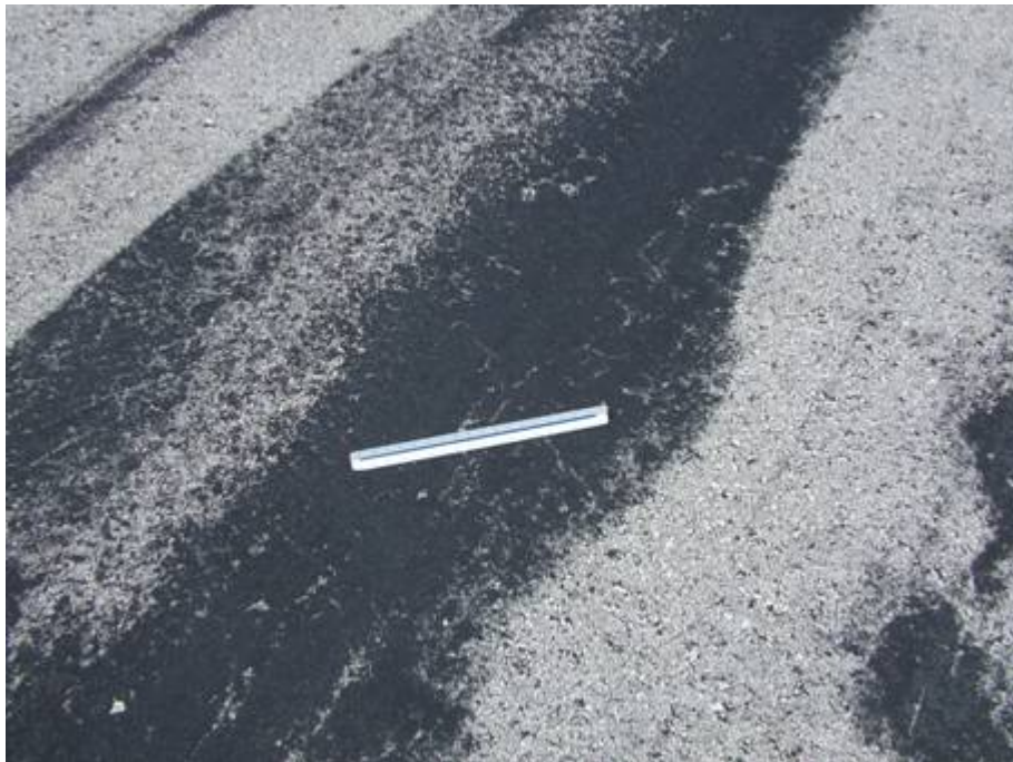
AP N Section 4120 SU 206: Low Severity Weathering (September 17, 2007)
