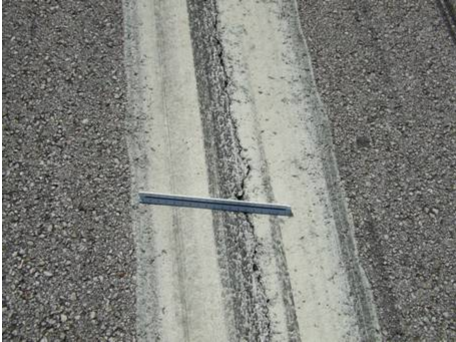
RW 8-26 Section 6105 SU 116: Low Severity L/T Cracking (September 17, 2007)
