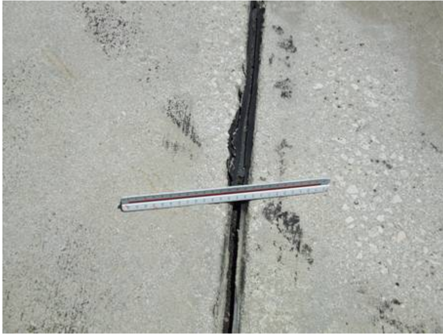
AP N Section 4110 SU 99: High Severity Joint Seal Damage (September 17, 2007)
