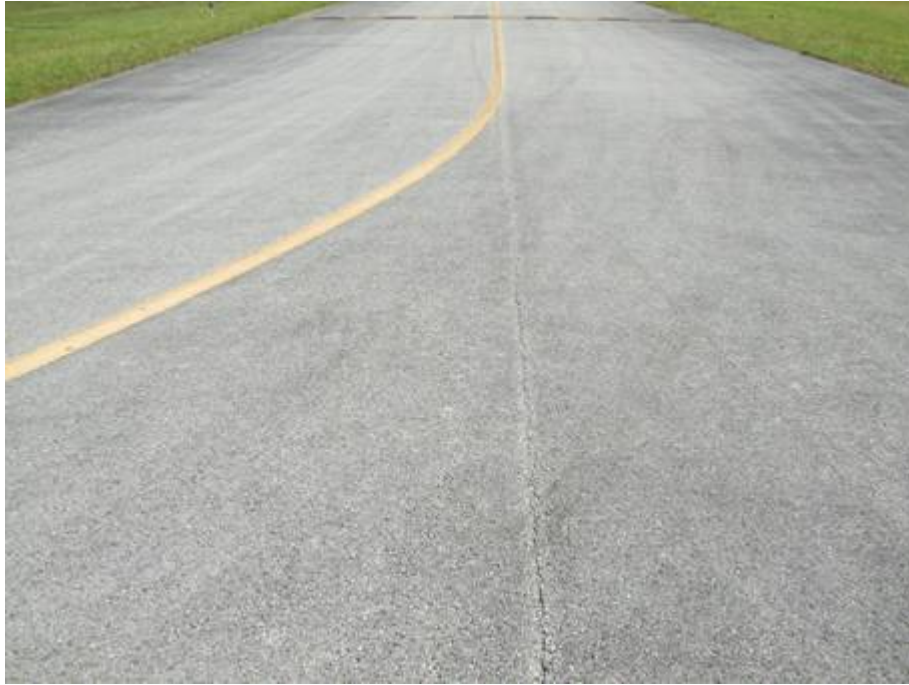
TW M Section 1305 SU 200: Low Severity L/T Cracking (September 17, 2007)
