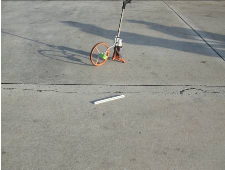
AP CC E Section 4305 SU 334: Medium Severity Joint Spall (November 30, 2007)
