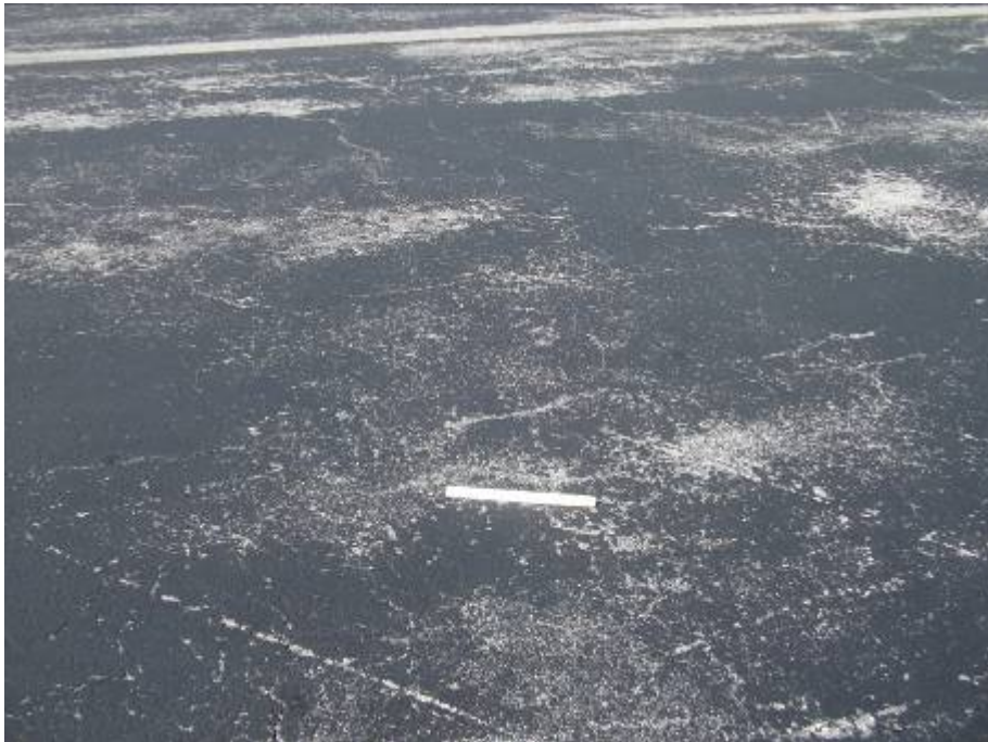
AP COMMON Section 4010 SU 356: Medium Severity Weathering (November 30, 2007)
