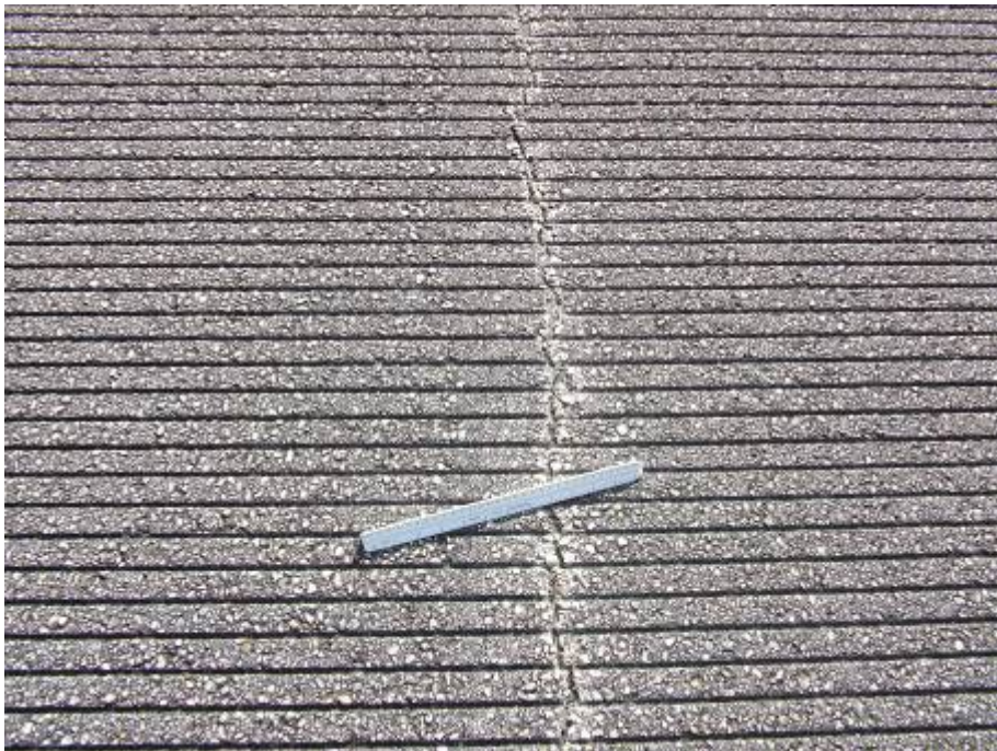
RW 13-31 Section 6290 SU 661: Low Severity L/T Cracking (November 30, 2007)
