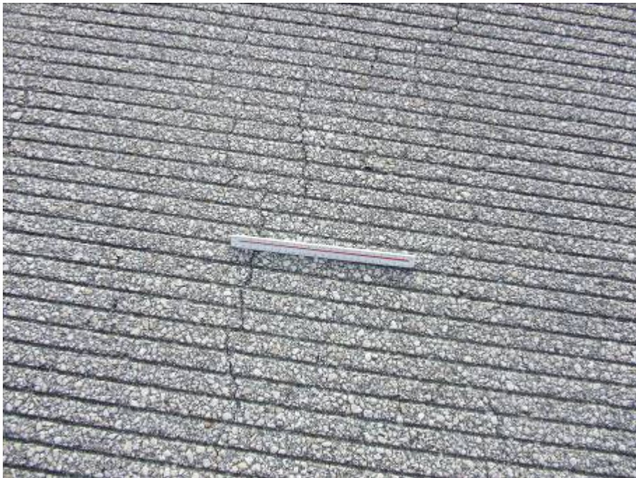
RW 13-31 Section 6215 SU 403: Low Severity L/T Cracking (November 30, 2007)
