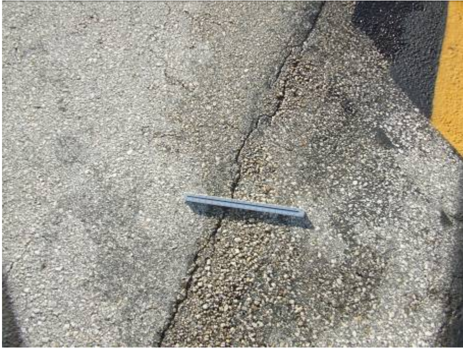
TW D Section 455 SU 530: Medium Severity L/T Cracking (November 30, 2007)
