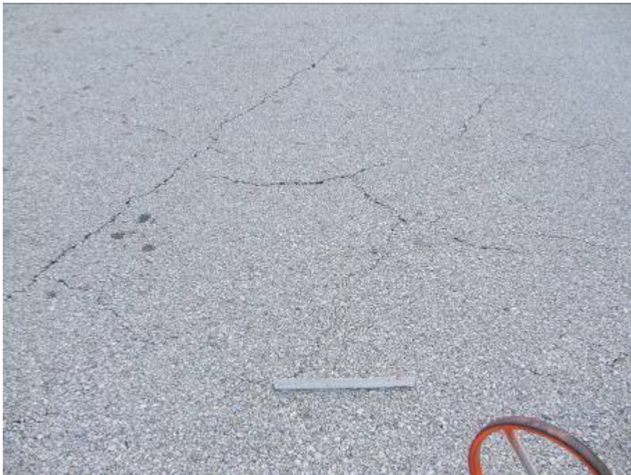
APCOMMON Section 4010 SU 526: Low Severity Block Cracking (November 30, 2007)
