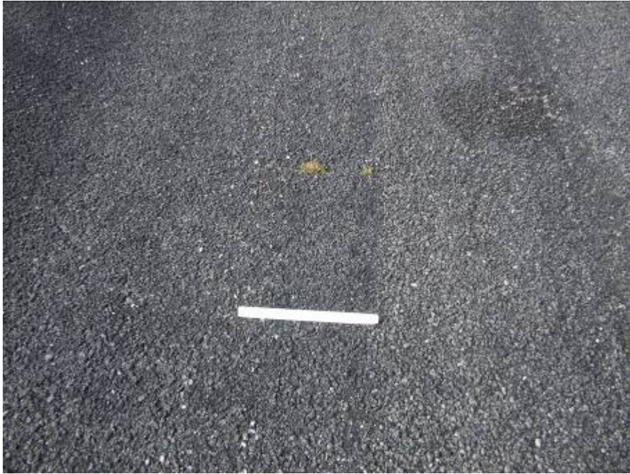
TW H 805 SU 530: Low Severity Weathering (November 30, 2007)
