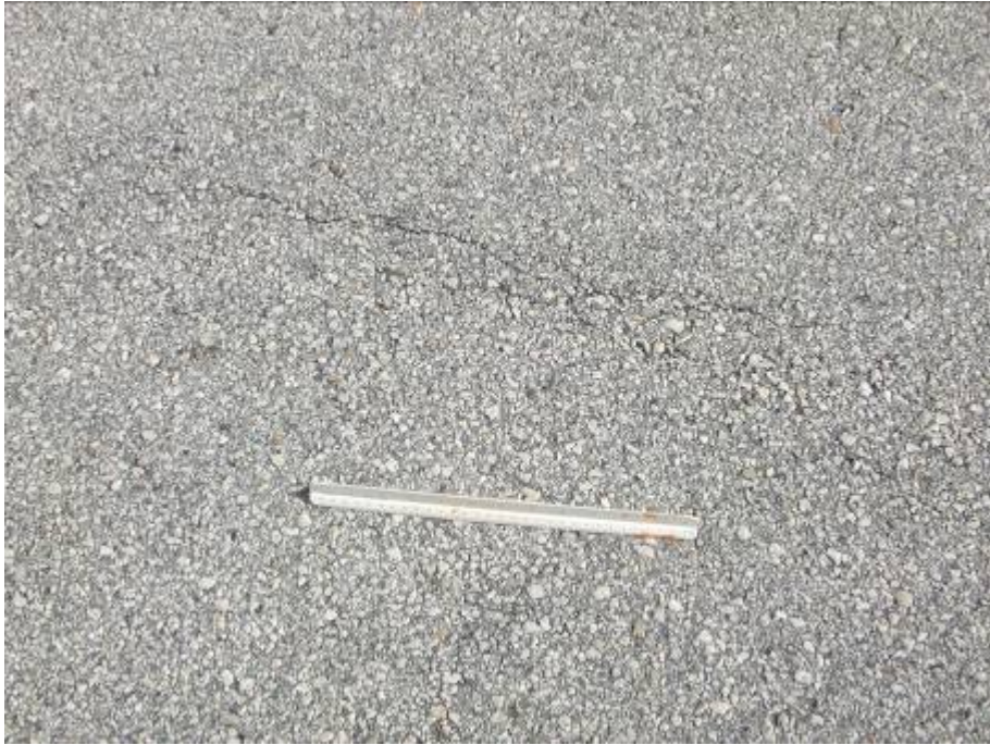
AP COMMON Section 4075 SU 457: Low Severity L/T Cracking (November 30, 2007)
