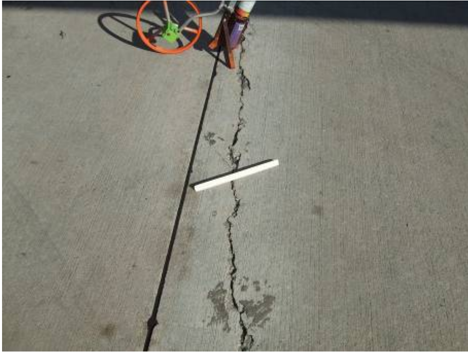
AP COMMON 4605 SU 337: Medium Severity Joint Spall (November 30, 2007)
