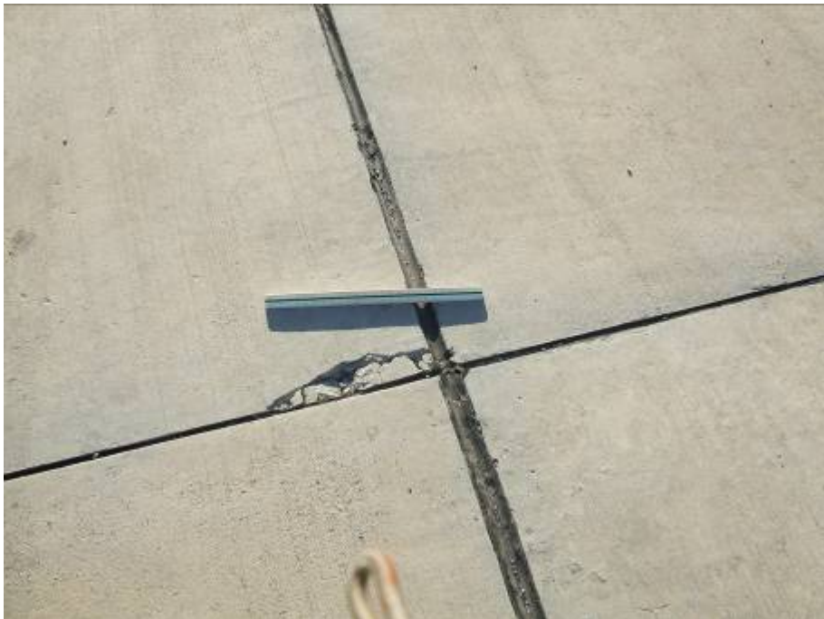
AP COMMON Section 4070 SU 203: Low Severity Joint Spall (November 30, 2007)
