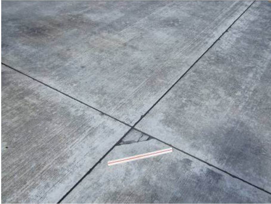
AP CC D Section 4205 SU 250: Low Severity Corner Spall (November 30, 2007)
