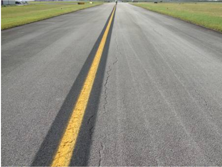
TW B Section 205: Low Severity L/T Cracking (October 10, 2007)
