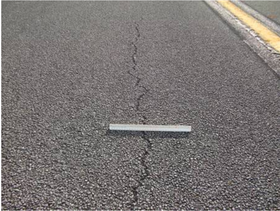
TW N Section 1405 SU 102: Medium Severity L/T Cracking (October 10, 2007)
