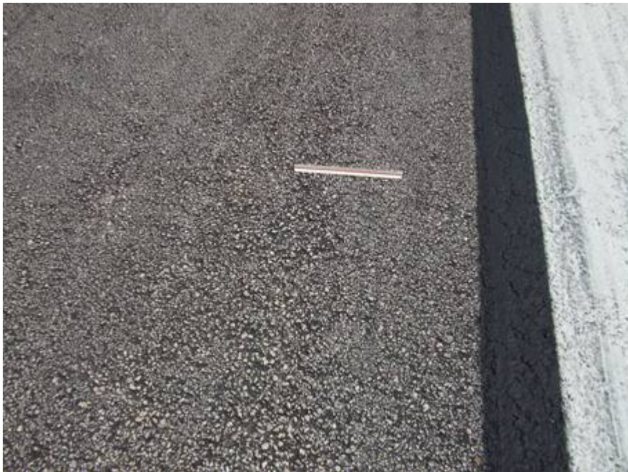
RW 9L-27R Section 6210 SU 1: Low/Medium Severity Weathering (October 10, 2007)
