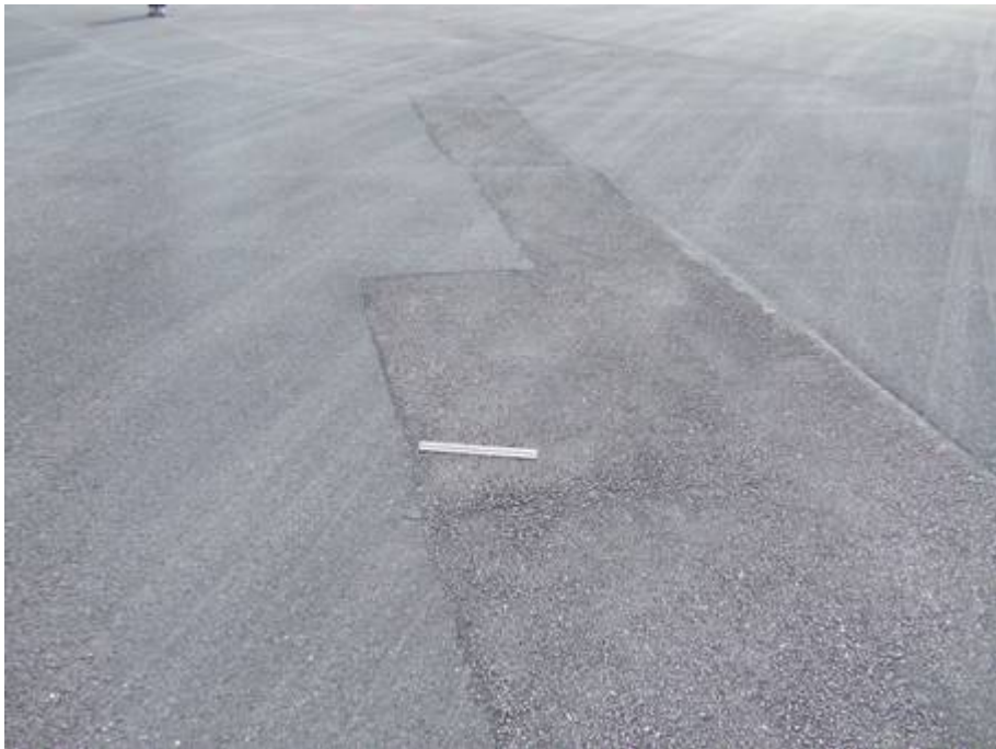
TW R Section 1810 SU 211: Low Severity Patch (October 10, 2007)
