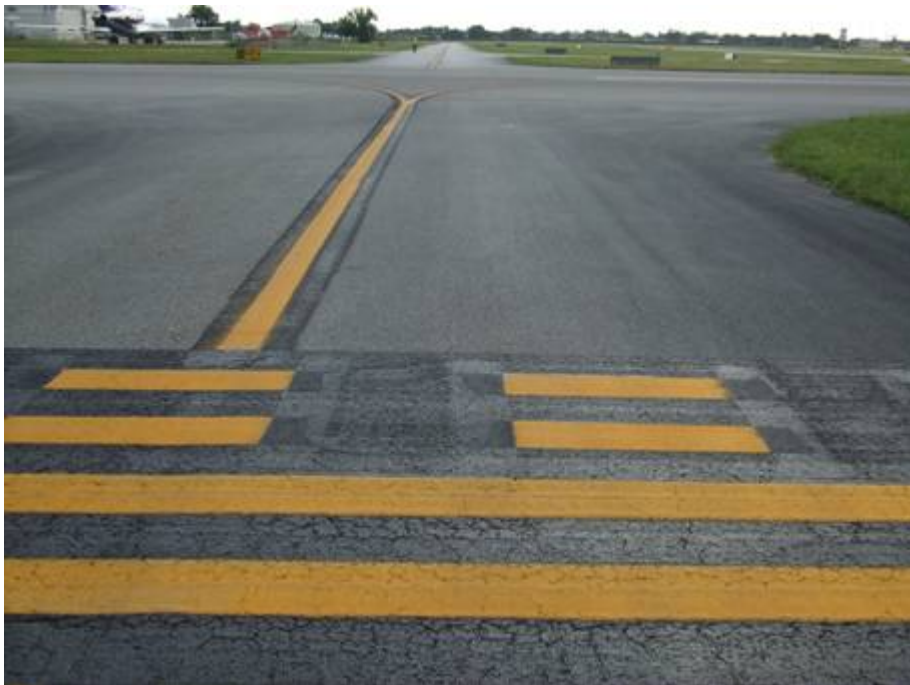
TW P Section 1610 SU 112: Medium Severity Weathering (October 10, 2007)
