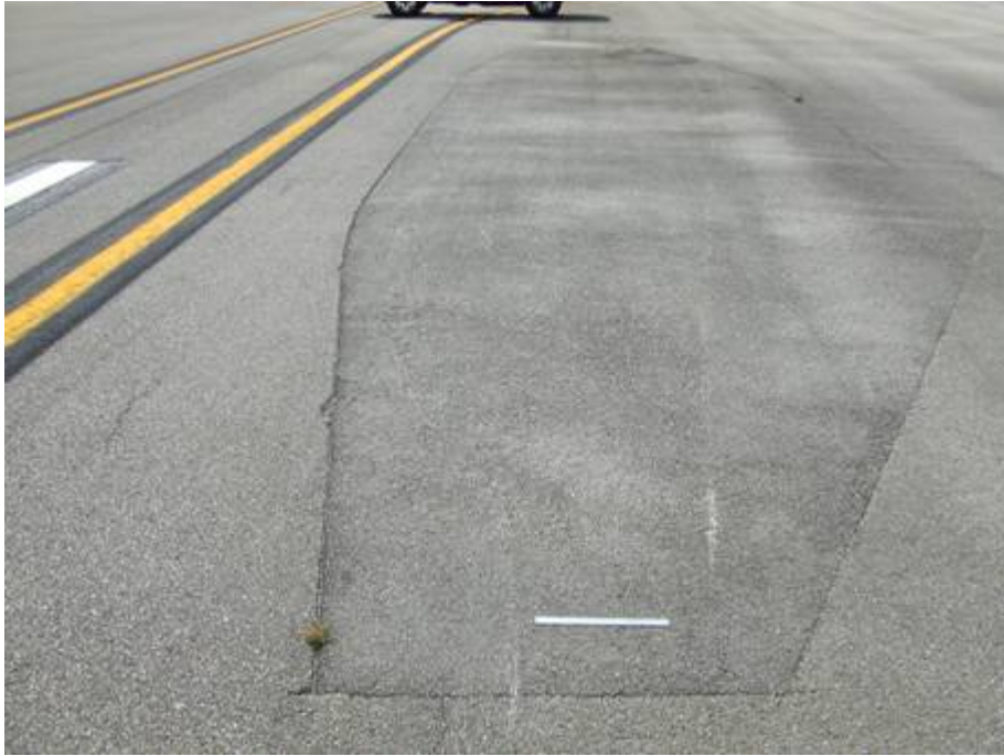
RW 18L-36R Section 6305 SU 117: Low Severity Patch (October 10, 2007)
