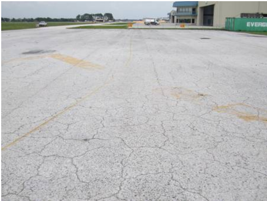
AP NW Section 4405 SU 201: Low Severity Block Cracking (June 19, 2007)
