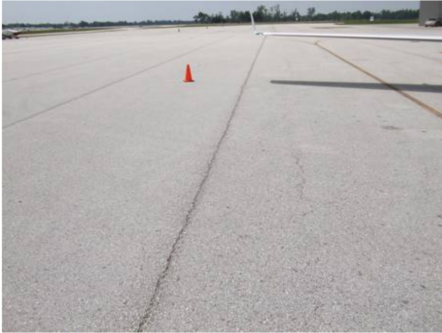
AP C NW Section 4305 SU 401: Low Severity L/T Cracking (June 19, 2007)
