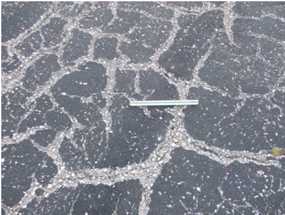
AP N Section 4112 SU 202: Medium Severity Weathering (June 19, 2007)
