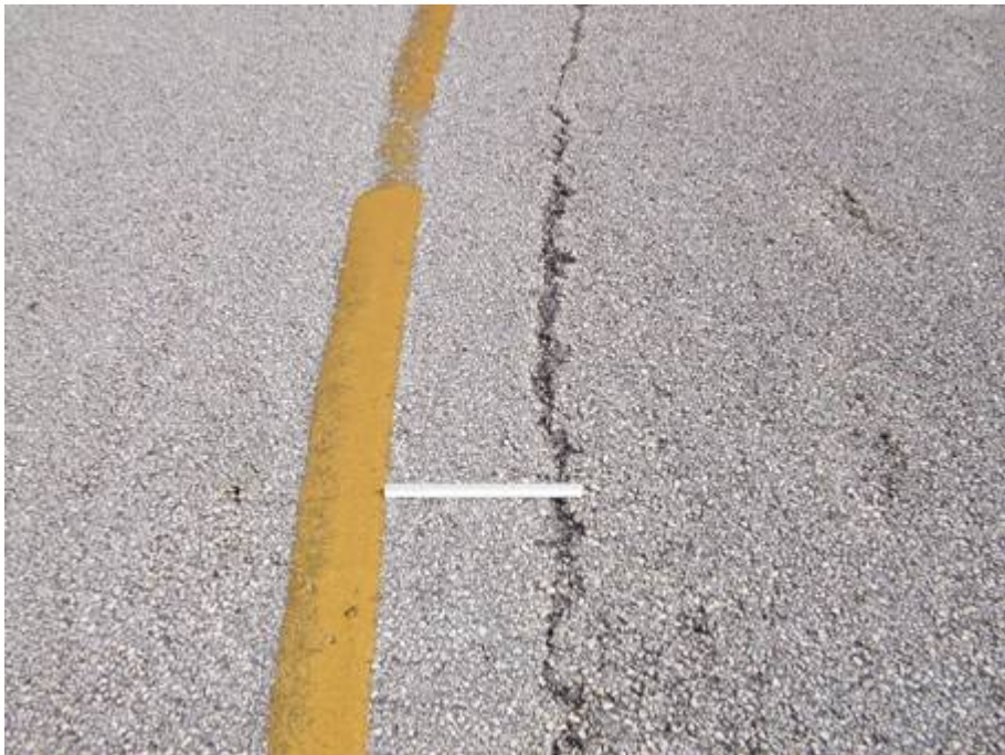
TW B Section 205 SU 201: Medium Severity L/T Cracking (June 19, 2007)
