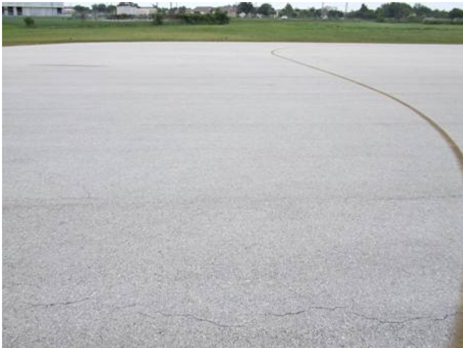
AP RU 15-33 Section 5110 SU 101: Low Severity L/T Cracking (June 19, 2007)
