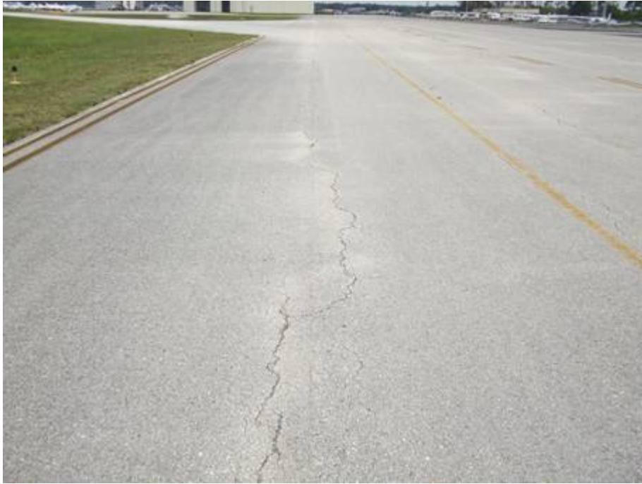
TW C Section 305 SU 302: Medium Severity L/T Cracking (June 19, 2007)
