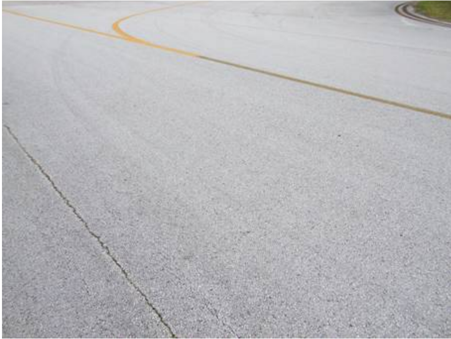
TW A Section 126 SU 111: Low Severity L/T Cracking (June 19, 2007)
