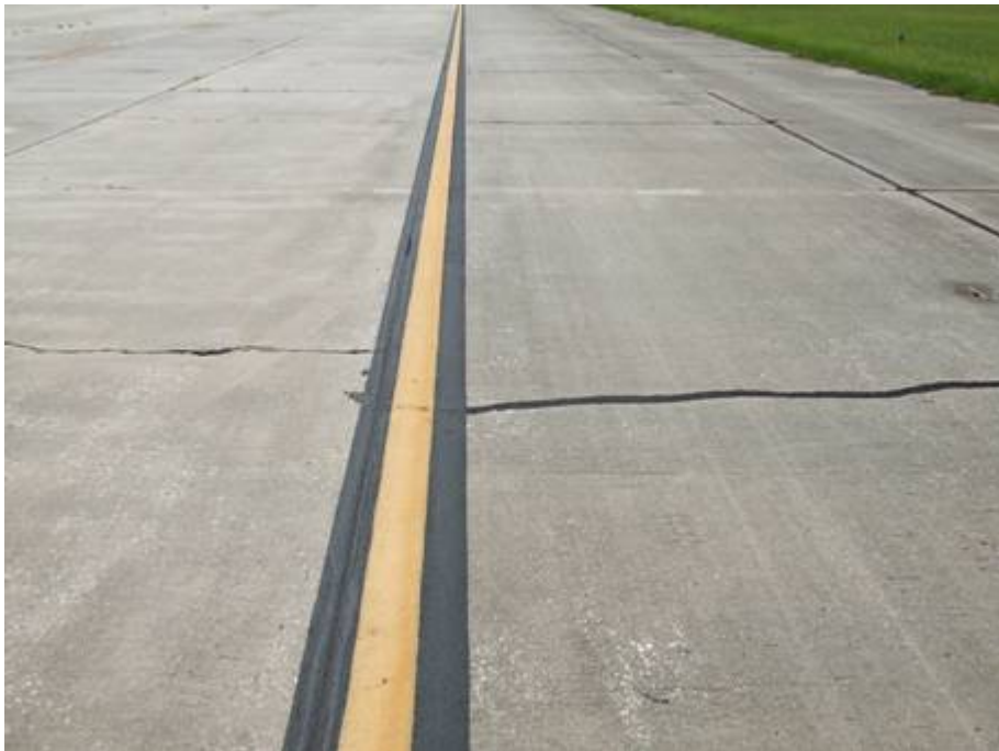
TW B Section 220 SU 230: Low Severity Linear Cracking (August 13, 2007)
