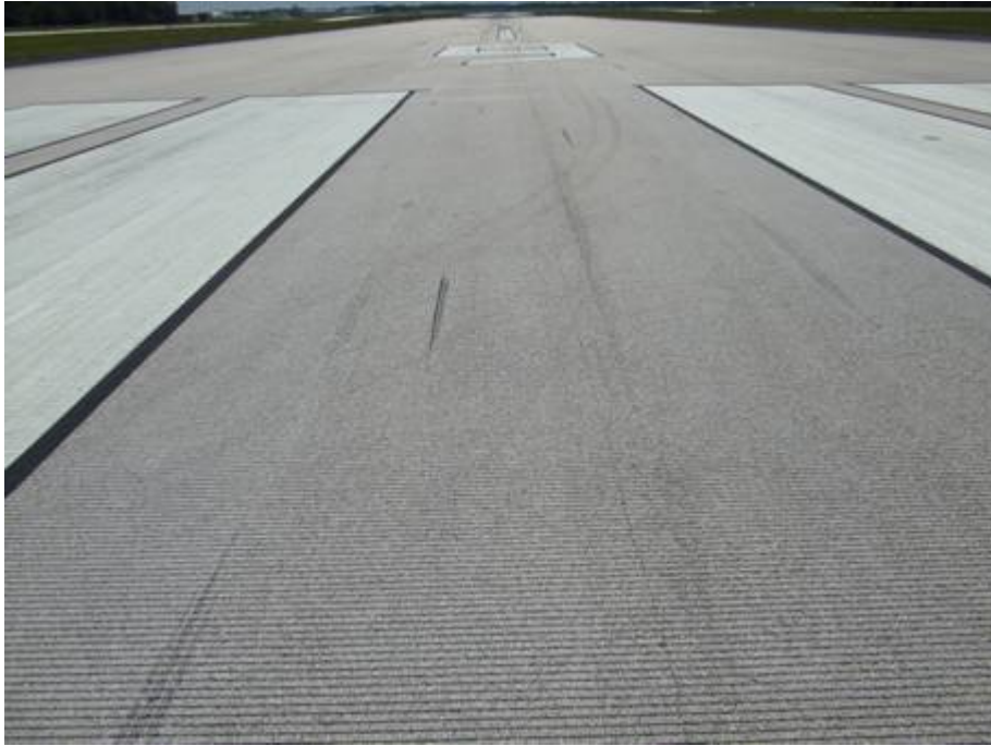
RW 9-27 Section 6105 SU 302: Low Severity L/T Cracking (August 13, 2007)
