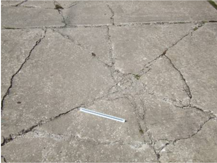
TW S Section 920 SU 601: High Severity Shattered Slab (August 13, 2007)
