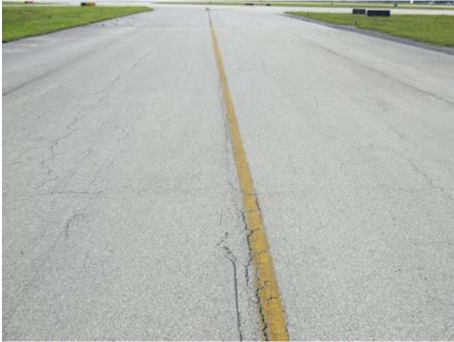
TW B Section 215 SU 224: Medium Severity L/T Cracking (August 13, 2007)
