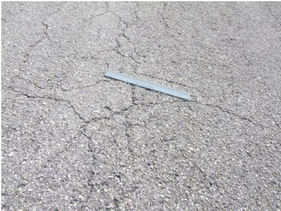
AP SW Section 4410 SU 501: Medium Severity Alligator Cracking (August 13, 2007)
