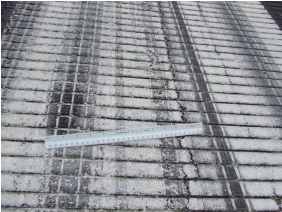
RW 9-27 Section 6155 SU 427: Low Severity L/T Cracking (August 13, 2007)
