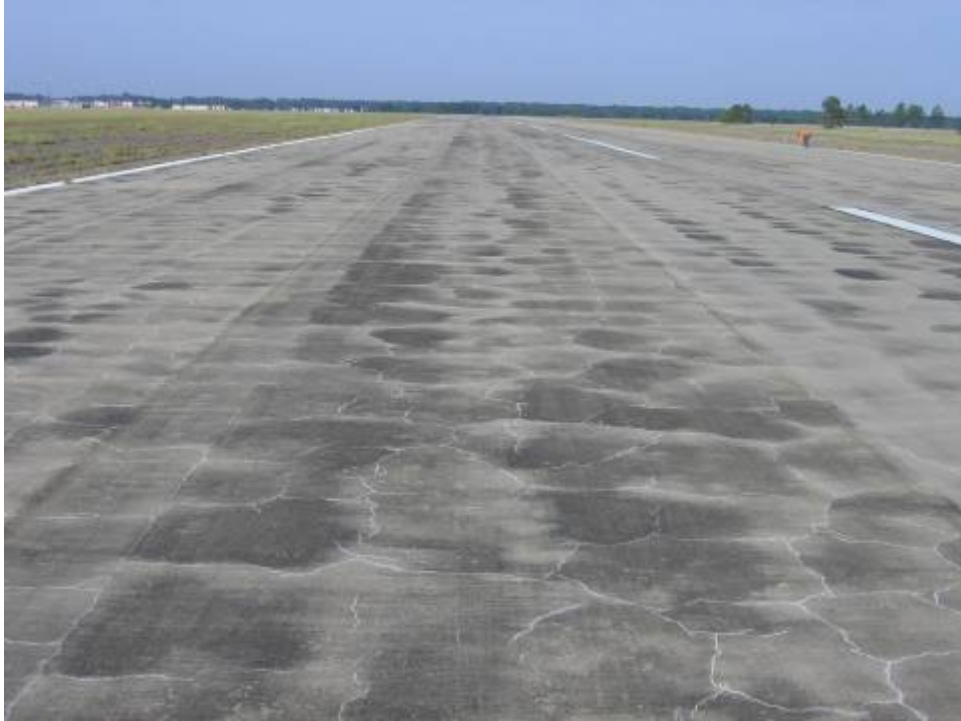
RW 8L-26R Section 6105 SU 343: Low Severity Block Cracking (October 3, 2006)
