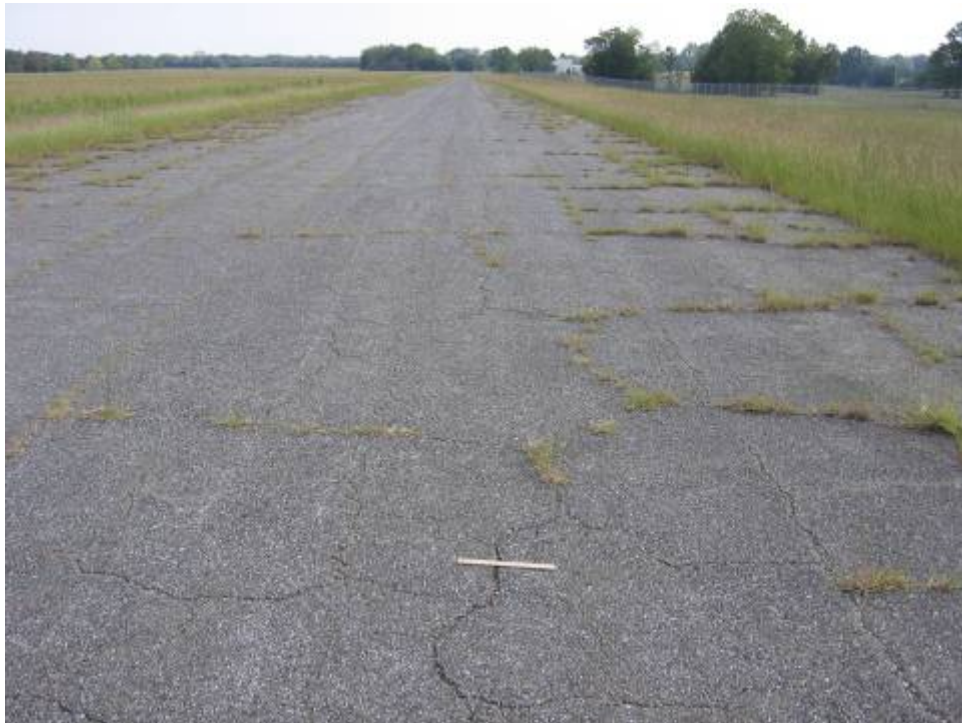
TW PARALL Section 105 SU 122: Medium Severity Block Cracking (October 3, 2006)
