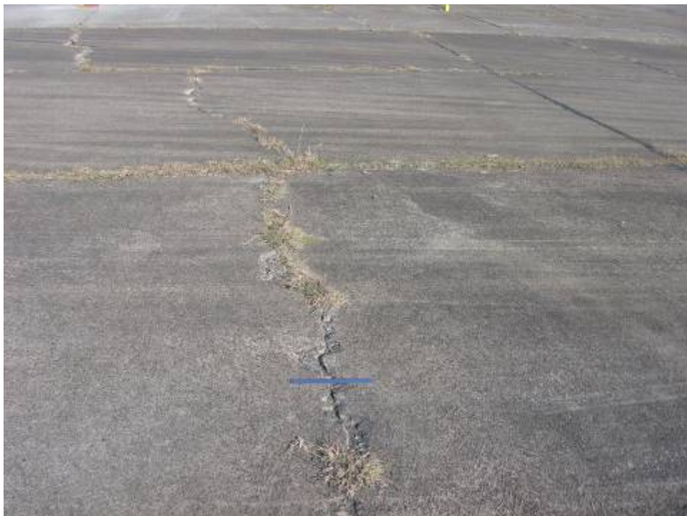
TW PARALL Section 150 SU 149: Medium Severity Linear Cracking (October 3, 2006)
