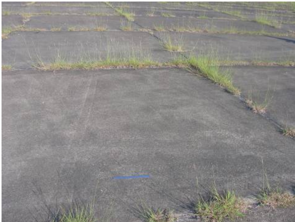
APRON Section 4105 SU 506: High Severity Joint Seal Damage (October 3, 2006)
