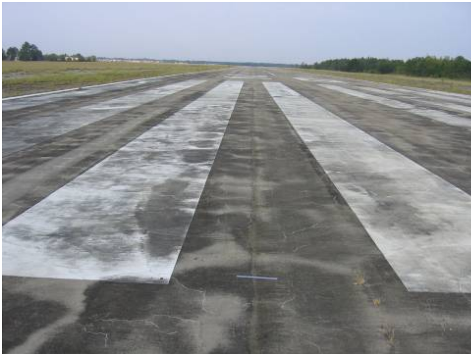
RW 8L-26R Section 6105 SU 300: Low Severity Block Cracking (October 3, 2006)
