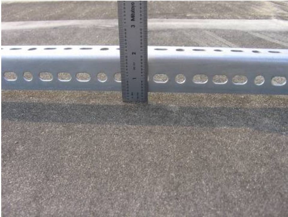
RW 8L-26R Section 6105 SU 300: Low Severity Swelling (October 3, 2006)
