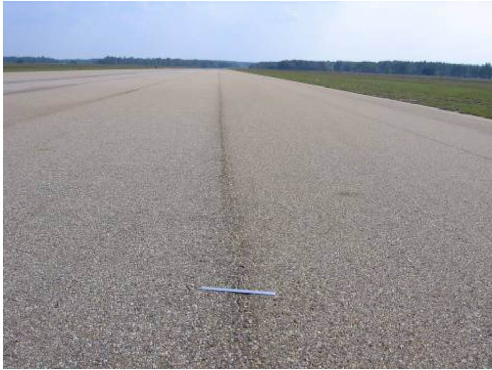
RW 18L-36R Section 6205 SU 156: Low Severity L/T Cracking (October 3, 2006)
