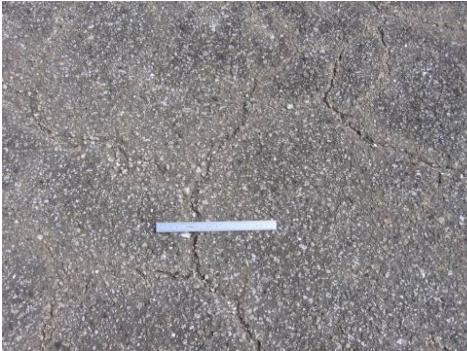
TW PARALL Section 105 SU 101: Low Severity Block Cracking (October 3, 2006)
