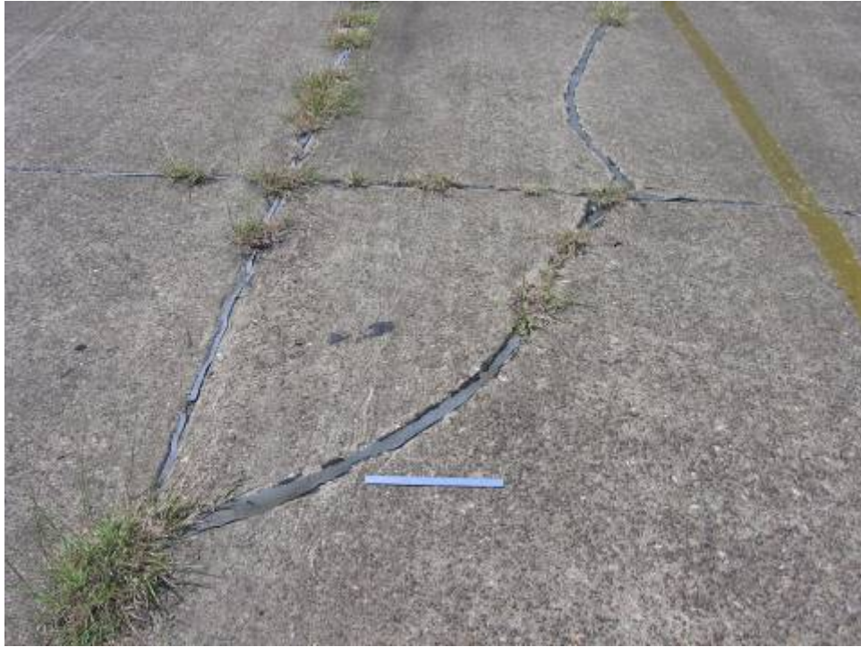
TW PARALL Section 150 SU 140: Medium Severity Corner Break (October 3, 2006)
