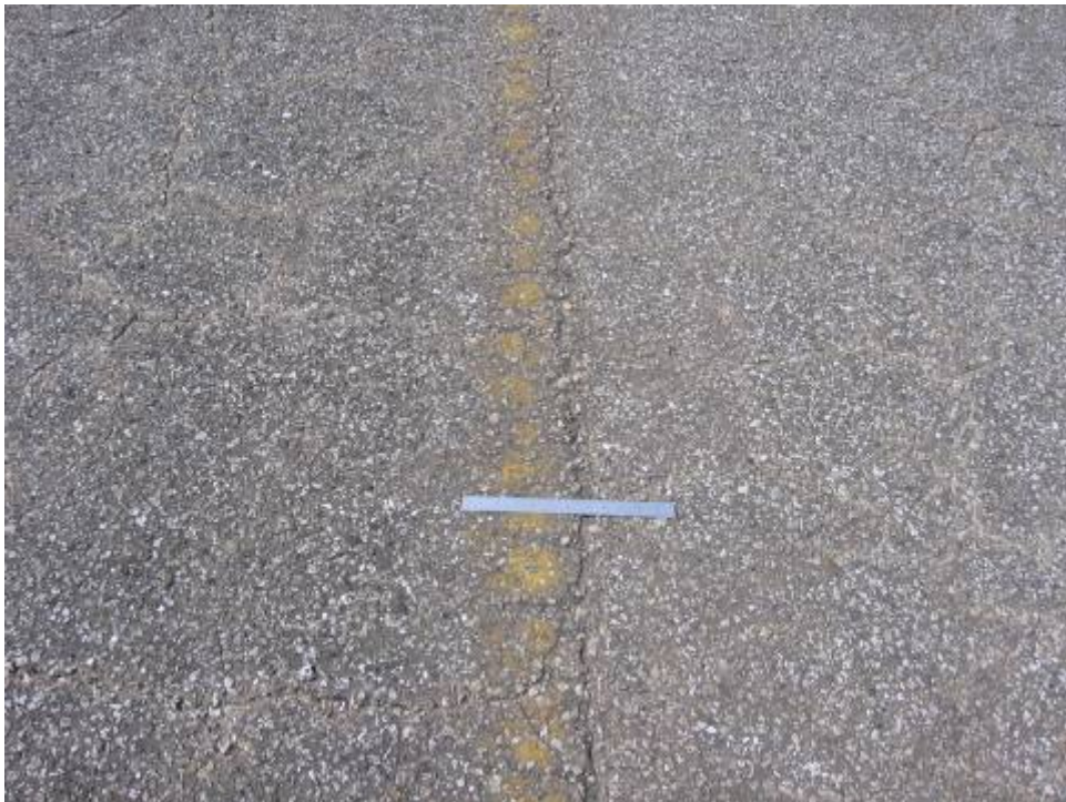
TW PARALL Section 105 SU 107: Low Severity L/T Cracking (October 3, 2006)
