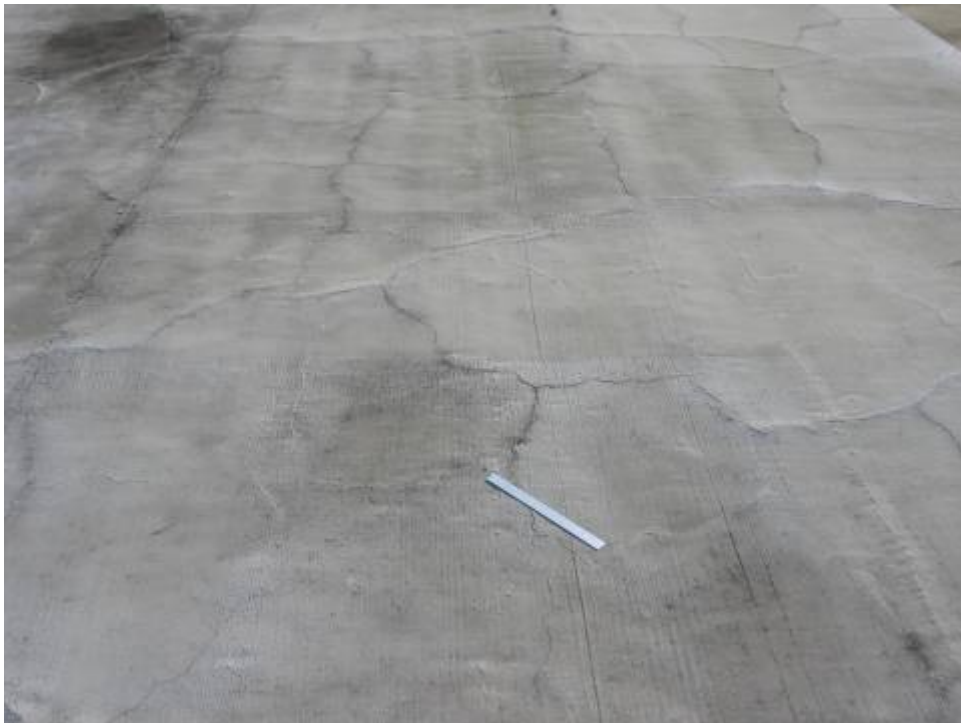
RW 8L-26R Section 6105 SU 322: Low Severity Block Cracking (October 3, 2006)
