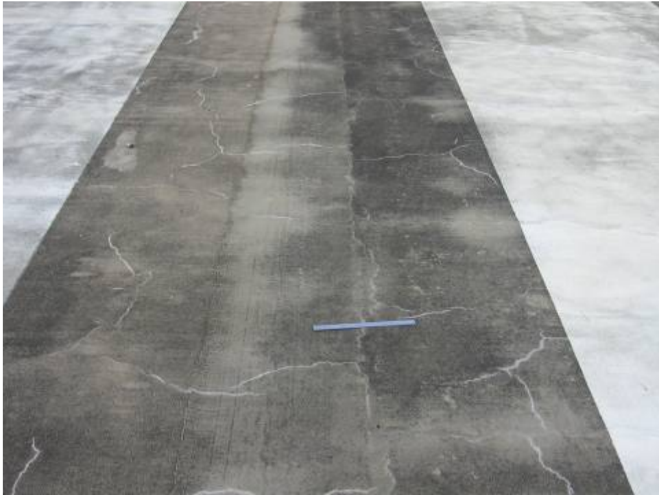
RW 8L-26R Section 6105 SU 301: Low Severity Block Cracking (October 3, 2006)
