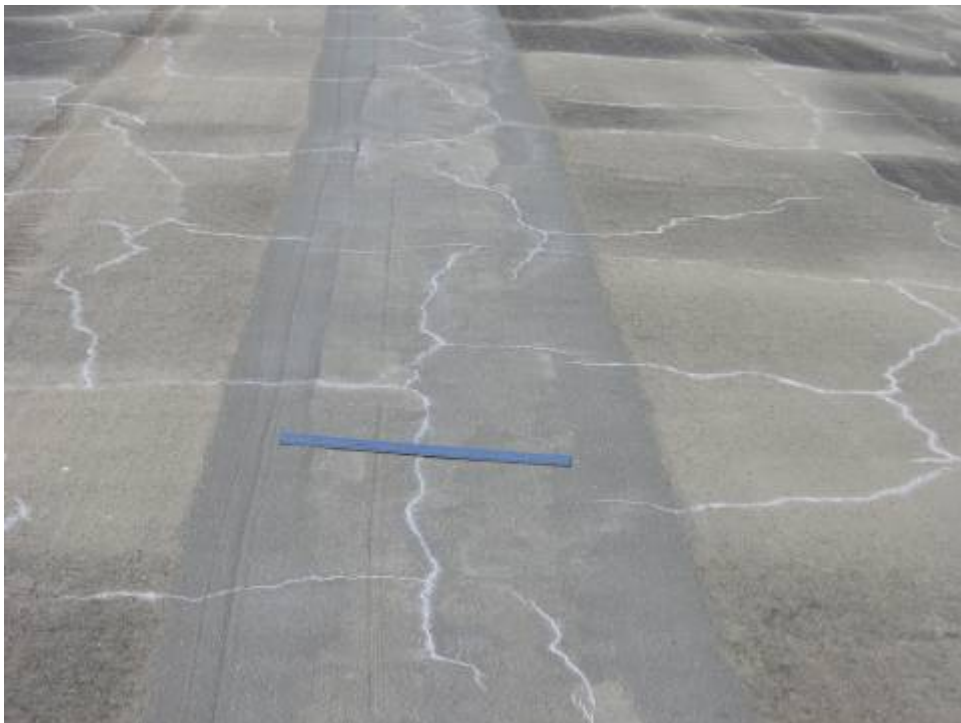
RW 8L-26R Section 6105 SU 378: Low Severity Block Cracking (October 3, 2006)
