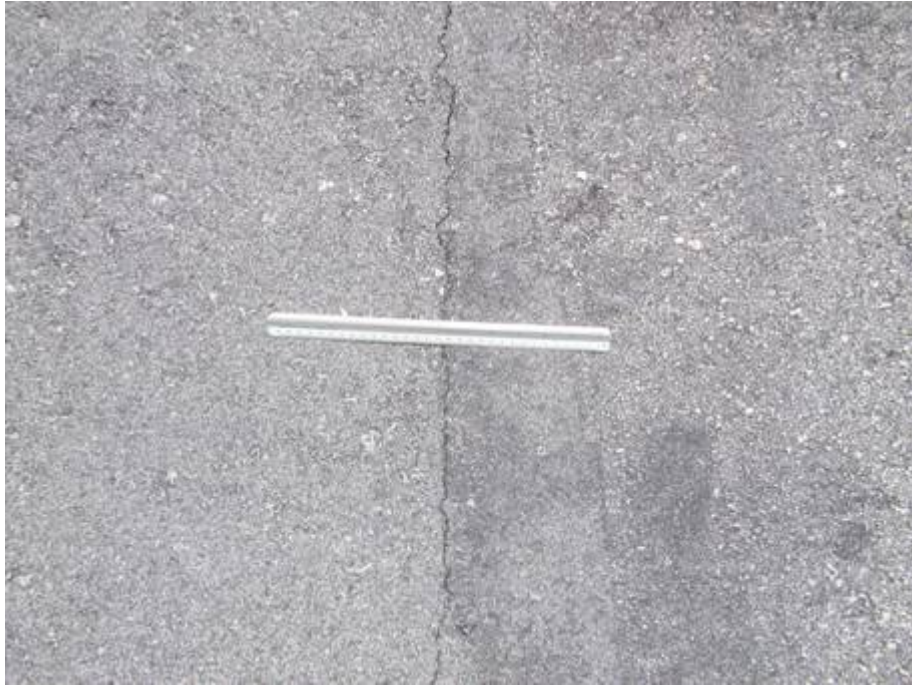
TW DB Section 410 SU 400: Low Severity L/T Cracking (July 9, 2007)
