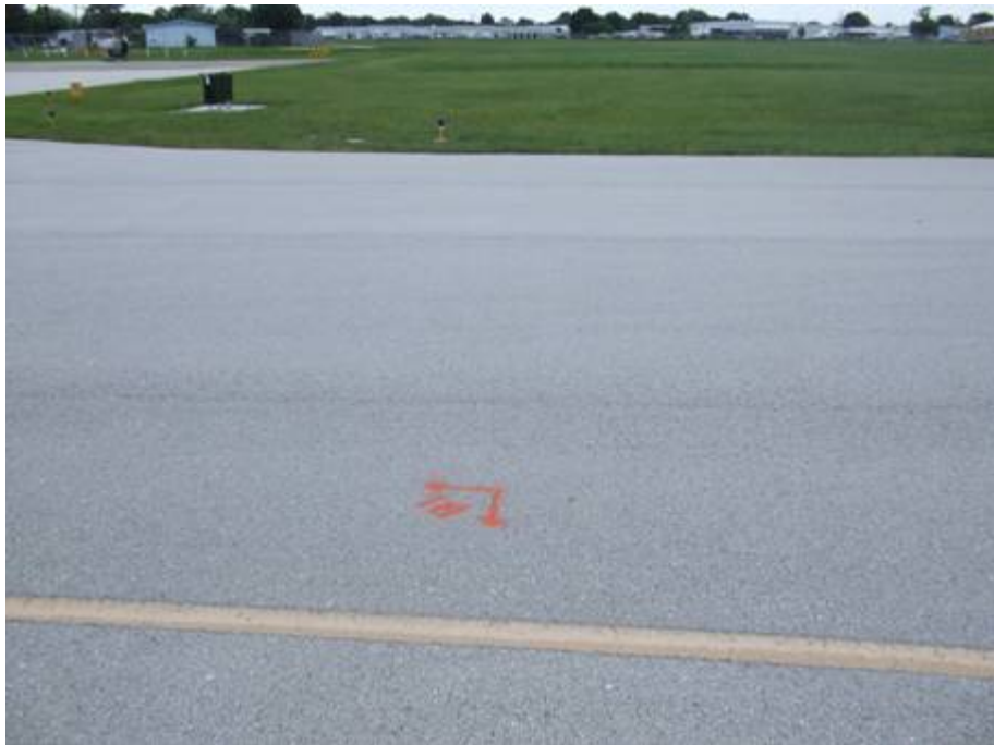
TW CA Section 305 SU 300: Low Severity L/T Cracking (July 9, 2007)
