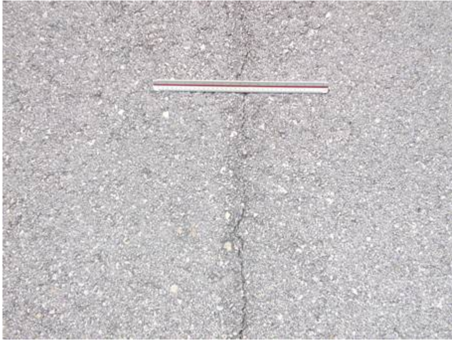
RW 11-29 Section 6105 SU 143: Low Severity L/T Cracking (July 9, 2007)
