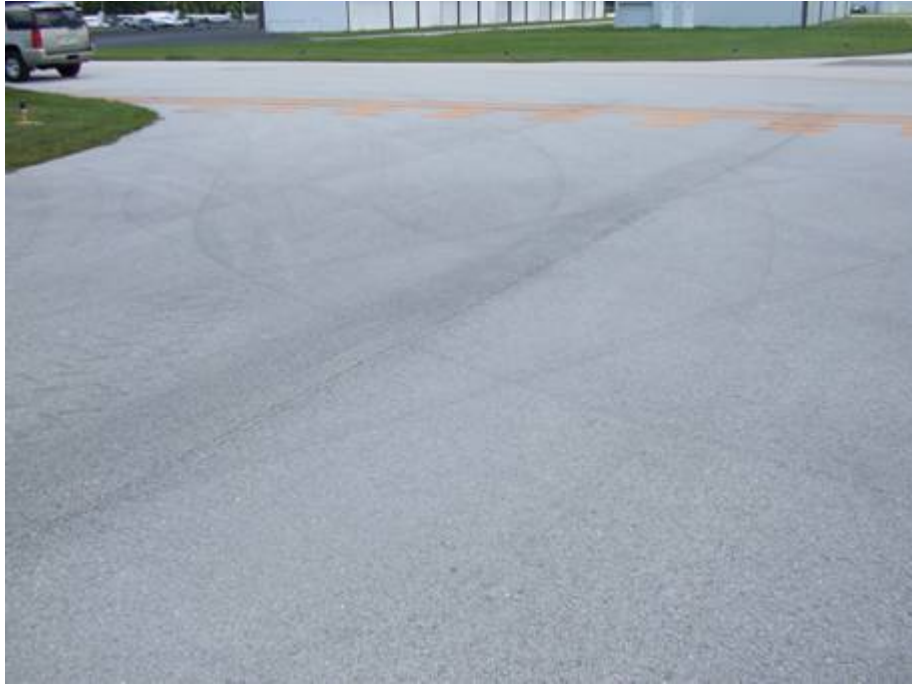
TW CA Section 310 SU 101: Low Severity L/T Cracking (July 9, 2007)
