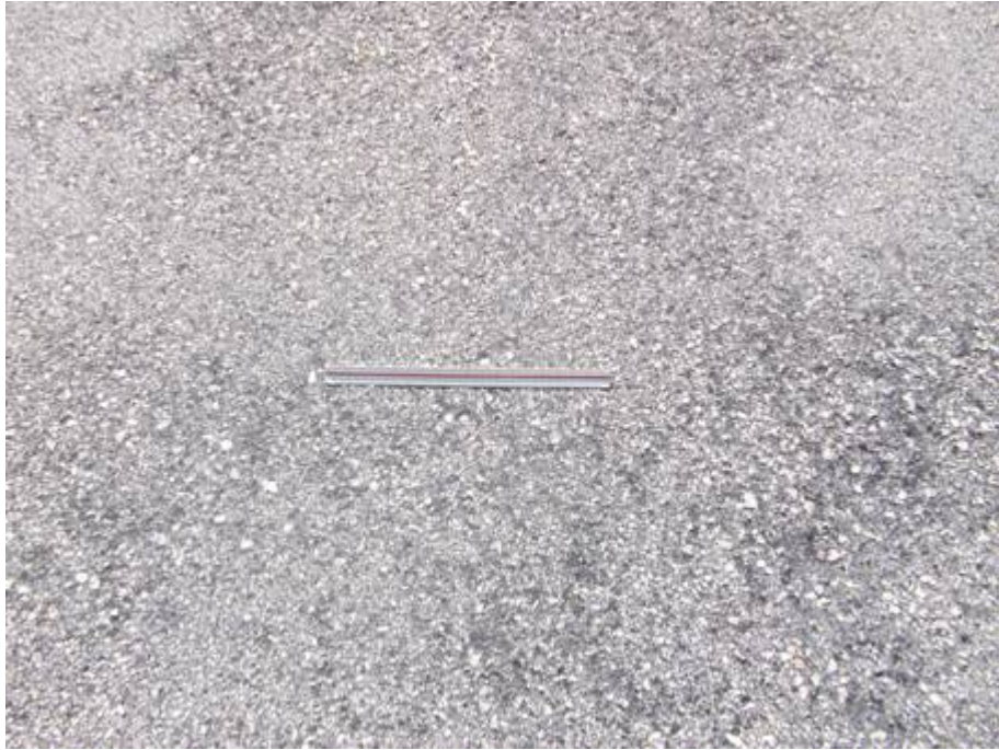
TW A Section 115 SU 300: Low Severity Weathering (July 9, 2007)
