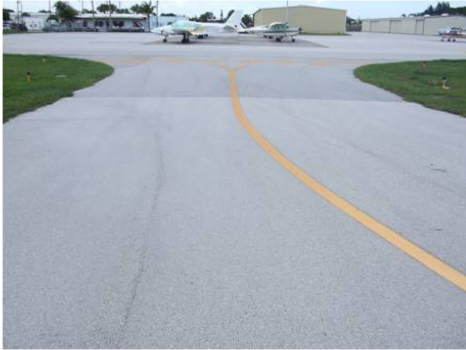
TW CB Section 315 SU 300: Low Severity L/T Cracking (July 9, 2007)
