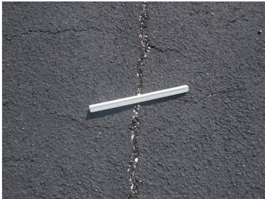
AP S Section 4106 SU 101: Medium Severity L/T Cracking (July 9, 2007)
