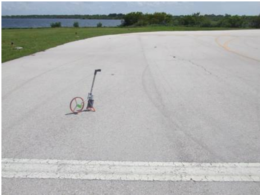
TW A Section 110 SU 100: Low Severity L/T Cracking (July 9, 2007)
