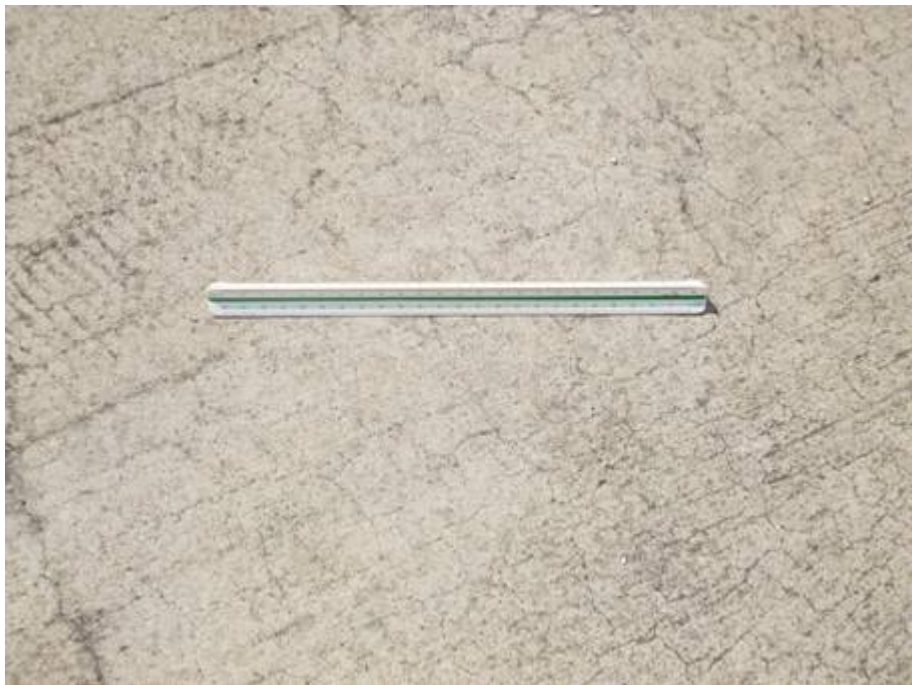
AP N Section 4203 SU 100: Low Severity Scaling (July 9, 2007)
