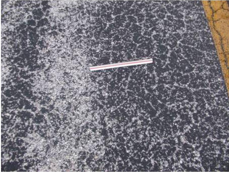
TW D Section 450 SU 102: Medium Severity Weathering (October 10, 2007)
