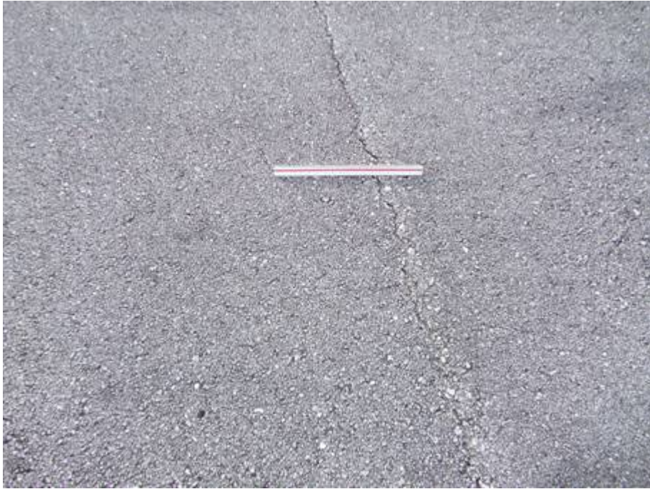
TW R Section 1825 SU 716: Low Severity L/T Cracking (October 10, 2007)
