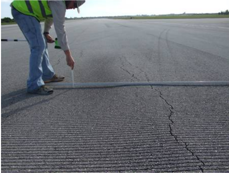
RW 9R-27L Section 6105 SU 382: Medium Severity Swell (October 10, 2007)
