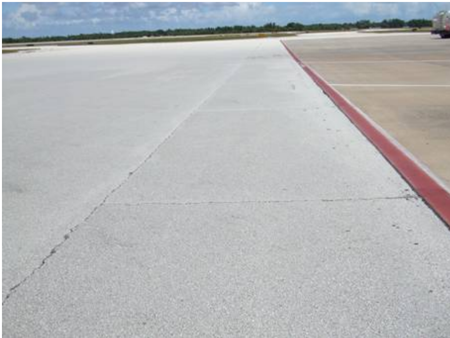
AP Term Section 4211 SU 800: Low Severity L/T Cracking (October 10, 2007)
