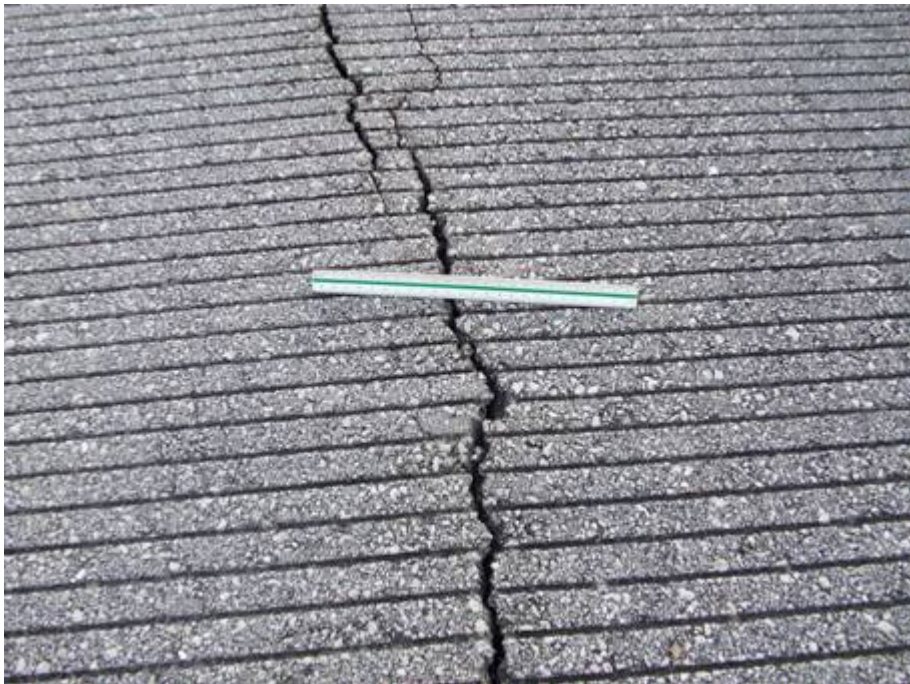
RW 9R-27L Section 6105 SU 318: Medium Severity L/T Cracking (October 10, 2007)
