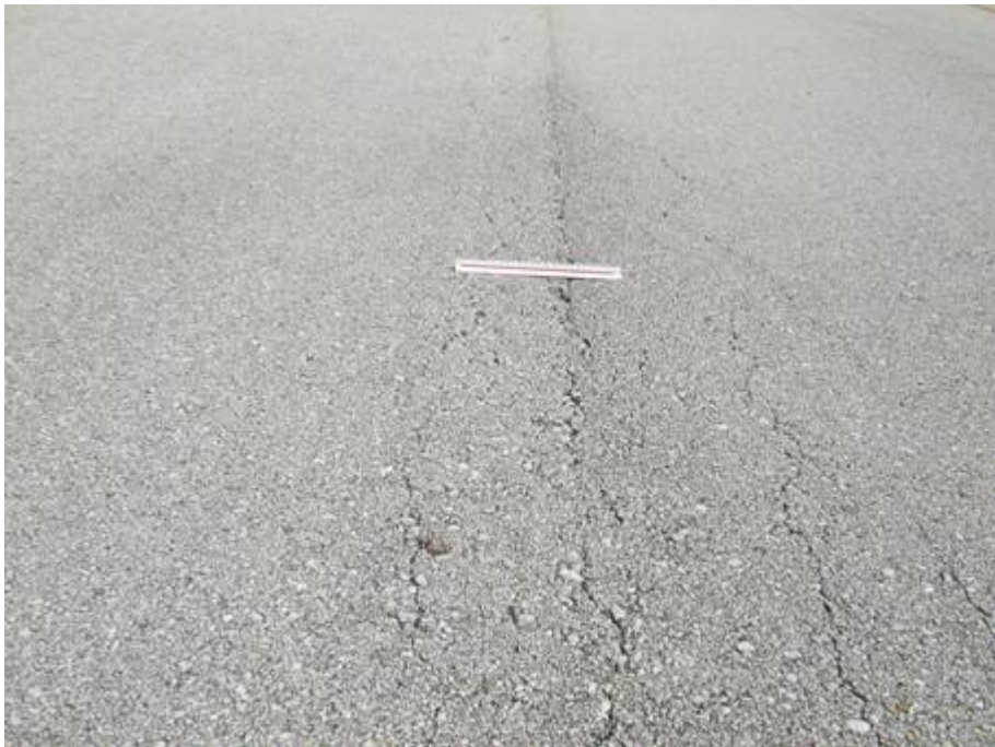
TW A Section 130 SU 105: Low Severity Alligator Cracking (October 10, 2007)
