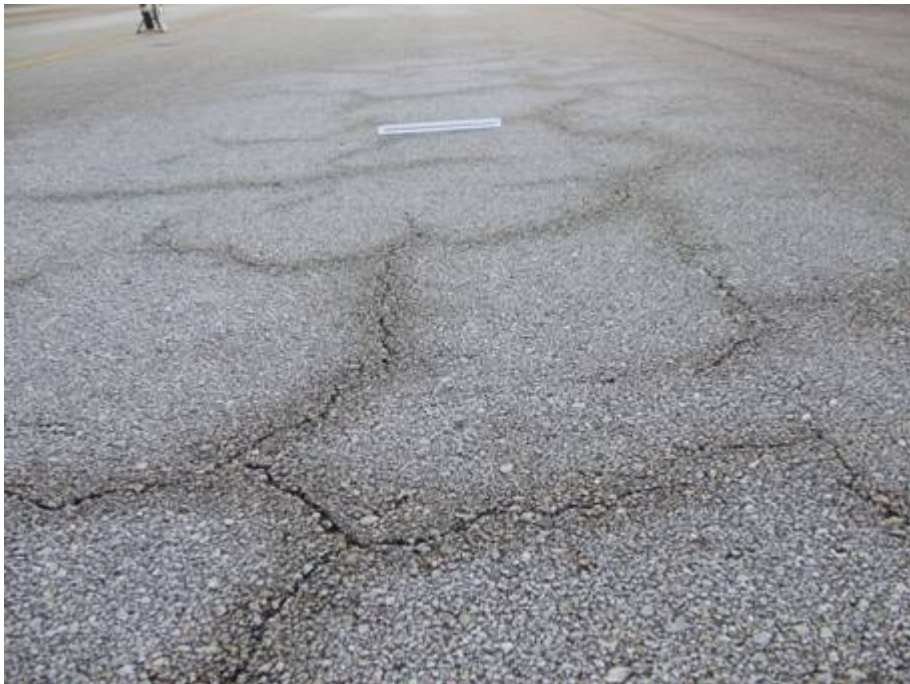
TW A Section 115 SU 105: Low Severity Block Cracking (October 10, 2007)
