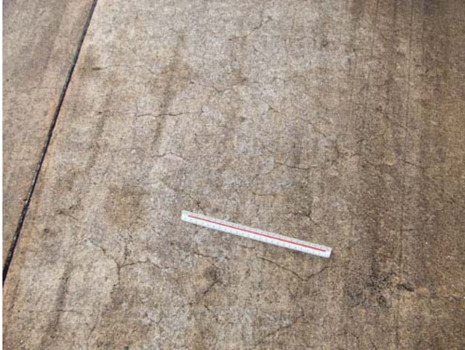
TW N Section 1435 SU 708: Low Severity Scalling (November 14, 2007)
