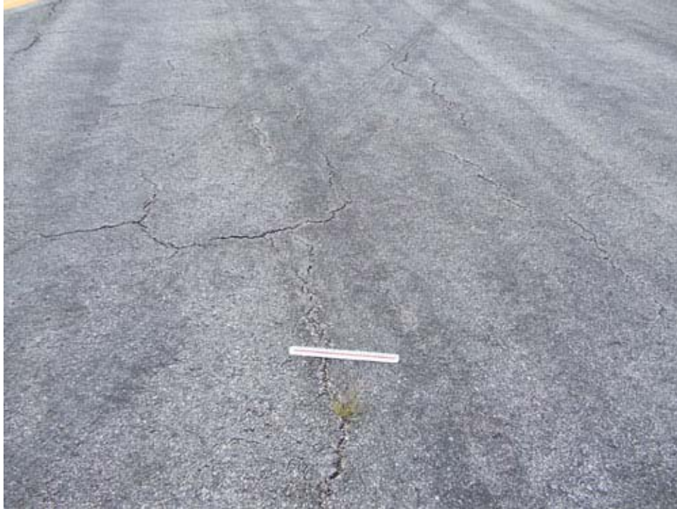
RW 18L-36R Section 6345 SU 391: Medium Severity Block Cracking (November 14, 2007)
