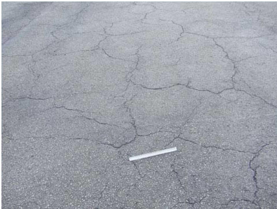
AP NE Section 4305 SU 262: Low Severity Block Cracking (November 14, 2007)
