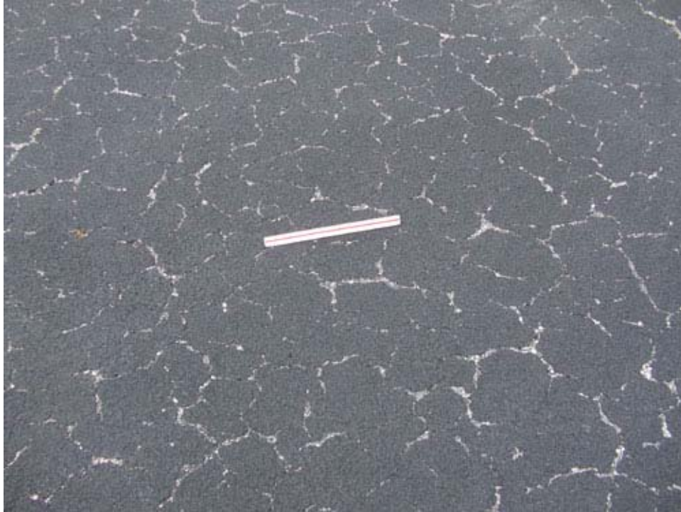
AP NE Section 4305 SU 136: Low Severity Weathering (November 14, 2007)
