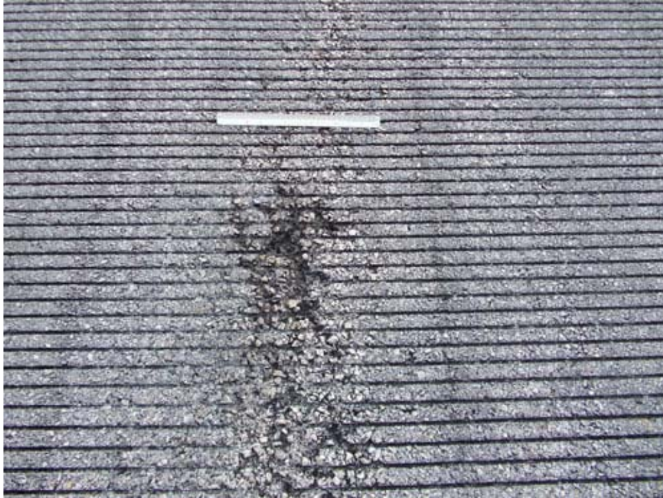
Runway 9L-27R Section 6115 SU 458: High Severity Weathering (November 14, 2007)
