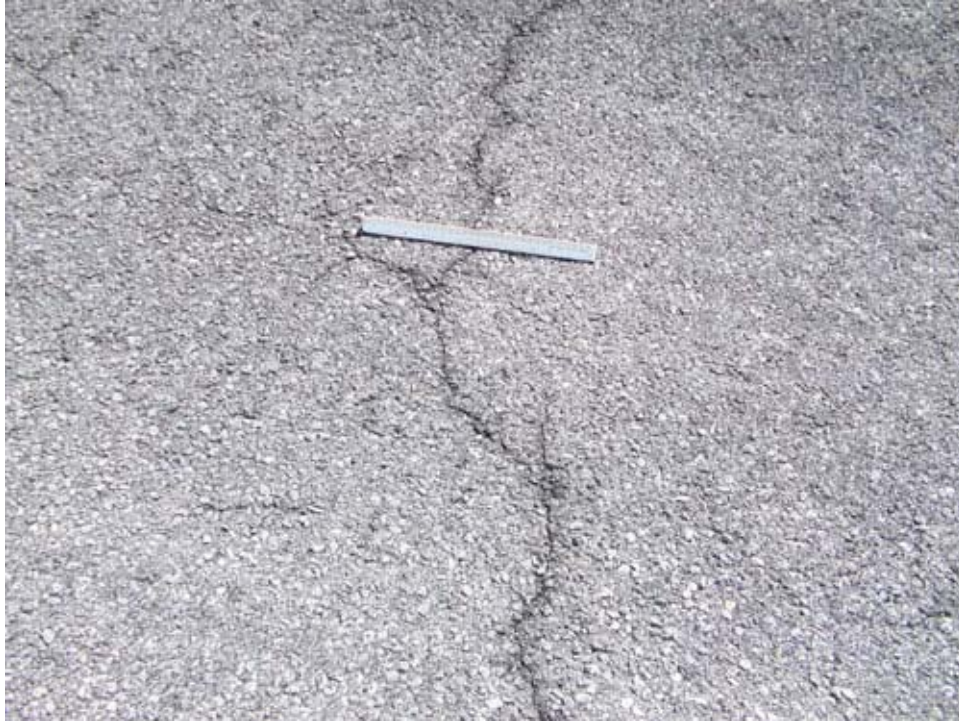
TW Y Section 2610 SU 101: Low Severity L/T Cracking (November 14, 2007)
