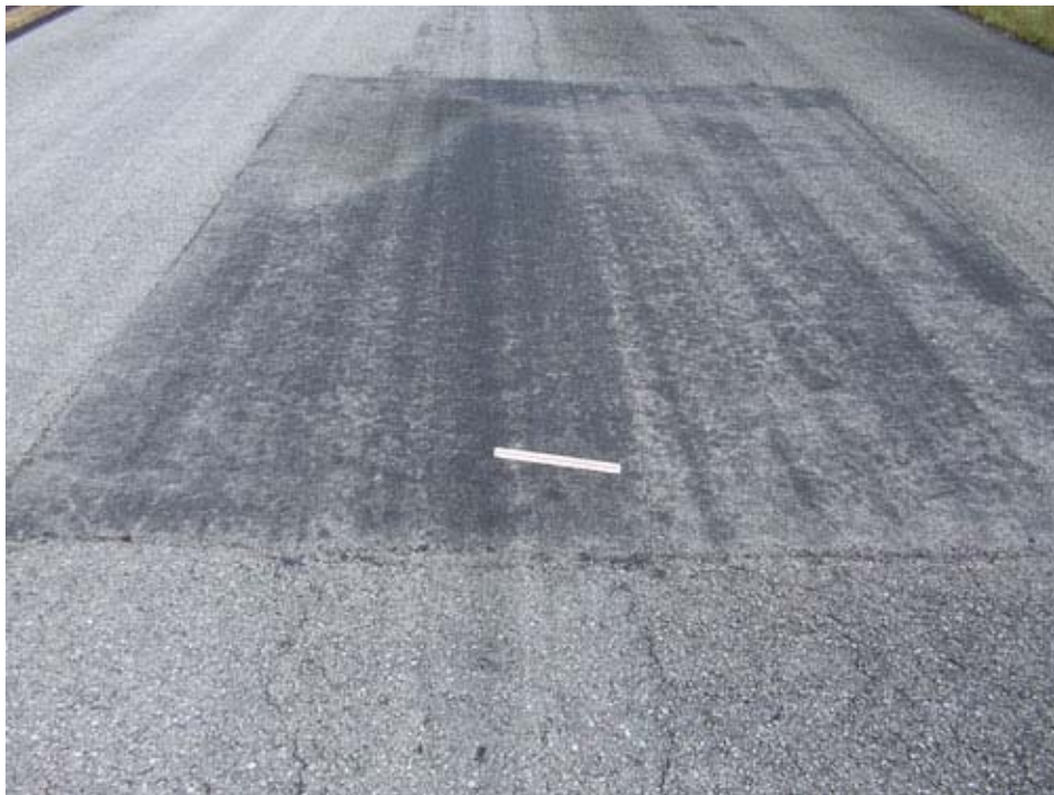
TW Y Section 2610 SU 128: Low Severity Patching (November 14, 2007)
