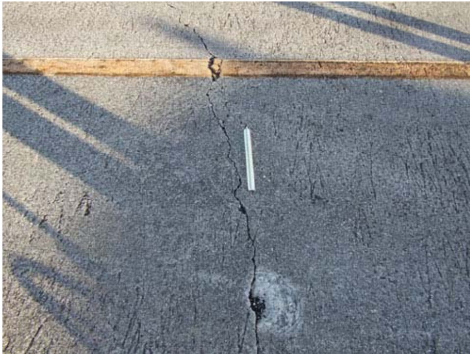
AP Center Section 4120 SU 601: Medium Severity Linear Cracking (November 14, 2007)
