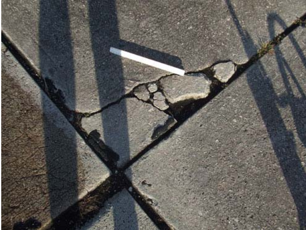
AP E Section 4110 SU 302: High Severity Corner Spalling (November 14, 2007)
