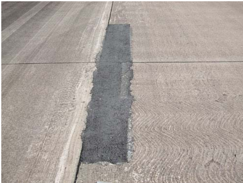
TW N Section 1410 SU 104: Low Severity Large Patch (November 14, 2007)
