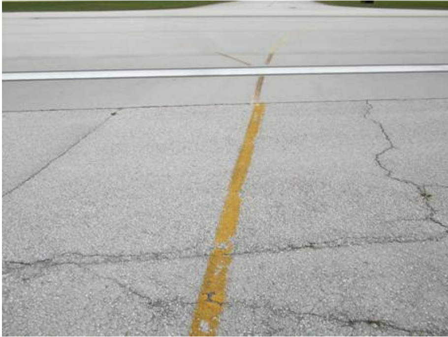
TW D Section 415 SU 413: Medium Severity L/T Cracking (June 13, 2007)
