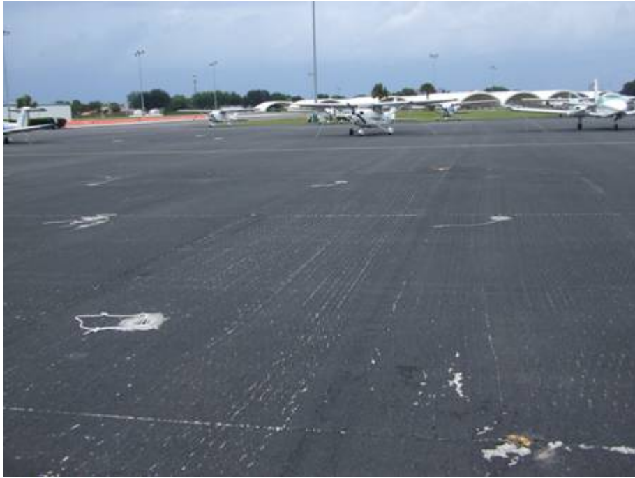
AP N Section 4145 SU 363: Low Severity Weathering (June 13, 2007)
