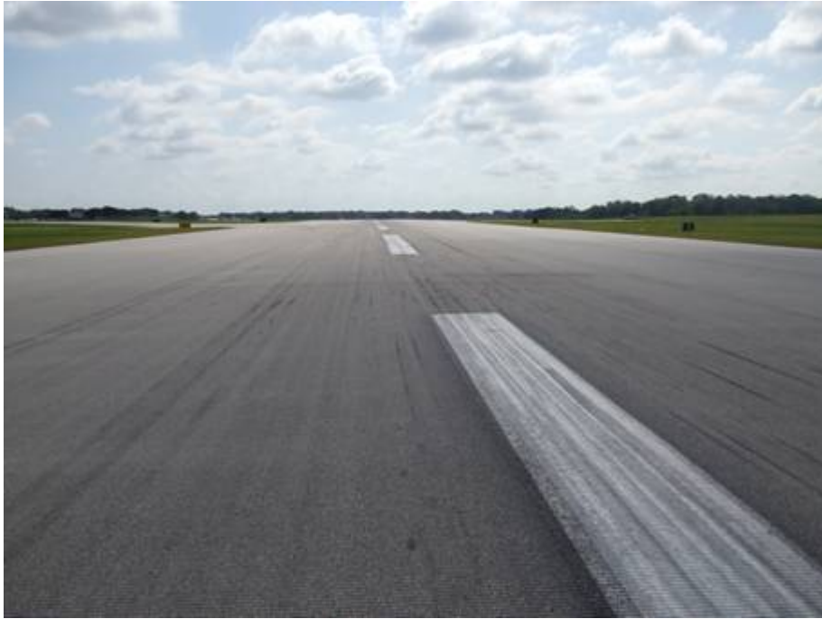
RW 7-25 Section 6115 SU 371: Low Severity L/T Cracking (June 13, 2007)
