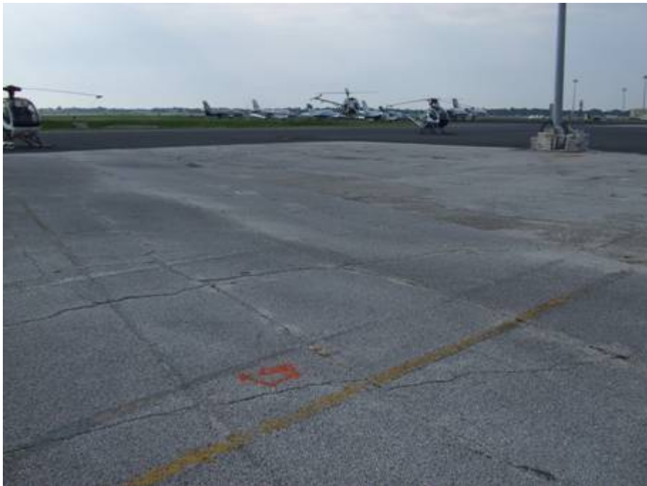
AP W Section 4655 SU 207: Medium Severity L/T Cracking (June 13, 2007)
