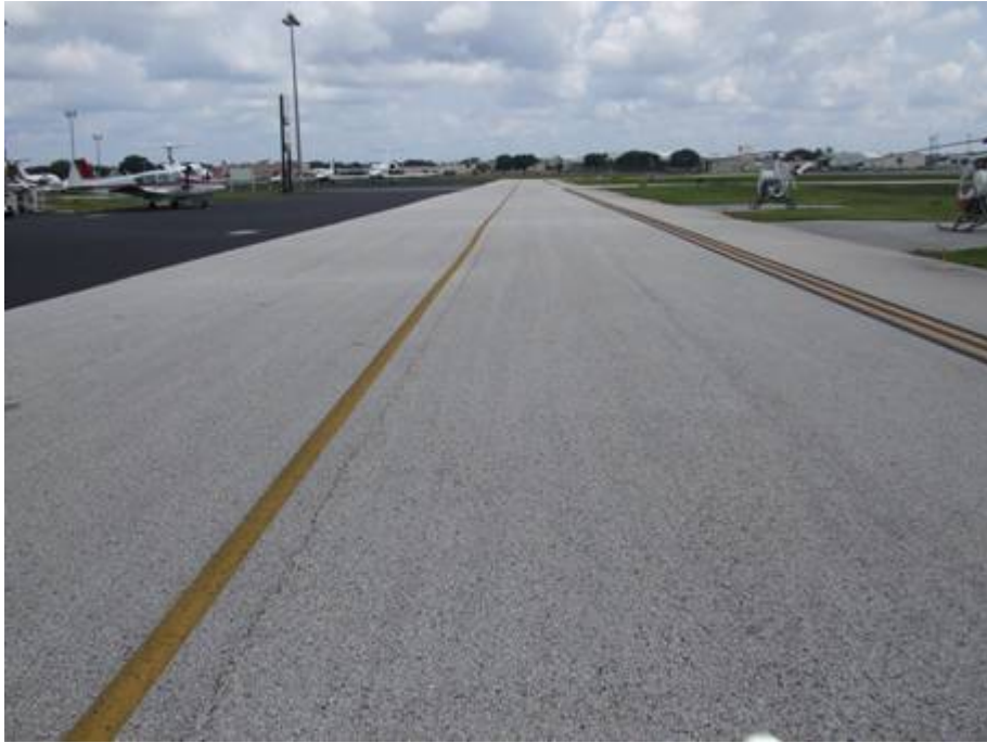
TW H Section 806 SU 103: Low Severity L/T Cracking (June 13, 2007)
