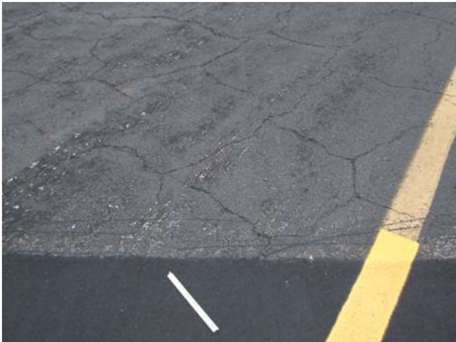
TW E Section 555 SU 144: Low Severity Block Cracking (June 13, 2007)
