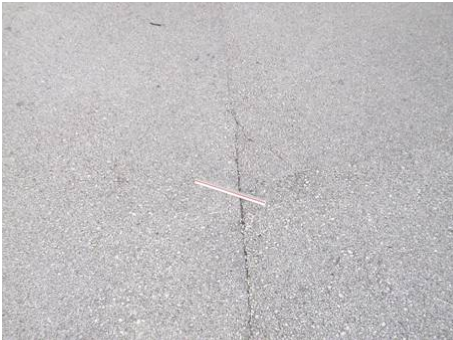
TW A Section 110 SU 99: Low Severity L/T Cracking (June 13, 2007)
