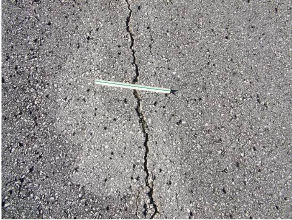
RW 4-22 Section 6205 SU 308: Low to Medium Severity L/T Cracking (January 30, 2008)
