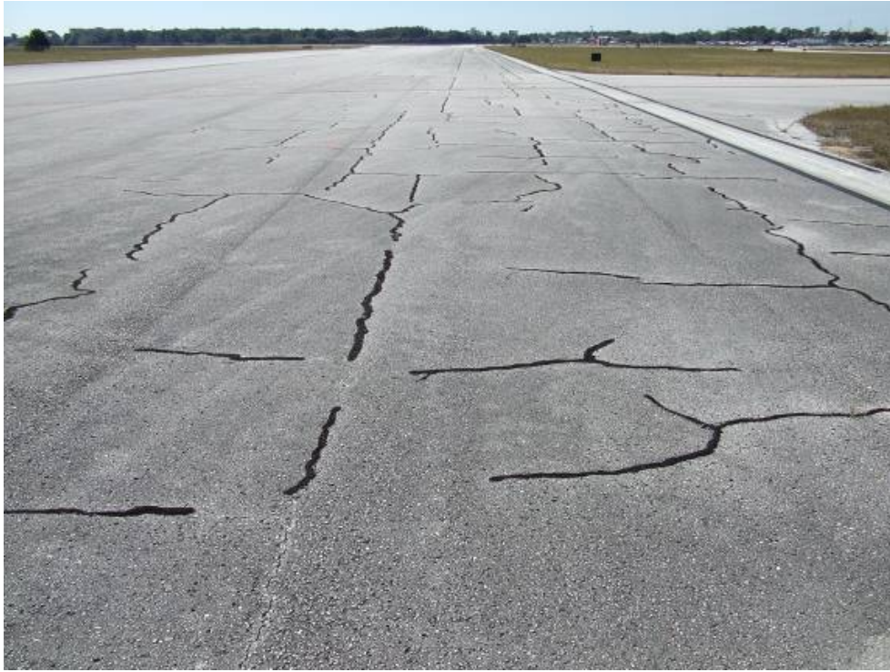
RW 4-22 Section 6210 SU 168: Low Severity L/T Cracking (January 30, 2008)
