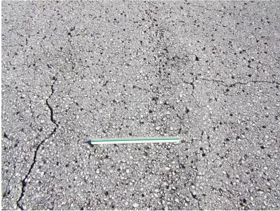
RW 4-22 Section 6205 SU 308: High Severity Weathering (January 30, 2008)
