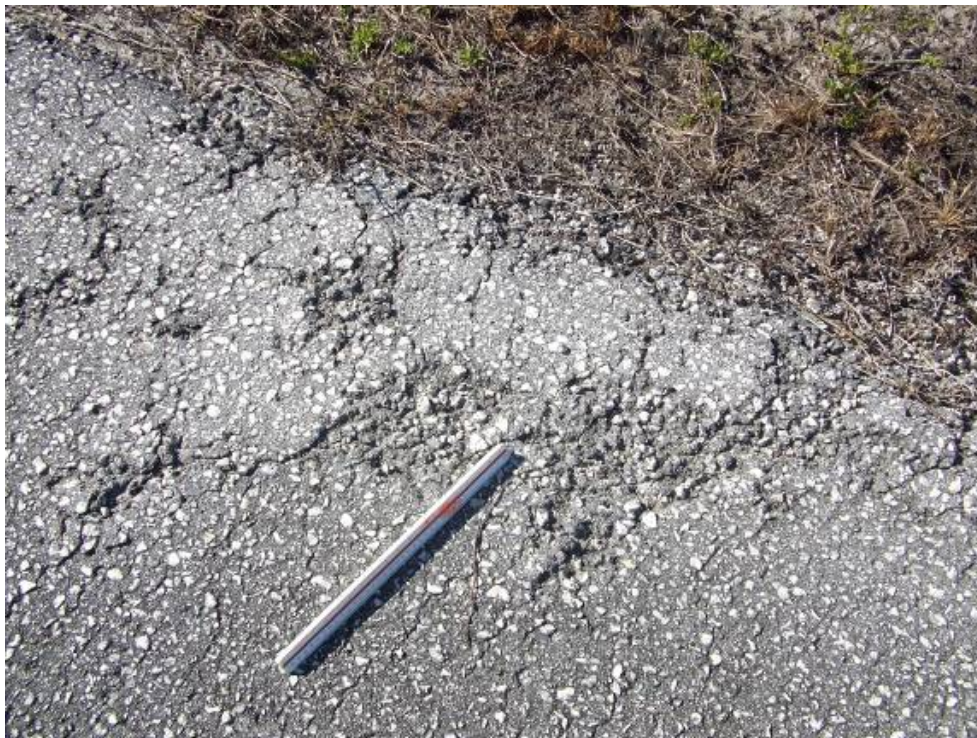
TW M Section 1325 SU 106: High Severity Weathering (January 30, 2008)
