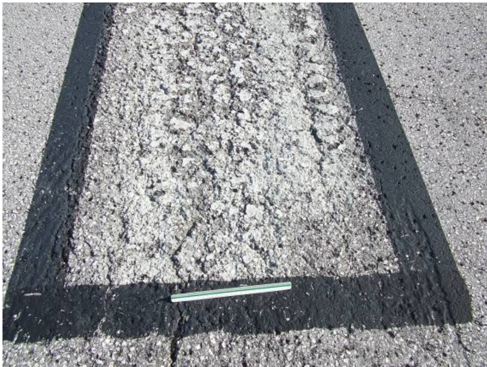
RW 4-22 Section 6205 SU 308: Medium Severity Weathering (January 30, 2008)
