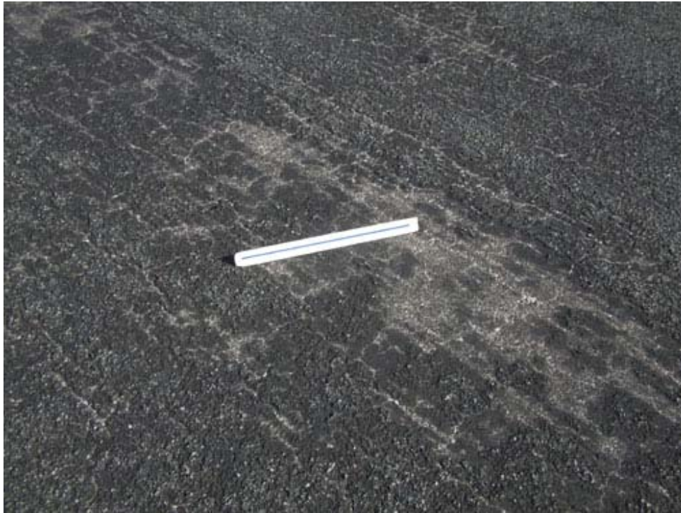
Apron S Section 4510 SU 502: Medium Severity Weathering (November 14, 2007)
