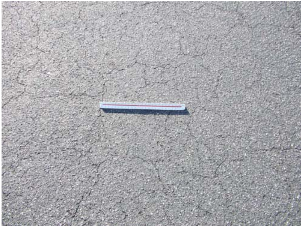
Apron S Section 4510 SU 502: Low Severity Weathering (November 14, 2007)
