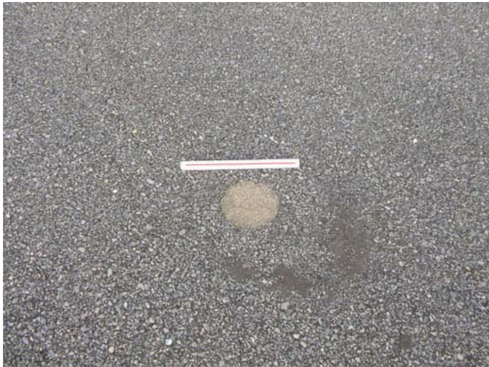
Taxiway A1 Section 120 SU 102: Low Severity Patching (November 14, 2007)
