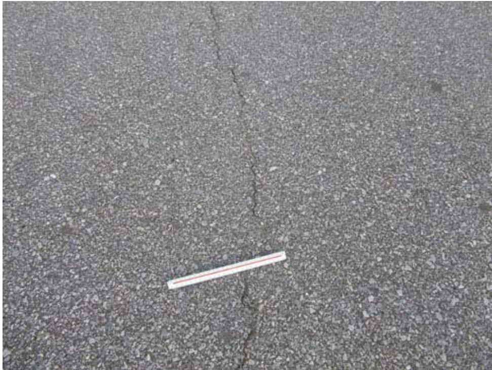
Taxiway A Section 115 SU 163: Low Severity L/T Cracking (November 14, 2007)
