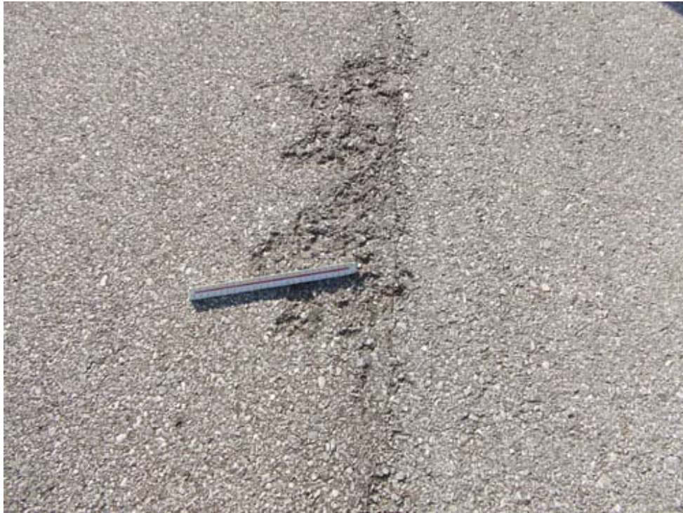
AP S Section 4505 SU 401: High Severity Weathering (November 14, 2007)
