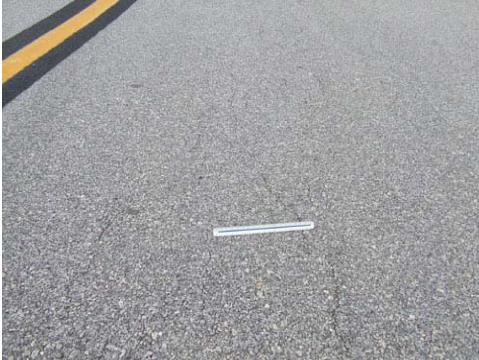
Taxiway A1 Section 120 SU 102: Low Severity L/T Cracking (November 14, 2007)
