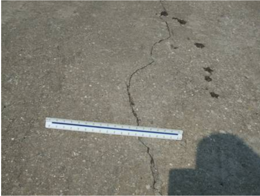
AP Cargo Section 4110 SU 153: Medium Severity Linear Cracking (August 13, 2007)
