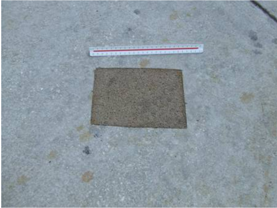
AP S Section 4410 SU 206: Low Severity Small Patch (August 13, 2007)
