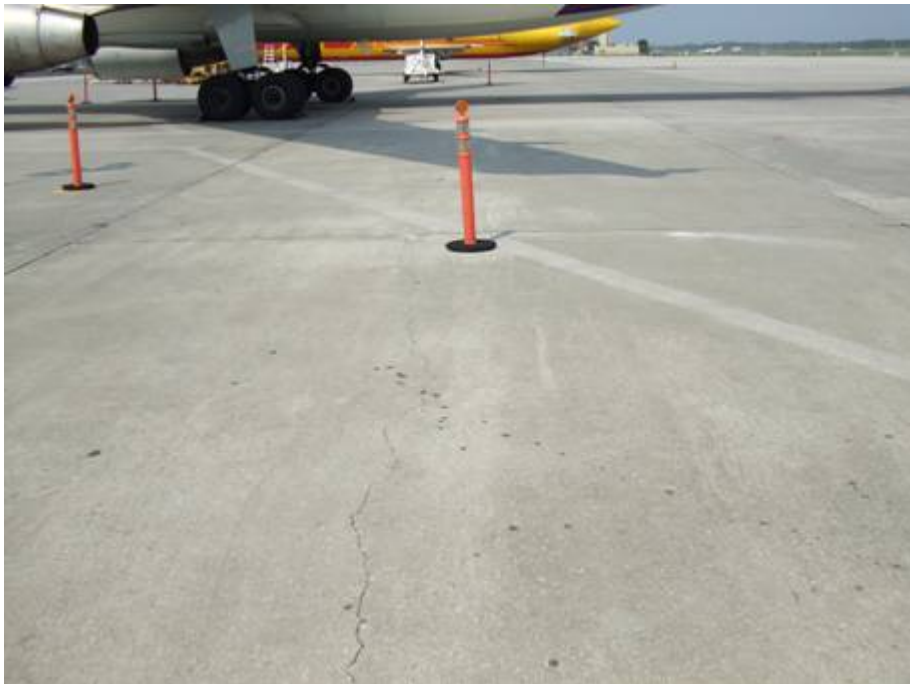
AP Cargo Section 4110 SU 153: Low Severity Linear Cracking (August 13, 2007)
