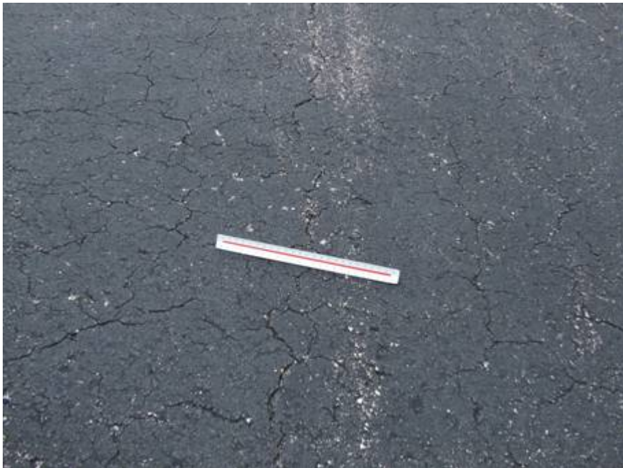
AP FBO Section 4205 SU 452: Low Severity Weathering (August 13, 2007)
