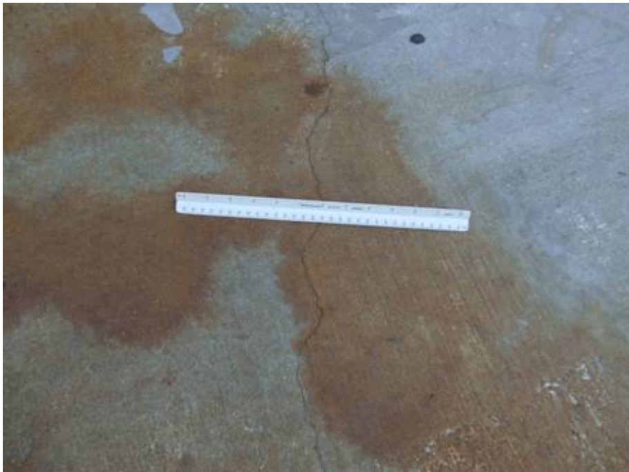
AP S Section 4410 SU 206: Shrinkage Cracking (August 13, 2007)
