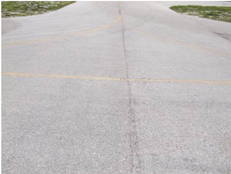
AP Section 4135 SU 200: Low Severity L/T Cracking (July 25, 2007)
