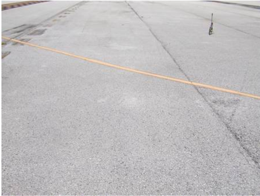
TW C Section 310 SU 150: Medium Severity L/T Cracking (July 25, 2007)
