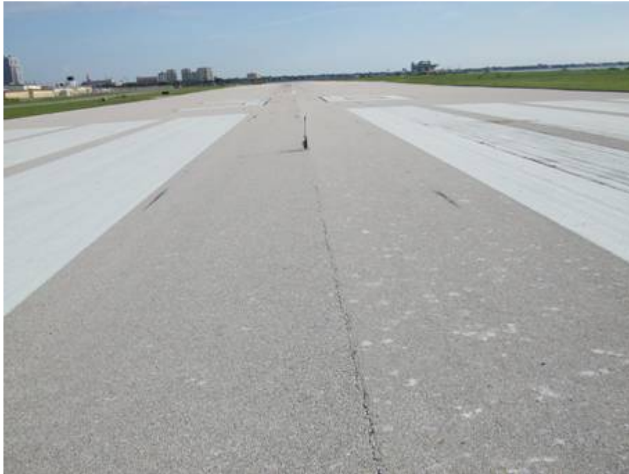
RW 18-36 Section 6105 SU 301: Low Severity L/T Cracking (July 25, 2007)
