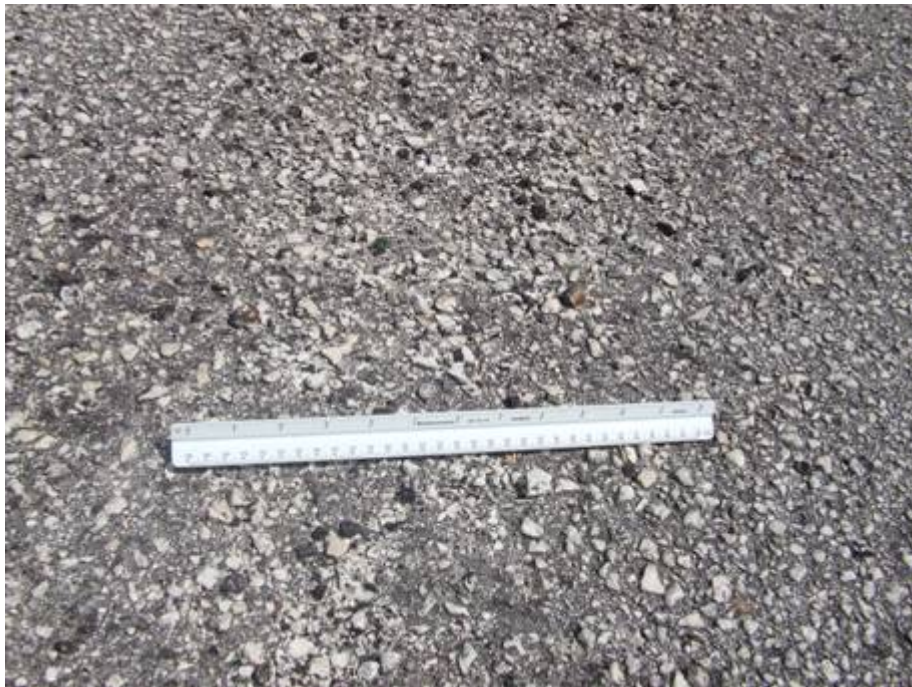
TW B Section 254 SU 122: Low Severity Weathering (July 25, 2007)
