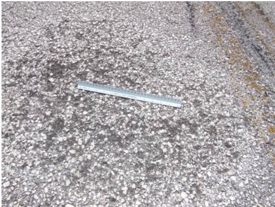
TW C Section 310 SU 150: Medium Severity Weathering (July 25, 2007)
