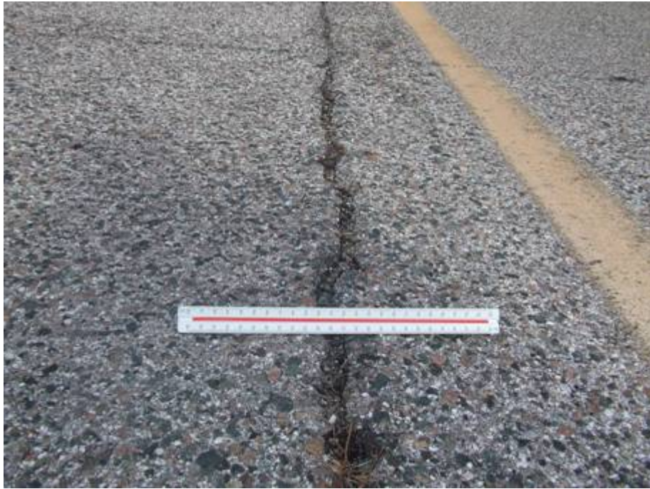
TW B Section 251 SU 100: Medium Severity L/T Cracking (July 25, 2007)
