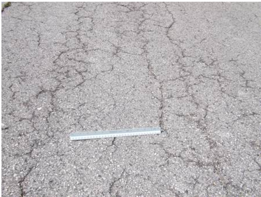
TW CONN C Section 605 SU 104: Low Severity Alligator Cracking (July 25, 2007)
