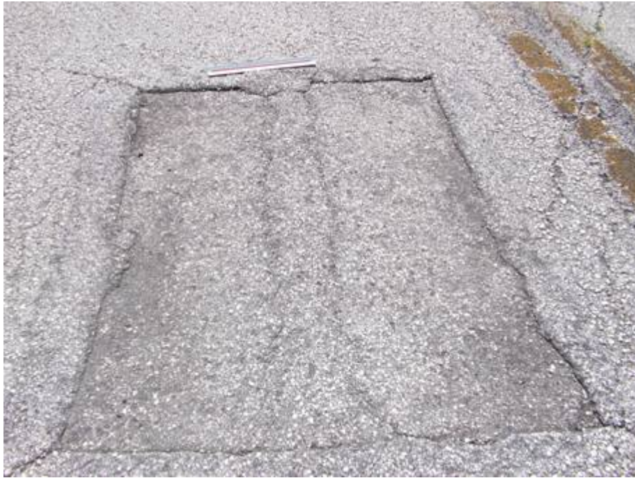
TW C Section 310 SU 150: Medium Severity Patching (July 25, 2007)
