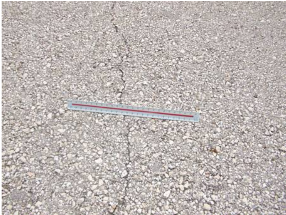
TW A Section 150 SU 100: Low Severity L/T Cracking (July 25, 2007)
