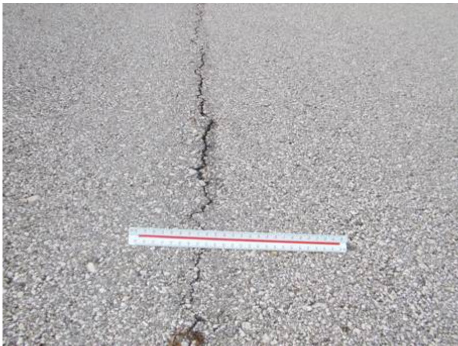
RW 18-36 Section 6110 SU 504: Low Severity L/T Cracking (July 25, 2007)
