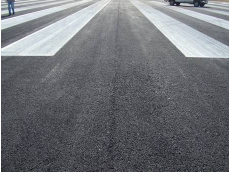
RW 9-27 Section 6105 SU 403: Low Severity Weathering (September 17, 2007)
