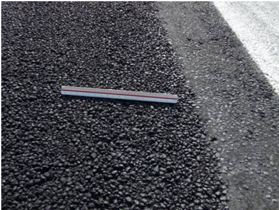
RW 9-27 Section 6105 SU 403: Medium Severity Weathering (September 17, 2007)
