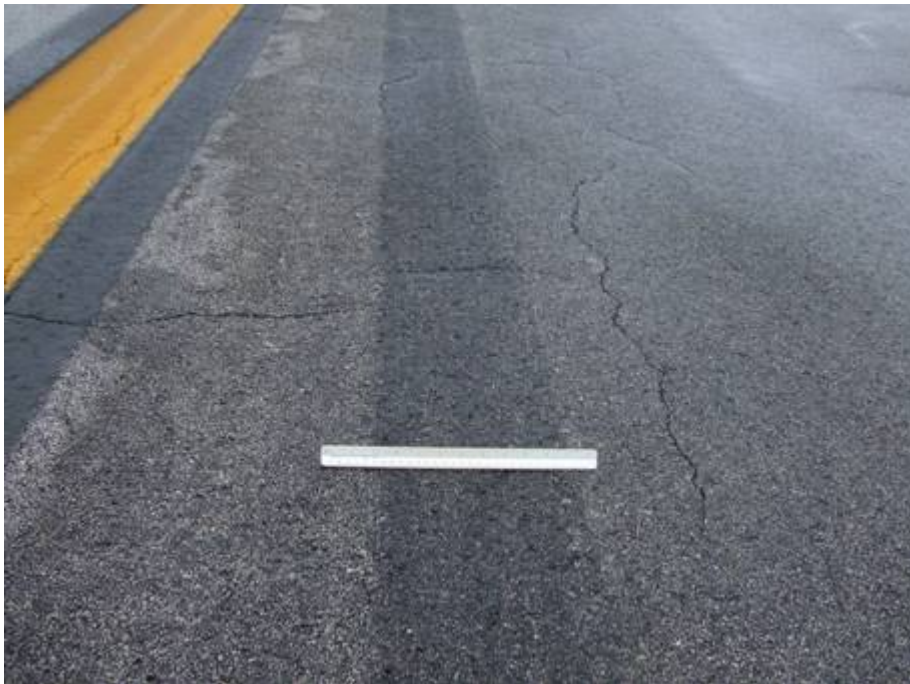
TW A Section 110 SU 111: Low Severity L/T Cracking (September 17, 2007)
