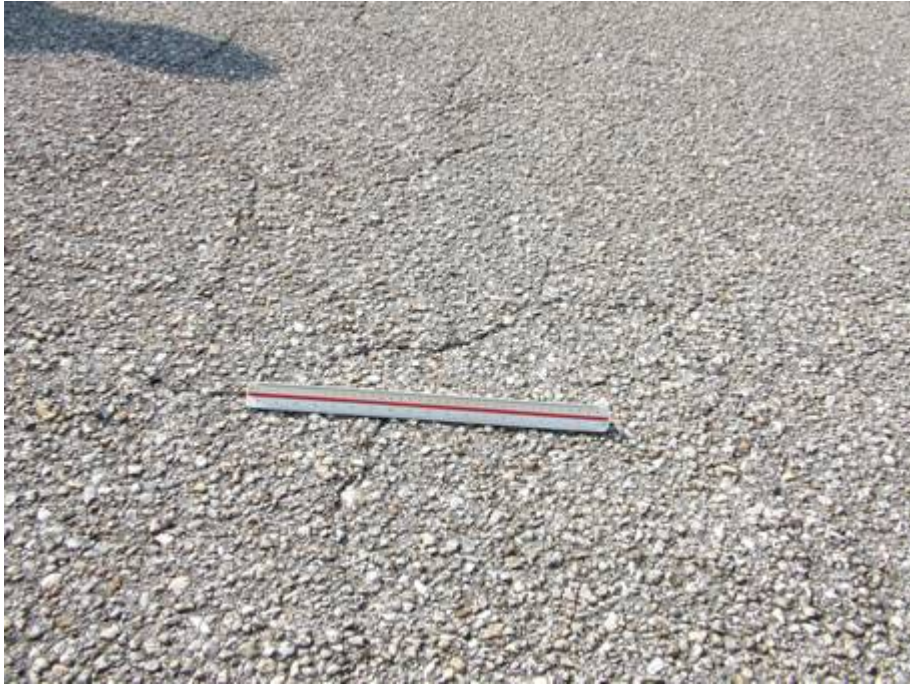
TW A6 Section 170 SU 602: Low Severity Block Cracking (September 17, 2007)
