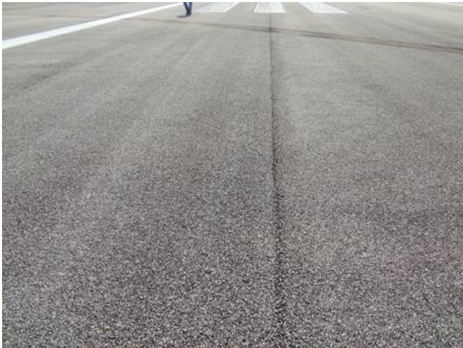
RW 9-27 Section 6110 SU 198: Construction Joint (September 17, 2007)
