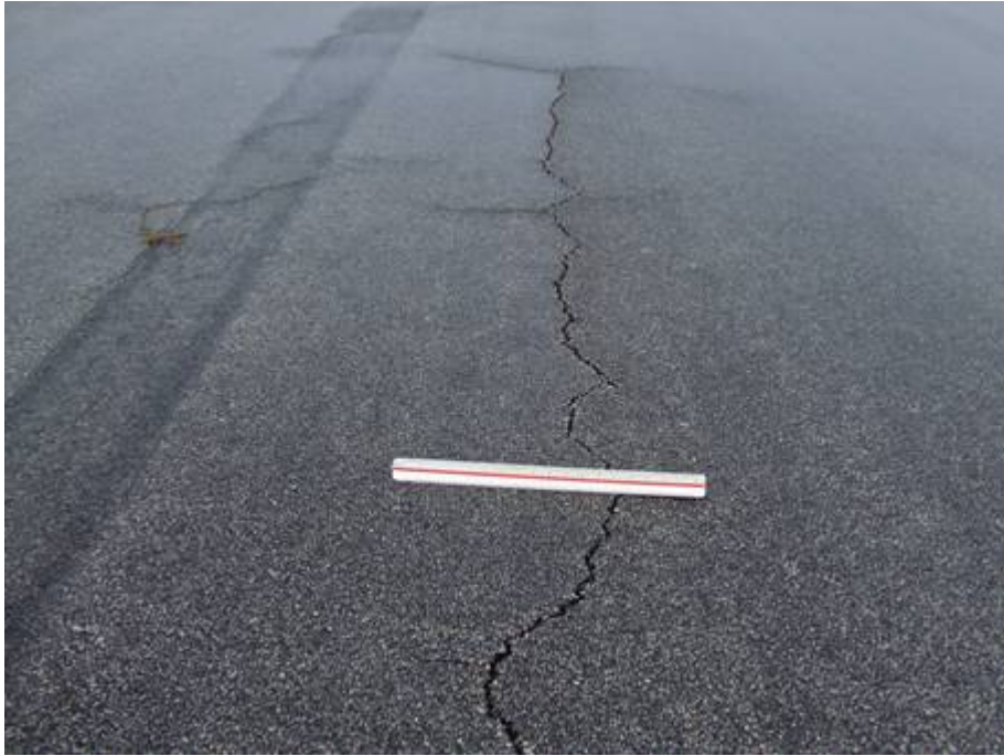
TW A Section 110 SU 106: Low Severity L/T Cracking (September 17, 2007)
