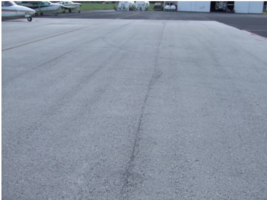
AP Section 4105 SU 202: Low Severity L/T Cracking (July 9, 2007)
