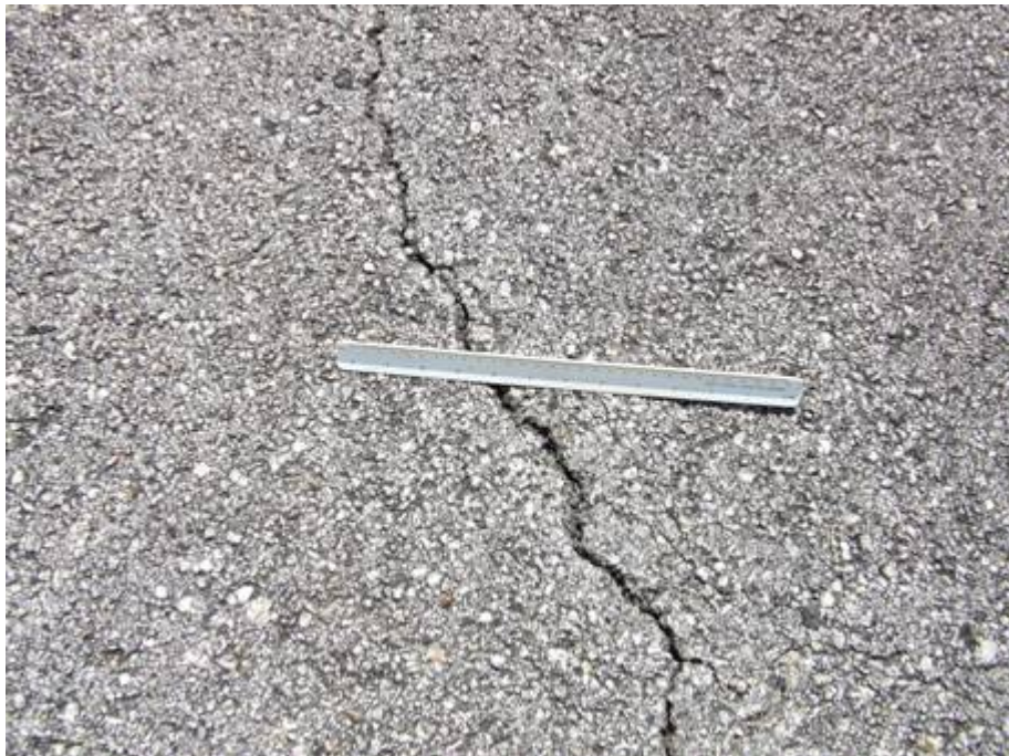
TW D Section 405 SU 100: Low Severity L/T Cracking (July 9, 2007)
