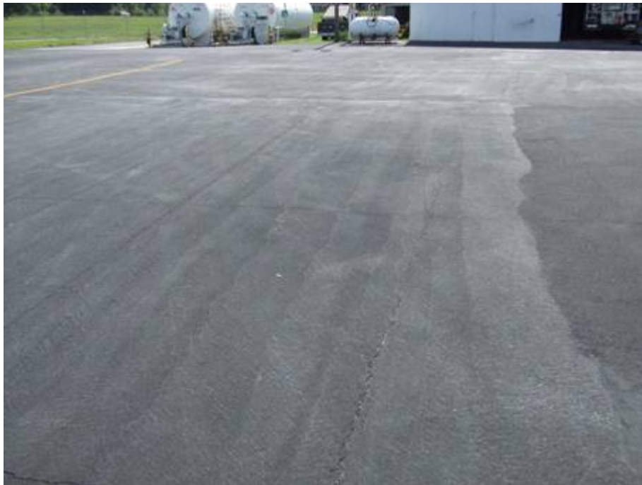
AP Section 4107 SU 203: Low Severity L/T Cracking (July 9, 2007)
