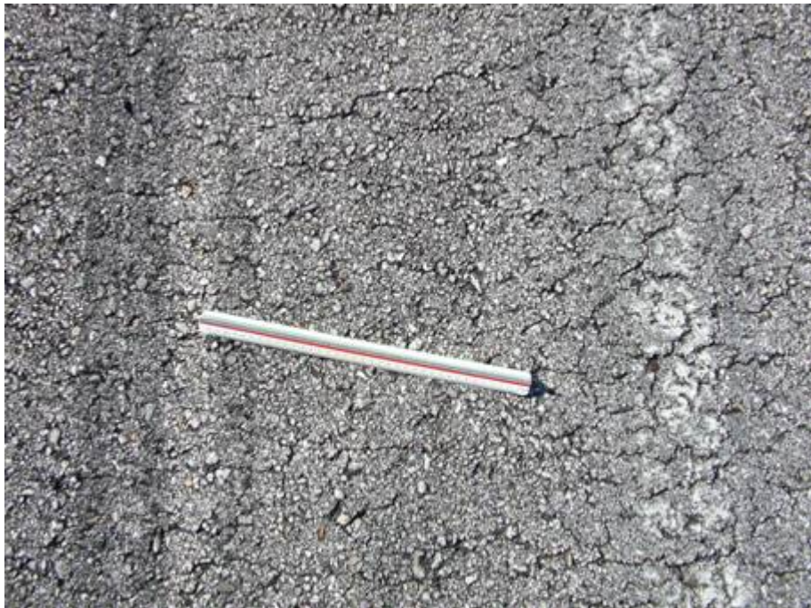
RW 15-33 Section 6105 SU 105: Low Severity Weathering (July 9, 2007)
