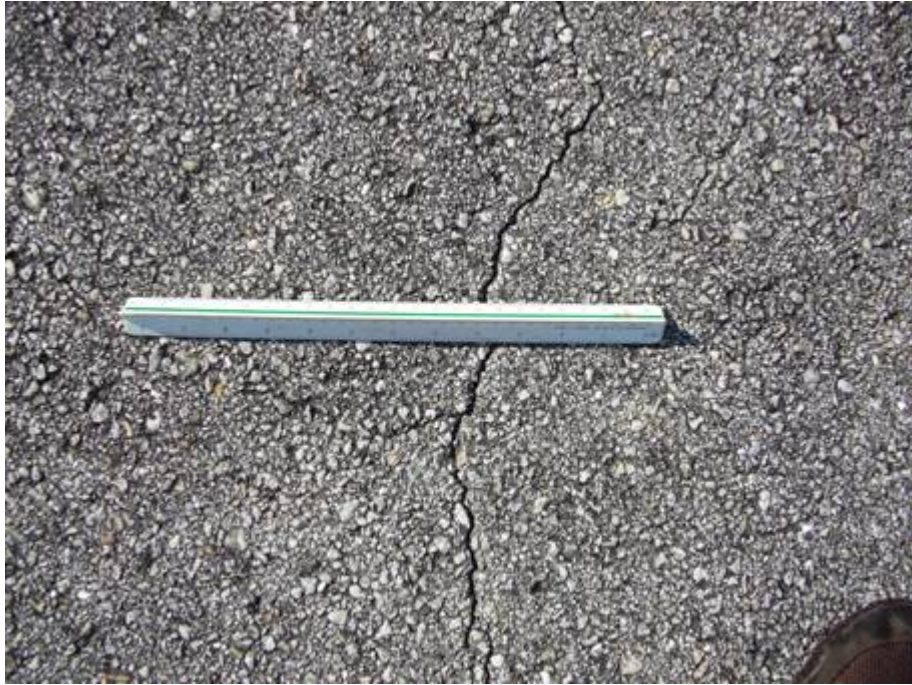
RW 15-33 Section 6105 SU 100: Low Severity L/T Cracking (July 9, 2007)
