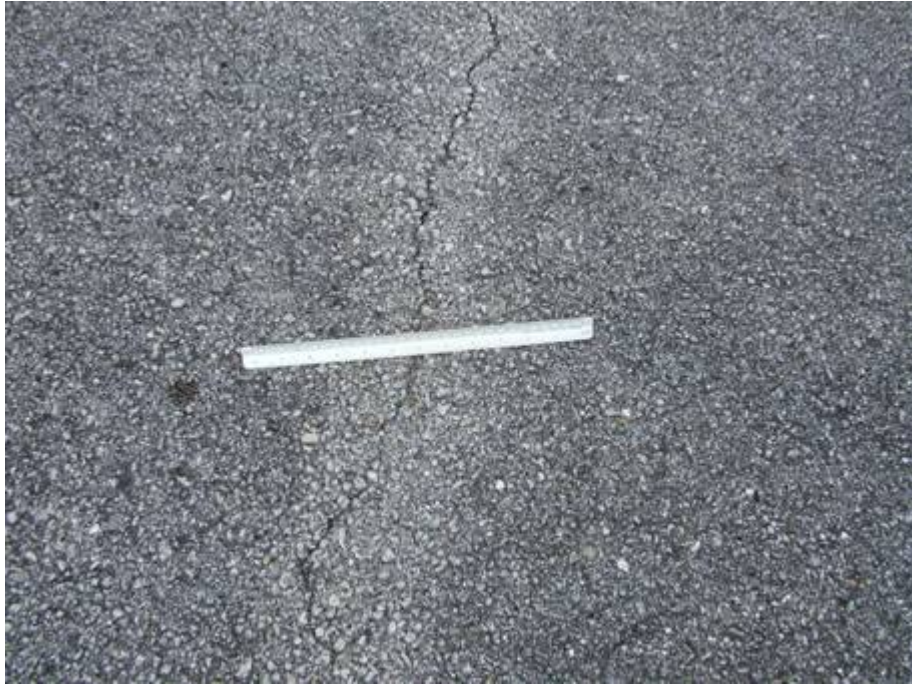
TW C Section 305 SU 100: Low Severity L/T Cracking (July 9, 2007)
