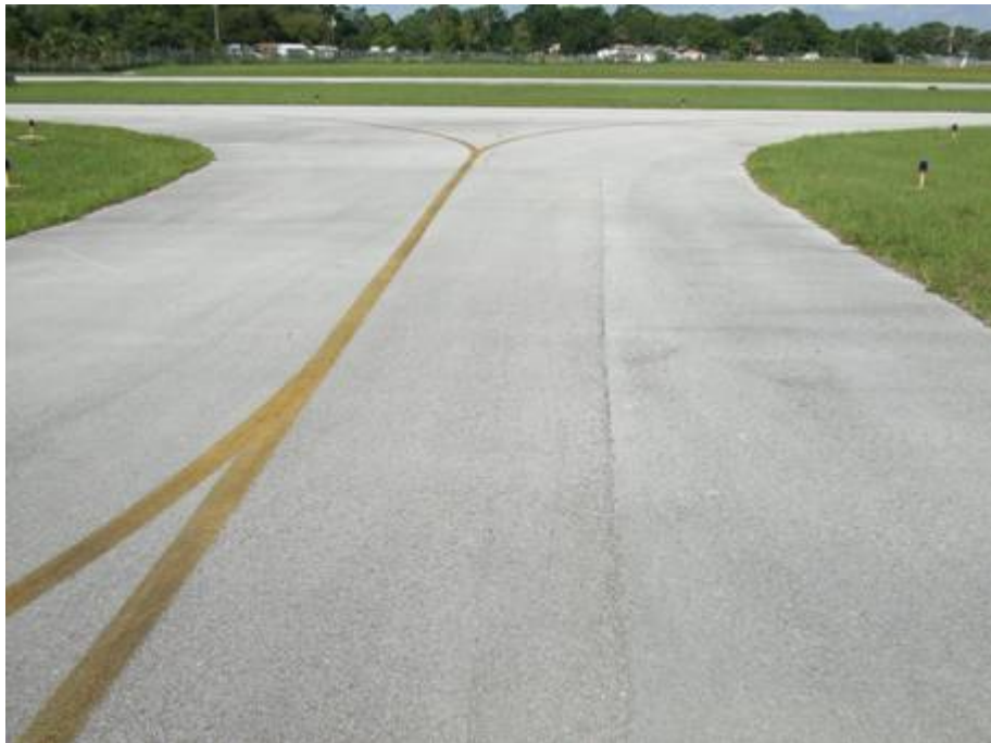
TW AP Section 115 SU 115: Low Severity L/T Cracking (July 9, 2007)
