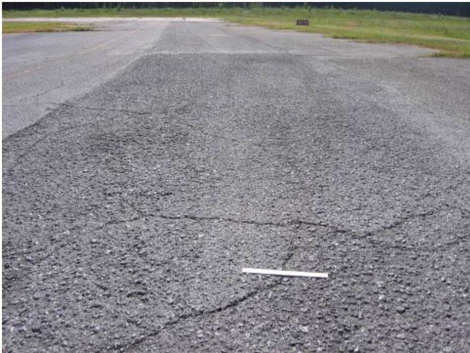
TW C Section 305 SU 104: Medium Severity Weathering (October 11, 2006)
