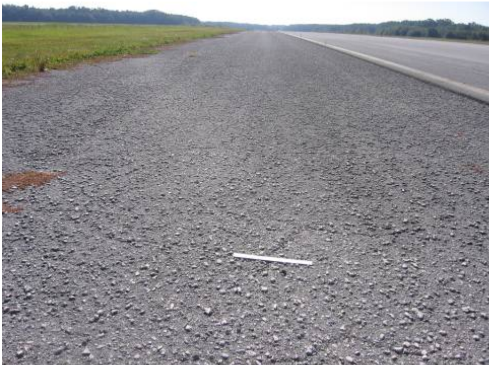
RW 14-32 Section 6220 SU 584: Medium Severity Weathering (October 11, 2006)
