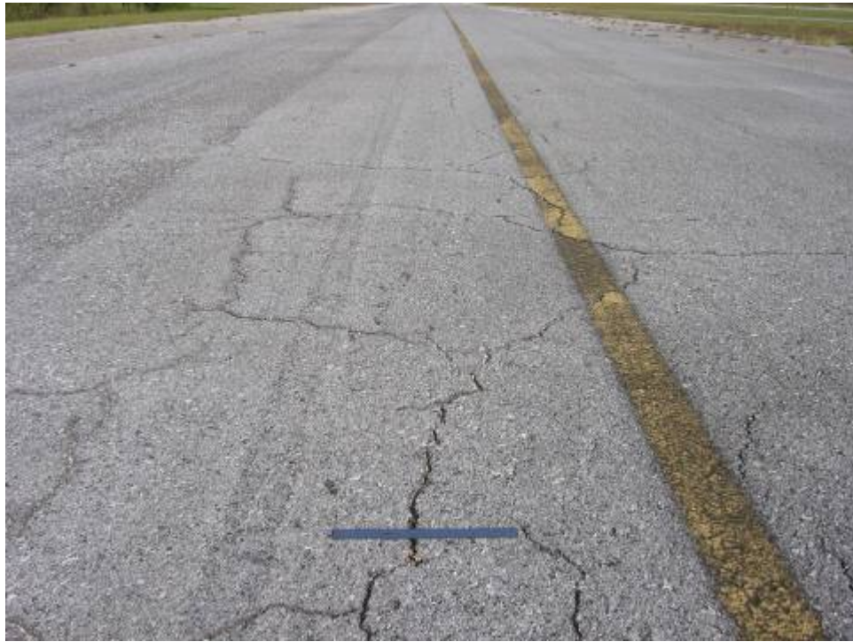
TW C Section 305 SU 131: Low Severity Block Cracking (October 11, 2006)
