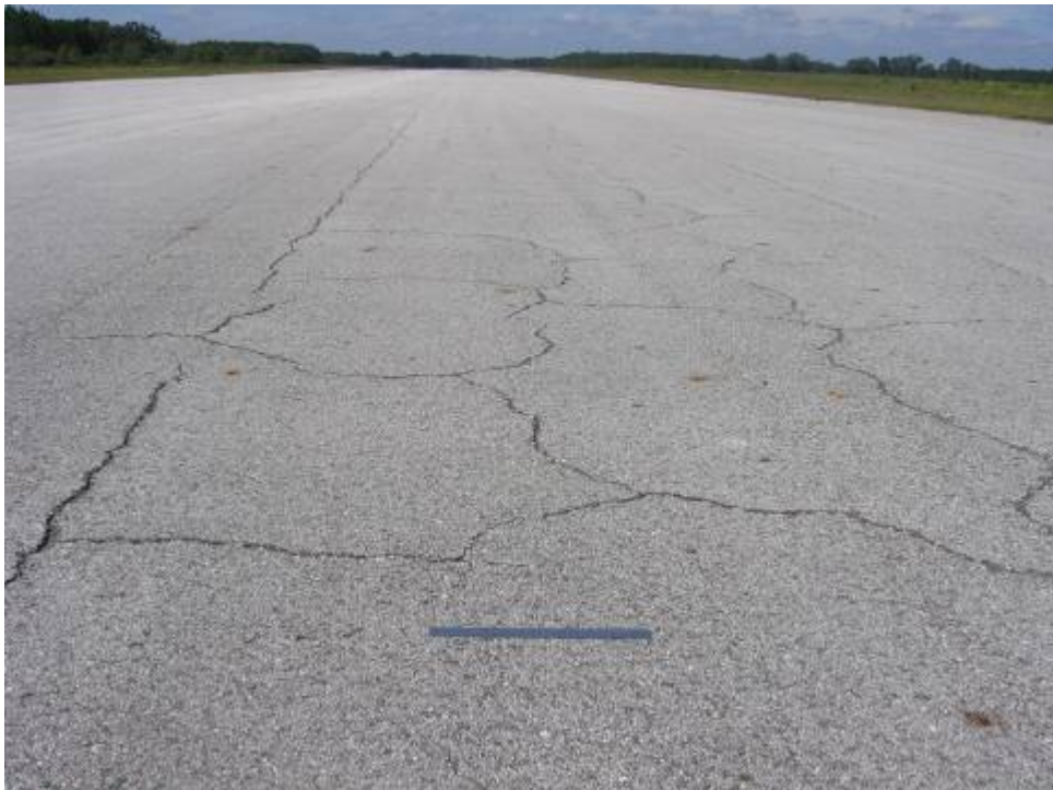
RW 14-32 Section 6215 SU 317: Low Severity Block Cracking (October 11, 2006)
