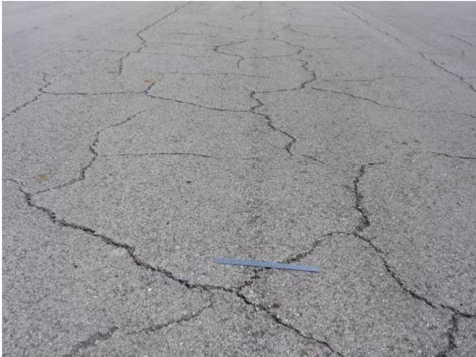
RW 14-32 Section 6215 SU 349: Medium Severity Block Cracking (October 11, 2006)
