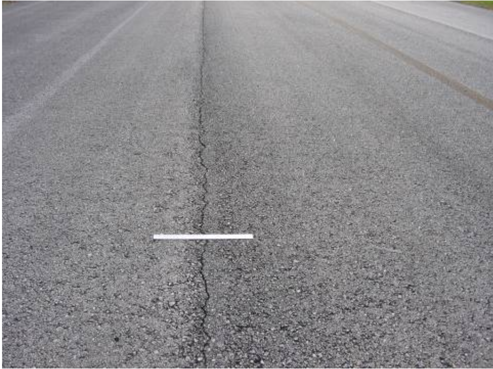
TW B Section 205 SU 104: Low Severity L/T Cracking (October 11, 2006)
