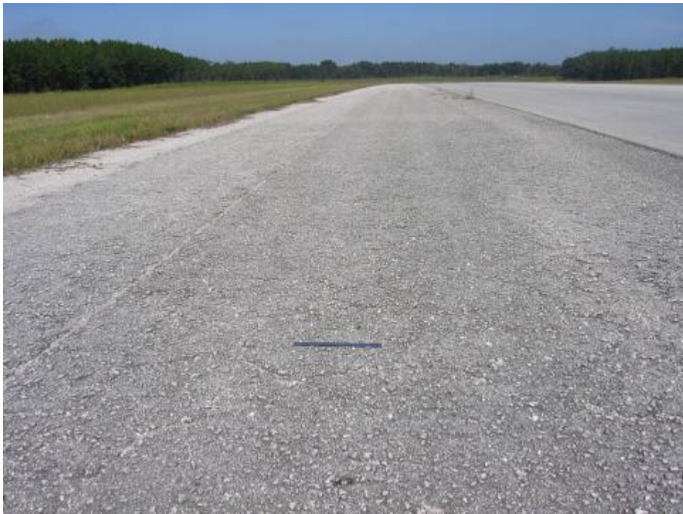
RW 14-32 Section 6220 SU 172: Low Severity Weathering (October 11, 2006)
