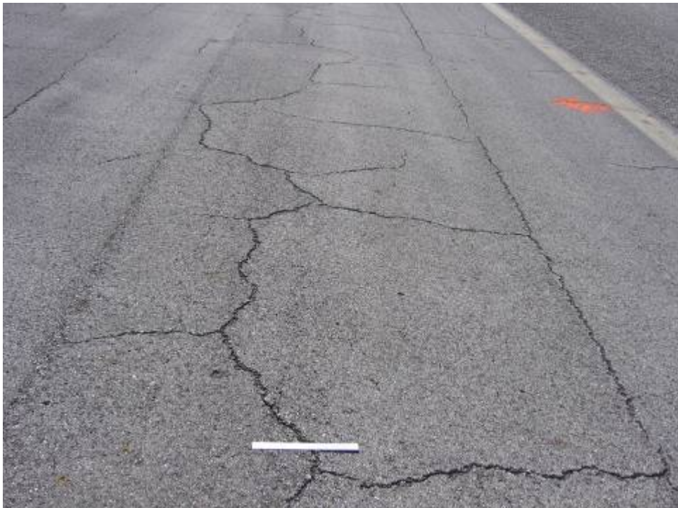
RW 14-32 Section 6215 SU 386: Low Severity Block Cracking (October 11, 2006)
