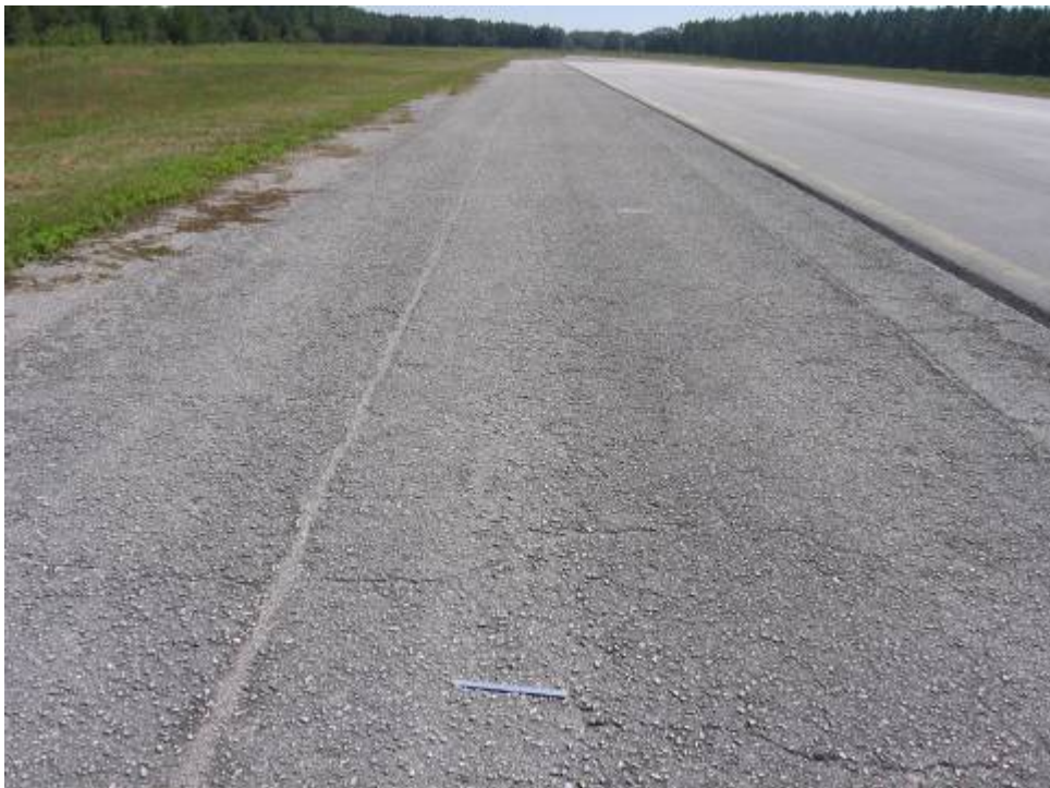
RW 14-32 Section 6220 SU 512: Low Severity Weathering (October 11, 2006)
