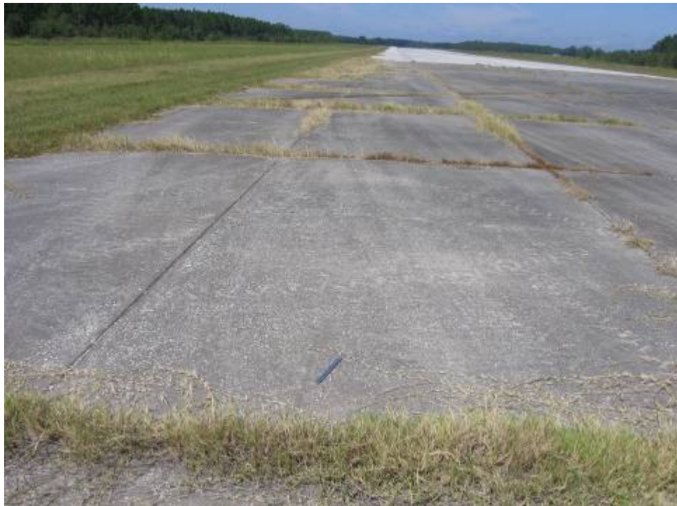
RW 14-32 Section 6210 SU 100: High Severity Joint Seal Damage (October 11, 2006)
