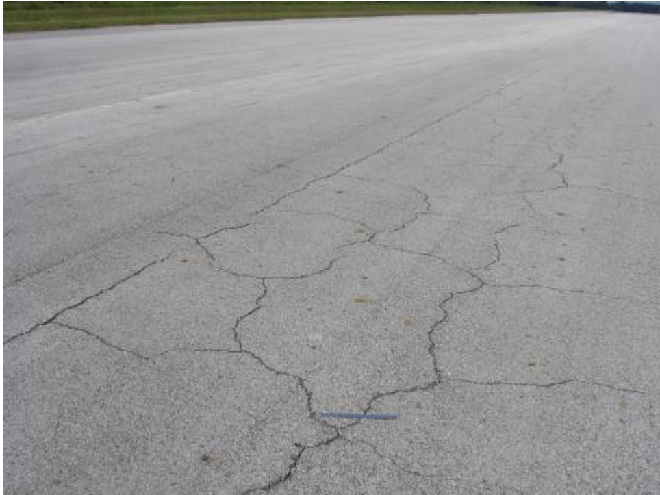
RW 14-32 Section 6220 SU 512: Low Severity Block Cracking (October 11, 2006)
