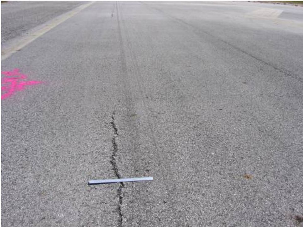
RW 14-32 Section 6215 SU 307: Medium Severity L/T Cracking (October 11, 2006)
