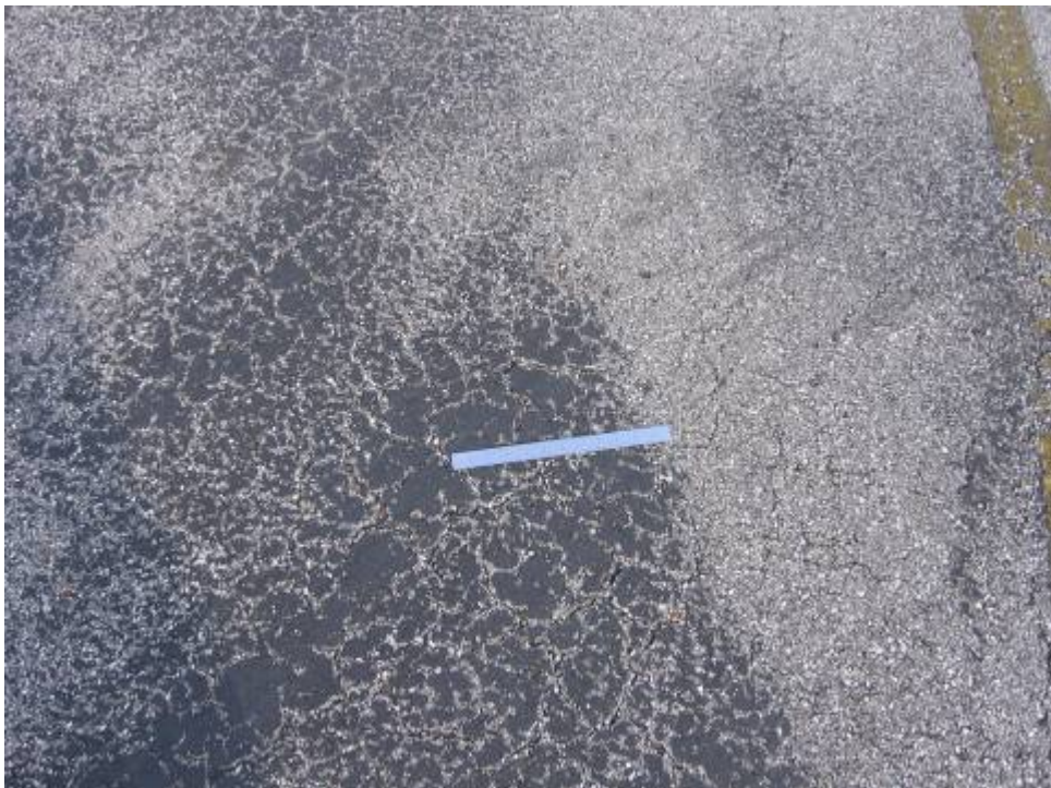
TW AP Section 405 SU 101: Medium Severity Weathering (October 11, 2006)
