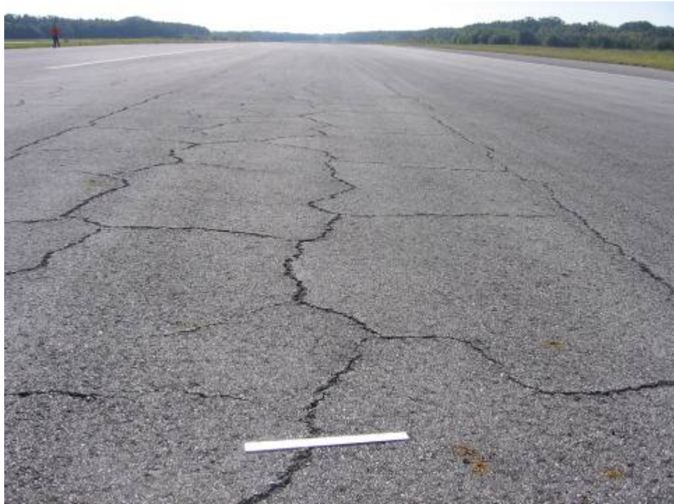
RW 14-32 Section 6215 SU 382: Medium Severity Block Cracking (October 11, 2006)
