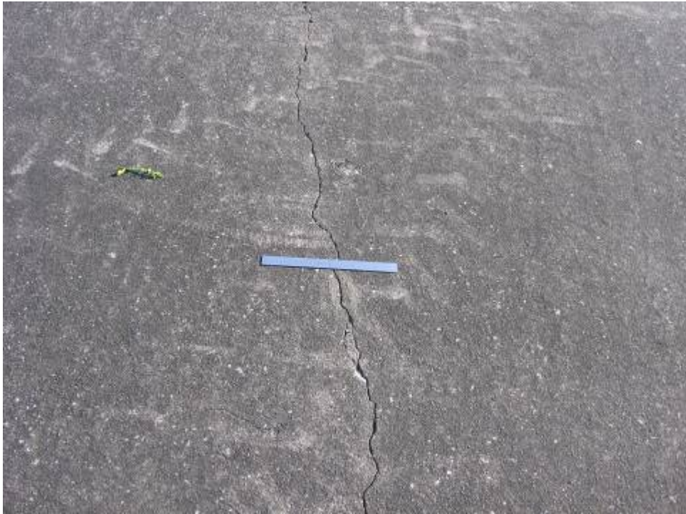
RW 14-32 Section 6240 SU 200: Low Severity Linear Cracking (October 10, 2006)
