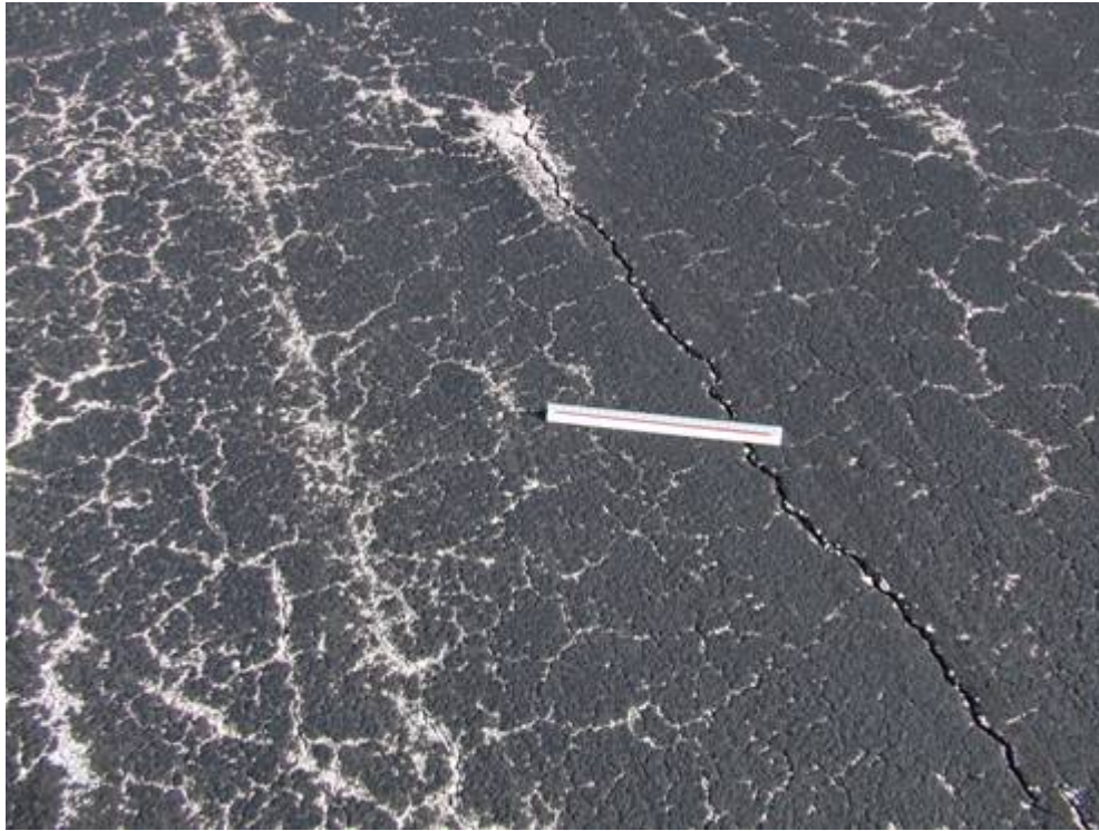
TW C Section 315 SU 701: Low Severity Weathering and L/T Cracking (June 25, 2007)
