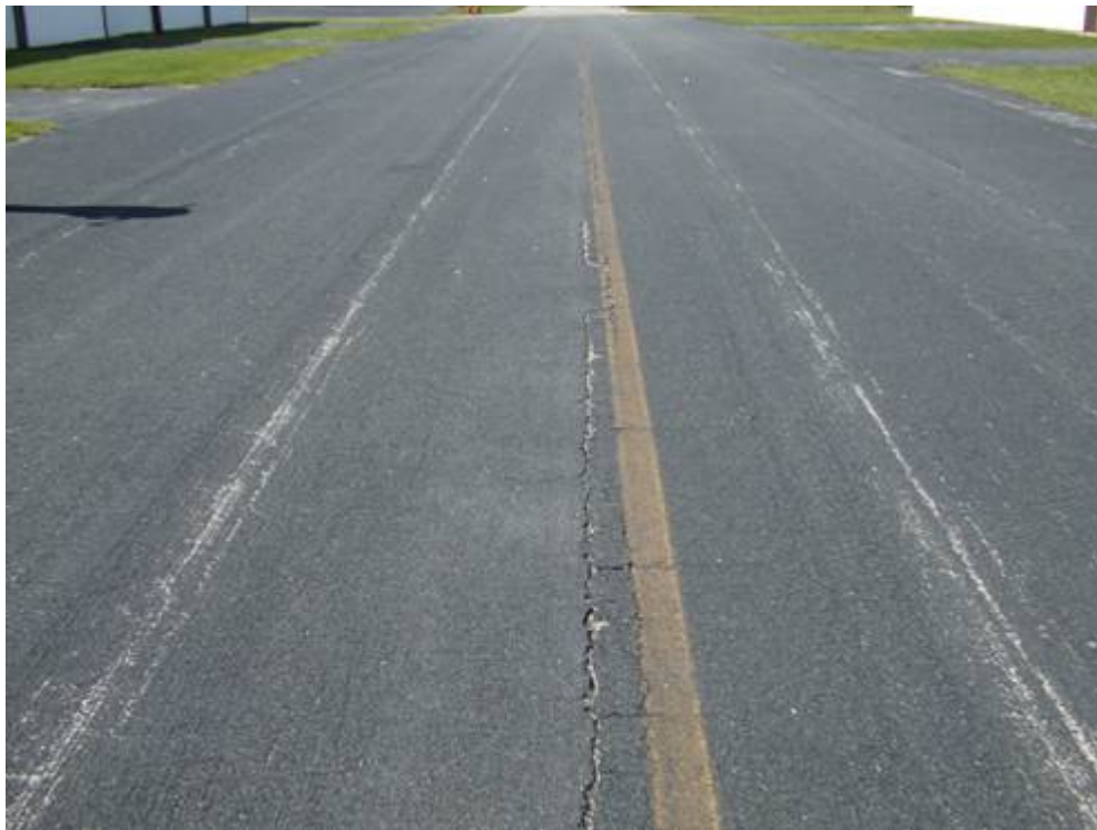
AP S Section 4227 SU 101: Medium Severity L/T Cracking (June 25, 2007)
