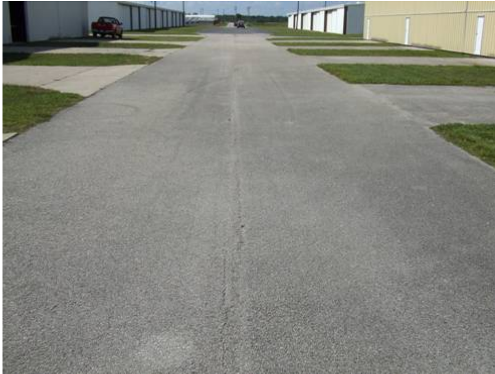
AP S Section 4240 SU 104: Low Severity L/T Cracking (June 25, 2007)
