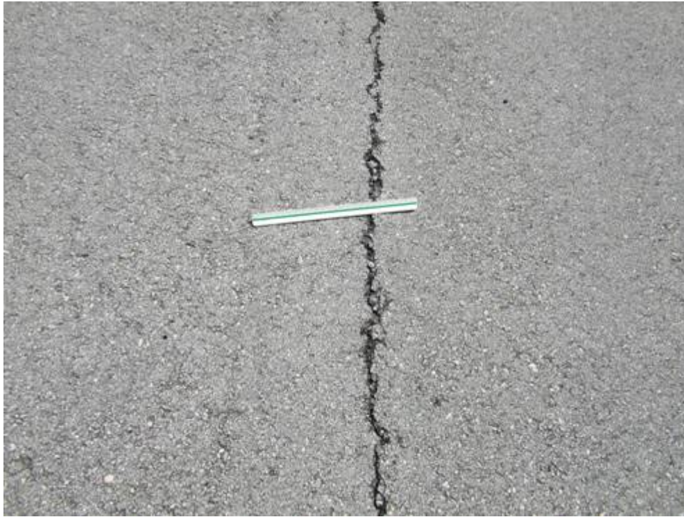
AP S Section 4215 SU 104: Medium Severity L/T Cracking (June 25, 2007)
