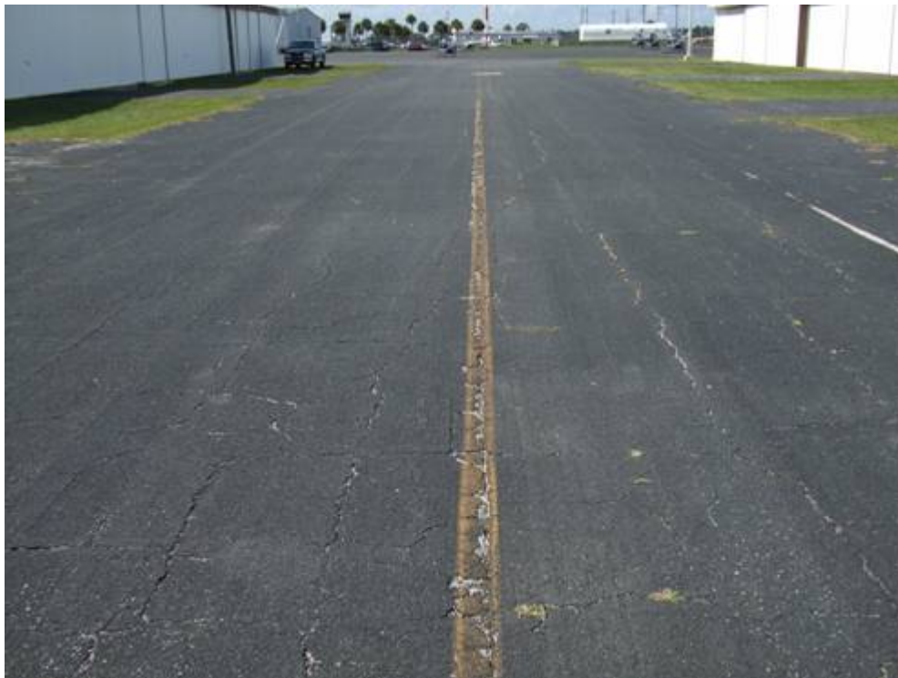
AP S Section 4226 SU 101: Medium Severity Block Cracking (June 25, 2007)
