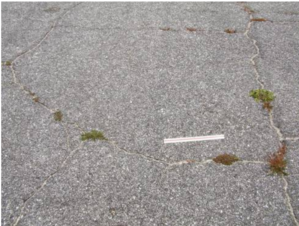
TW F 620 SU 304: Medium Severity Block Cracking (June 25, 2007)
