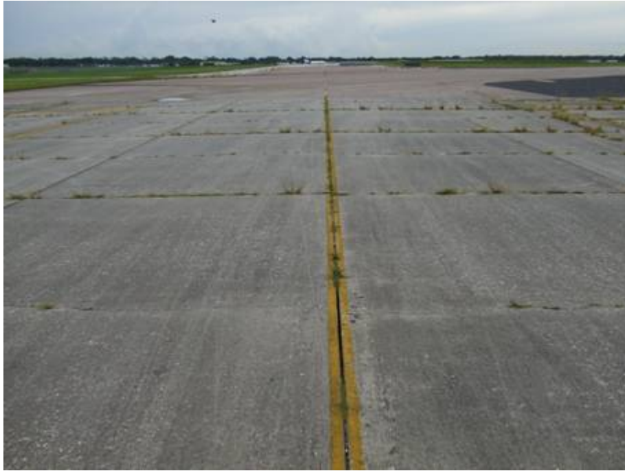
TW B Section 230 SU 135: High Severity Joint Seal Damage (July 25, 2007)
