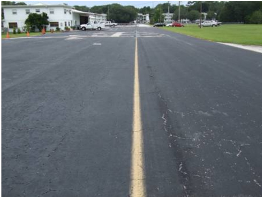
AP TW D Section 5205 SU 201: Low Severity Weathering (July 25, 2007)
