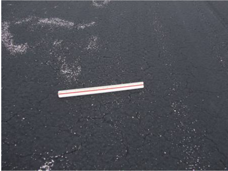
TW A Section 105 SU 141: Low Severity Weathering (July 25, 2007)
