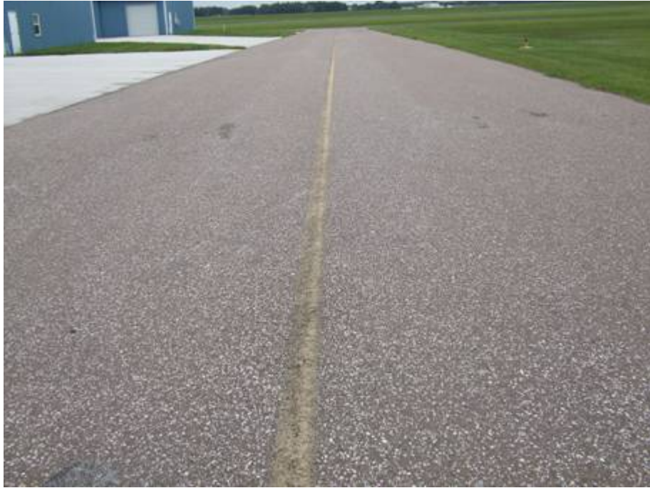
TW E Section 610 SU 104: Low Severity Weathering (July 25, 2007)
