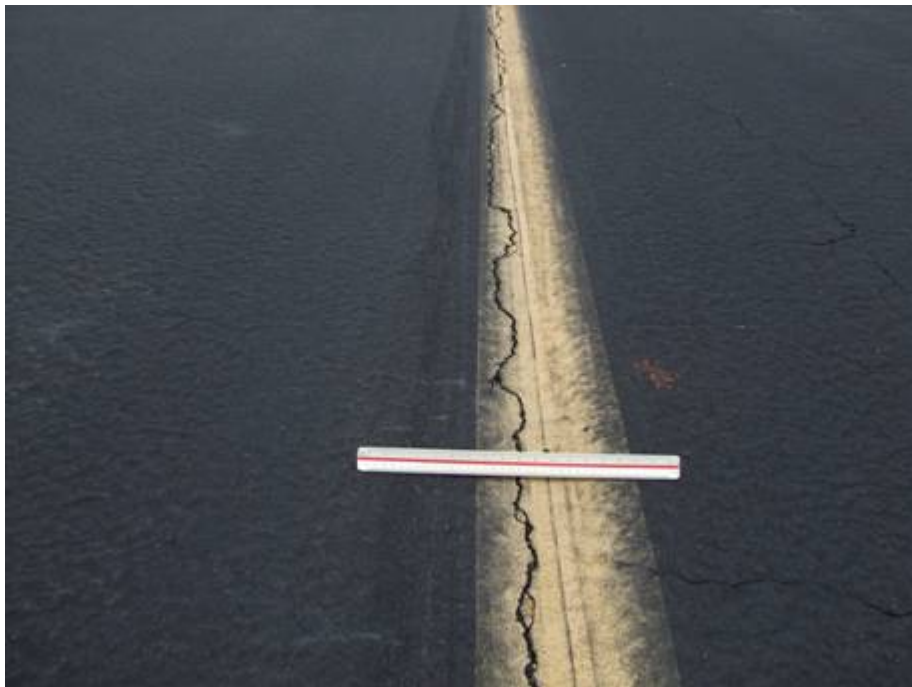
TW D Section 405 SU 103: Low Severity L/T Cracking (July 25, 2007)
