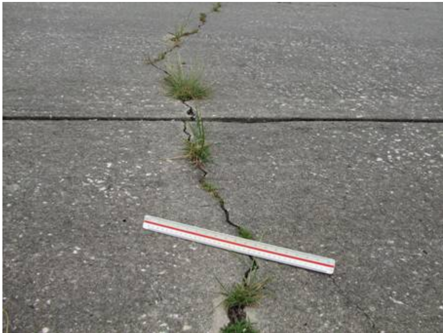
TW B Section 230 SU 135: Medium Severity Linear Cracking (July 25, 2007)
