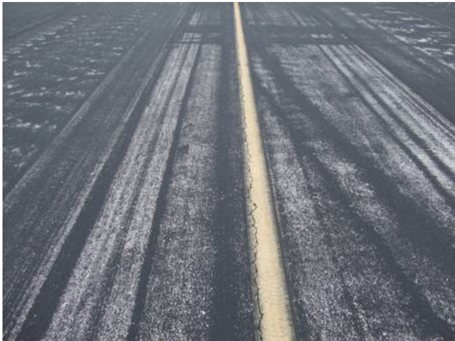
TW A Section 110 SU 137: Low Severity Weathering (July 25, 2007)
