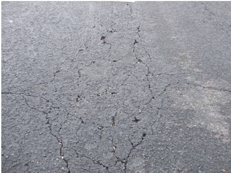
RW 4-22 Section 6105 SU 120: Low to Medium Severity Alligator Cracking (July 25, 2007)
