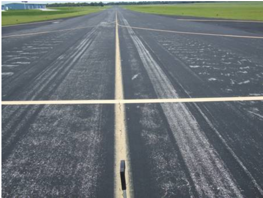
TW A Section 107 SU 135: Low Severity Weathering (July 25, 2007)
