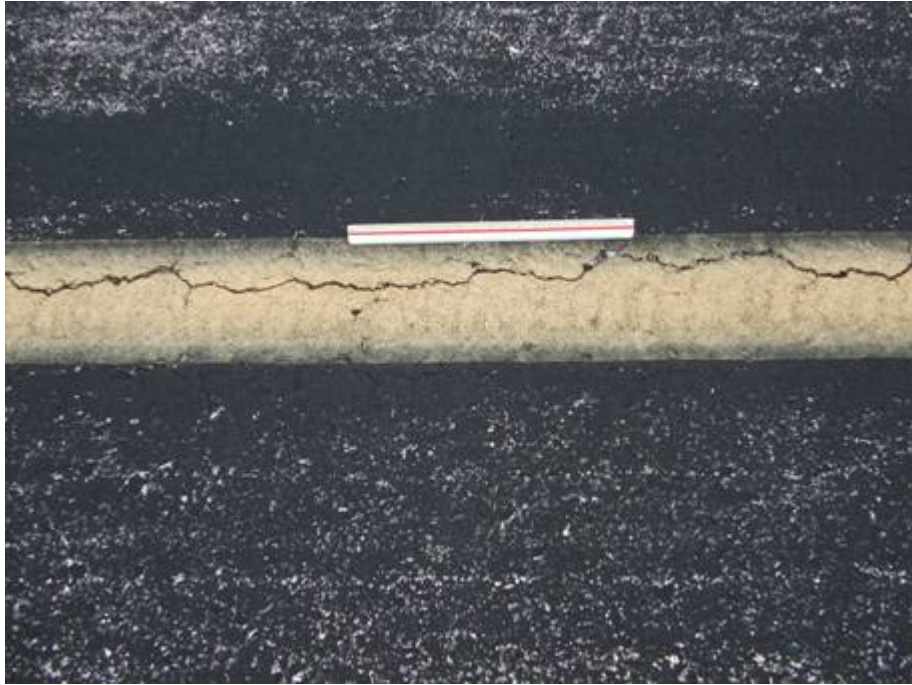
TW A Section 107 SU 135: Low Severity L/T Cracking (July 25, 2007)
