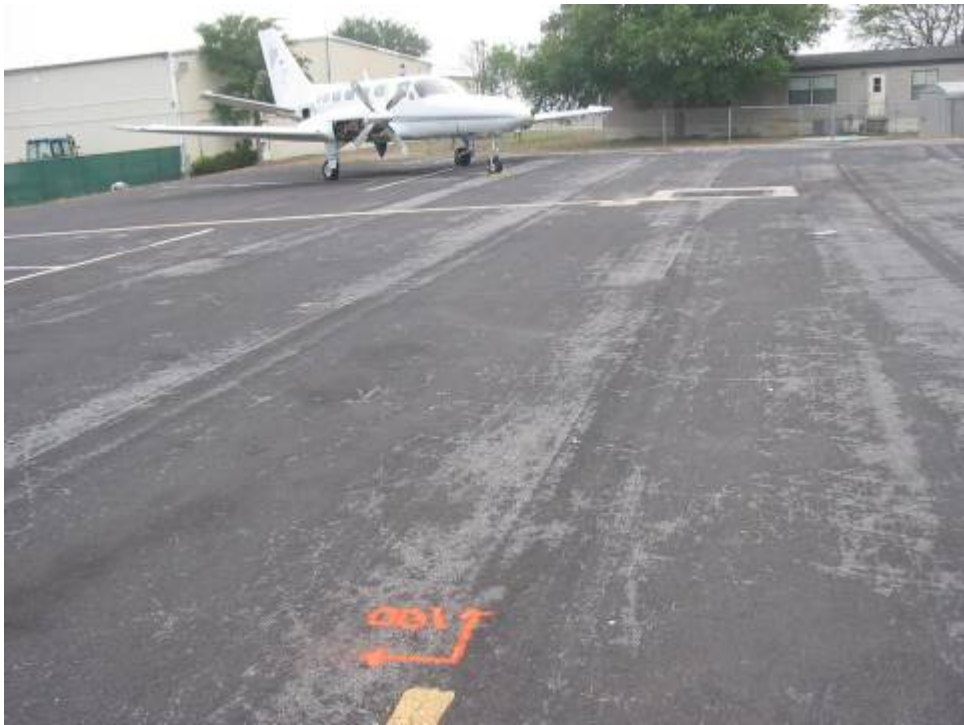
AP N Section 4310 SU 100: Medium Severity Weathering (May 14, 2007)
