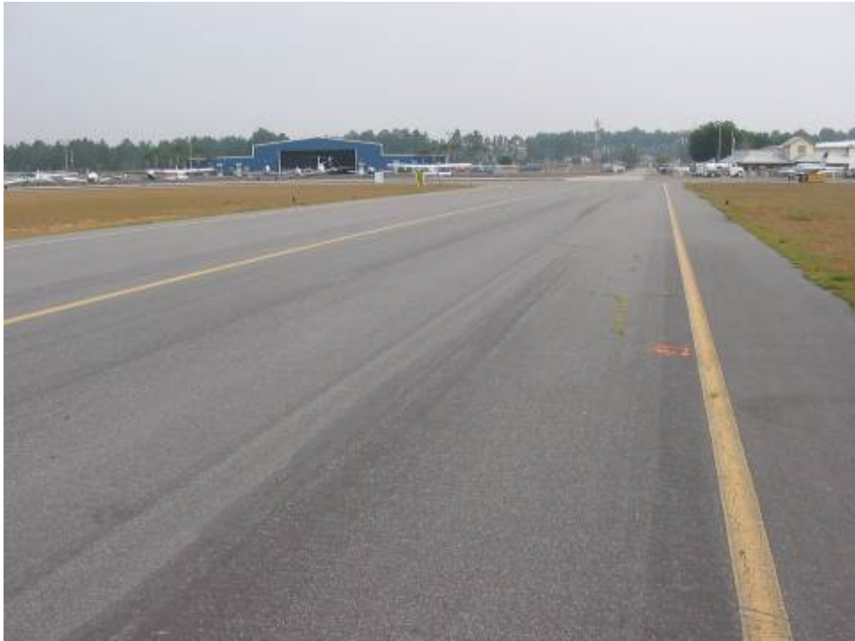
TW HS CONN Section 305 SU 101: Low Severity L/T Cracking (May 14, 2007)
