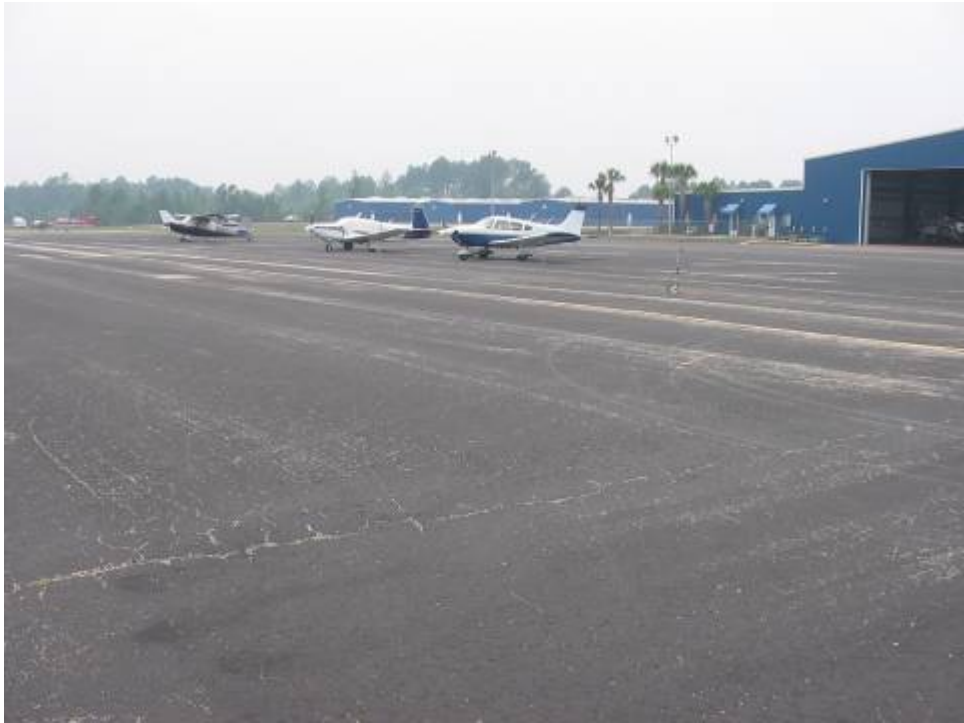
AP NW Section 4110 SU 353: Medium Severity Weathering (May 14, 2007)
