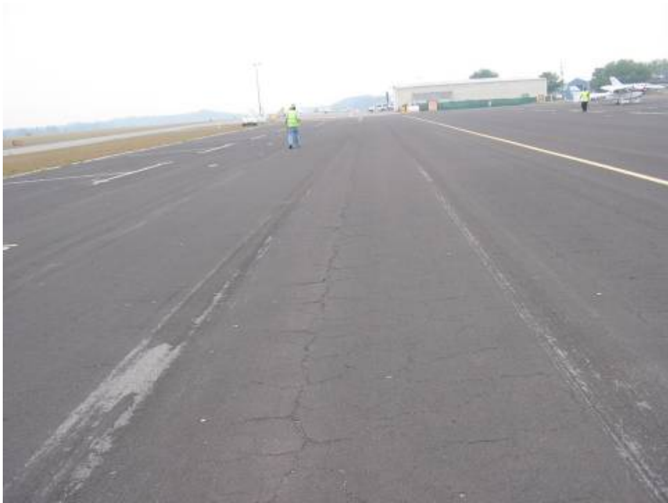
AP N Section 4305 SU 502: Medium Severity L/T Cracking (May 14, 2007)
