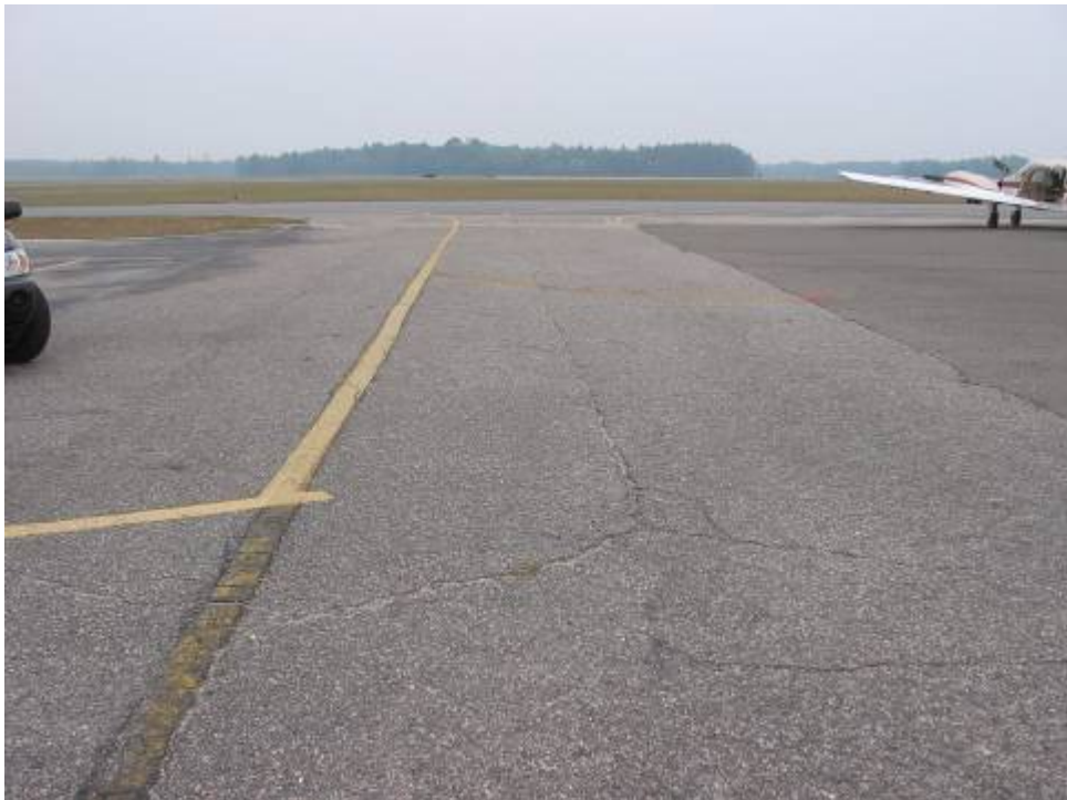
TW E FBO Section 710 SU 101: Medium Severity L/T Cracking
