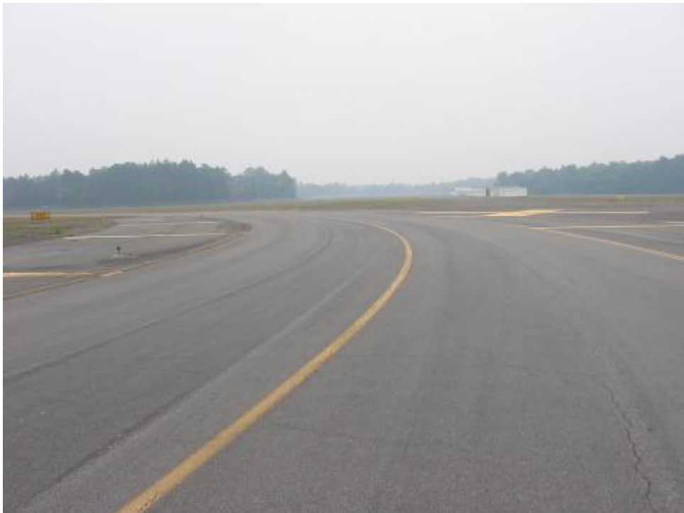
TW B Section 205 SU 102: Low Severity L/T Cracking (May 14, 2007)
