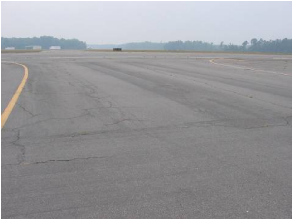
TW CONN RW Section 610 SU 100: Low Severity Block Cracking (May 14, 2007)
