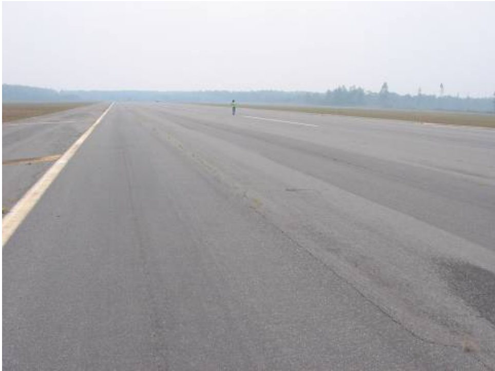
RW 11-29 Section 6205 SU 103: Low Severity L/T Cracking (May 14, 2007)
