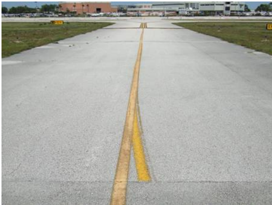
TW E-3 Section 540 SU 302: Low Severity L/T Cracking (June 5, 2007)
