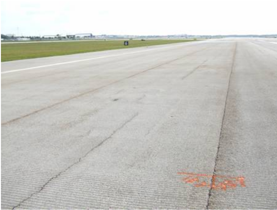
RW 7L-25R Section 6129 SU 558: Low/Medium Severity L/T Cracking (June 5, 2007)
