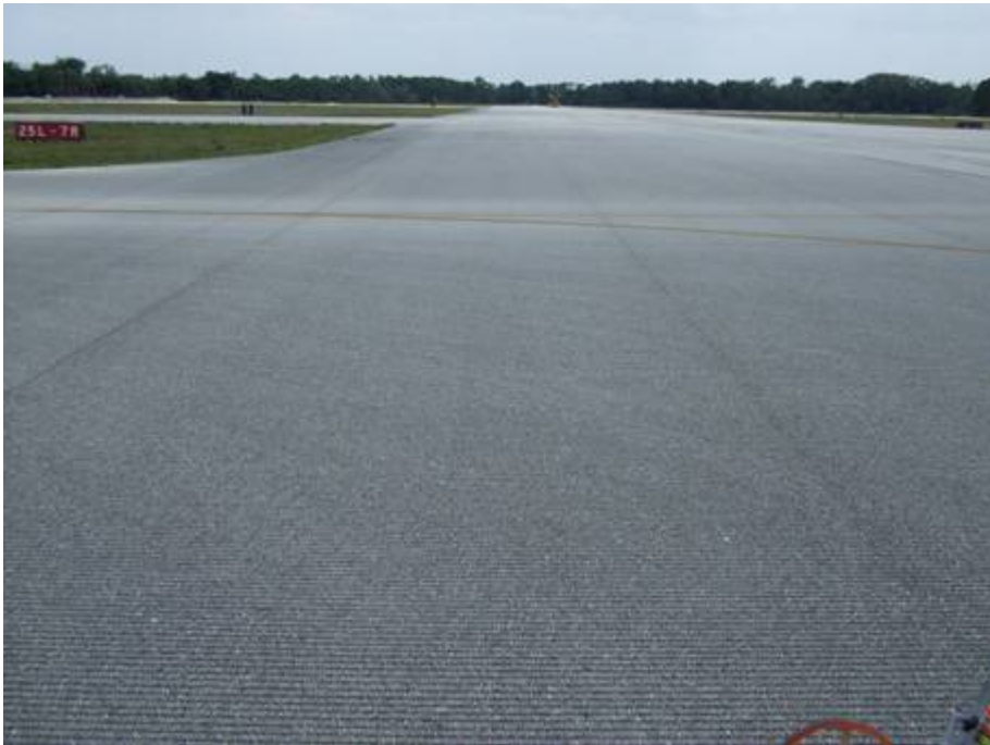
RW 16-34 Section 6210 SU 116: Low Severity L/T Cracking (June 5, 2007)
