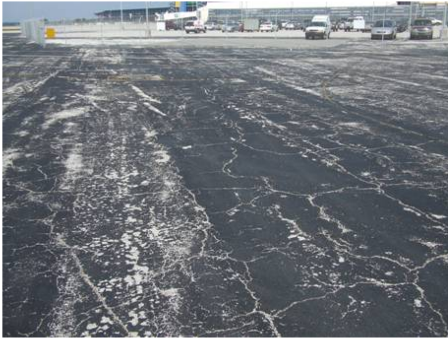
AP Section 4255 SU 403: High Severity Weathering (June 5, 2007)
