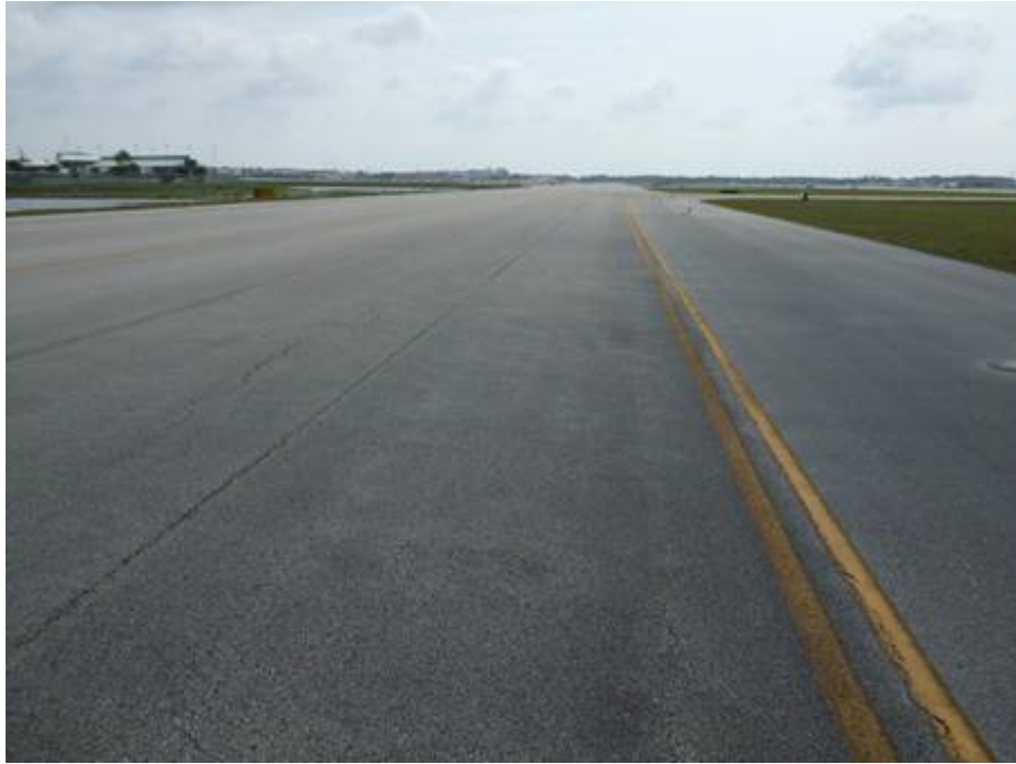
TW N Section 1408 SU 159: Medium Severity L/T Cracking (June 5, 2007)
