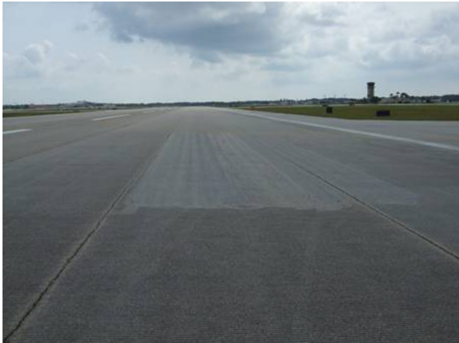
RW 7L-25R Section 6138 SU 170: Medium Severity L/T Cracking (June 5, 2007)
