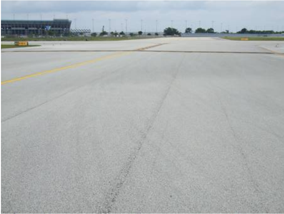
TW N-5 Section 1450 SU 502: Low Severity L/T Cracking (June 5, 2007)
