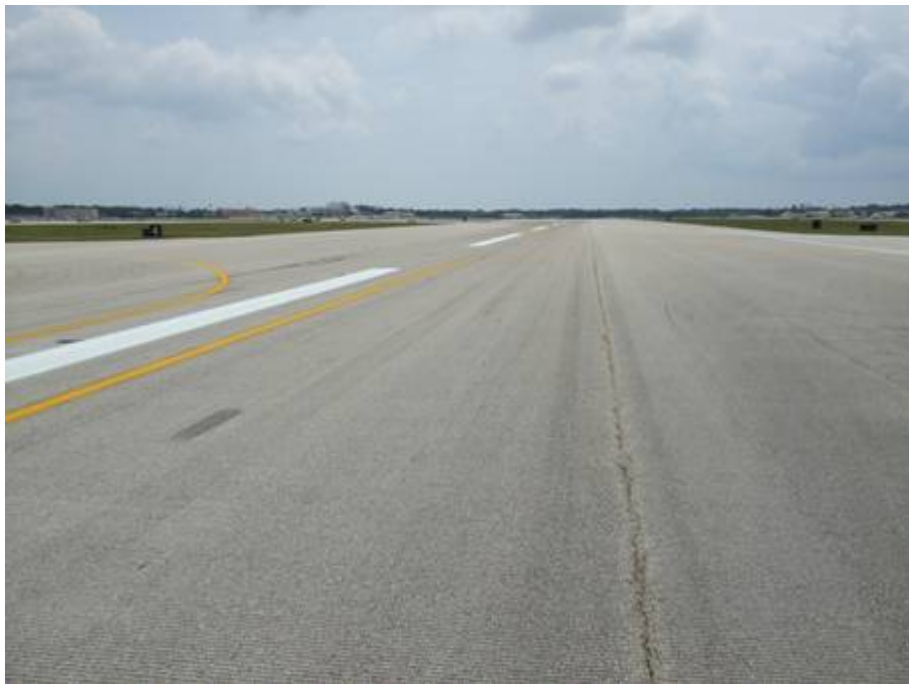
RW 7L-25R Section 6150 SU 382: Medium Severity L/T Cracking (June 5, 2007)
