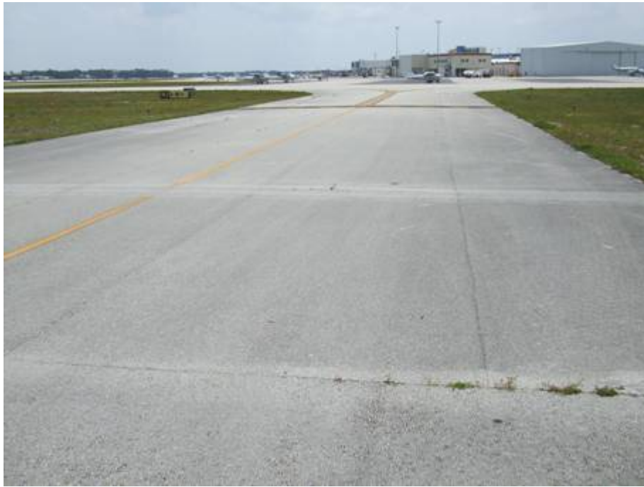
TW W-3 Section 2350 SU 302: Low to Medium Severity L/T Cracking (June 5, 2007)
