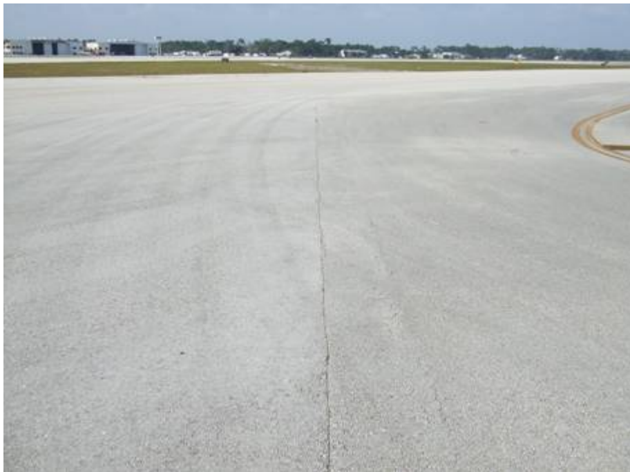
TW A Section 115 SU 201: Low Severity L/T Cracking (June 5, 2007)
