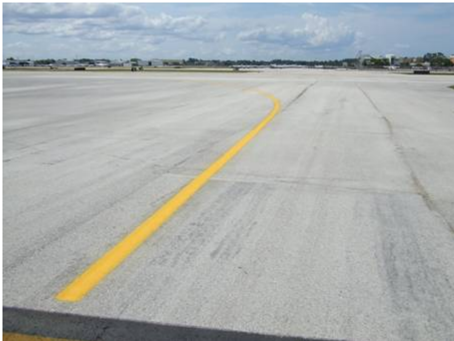
TW P Section 840 SU 210: Low Severity L/T Cracking (June 5, 2007)
