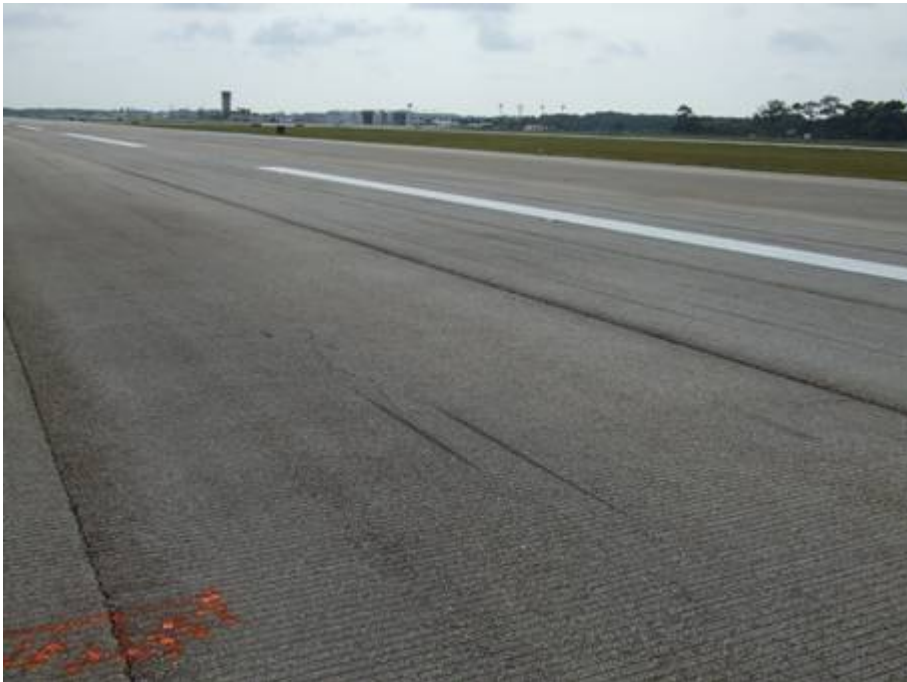
RW 7L-25R Section 6127 SU 357: Medium Severity L/T Cracking (June 5, 2007)
