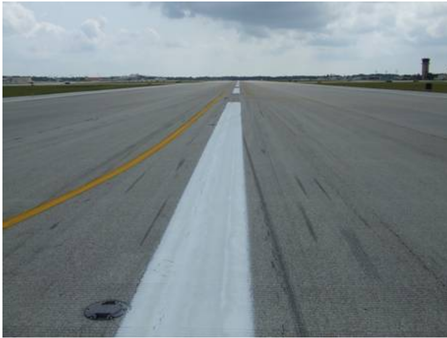
RW 7L-25R Section 6145 SU 371: Low Severity L/T Cracking (June 5, 2007)
