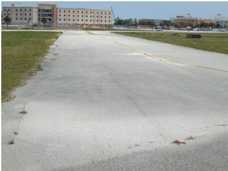
TW E-4 Section 550 SU 402: Low Severity L/T Cracking (June 5, 2007)
