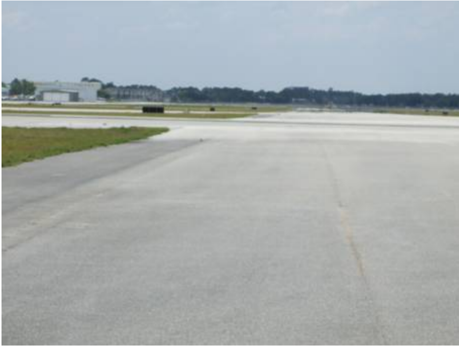
RW 16-34 Section 6230 SU 352: Low Severity L/T Cracking (June 5, 2007)
