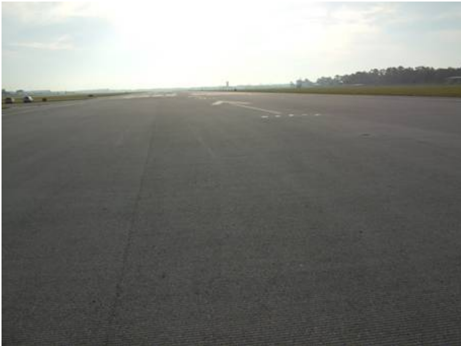
RW 7L-25R Section 6102 SU 292: Low Severity L/T Cracking (June 5, 2007)
