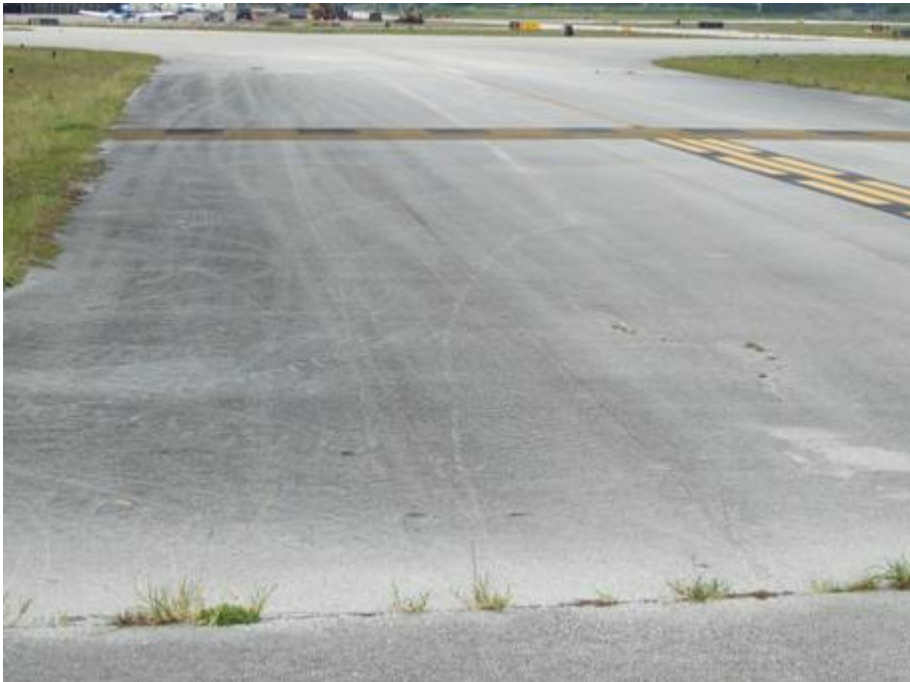
TW W Section 2335 SU 202: Medium Severity L/T Cracking (June 5, 2007)
