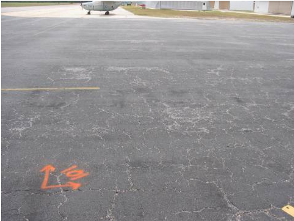
AP N Section 4205 SU 101: Medium Severity Weathering (May 7, 2007)
