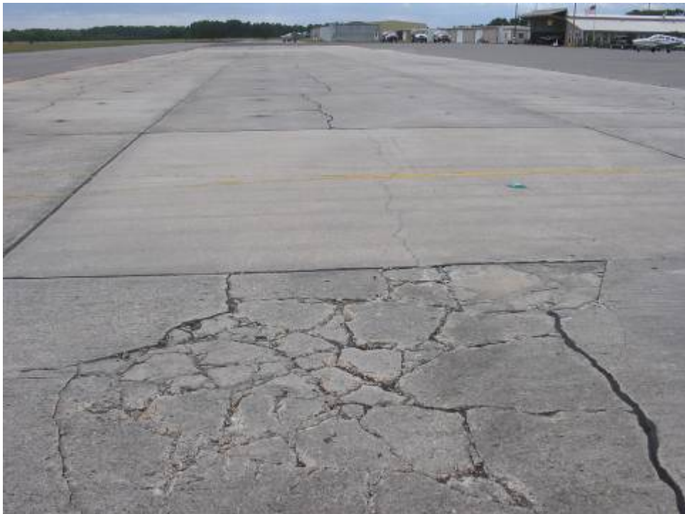
AP N Section 4210 SU 219: High Severity Shattered Slab (May 7, 2007)
