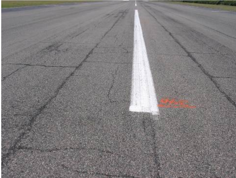
RW 13-31 Section 6215 SU 340: Medium Severity Block Cracking (May 7, 2007)
