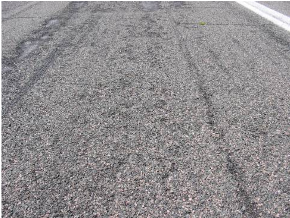
RW 13-31 Section 6215 SU 315: High Severity Weathering (May 7, 2007)
