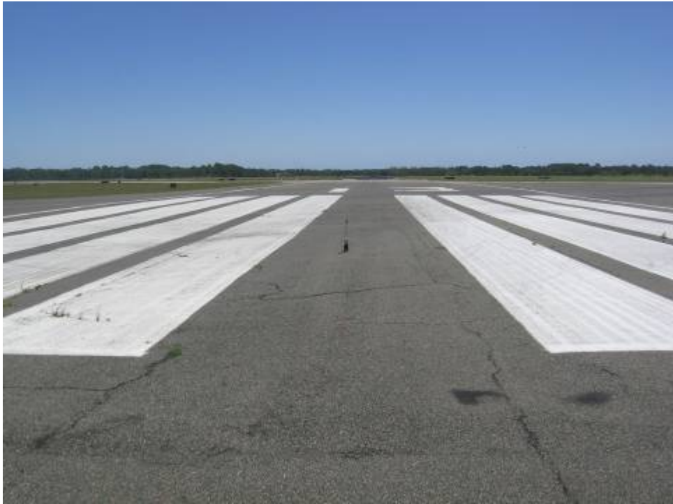
RW 13-31 Section 6215 SU 305: Low Severity L/T Cracking (May 7, 2007)
