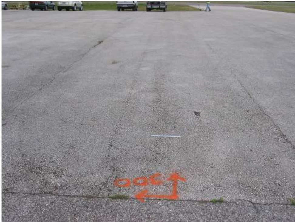
AP NW Section 4110 SU 300: Low Severity L/T Cracking (May 7, 2007)
