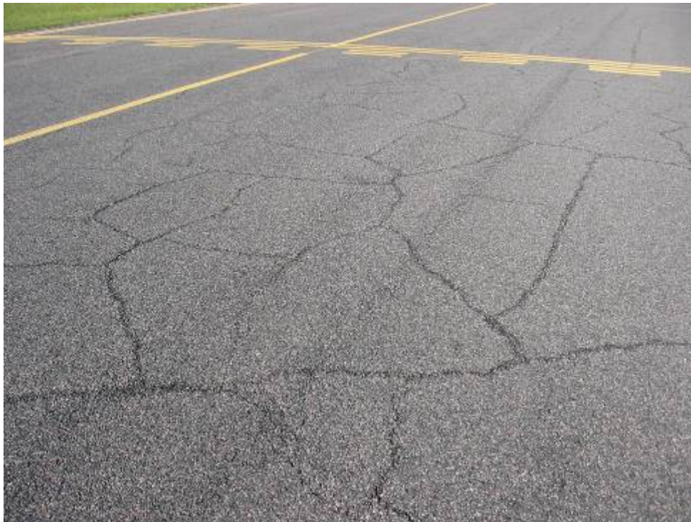
TW A Section 310 SU 101: Medium Severity Block Cracking (May 7, 2007)
