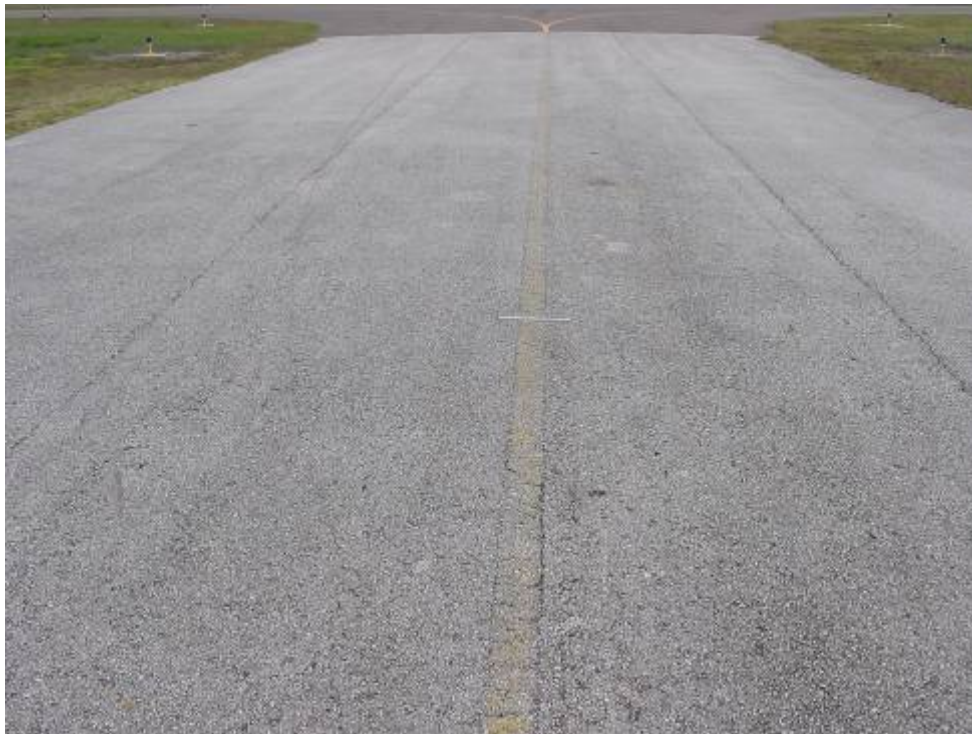
TW W AP Section 505 SU 100: Low Severity L/T Cracking (May 7, 2007)
