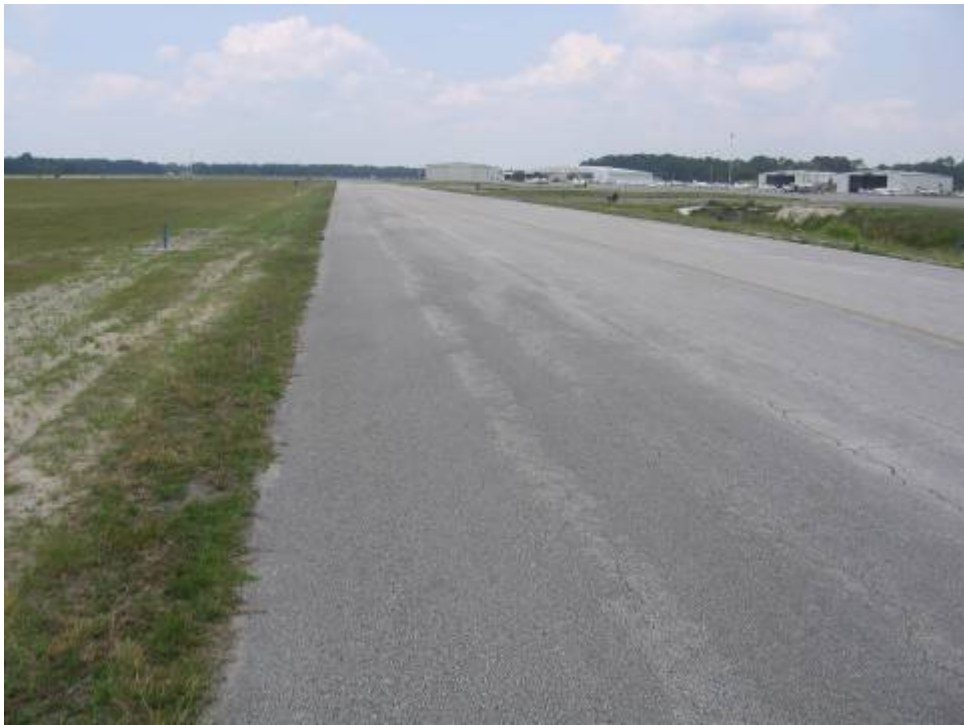
TW A Section 120 SU 107: Low Severity L/T Cracking (May 23, 2007)
