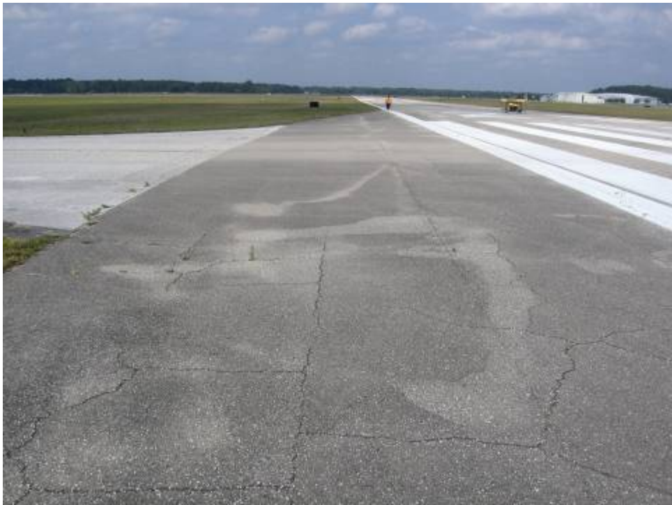
TW B Section 202 SU 778: Low Severity Block Cracking (May 23, 2007)
