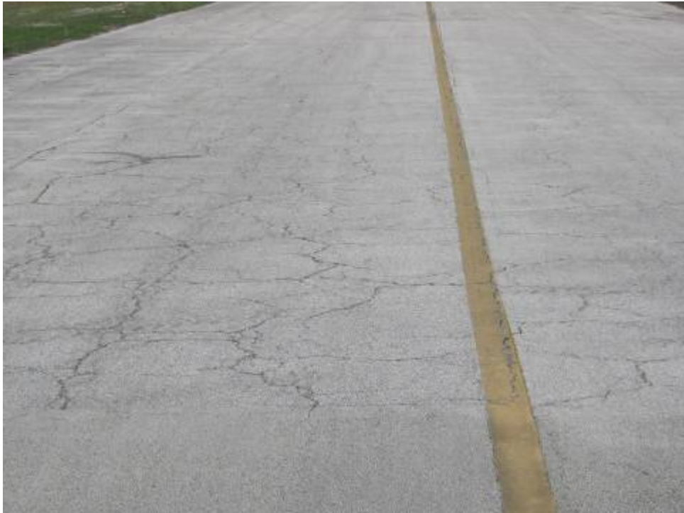
TW A Section 125 SU 102: Medium Severity Block Cracking (May 23, 2007)
