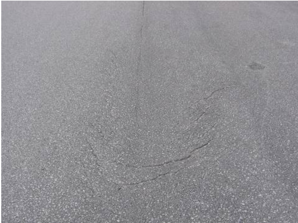
TW A Section 110 SU 102: Slippage Cracking (May 23, 2007)
