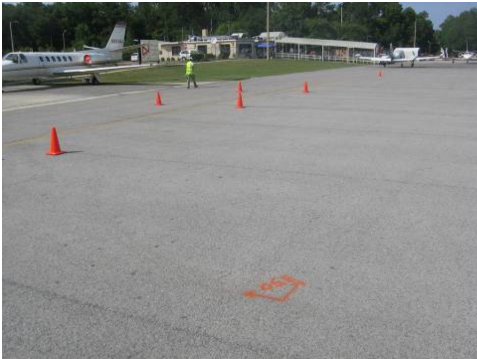
TW D Section 405 SU 350: Low Severity L/T Cracking (May 23, 2007)
