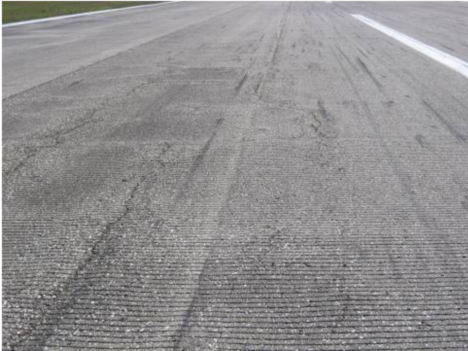
RW 7-25 Section 6107 SU 570: Medium Severity L/T Cracking (May 23, 2007)
