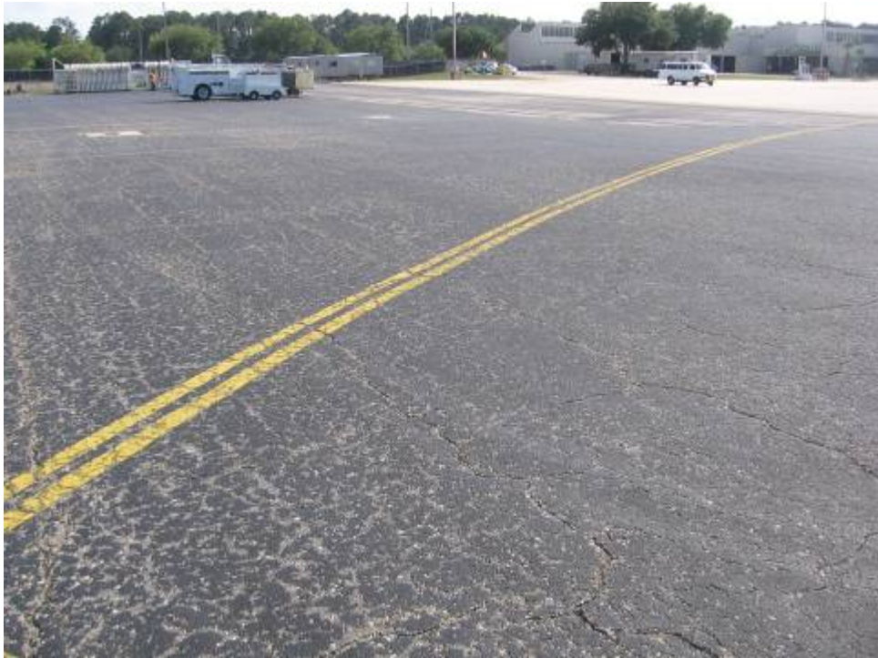
AP S Section 4120 SU 107: Medium Severity Block Cracking (May 23, 2007)
