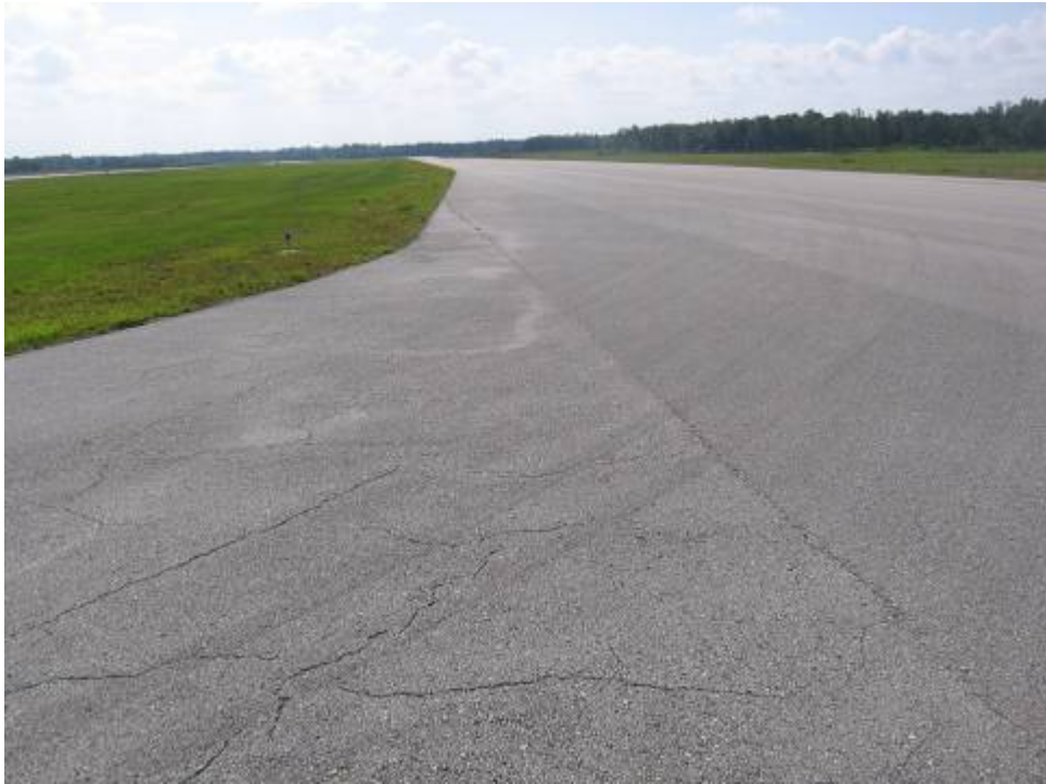
TW E Section 535 SU 309: Low Severity Block Cracking (May 23, 2007)
