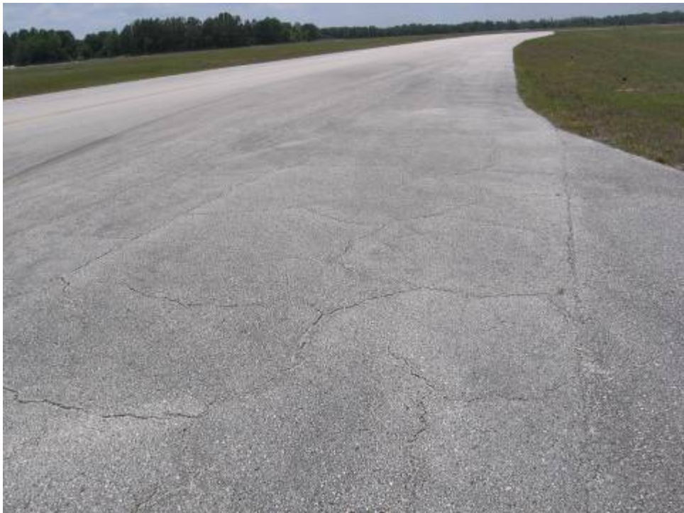
TW E Section 545 SU 408: Low Severity Block Cracking (May 23, 2007)
