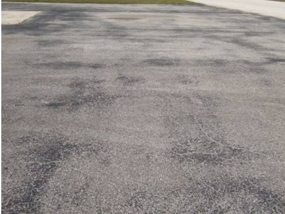
AP S Section 4205 SU 100: High Severity Weathering (June 13, 2007)
