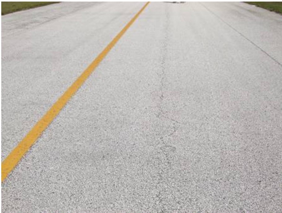
TW J Section 1005 SU 303: Low Severity L/T Cracking (June 13, 2007)
