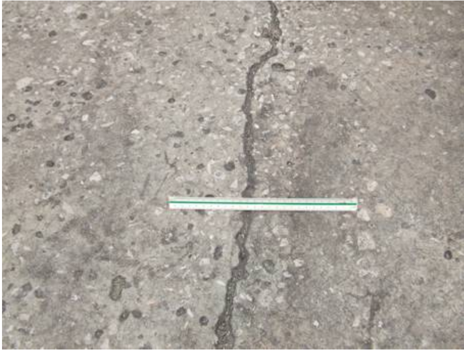
AP HANG Section 4305 SU 102: Low Severity Linear Cracking (June 13, 2007)
