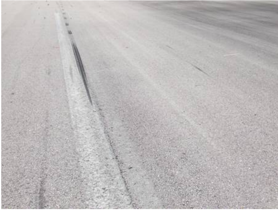
RW 3-21 Section 6115 SU 184: Low Severity L/T Cracking (June 13, 2007)
