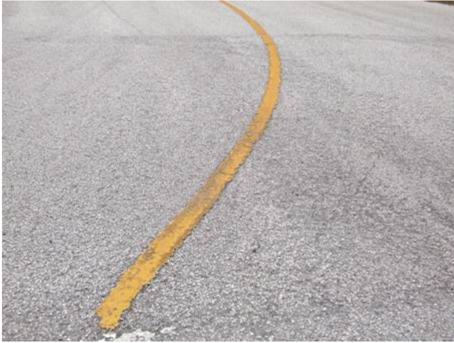
TW J Section 1002 SU 100: Medium Severity Weathering (June 13, 2007)
