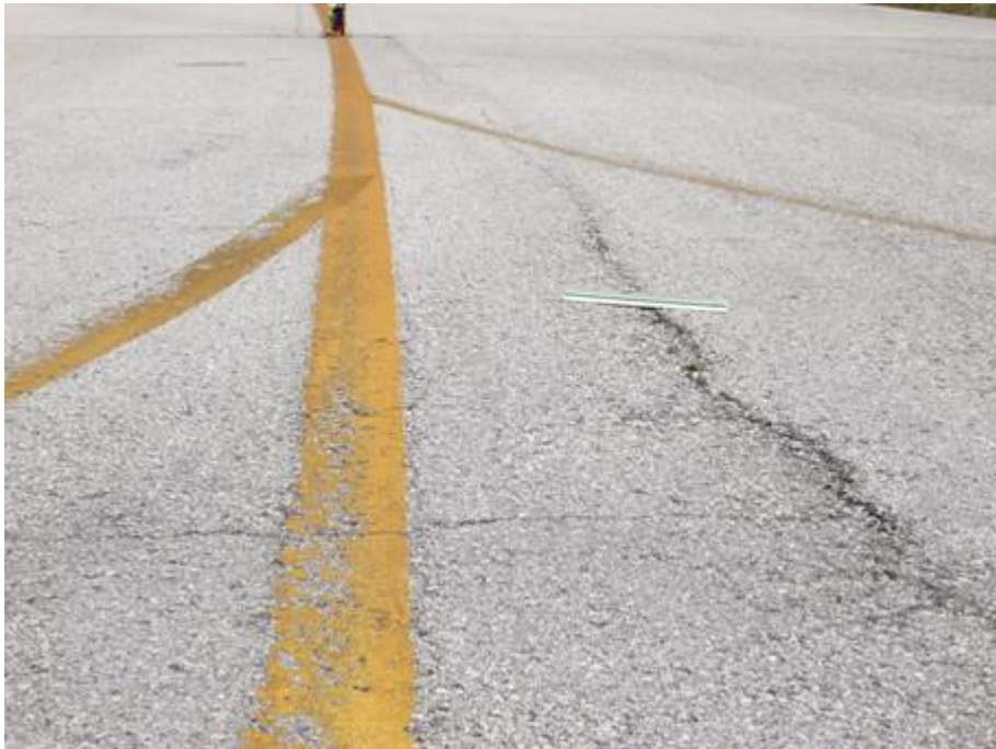
TW A Section 107 SU 112: Medium Severity L/T Cracking (June 13, 2007)
