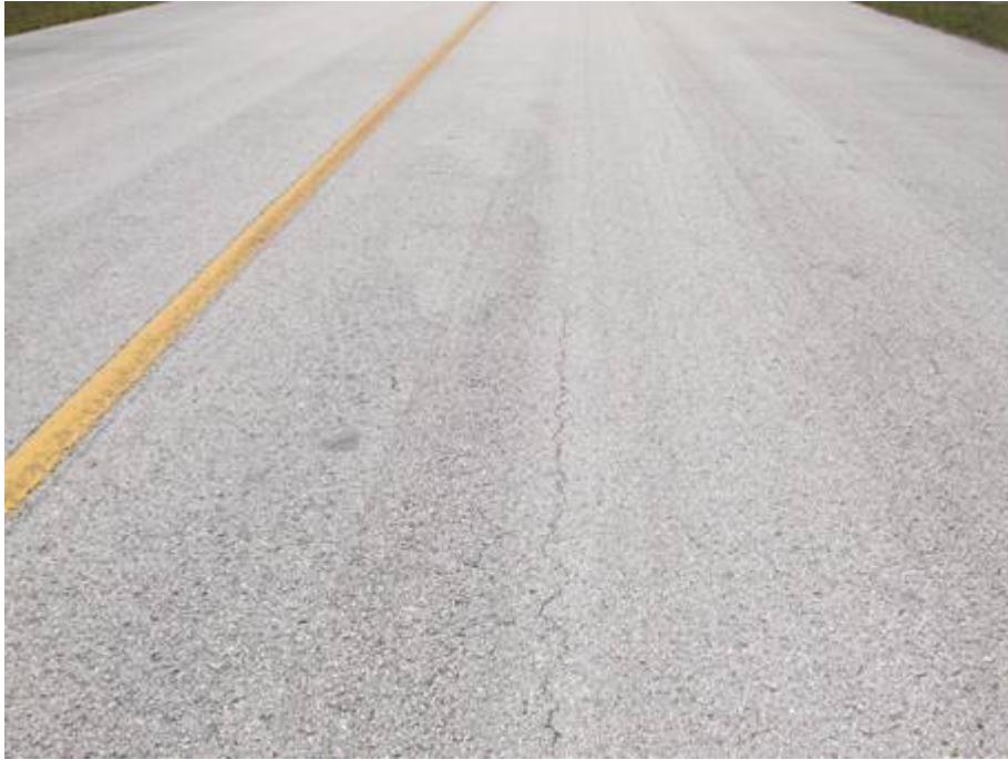
TW A Section 105 SU 109: Low Severity L/T Cracking (June 13, 2007)
