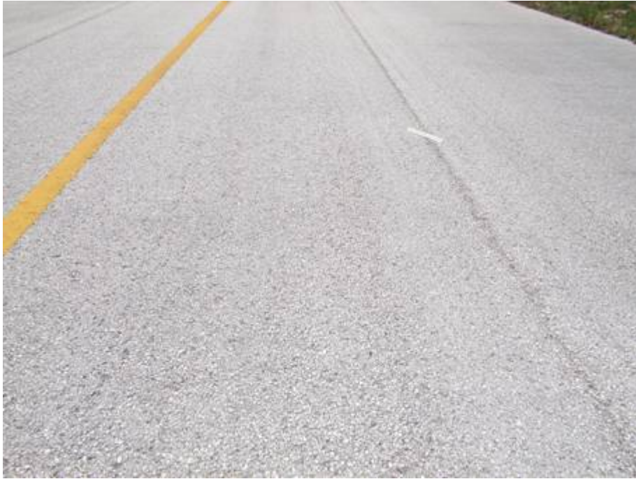
TW K Section 1105 SU 103: Low Severity L/T Cracking (June 13, 2007)
