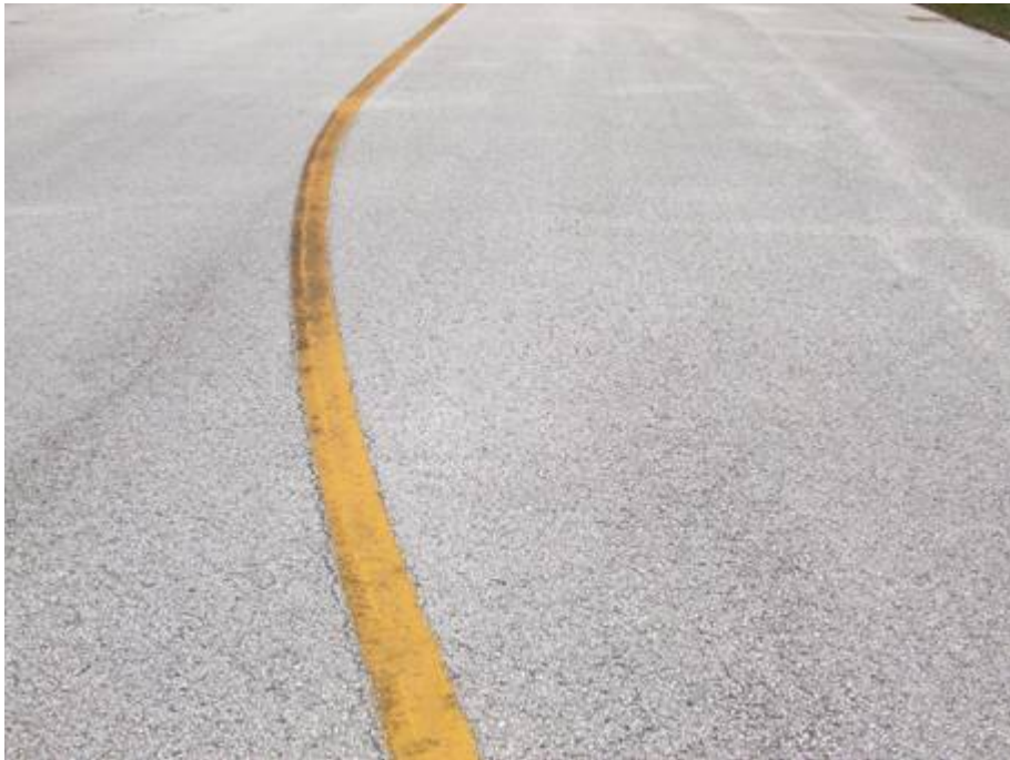
TW K Section 1110 SU 100: Low Severity Weathering (June 13, 2007)
