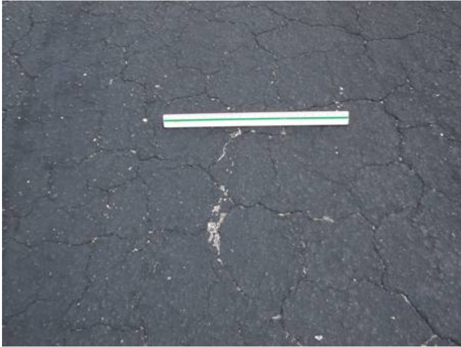
AP HANG Section 4325 SU 200: Low Severity Weathering (June 13, 2007)
