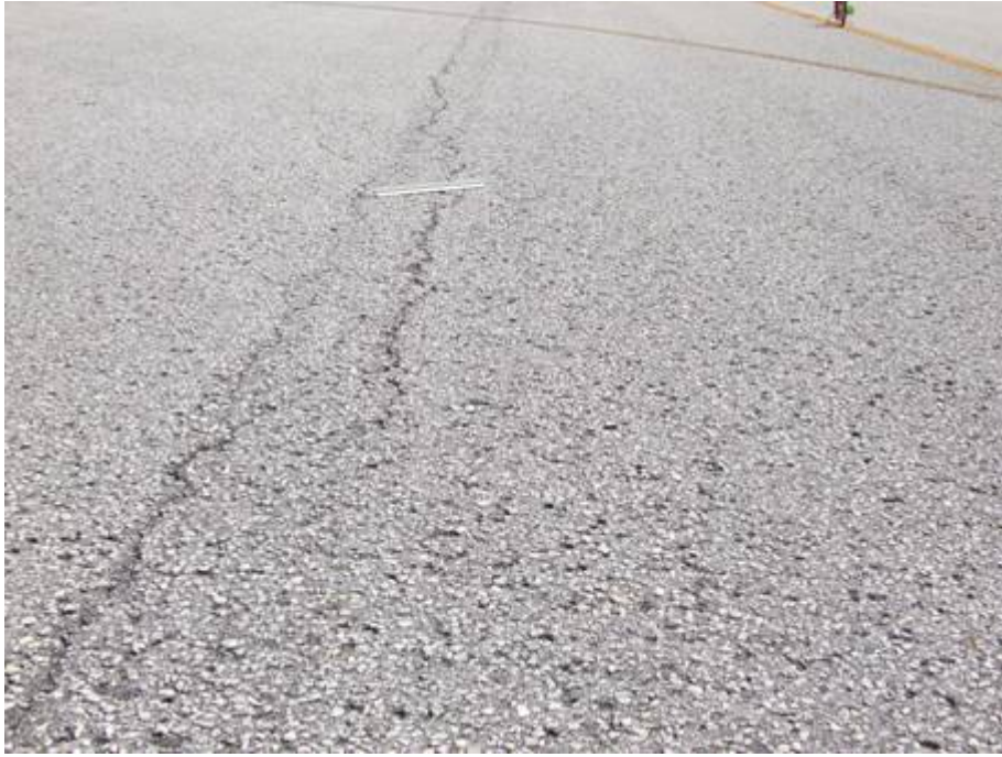
TW B Section 205 SU 199: Medium Severity L/T Cracking and Weathering (June 13, 2007)
