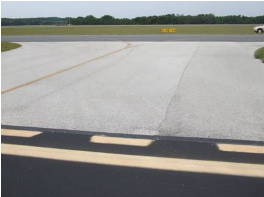
TW D Section 506 SU 602: Low Severity L/T Cracking (June 13, 2007)
