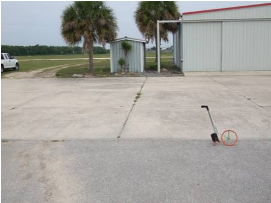
AP HANG Section 4305 SU 102: High Severity Joint Seal Damage (June 13, 2007)
