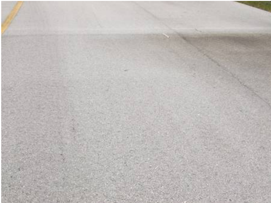
TW B Section 210 SU 105: Low Severity L/T Cracking (June 13, 2007)
