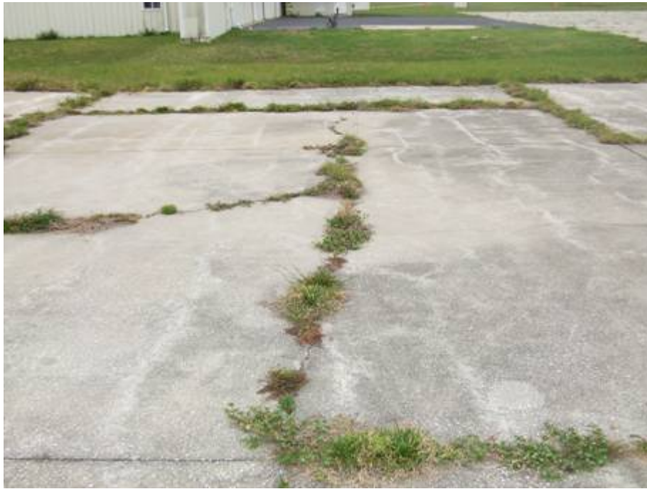
AP Section 4105: High Severity Jt Seal Damage, Medium Severity Cracking (June 11, 2007)
