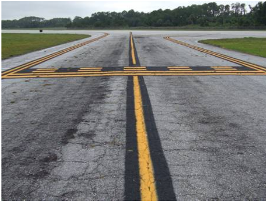
TW A Section 120 SU 101, Medium Severity Block Cracking (June 11, 2007)
