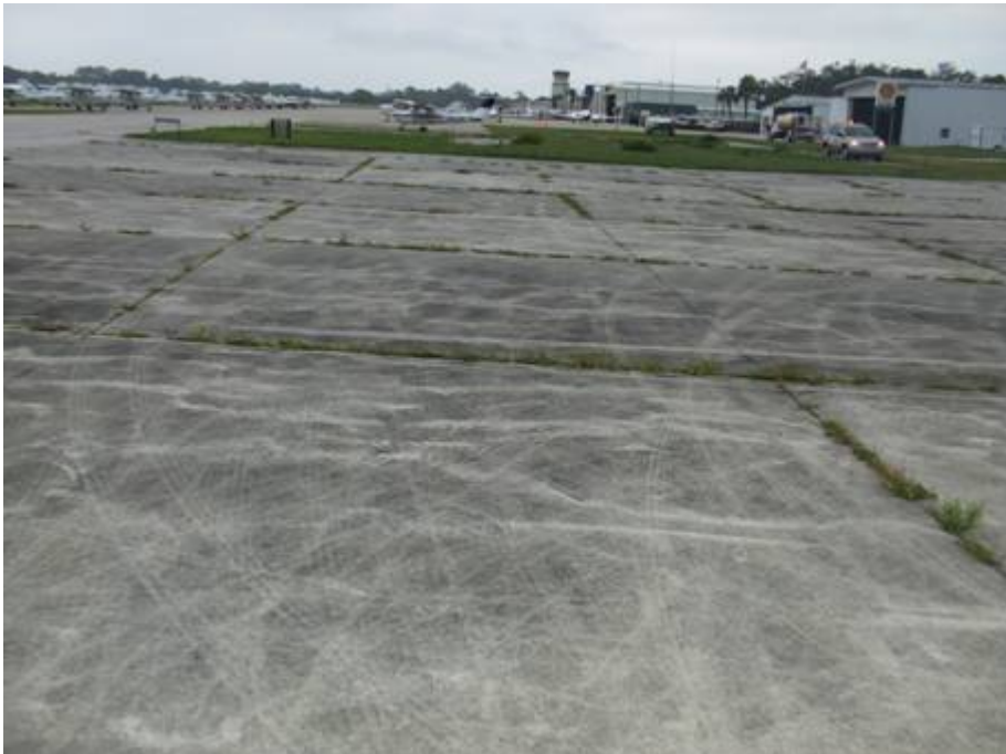
AP Section 4102: High Severity Joint Seal Damage (June 11, 2007)
