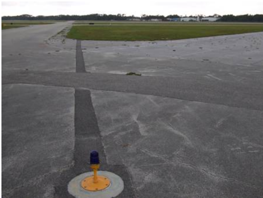
RW 15-33 Section 6330 SU 100, Low Severity Patching, Block Cracking (June 11, 2007)
