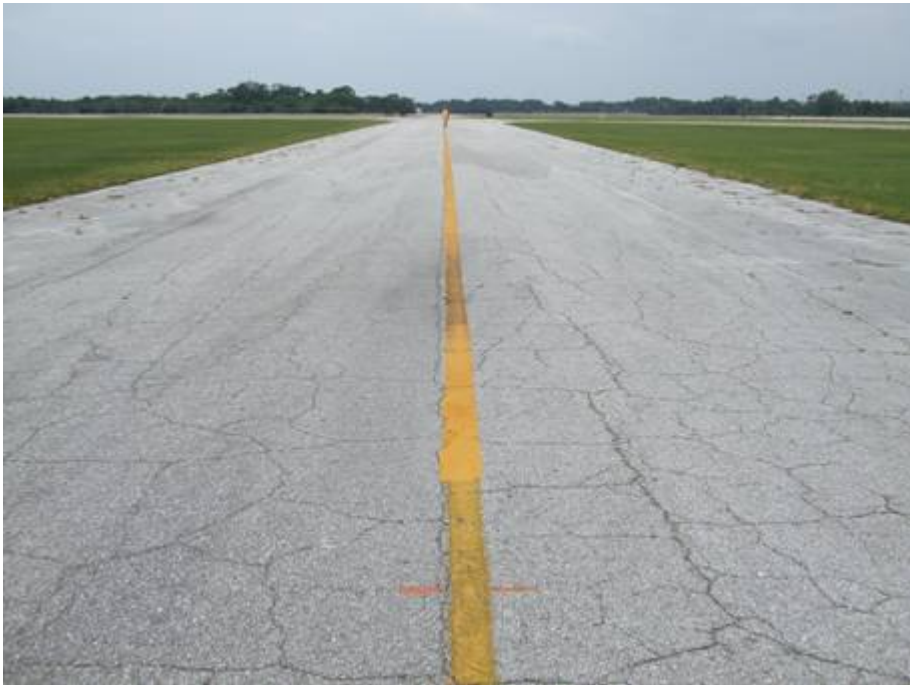
TW D Section 410 SU 305, Medium Severity Block Cracking (June 11, 2007)
