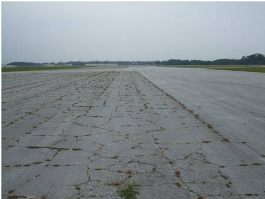
RW 15-33 Section 6305 SU 160, Medium Severity Block Cracking (June 11, 2007)
