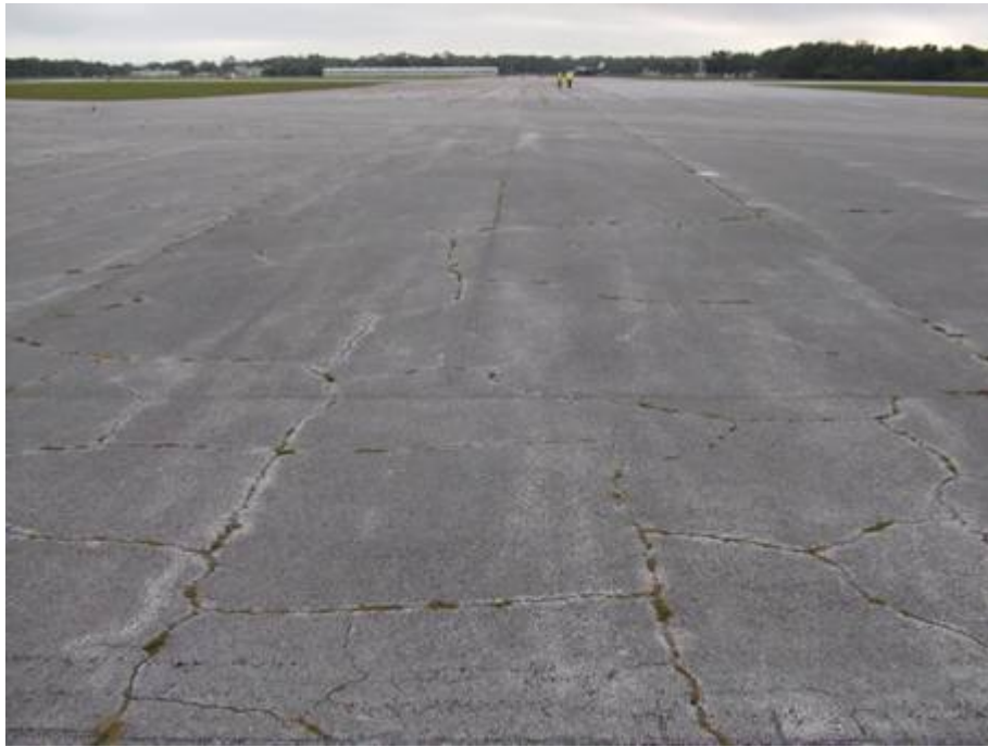
RW 15-33 Section 6320 SU 143, Medium Severity Block Cracking (June 11, 2007)
