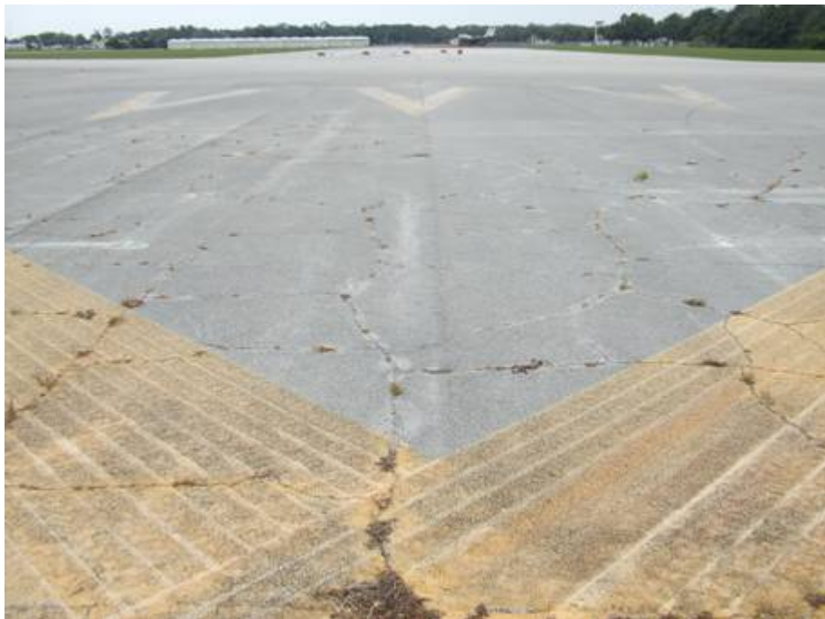
RW 15-33 Section 6310 SU 130, Medium Severity Block Cracking (June 11, 2007)
