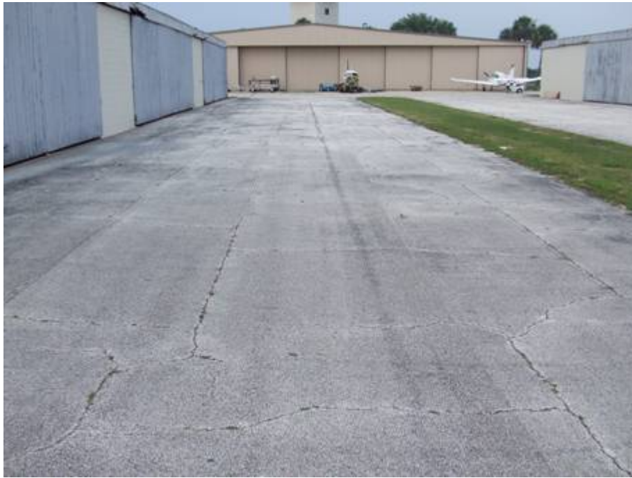
AP Section 4140: Medium Severity Block Cracking (June 11, 2007)
