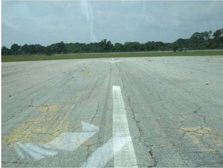
RW 2-20 Section 6405: Medium Severity Block Cracking (June 11, 2007)
