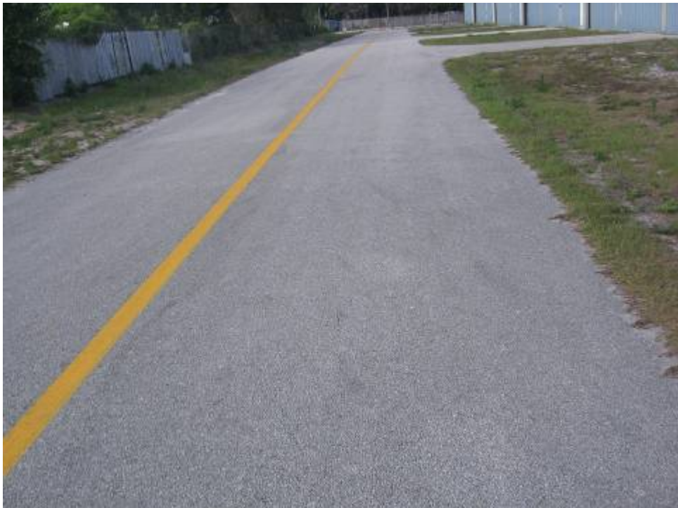
AP T-HANG Section 4310: Low Severity Weathering (May 24, 2007)
