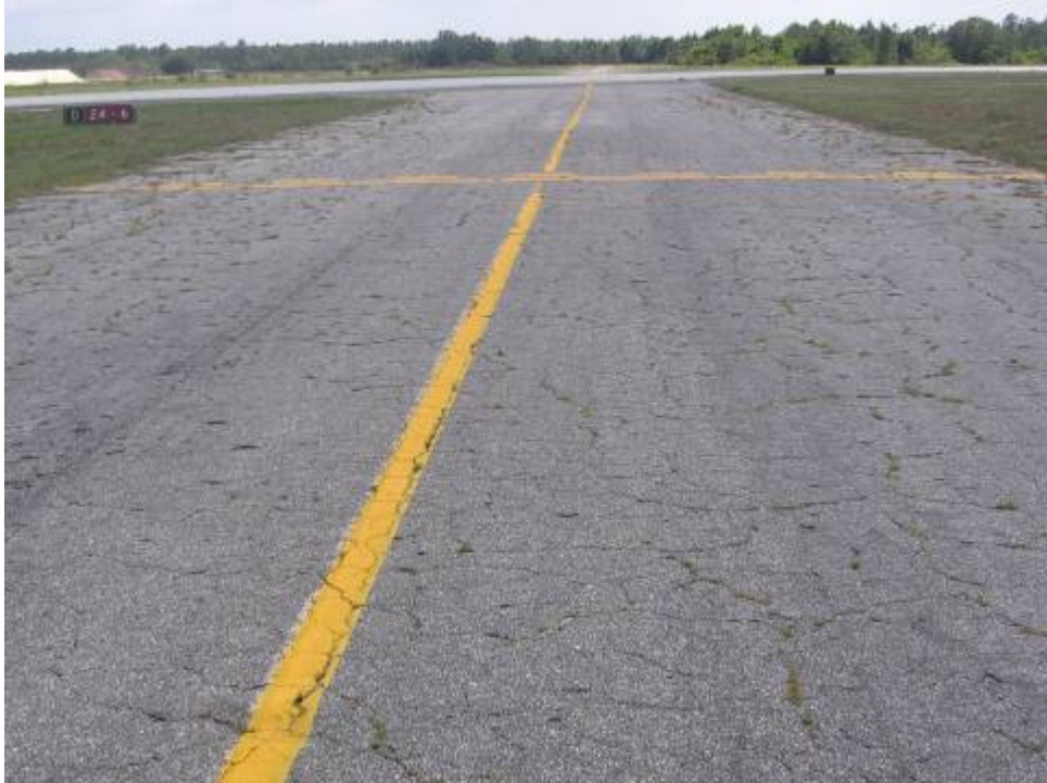
TW D Section 405: Medium Severity Block Cracking (May 24, 2007)
