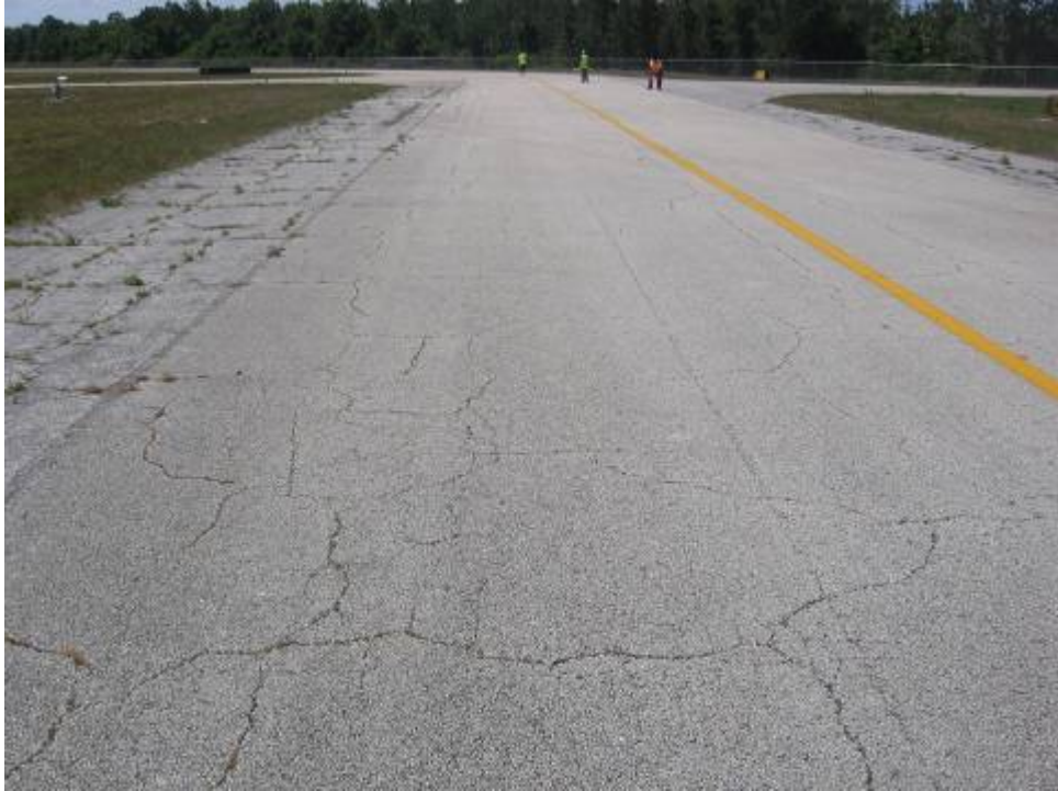
TW A Section 110: Medium Severity Block Cracking (May 24, 2007)
