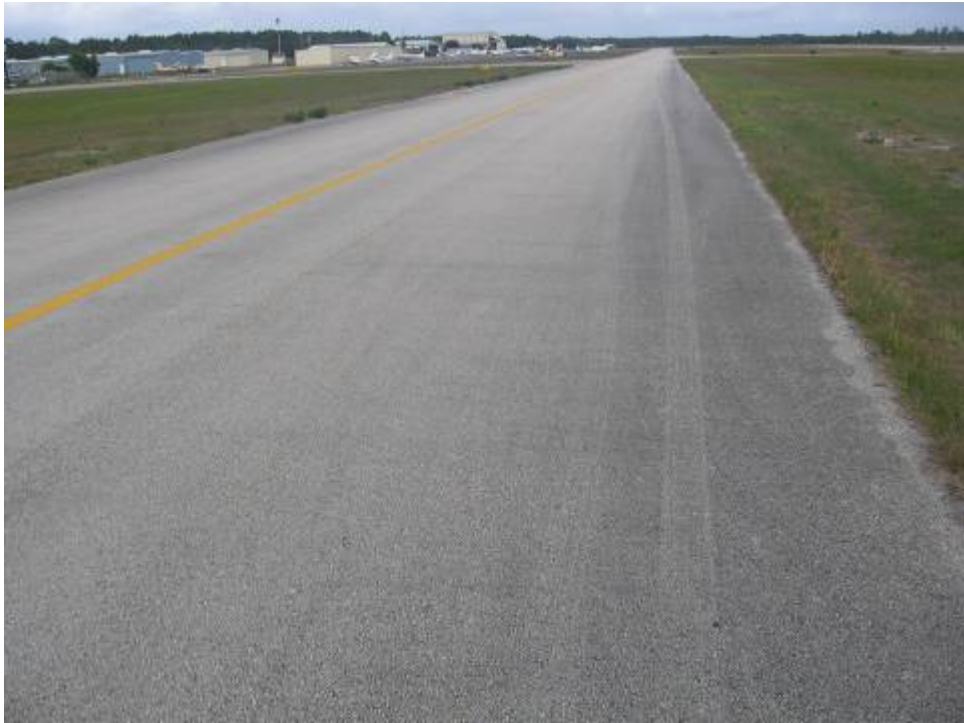
TW B Section 205: Low Severity Linear/Transverse Cracking (May 24, 2007)
