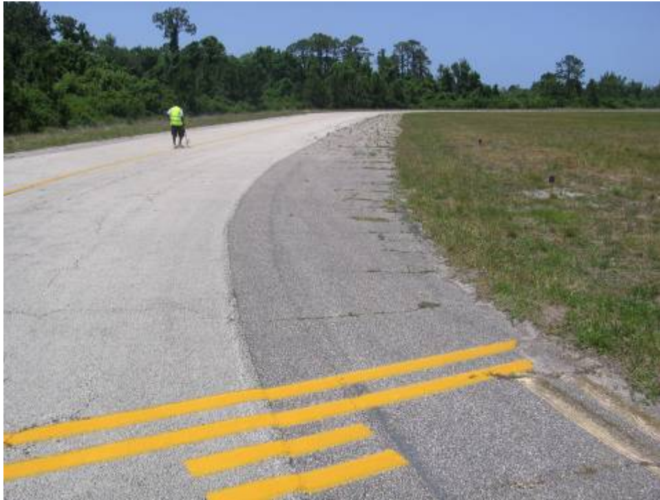
TW E Section 512: Low Severity Block Cracking (May 24, 2007)
