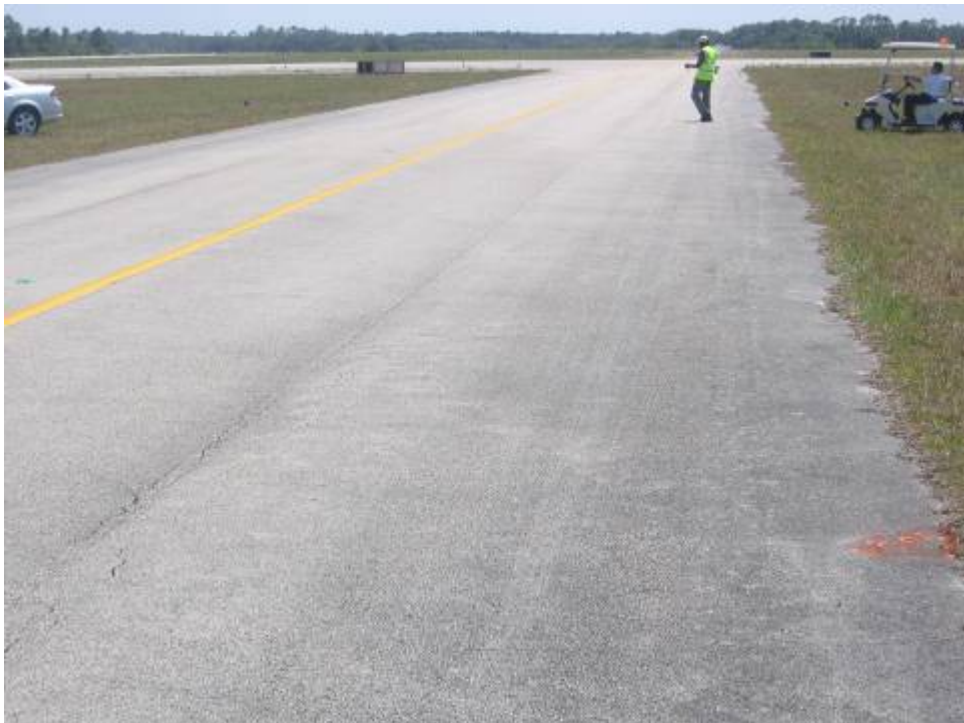
TW E Section 505: Low Severity Linear/Transverse Cracking (May 24, 2007)
