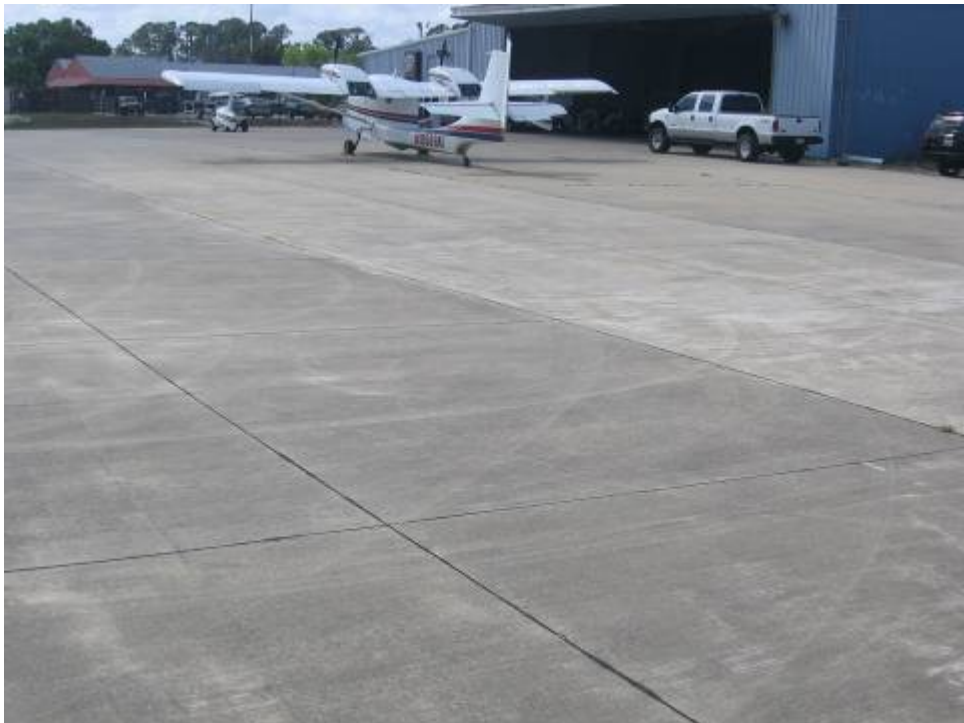
AP Section 4125: Low Severity Scaling (May 24, 2007)
