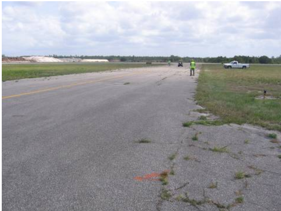
TW D Section 407: Low Severity Linear/Transverse Cracking (May 24, 2007)
