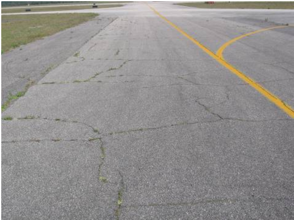
TW C Section 307: Low Severity Block Cracking (May 24, 2007)
