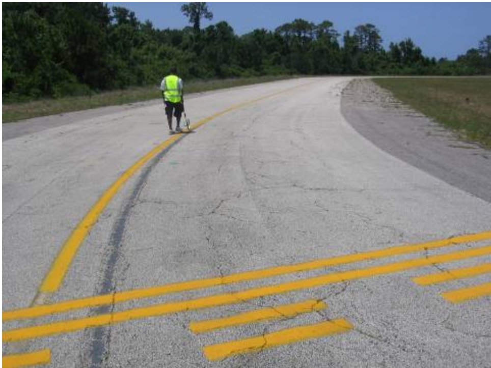
TW E Section 510: Low Severity Block Cracking (May 24, 2007)
