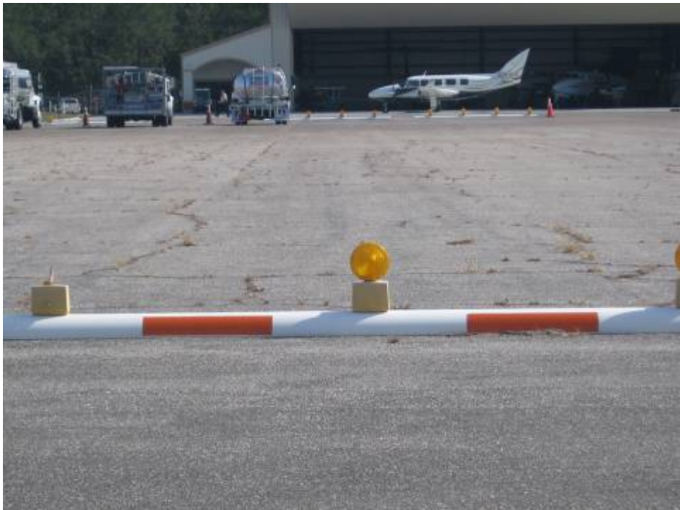
TW F Section 605: Medium Severity Block Cracking (May 24, 2007)
