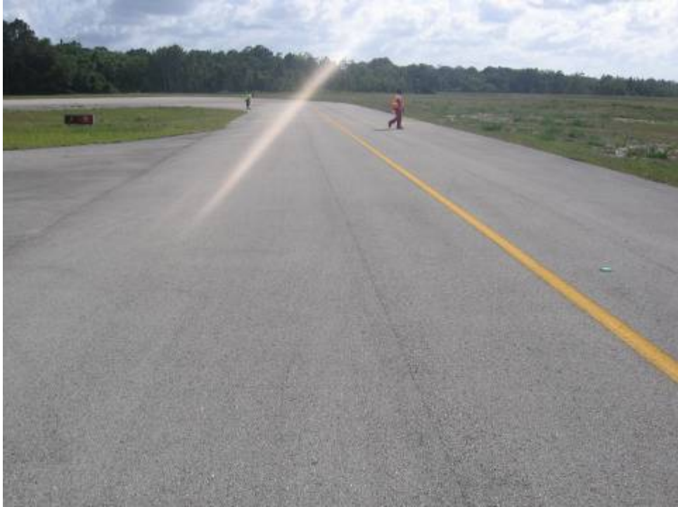
TW A Section 102: Low Severity Linear/Transverse Cracking (May 24, 2007)
