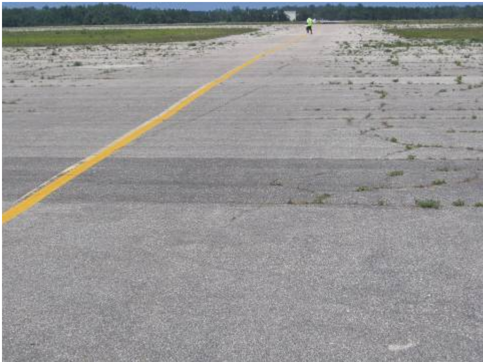
TW E Section 515: Medium Severity Linear/Transverse Cracking (May 24, 2007)
