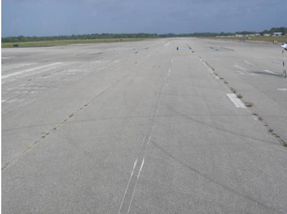
RW 11-29 Section 6105: Medium Severity Linear/Transverse Cracking (May 24, 2007)
