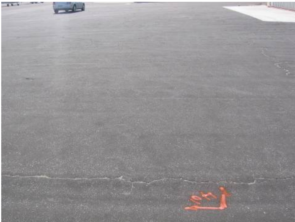
AP Section 4115: Medium Severity Block Cracking (May 24, 2007)
