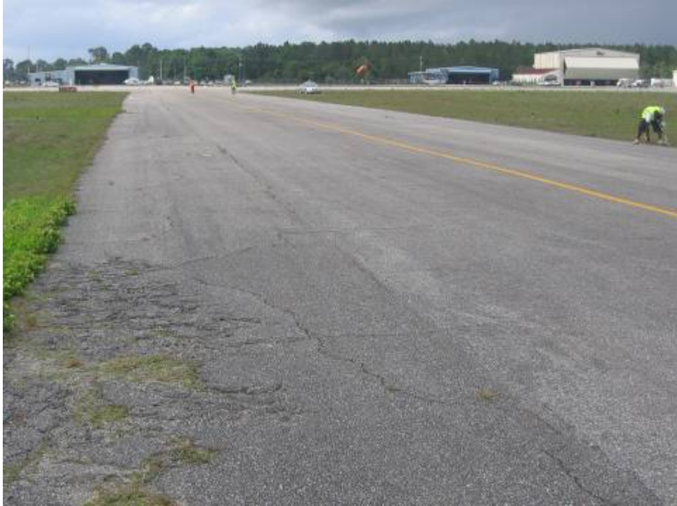
TW D Section 410: High Severity Weathering (May 24, 2007)
