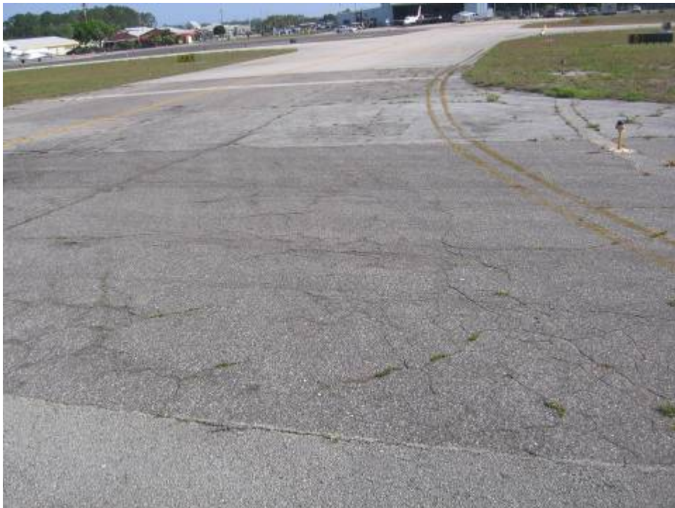
TW D Section 414: Medium Severity Block Cracking (May 24, 2007)
