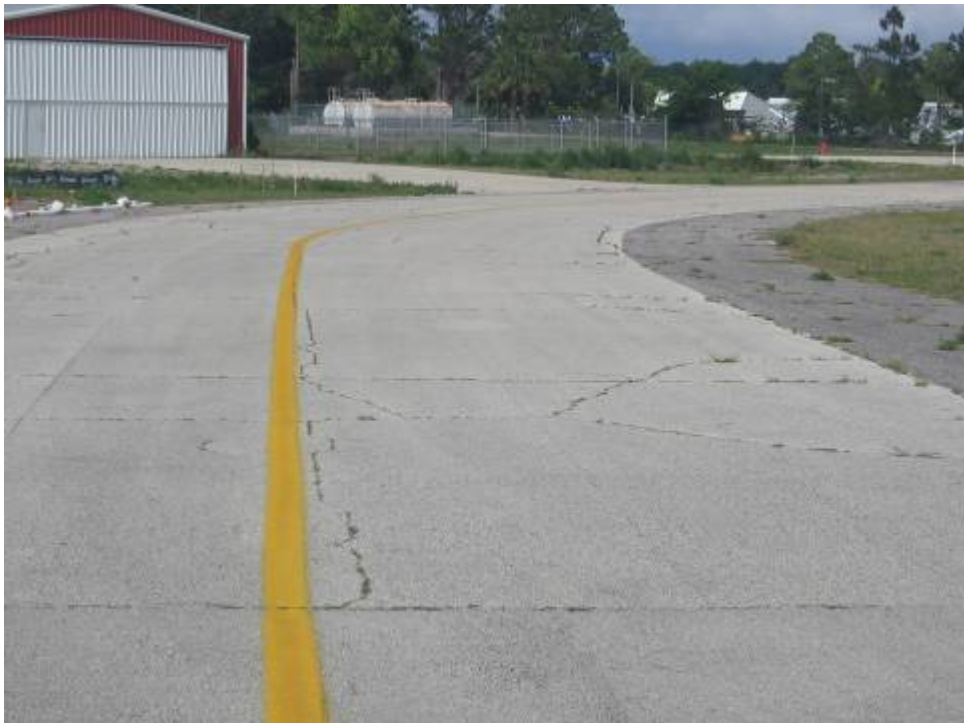
TW A Section 104: Medium Severity Block Cracking (May 24, 2007)
