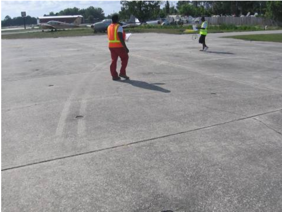
AP Section 4105: Low Severity Joint Seal Damage (May 24, 2007)
