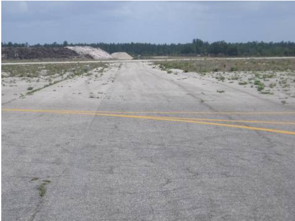
TW C Section 310: Low Severity Weathering (May 24, 2007)
