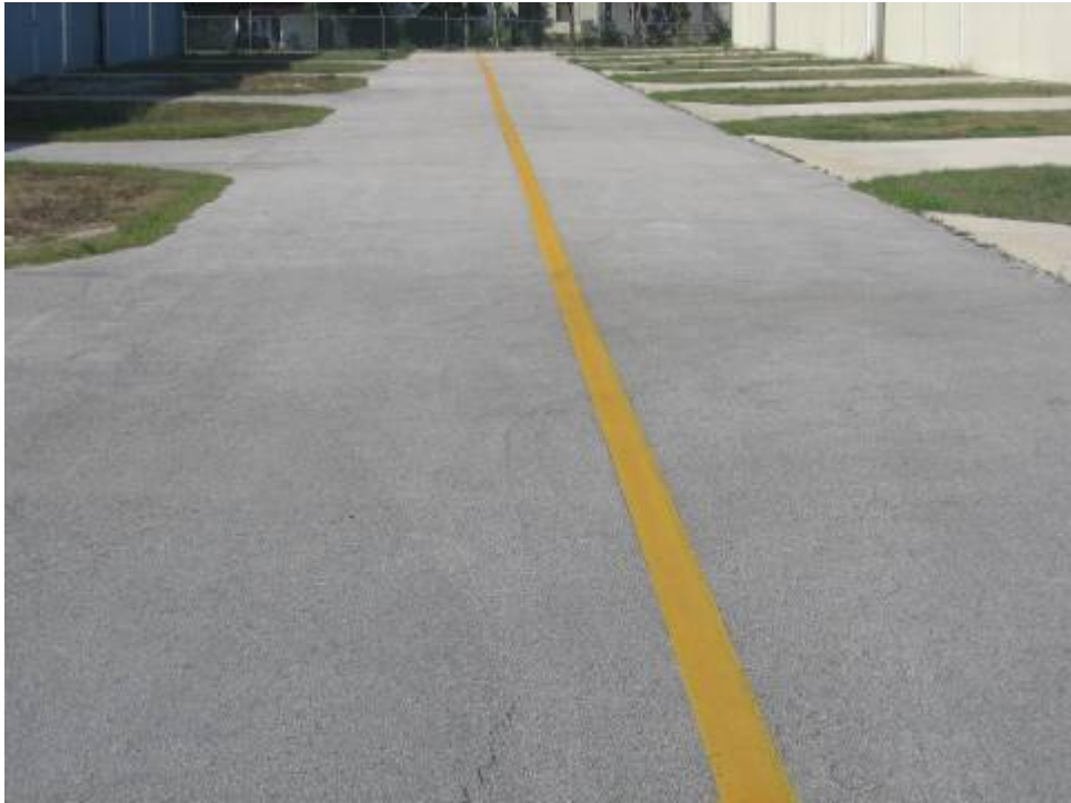
AP T-HANG Section 4315: Low Severity Weathering (May 24, 2007)
