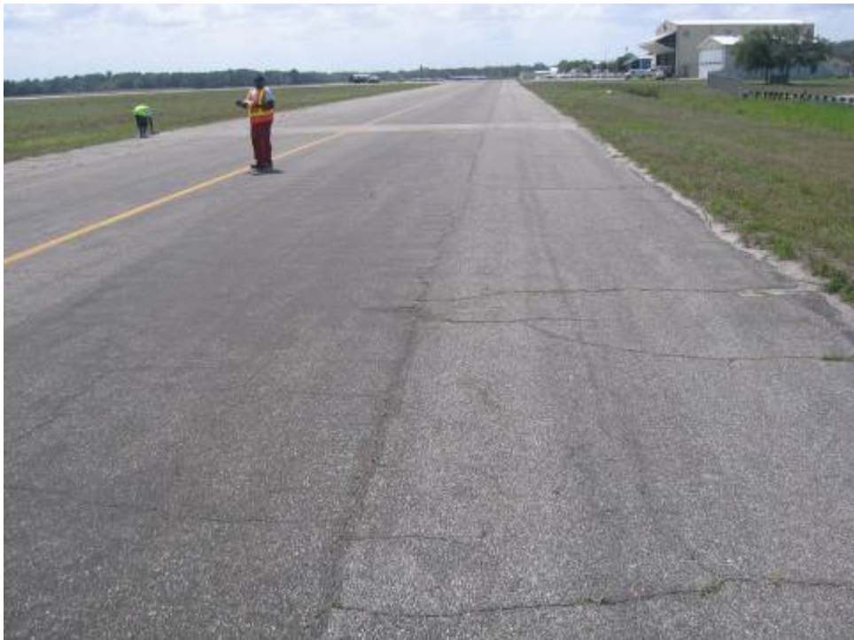
TW A Section 105: Low Severity Block Cracking (May 24, 2007)
