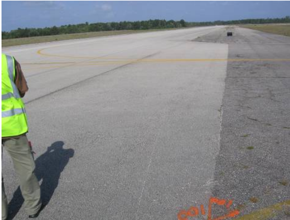
TW D Section 415: Low Severity Weathering (May 24, 2007)
