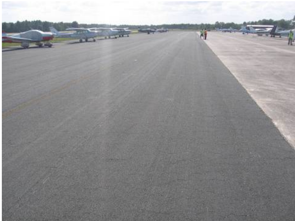
AP Section 4135: Low Severity Weathering (May 24, 2007)
