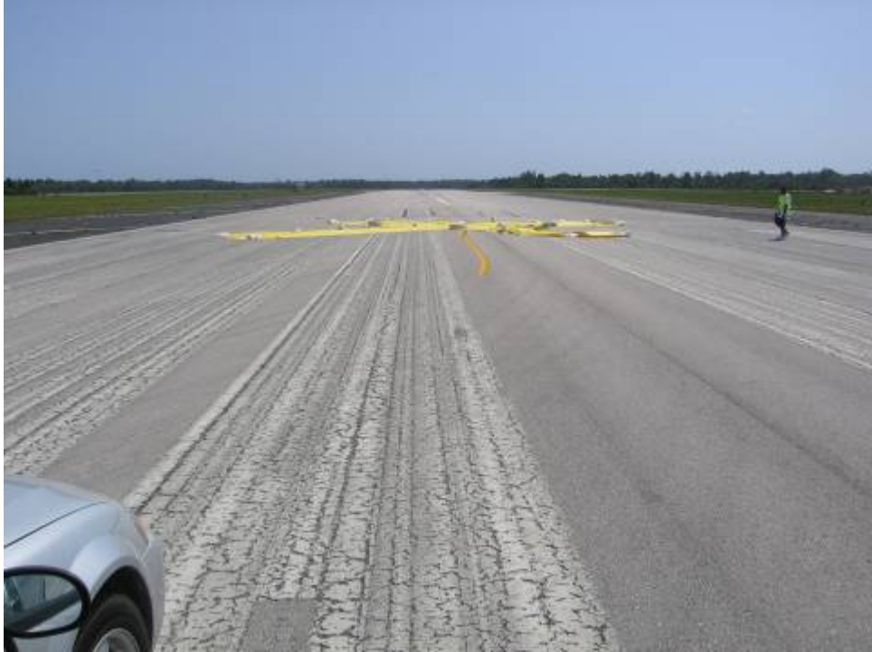
RW 6-24 Section 6205: Low Severity Weathering (May 24, 2007)
