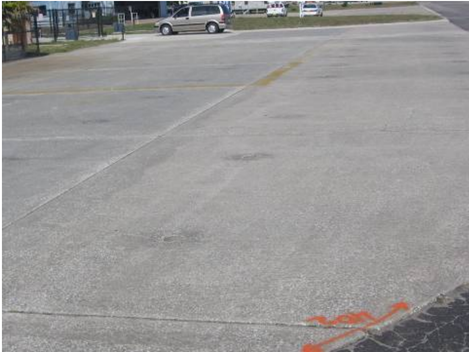
AP Section 4120: Low Severity Joint Seal Damage (May 24, 2007)
