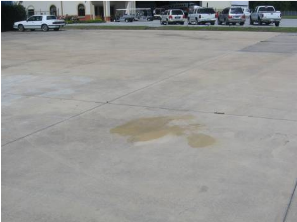
AP Section 4130: Low Severity Scaling (May 24, 2007)
