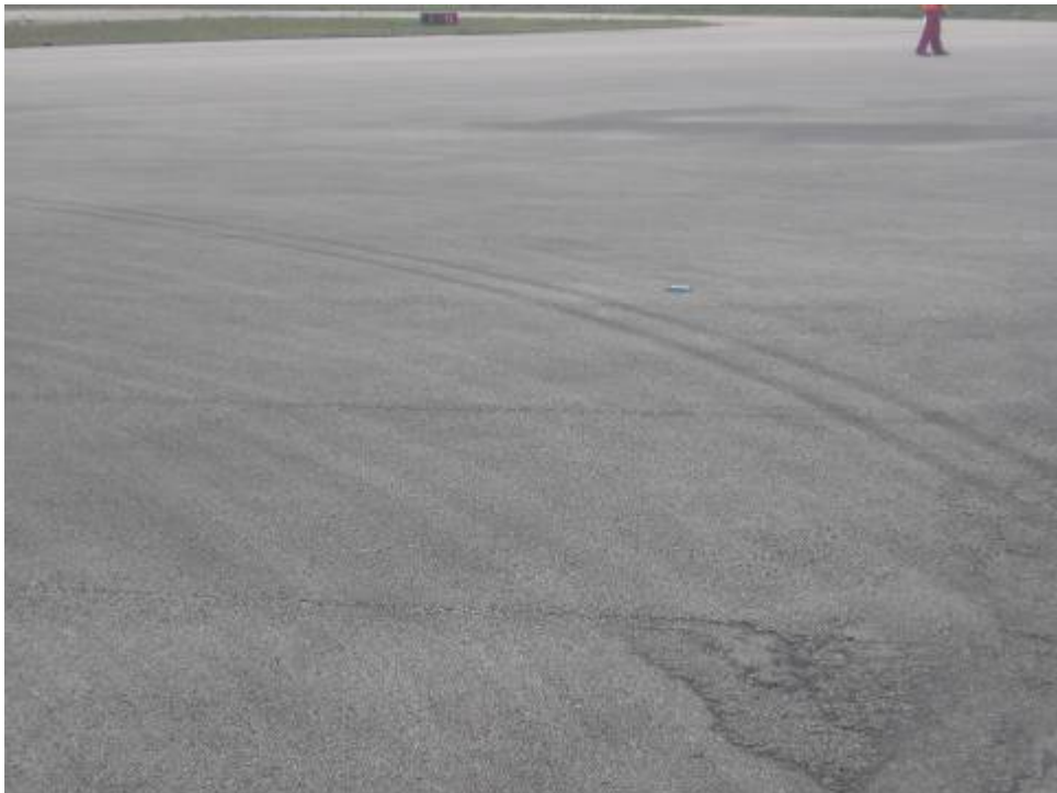
AP RU 11 Section 5105: Low Severity Weathering (May 24, 2007)
