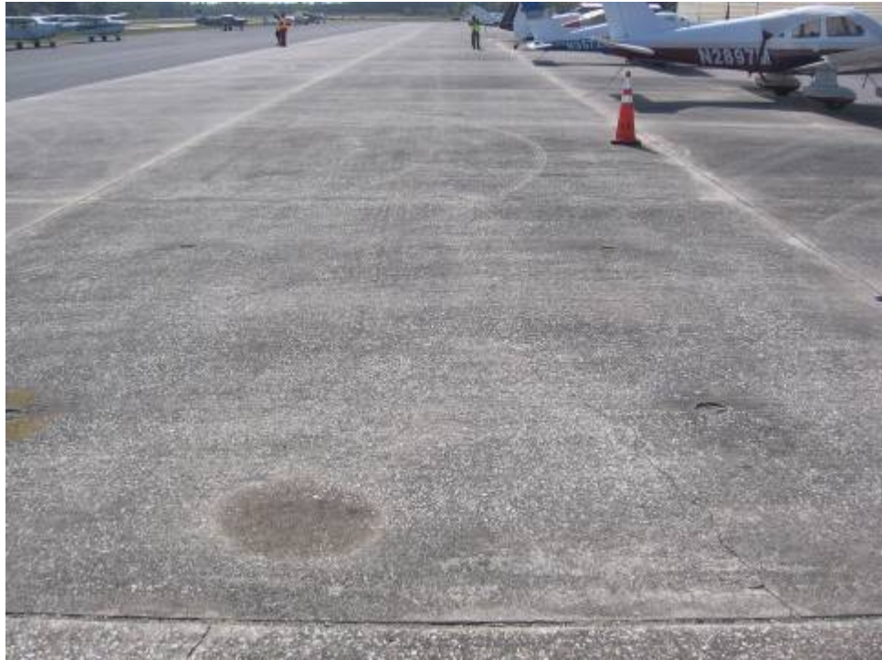
AP Section 4110: Low Severity Scaling (May 24, 2007)
