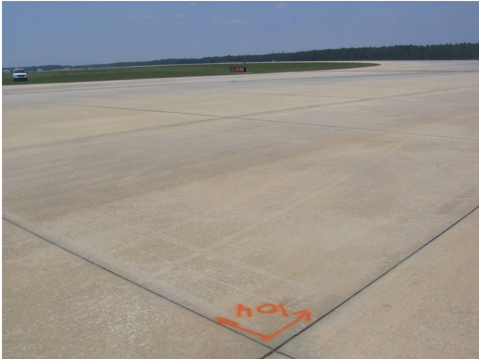
TW G Section 1060: Low Severity Scaling (May 14, 2007)
