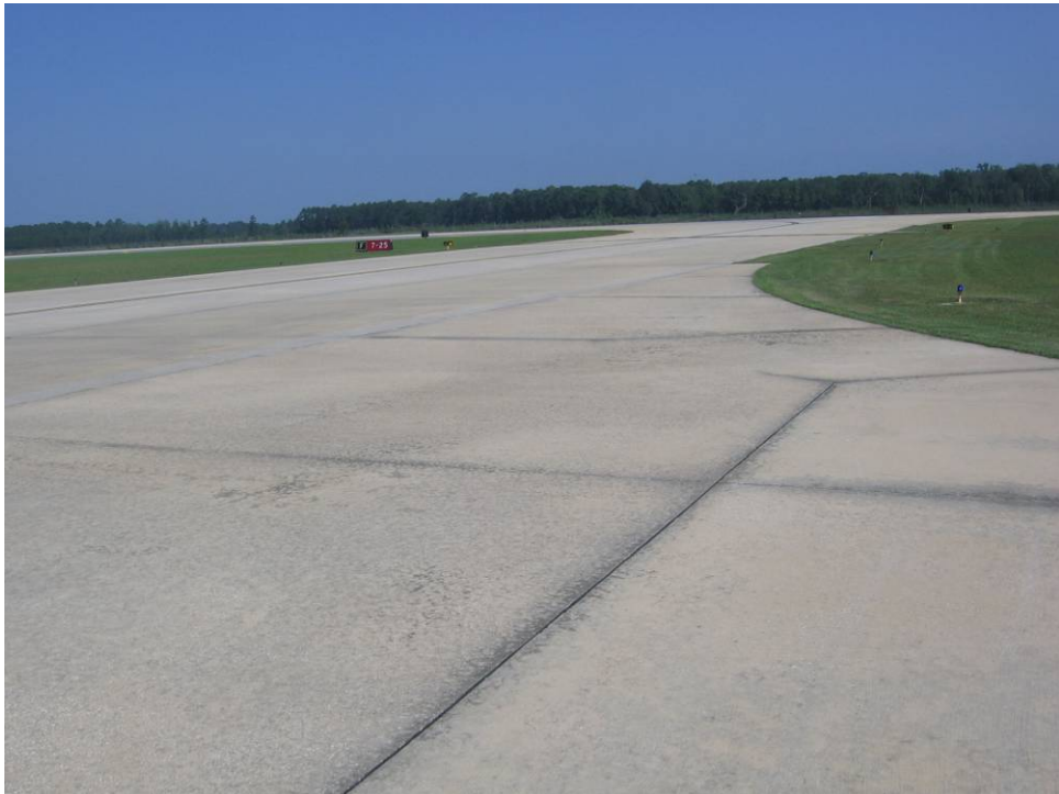
TW F Section 1175: Low Severity Scaling (May 14, 2007)
