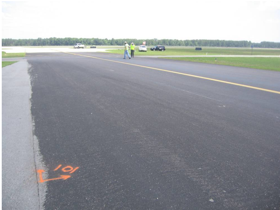
TW G Section 1030: Low Severity Weathering (May 14, 2007)
