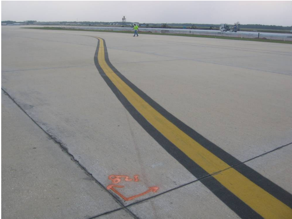
TW P Section 645: Low Severity Scaling (May 14, 2007)
