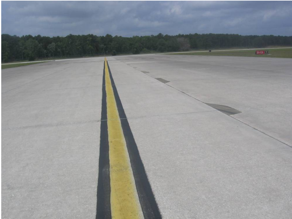
TW S, T Section 1280: Low Severity Small Patch (May 14, 2007)
