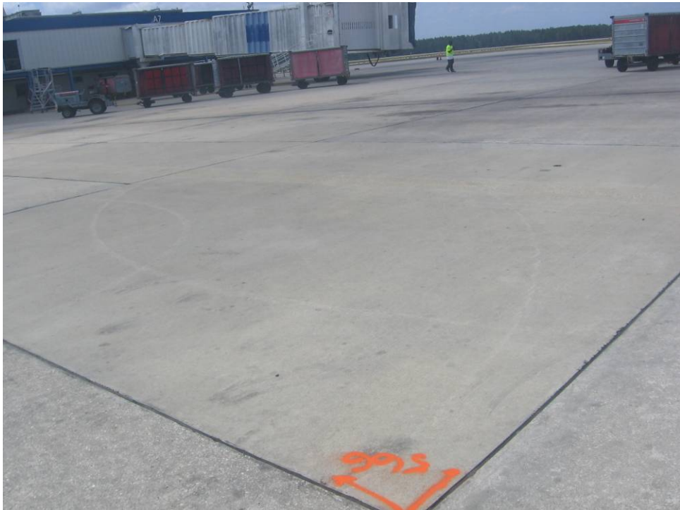
AP TERM Section 4375: Low Severity Scaling (May 14, 2007)
