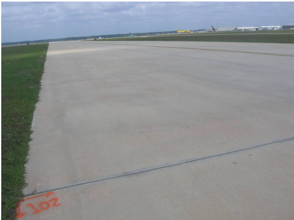
TW N, U Section 310: Low Severity Scaling (May 14, 2007)
