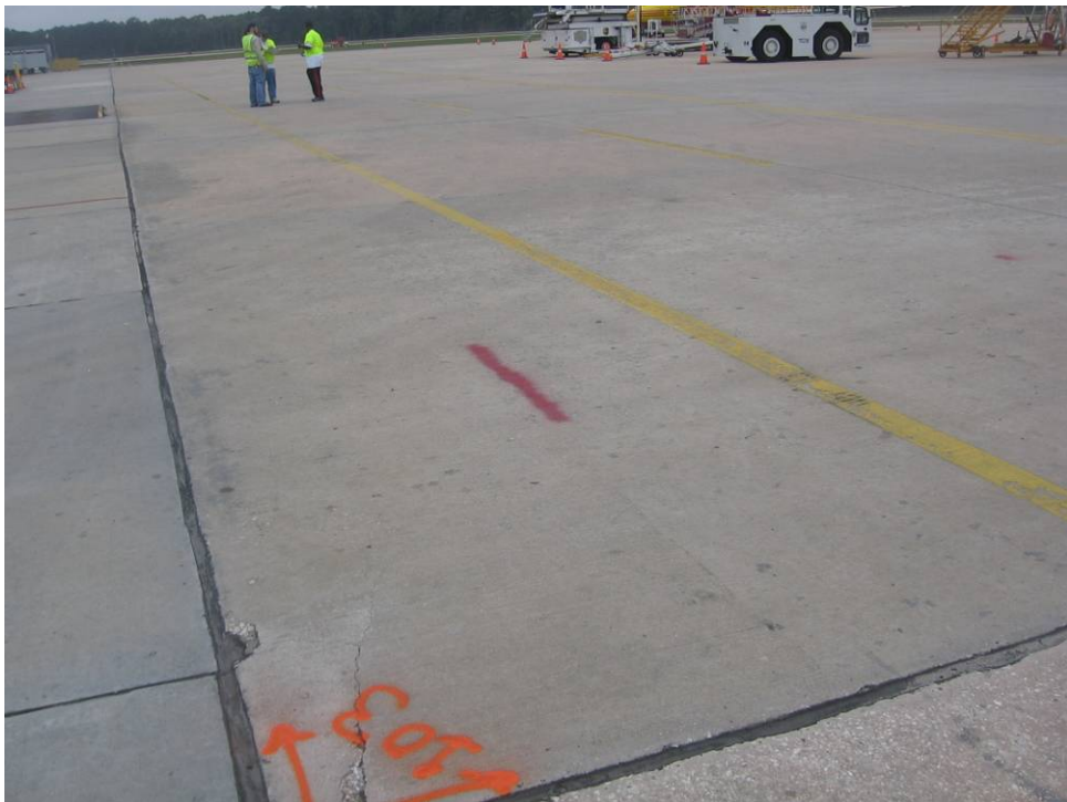
AP Cargo Section 4120: Low Severity Corner Spall (May 14, 2007)
