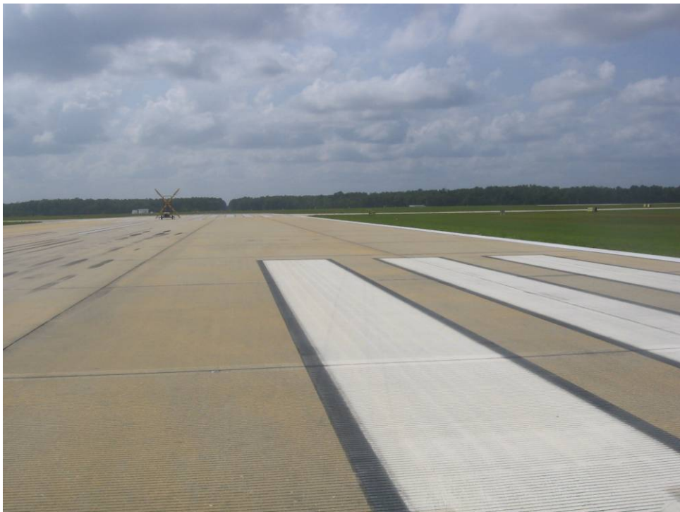
RW 13-31 Section 6225: Low Severity Small Patch (May 14, 2007)
