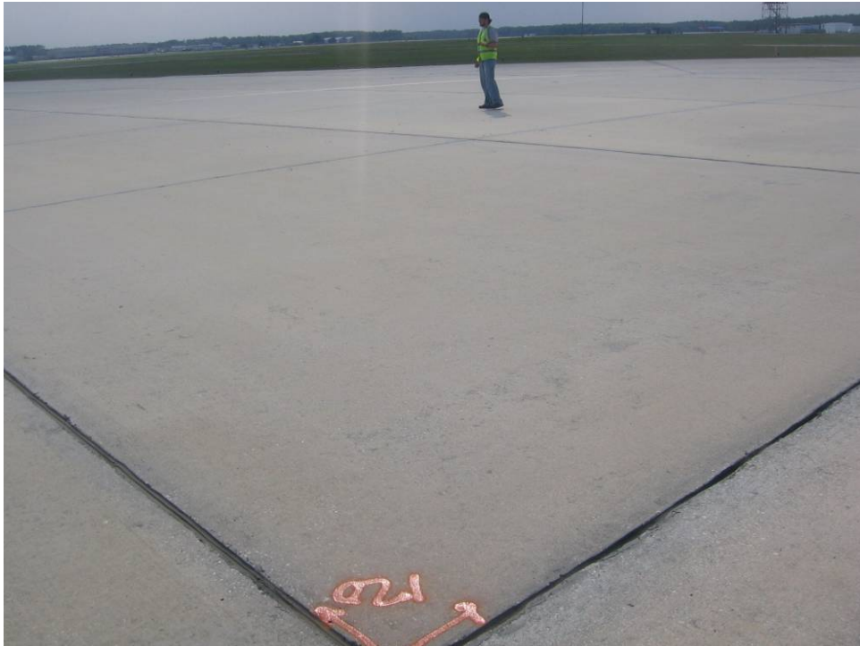
TW P Section 641: Low Severity Joint Seal Damage (May 14, 2007)
