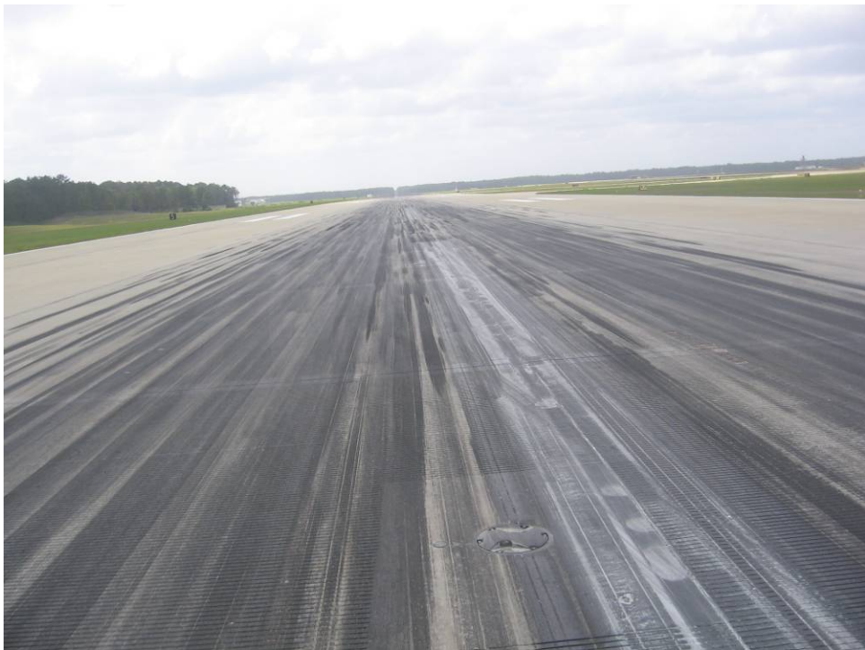
RW 13-31 Section 6210: Low Severity Small Patch (May 14, 2007)
