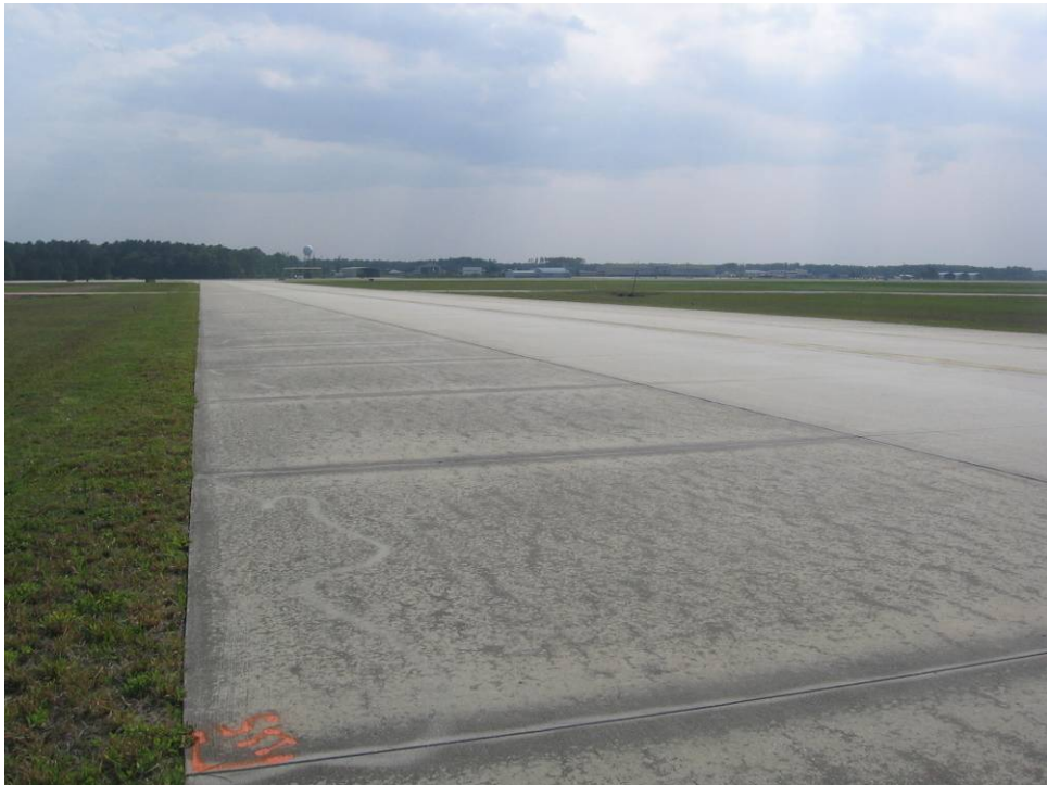
TW L Section 225: Low Severity Scaling (May 14, 2007)
