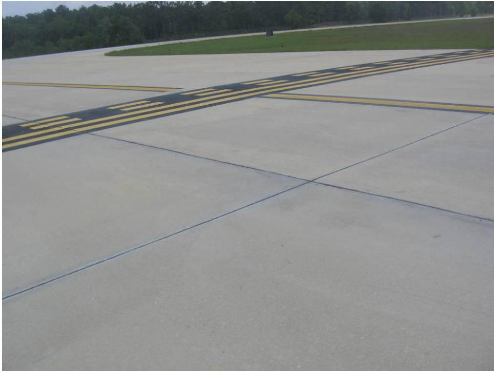
TW N, U Section 390: Low Severity Scaling (May 14, 2007)
