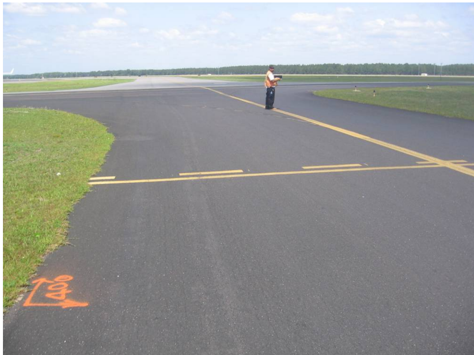
TW G Section 1035: Low Severity Weathering (May 14, 2007)
