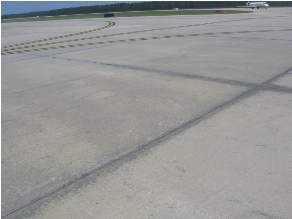
TW G Section 1020: Low Severity Scaling (May 14, 2007)
