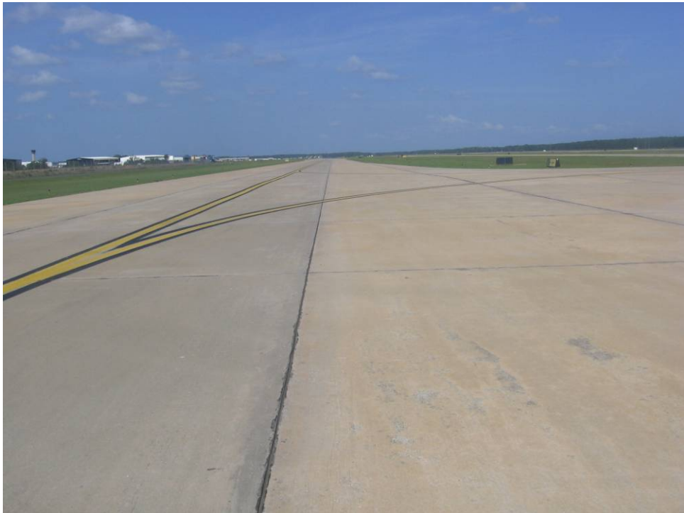
TW B Section 810: Low Severity Scaling (May 14, 2007)
