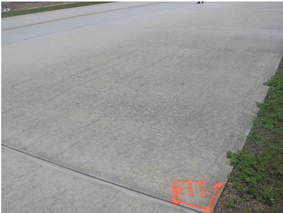
TW N, U Section 312: Low Severity Scaling (May 14, 2007)
