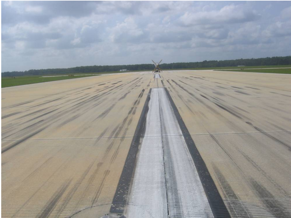
RW 13-31 Section 6220: Low Severity Large Patch (May 14, 2007)
