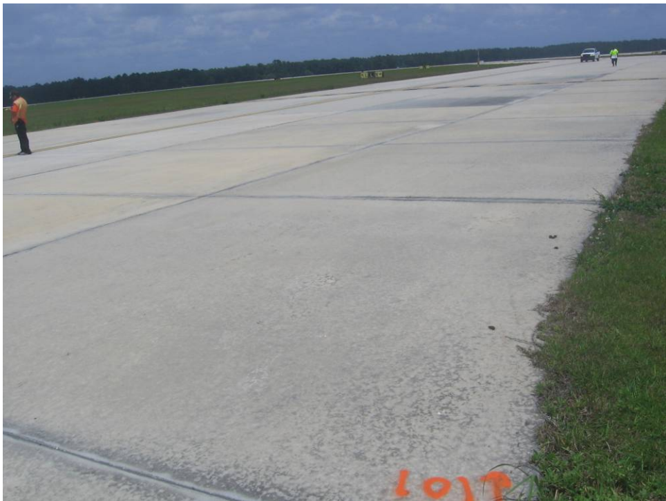
TW L Section 225: Low Severity Scaling (May 14, 2007)
