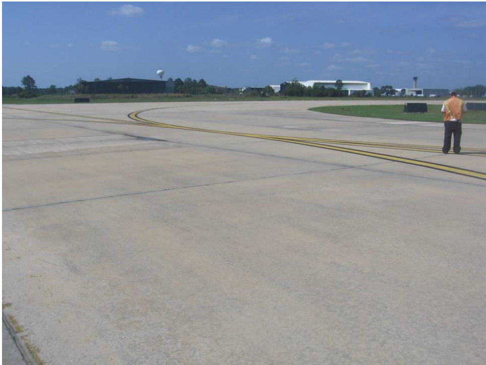
TW F Section 1145: Low Severity Scaling (May 14, 2007)
