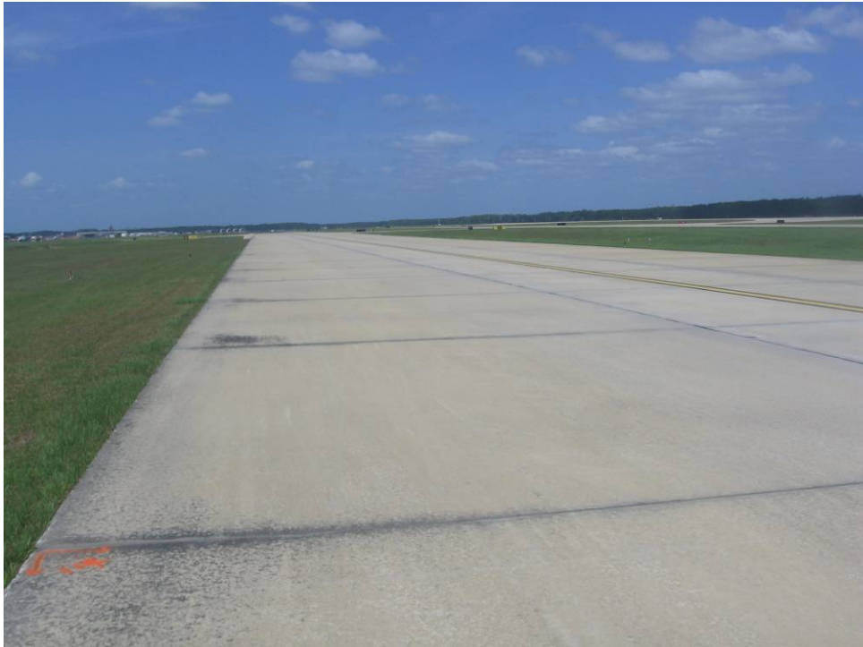
TW B Section 805: Low Severity Scaling (May 14, 2007)
