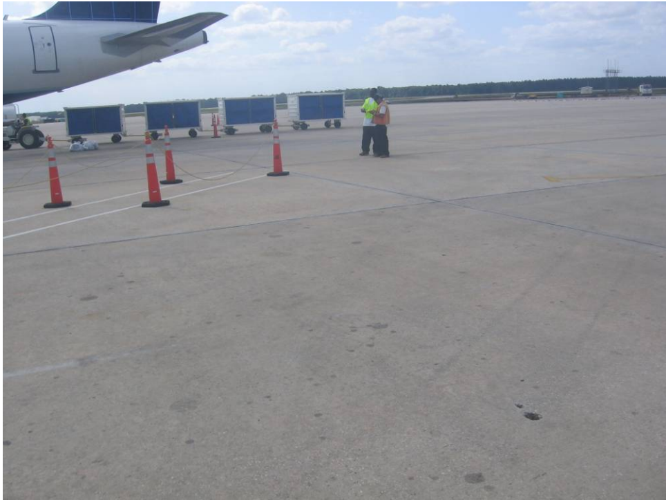
AP TERM Section 4330: Low Severity Scaling (May 14, 2007)
