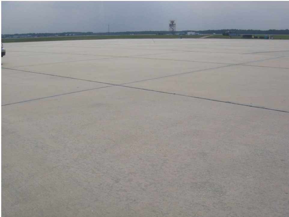
TW P Section 640: Low Severity Scaling (May 14, 2007)
