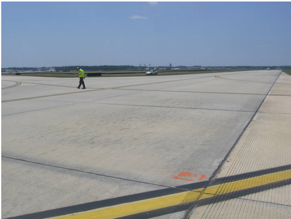
TW A Section 120: Low Severity Joint Seal Damage (May 14, 2007)
