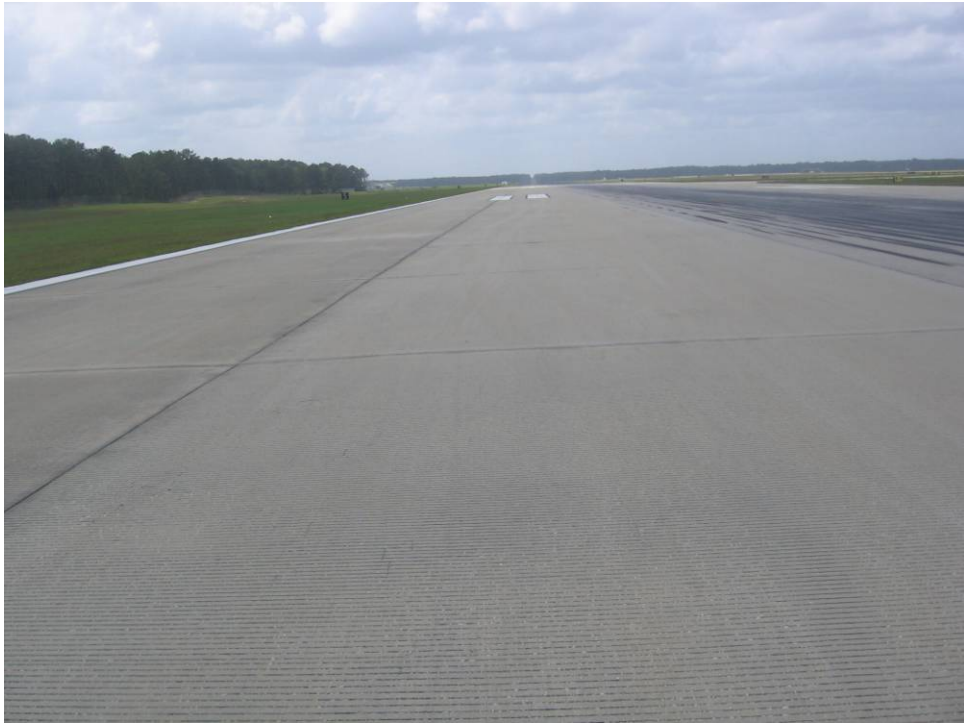
RW 13-31 Section 6215: Low Severity Scaling (May 14, 2007)
