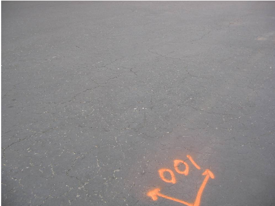
AP Cargo Section 4115 SU 100: Medium Severity Weathering (May 14, 2007)
