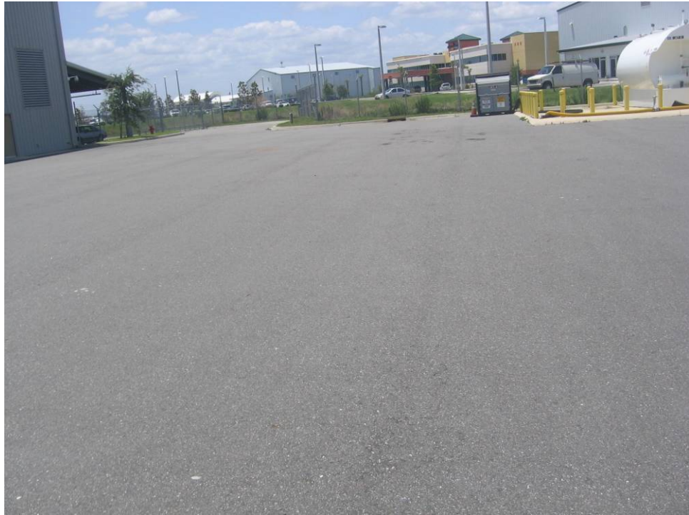
TW G Section 1045: Low Severity Weathering (May 14, 2007)
