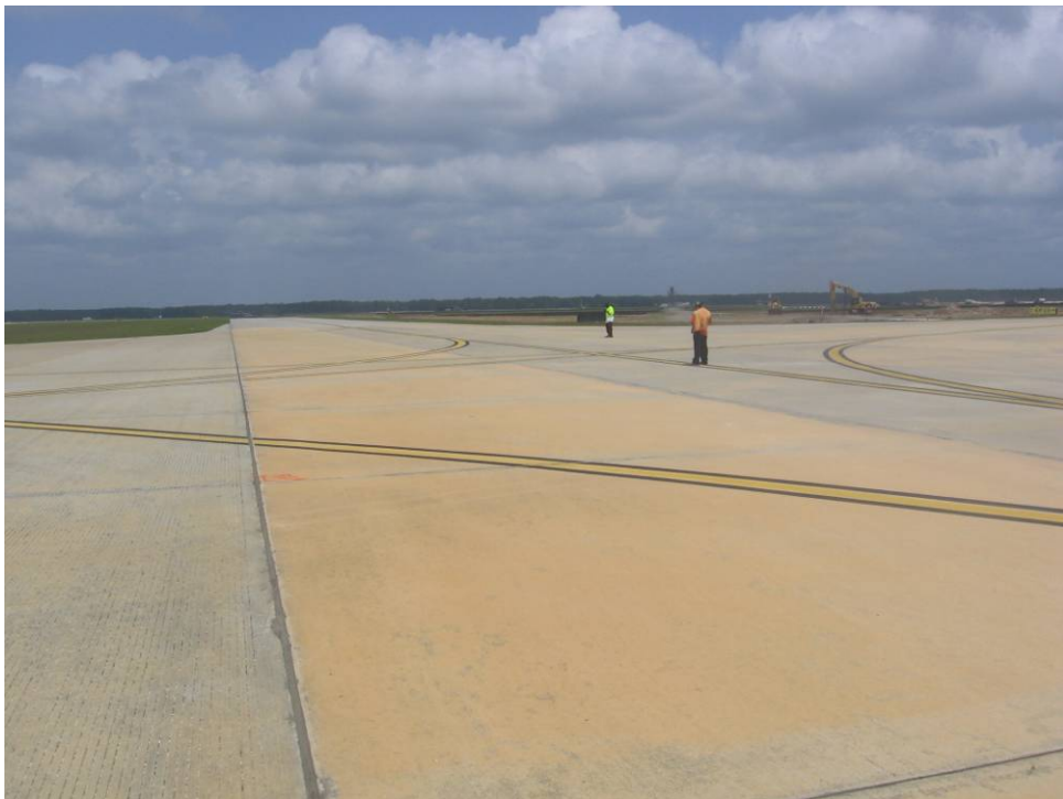
TW N, U Section 315: Low Severity Scaling (May 14, 2007)
