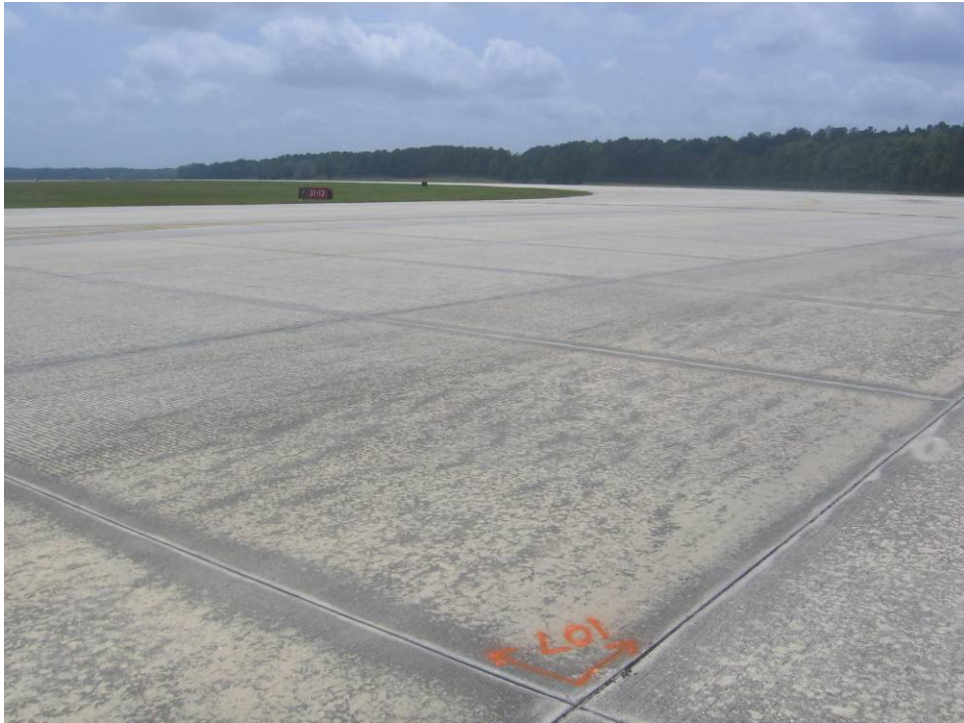
TW P Section 650: Low Severity Scaling (May 14, 2007)
