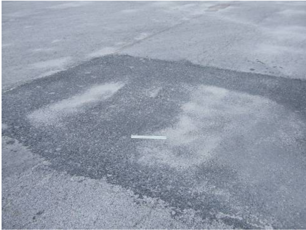
AP E Section 4228 SU 101: Medium Severity Patching (December 19, 2007)
