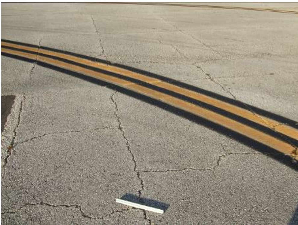
TW A6 Section 130 SU 605: Medium Severity Block Cracking (December 19, 2007)
