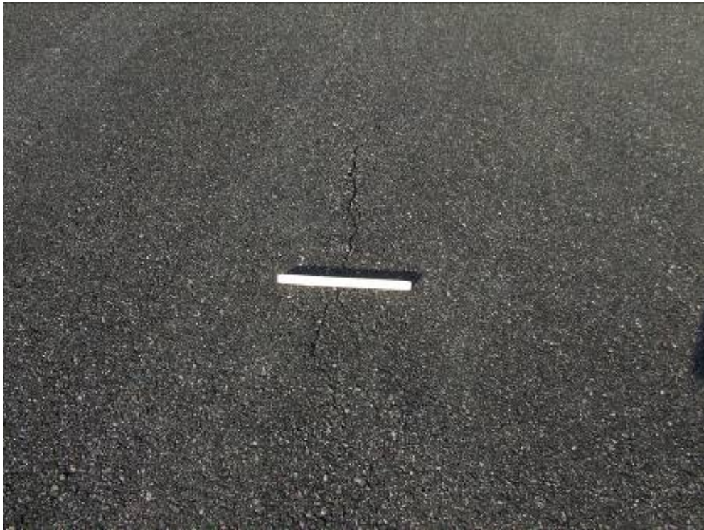
AP RW 10-28 Section 5125 SU 202: Low Severity L/T Cracking (December 19, 2007)
