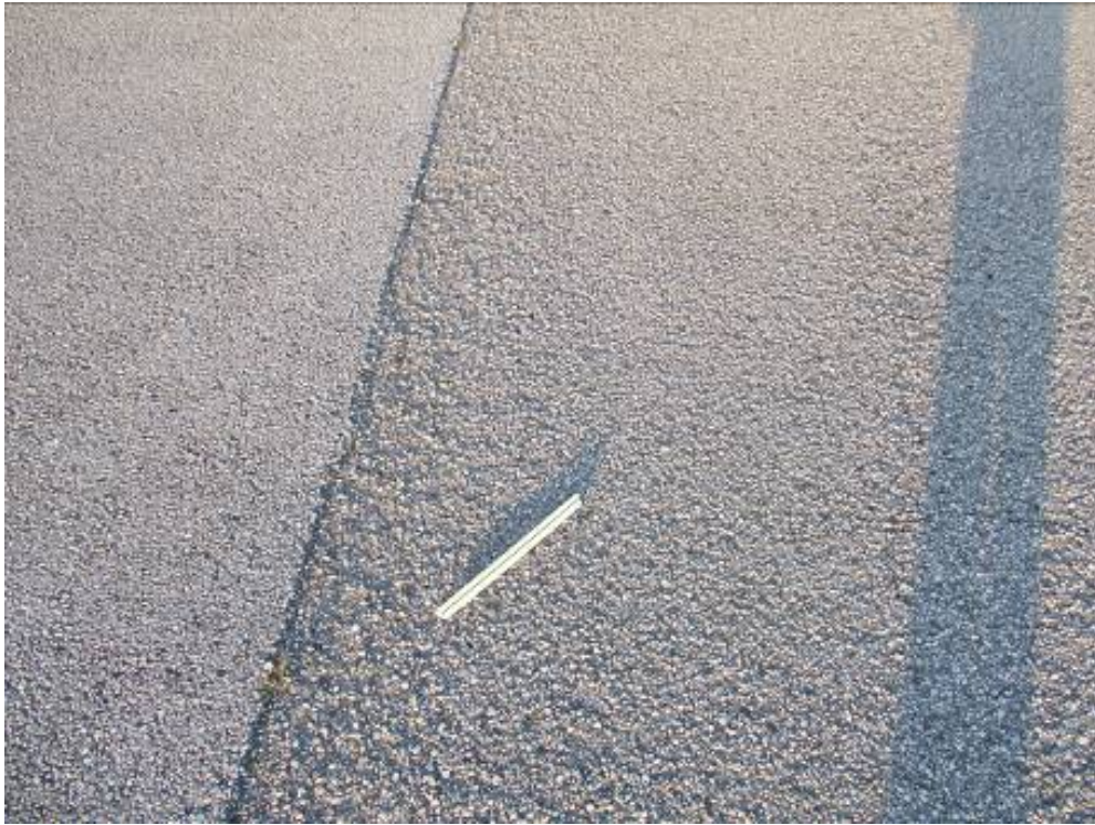
TW C Section 305 SU 102: Low Severity Weathering (December 19, 2007)
