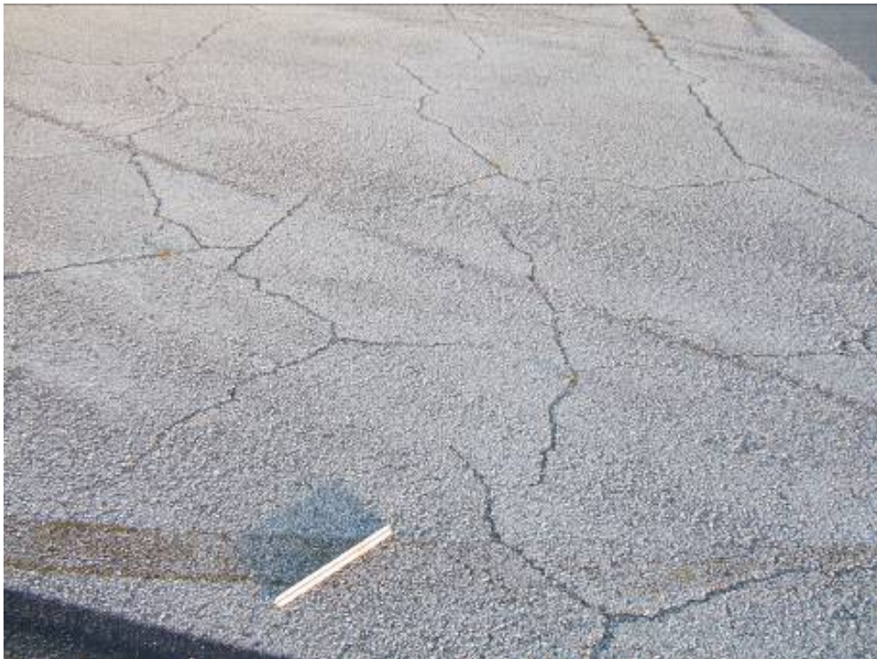
TW C Section 304 SU 100: Medium Severity Block Cracking (December 19, 2007)
