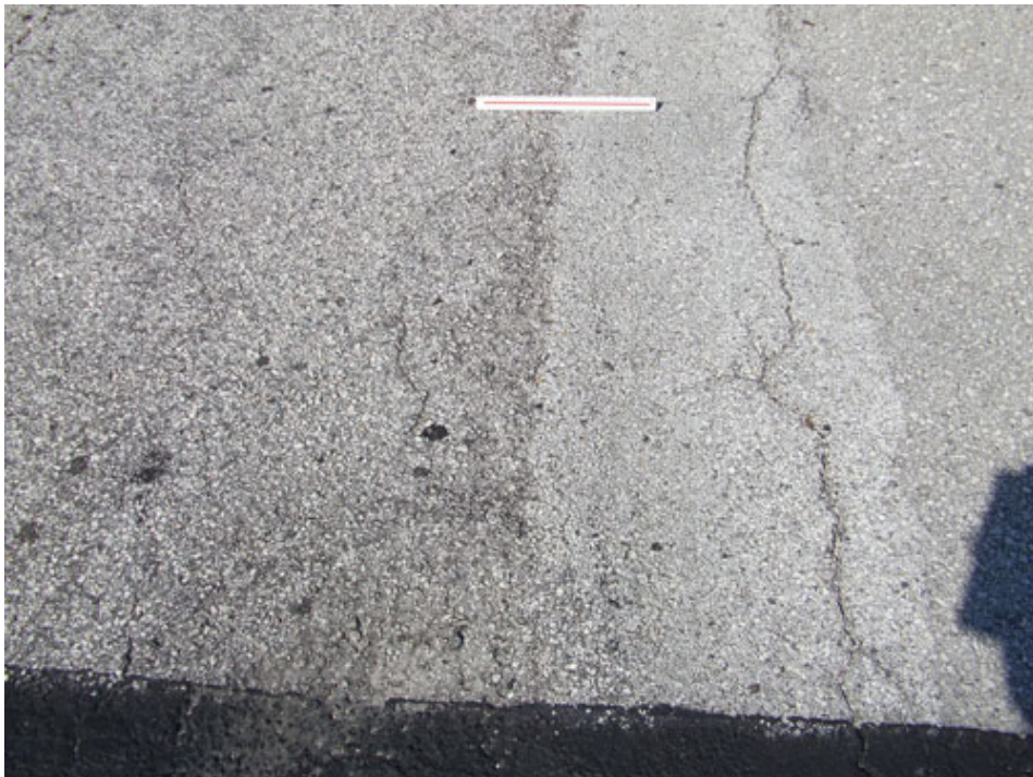
Taxiway P Section 1505 SU 101: Low Severity L/T Cracking (December 14, 2007)
