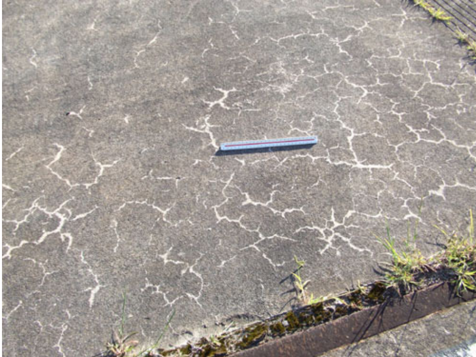
Apron E Section 4505 SU 202: Low Severity Scaling (December 14, 2007)
