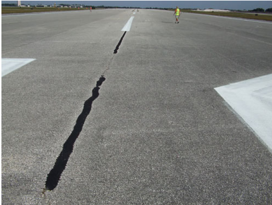
Runway 18-36 Section 6205 SU 301: Low Severity L/T Cracking (December 14, 2007)
