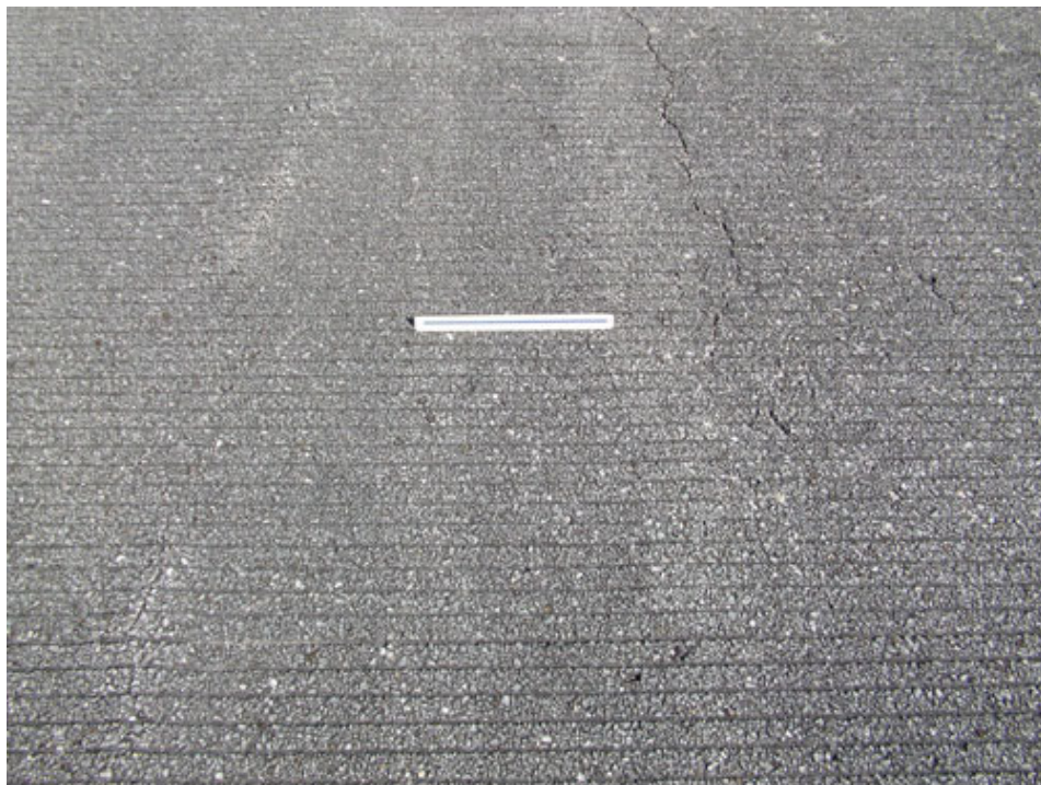
Runway 18-36 Section 6210 SU 104: Low Severity L/T Cracking (December 14, 2007)
