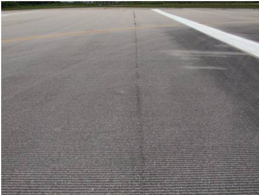
RW 5-23 Section 6160 SU 624: Low Severity L/T Cracking (August 13, 2007)
