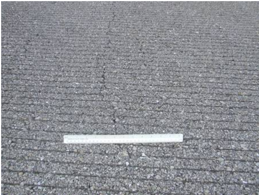
RW 5-23 Section 6105 SU 301: Low Severity L/T Cracking (August 13, 2007)
