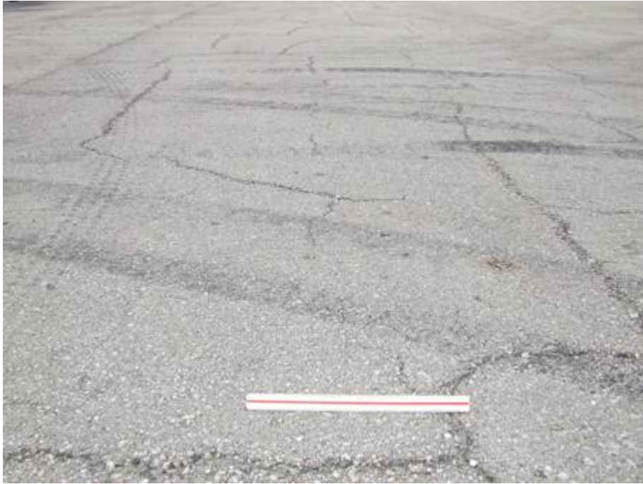
RW 13-31 Section 6210 SU 156: Medium Severity Block Cracking (August 13, 2007)
