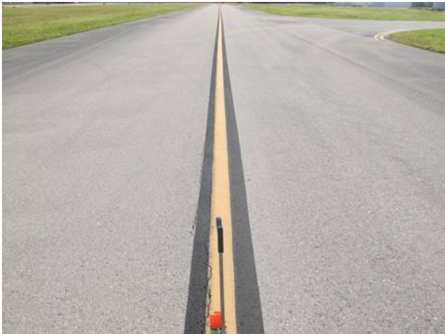
TW A Section 110 SU 118: Low Severity L/T Cracking (August 13, 2007)
