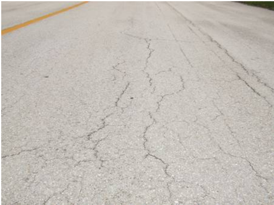
TW D-2 Section 160 SU 101: Low Severity Alligator Cracking (August 13, 2007)
