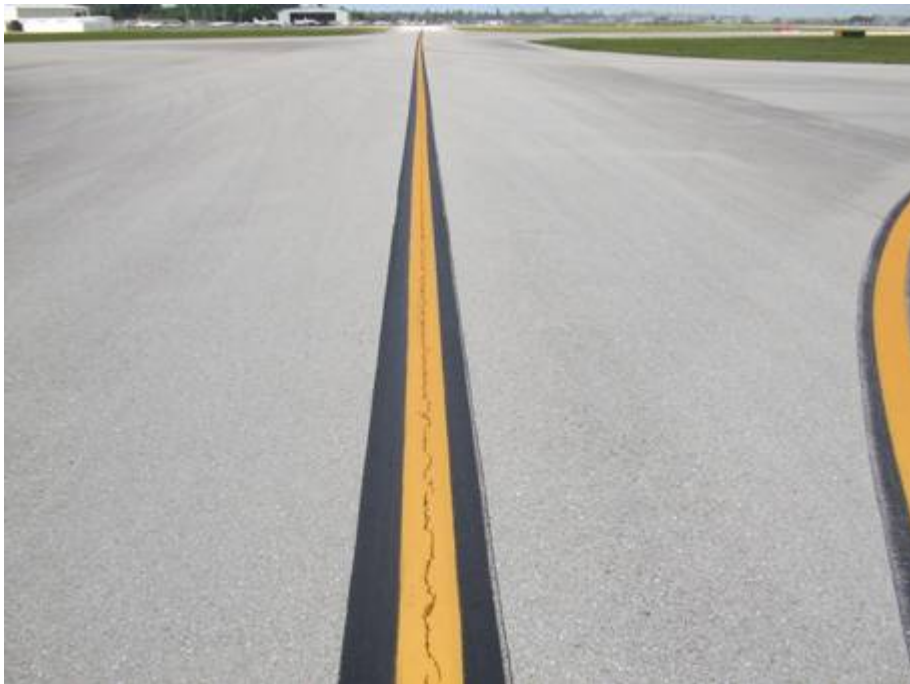
TW A Section 110 SU 141: Low Severity L/T Cracking (August 13, 2007)
