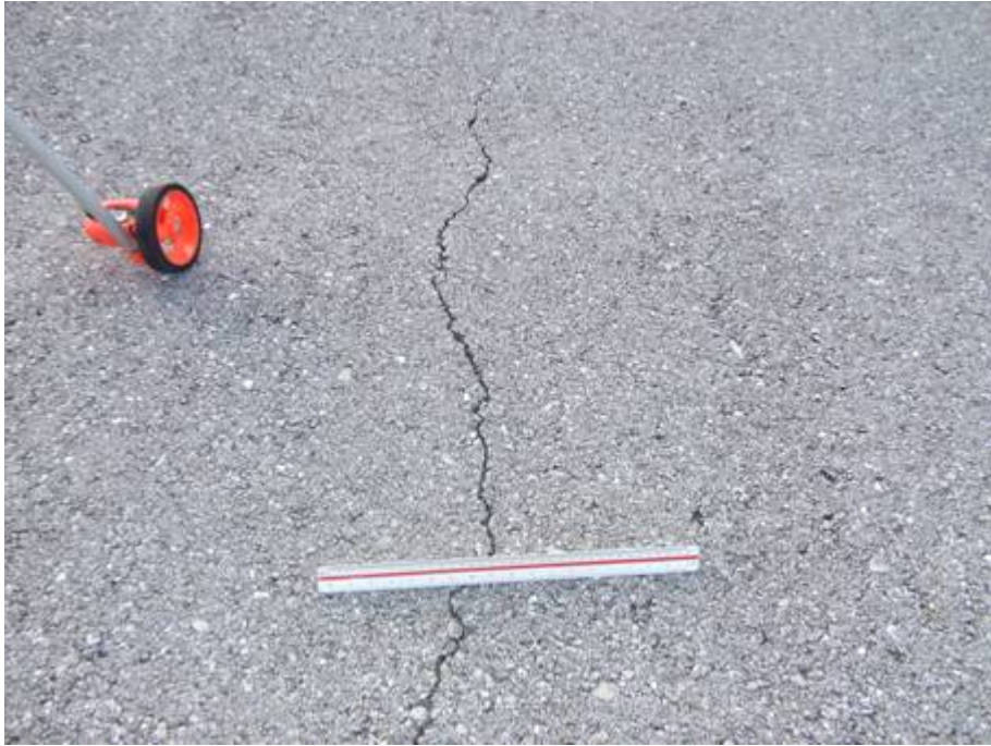
TW A-6 Section 180 SU 101: Low Severity L/T Cracking (August 13, 2007)
