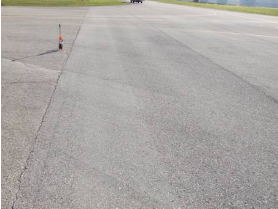
TW B Section 210 SU 120: Low Severity L/T Cracking (August 13, 2007)
