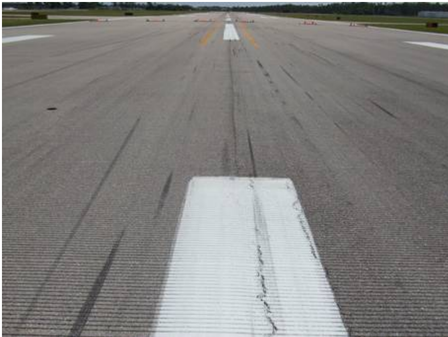
RW 5-23 Section 6125 SU 378: Medium Severity L/T Cracking (August 13, 2007)
