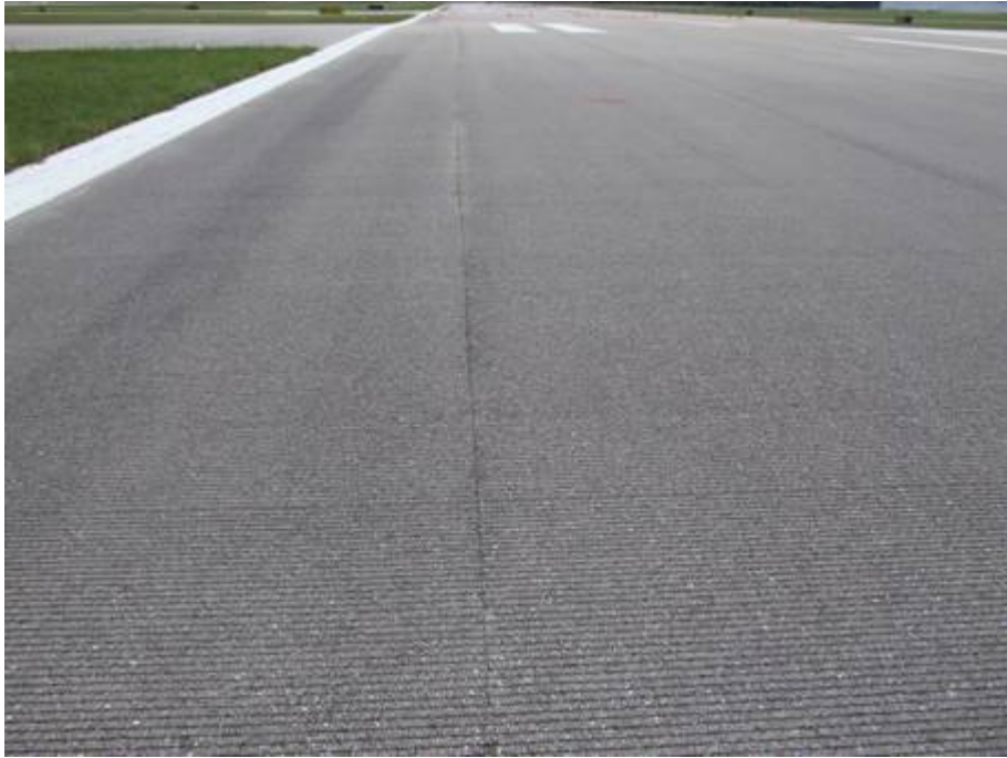
RW 5-23 Section 6130 SU 176: Low Severity L/T Cracking (August 13, 2007)
