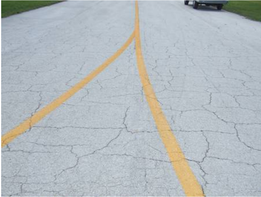
TW D-2 Section 162 SU 100: Medium Severity Block Cracking (August 13, 2007)
