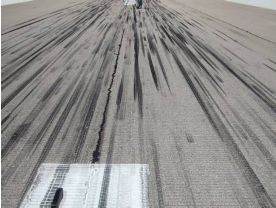
RW 5-23 Section 6145 SU 397: Low Severity L/T Cracking (August 13, 2007)
