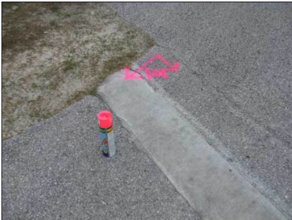
Apron General Aviation, Section 4010, Sample Unit 101 – Low severity (48) Longitudinal and Transverse Cracking, low severity (50) Patching, low severity (52) Weathering and Raveling.
