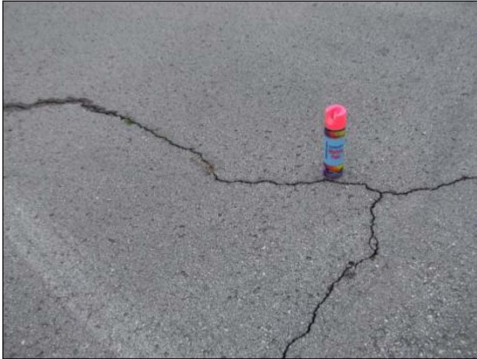
Apron General Aviation, Section 4005, Sample Unit 201 – Low severity (48) Longitudinal and Transverse Cracking, low severity (52) Weathering and Raveling.
