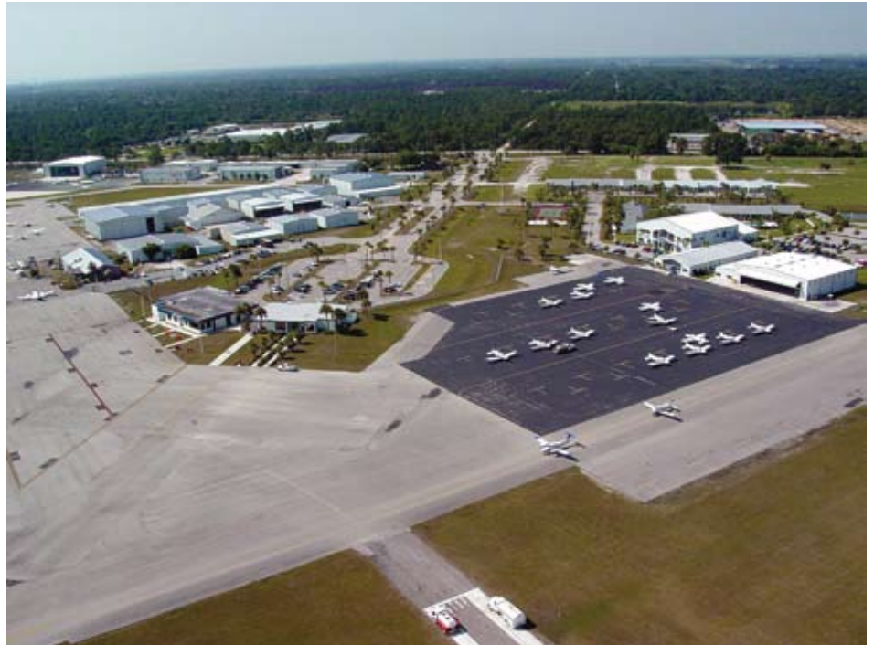
Courtesy of St. Lucie County International Airport
