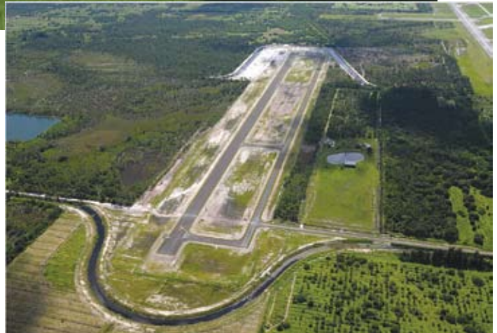
Photographs courtesy of St. Lucie County International Airport
