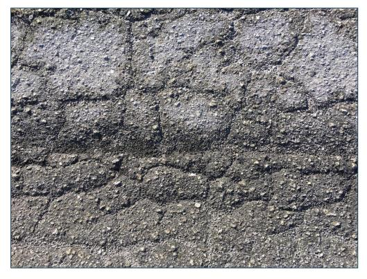
Taxiway C, Section 305, Sample Unit 305 - Medium Severity (41) Alligator Cracking, Low Severity (53) Rutting, Low Severity (52) Raveling
