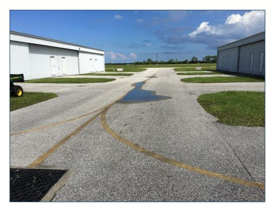
Apron T-Hang, Section 5305, Sample Unit 301 – Low Severity (48) Longitudinal and Transverse Cracking, Low Severity (45) Depression, Low Severity (57) Weathering
