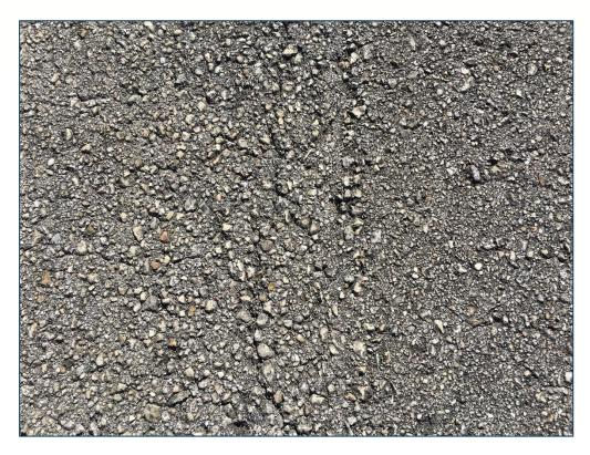
Runway 10-28, Section 6305, Sample Unit 514 - Low Severity (52) Raveling
