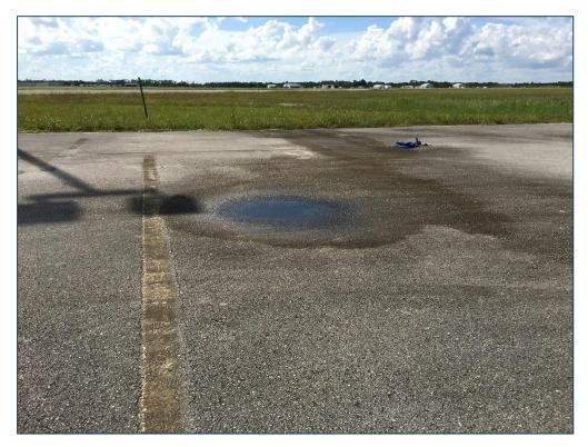
Apron Term, Section 5705, Sample Unit 101 - Low Severity (45) Depression, Low Severity (57) Weathering
