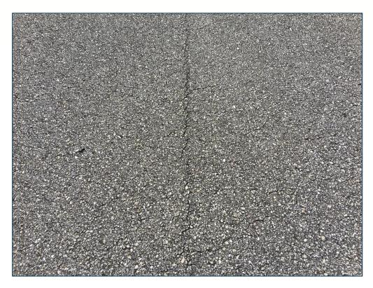
Apron RU SW, Section 5405, Sample Unit 301 - Low Severity (48) Longitudinal and Transverse Cracking, Low Severity (57) Weathering
