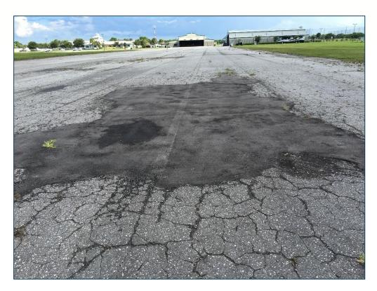
Apron SE, Section 5605, Sample Unit 101 – Low Severity (43) Block Cracking, Medium Severity (50) Patching, Medium Severity (41) Alligator Cracking, Low Severity (52) Raveling
