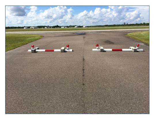
Taxiway E, Section 700, Sample Unit 101 - Low Severity (48) Longitudinal and Transverse Cracking, Low Severity (57) Weathering
