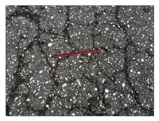
Apron SE, Section 5605, Sample Unit 203 – Low Severity (41) Alligator Cracking, Low Severity (43) Block Cracking, Low Severity (52) Raveling
