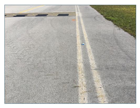
Taxiway CONN, Section 515, Sample Unit 100 - Low Severity (48) Longitudinal and Transverse Cracking, Low Severity (57) Weathering, Low Severity (52) Raveling
