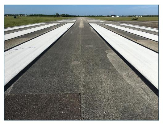
Runway 5-23, Section 6205, Sample Unit 379 – Low Severity (48) Longitudinal and Transverse Cracking, Low Severity (50) Patching, Low Severity (57) Weathering, Low Severity (52) Raveling
