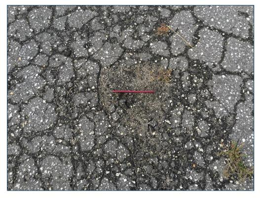
Apron SE, Section 5605, Sample Unit 101 - Low Severity (52) Raveling and Medium Severity (41) Alligator Cracking
