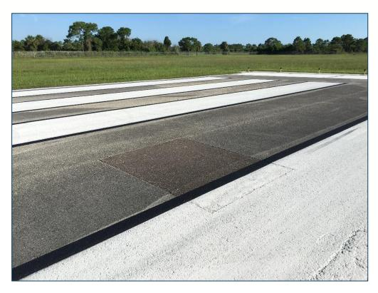
Runway 5-23, Section 6205, Sample Unit 379 - Low Severity (48) Longitudinal and Transverse Cracking, Low Severity (50) Patching, Low Severity (57) Weathering
