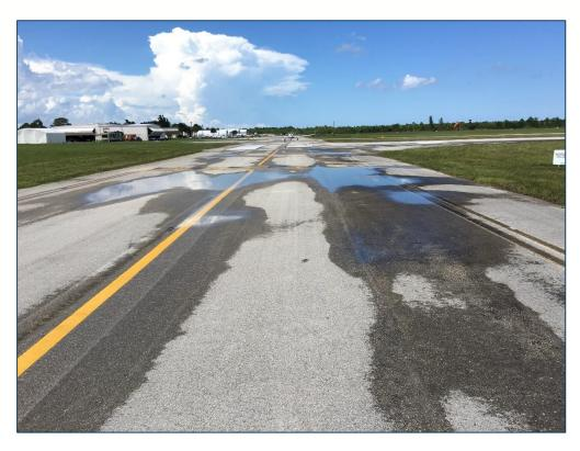
Taxiway A, Section 425, Sample Unit 99 – Low Severity (45) Depression, Low Severity (52) Raveling, Low Severity (48) Longitudinal and Transverse Cracking, Low Severity (57) Weathering
