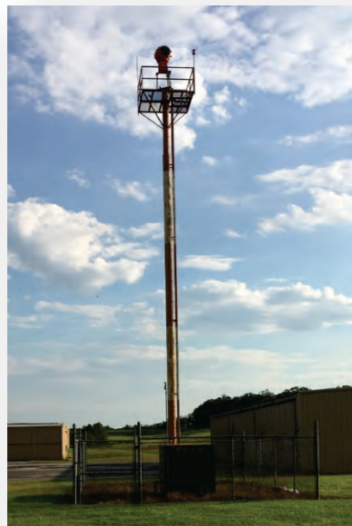
Photo 3 - Existing Rotating Beacon Source: AECOM (2018)
