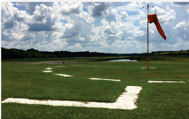
Photo 4 - Segmented Circle collocated with a lighted Wind Cone Source: AECOM (2018)
