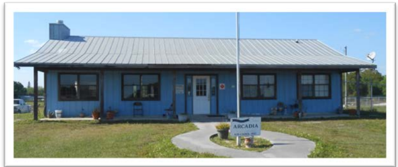
Existing Terminal Building
