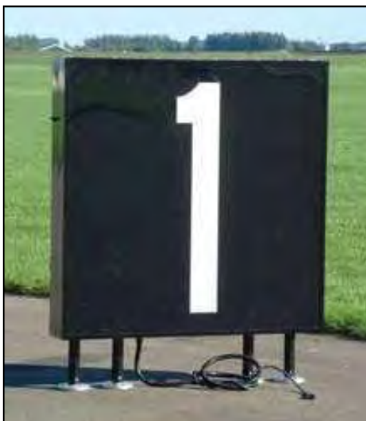
Typical Runway Distance Remaining Sign indicating 1000 feet left until the end of the runway
