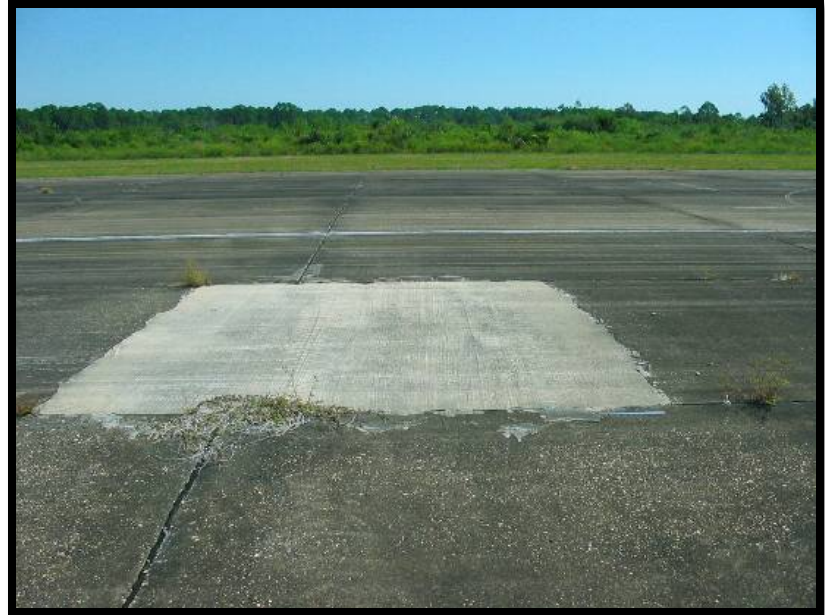
Low Severity Patching: Little or no deterioration
