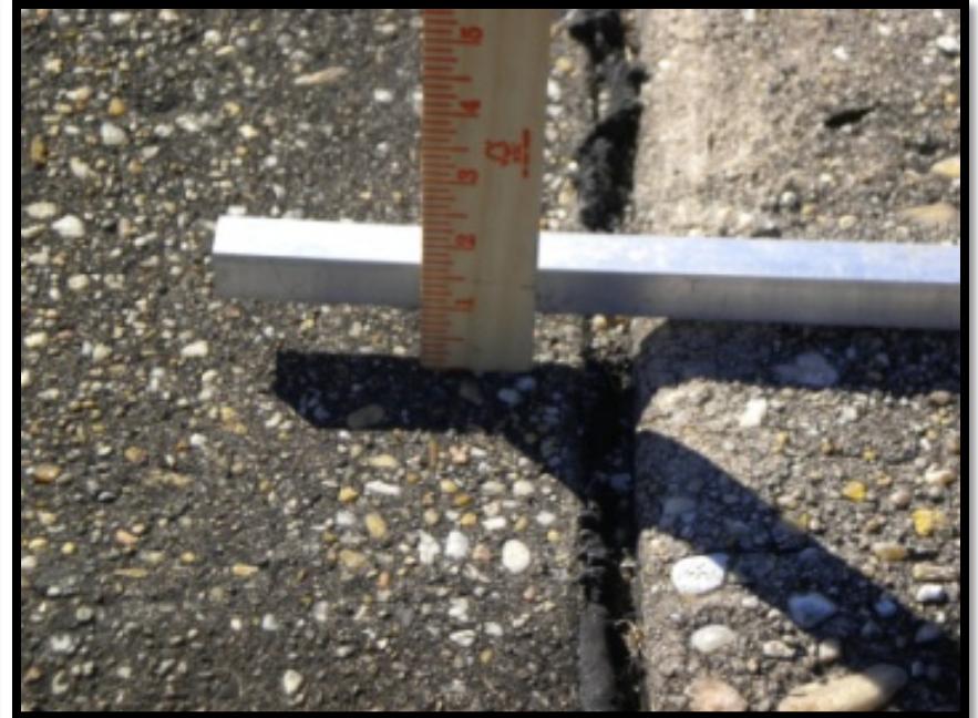
High Severity Settlement: Settlement on the Runway (inoperable)
