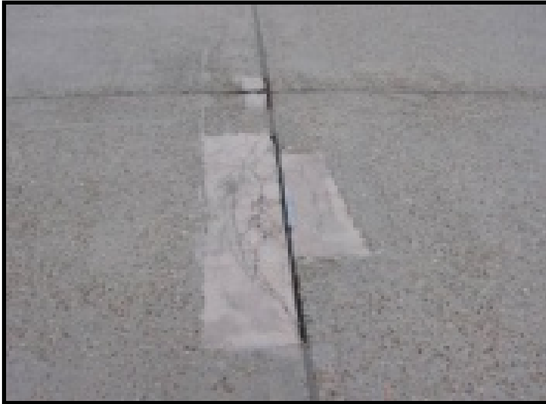
Medium Severity Patching: Small patch; moderate spalling
