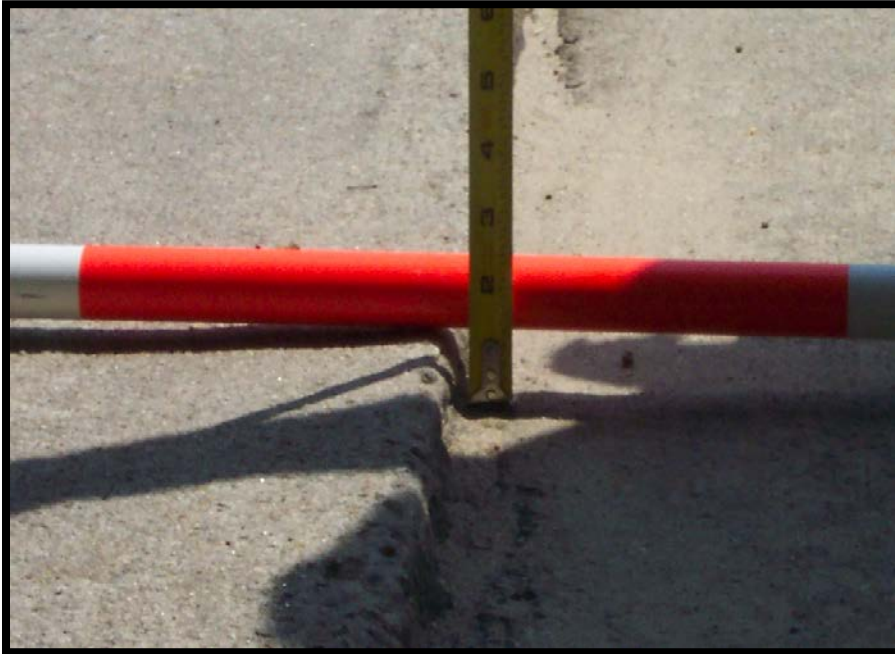
High Severity Settlement: Settlement on the Runway (inoperable)
