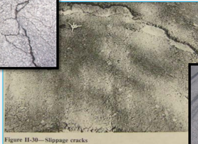
Figure II-30—Slippage cracks
