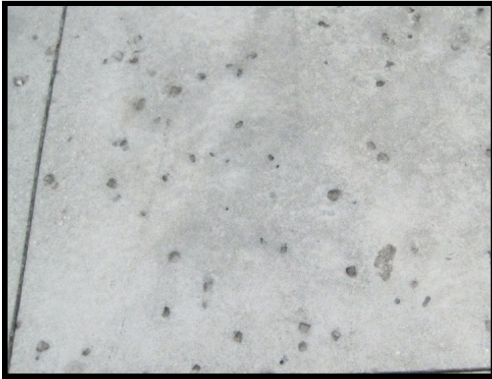
Extensive pop-outs of large aggregate from surface.
