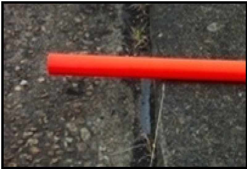
Low Severity Settlement: \frac{3}{4} " at the apron
