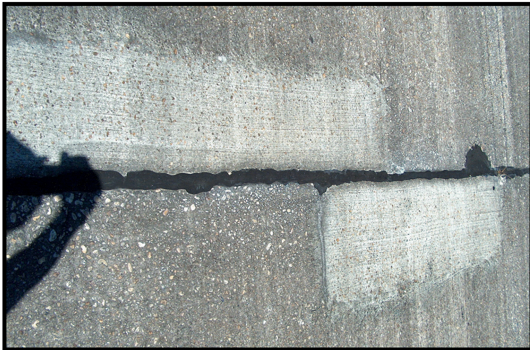
Low Severity Patching: Small patch; little or no deterioration
