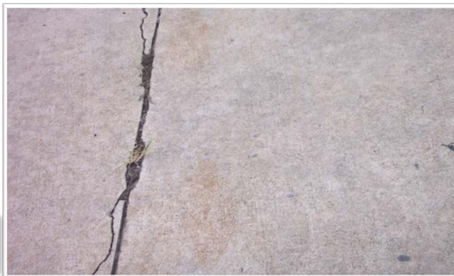
Low Severity D-Cracking: D-Cracking
