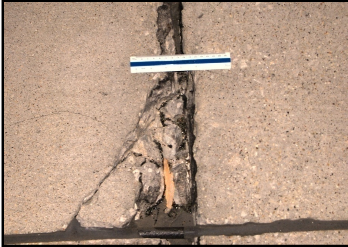
High Severity Corner Spalling: Heavily damaged; badly FOD
