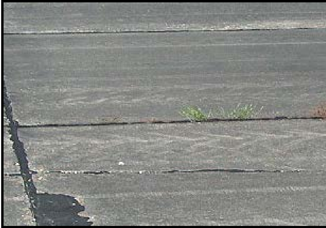
Medium Severity Longitudinal Cracking: Moderately spalled, some FOD
