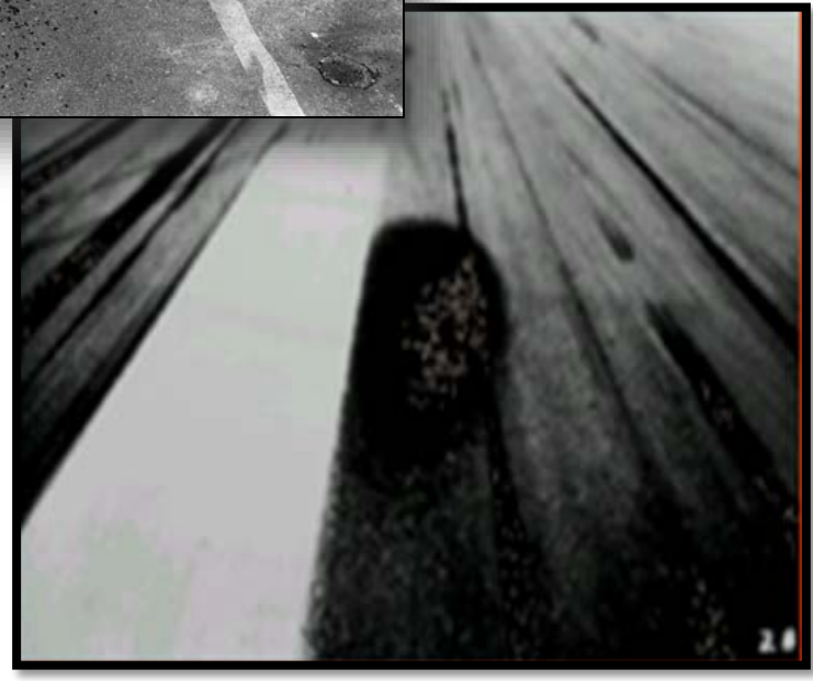
Jet Blast Erosion: (No severity) Common at the end of runways
