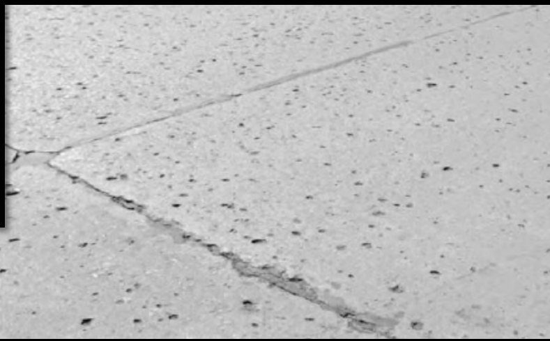
Extensive pop-outs of large aggregate from surface.
