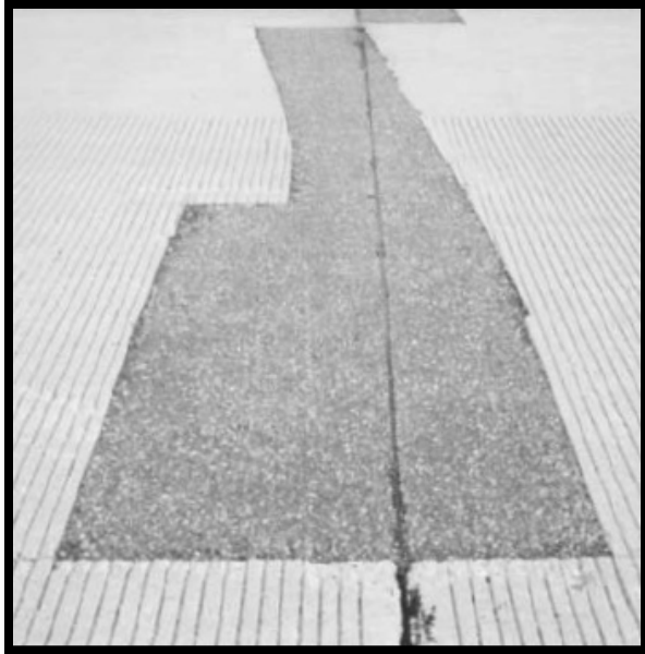
Low Severity Patching: Little or no deterioration
