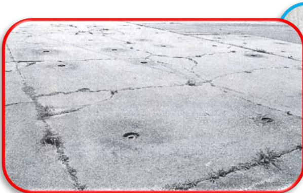
Shattered slab
