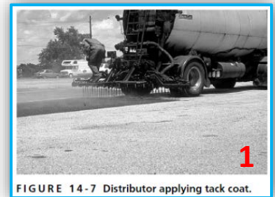
FIGURE 14-7 Distributor applying tack coat.
