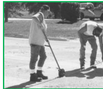
Installation of backer rod
