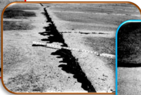
Medium -severity settlement on apron >1/2 in.
