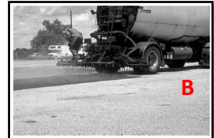
FIGURE 14-7 Distributor applying tack coat.
