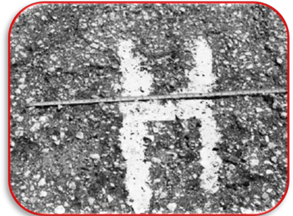
High-Severity Raveling, Dense Mix
