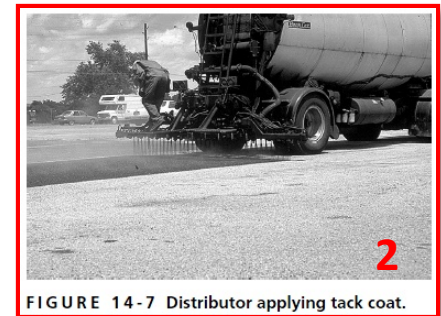
FIGURE 14-7 Distributor applying tack coat.
