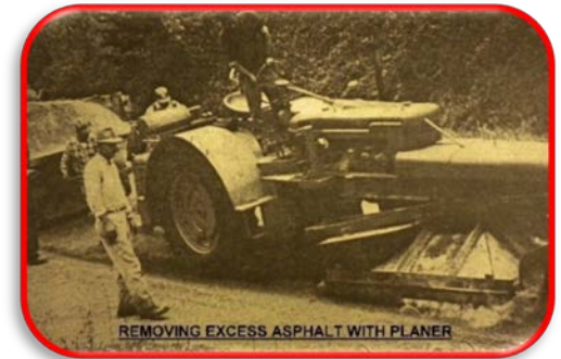
REMOVING EXCESS ASPHALT WITH A PLANER
