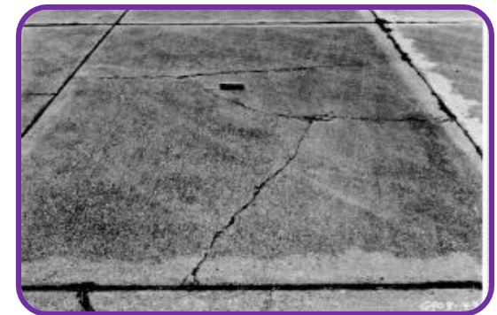
Medium-severity intersecting cracks 85
