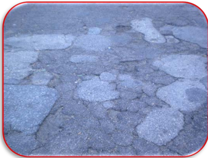
Irregularities in the asphalt surface
