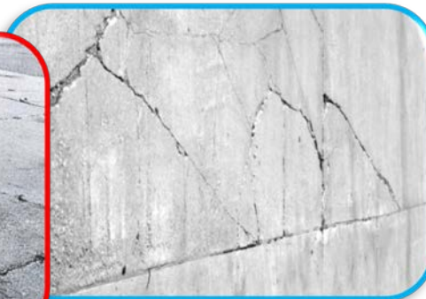
Shattered slab
