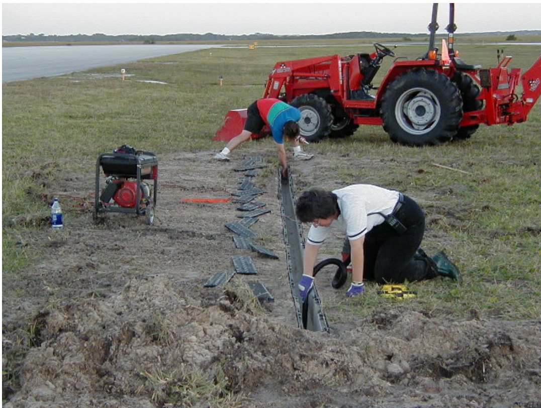
Figure 7 - Trench Drain Installation for an Overland Flow BMP Site
